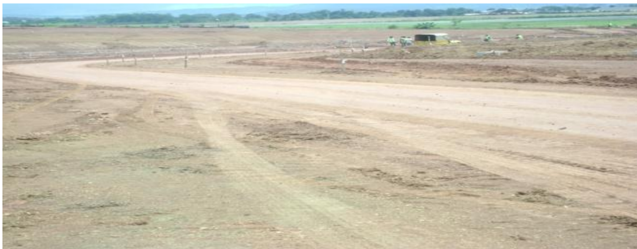
Picture 6: Runway Extension/ Resurfacing work at Enugu Airport
