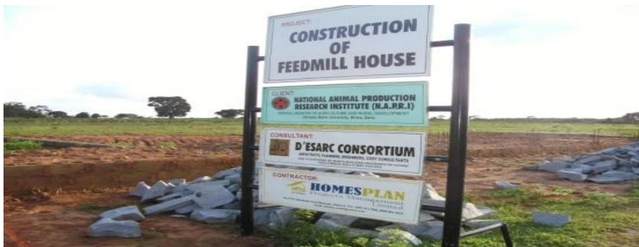
Picture 9: On-going construction of Feed mill House at NAPRI, Ibadan v.
