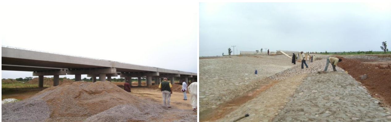
Picture 4: Stone base works in progress at the Wudil Bypass
