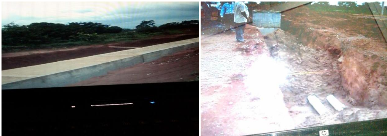
Picture 2: Underground water drainage / underground Foul Sewer
