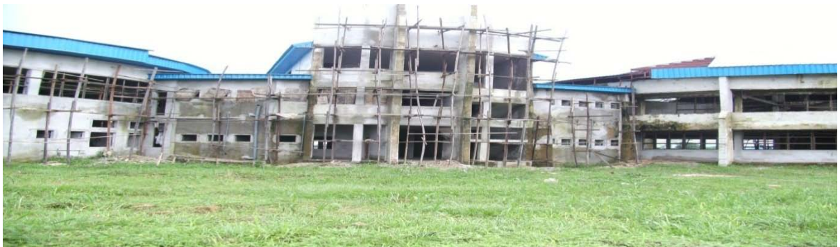
Picture 4.12: Construction of 1000 -Seat Auditorium at Maritime Academy, Oron
