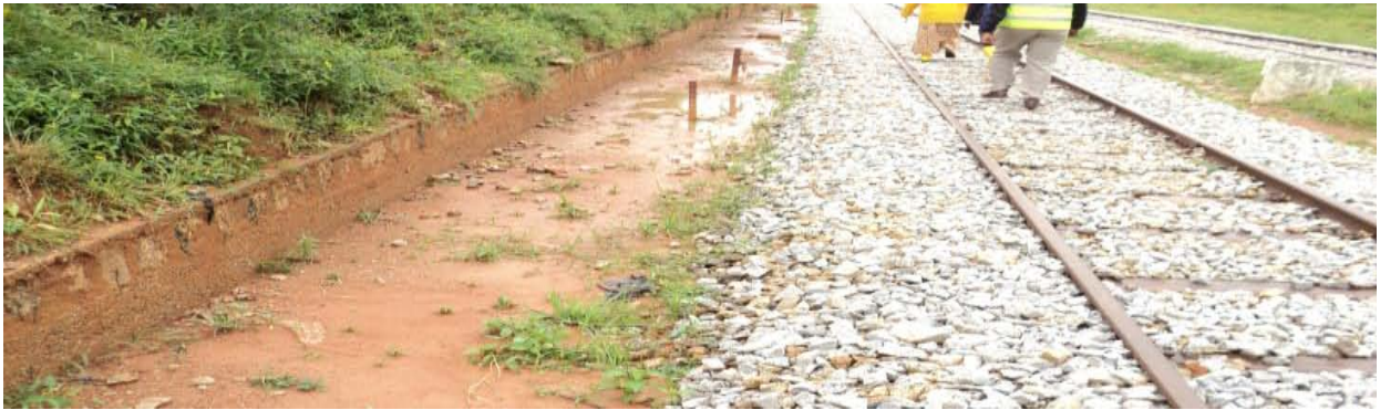
Picture 4.11(a): Re-ballasted portion of the rail line with embankment works at Km96
