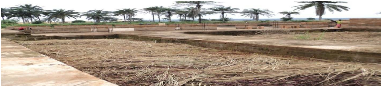
Picture 4.41: Ongoing-going construction of school of education
