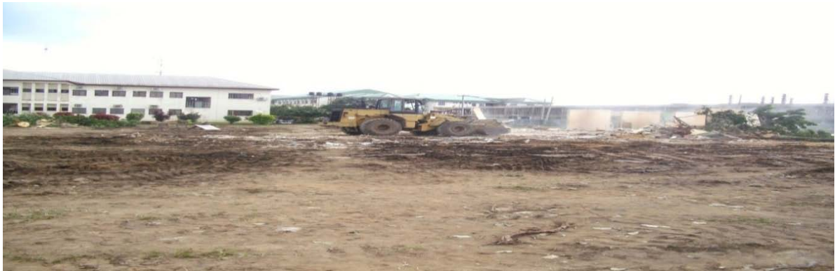
Picture 4.37: Construction of Pharmacy Building Phase 2 (Lecture Hall) at Uni-Port
