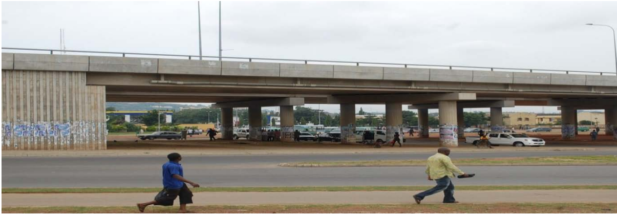
Picture 4.2: Completed Flyover Bridge at AYA – Asokoro, Abuja
