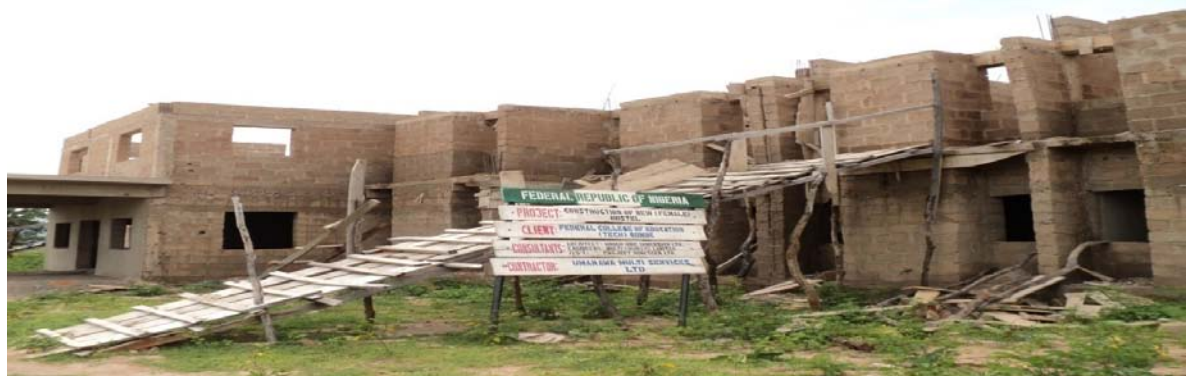
Picture 4.34: Construction of Female Hostel at FCE, Gombe
