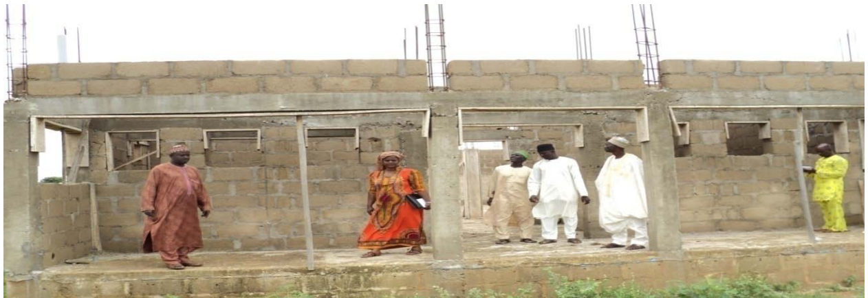
Picture 4.31(b): Construction of Male hostel which was stalled at the Project site
