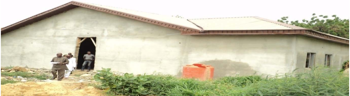
Picture 4.24: Construction of Brachytherapy Block
