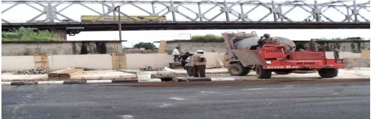
Picture 4.15(a): Ongoing construction of block wall
