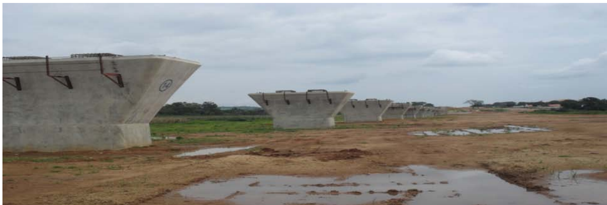
Picture 4.17: Erected T- beams along the rail track bridge.
