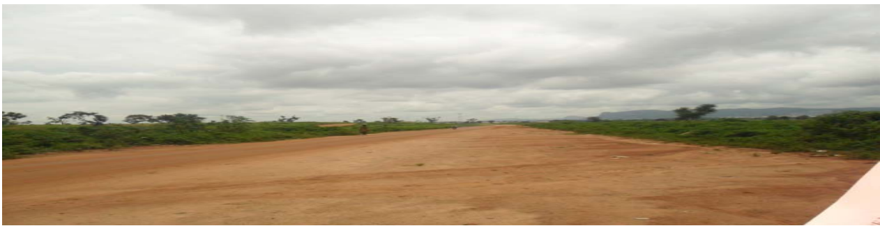
Picture 4.3(b): On-going removal of topsoil at the project site
