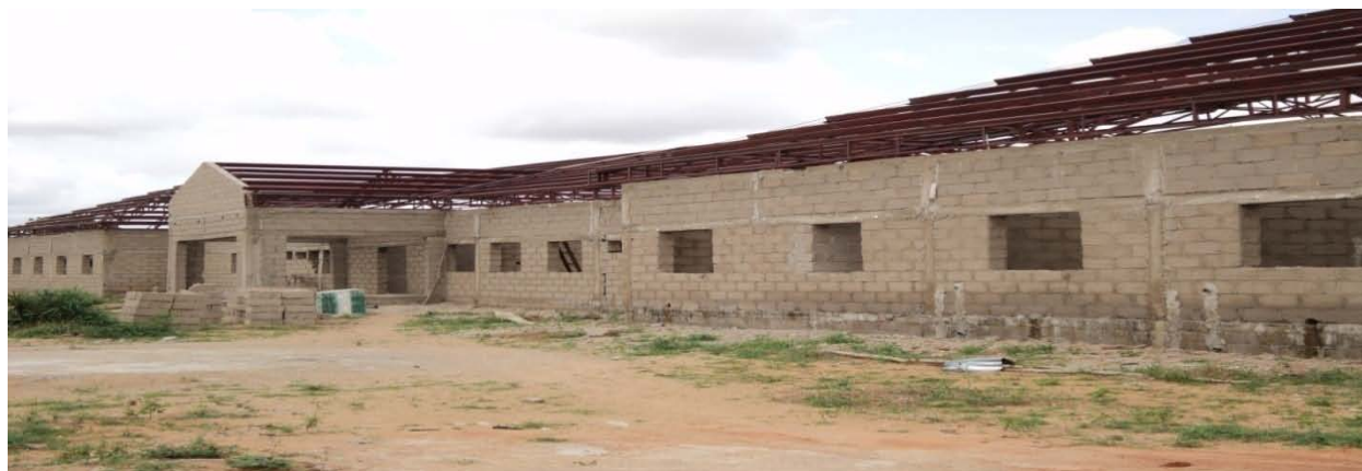
Picture 4.27: Ongoing-going construction of Pediatric complex at FMC, Azare
