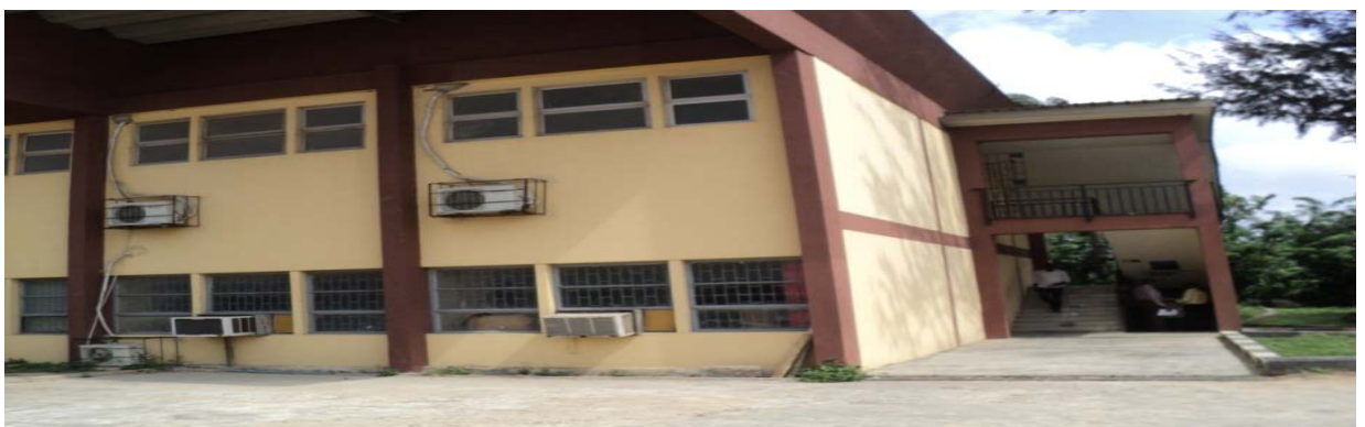
Picture 4.40: One of the Rehabilitated Academic Building at the Main Campus, University of Lagos
