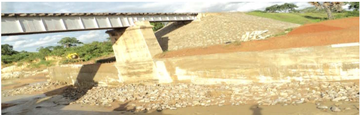
Picture 4.11(a): Re-ballasted portion of the rail line with embankment works at Km96
