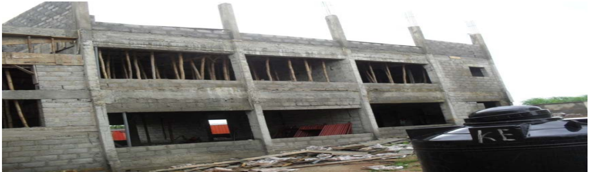
Picture 4.22: Ongoing-going work at the Climate Research Centre
