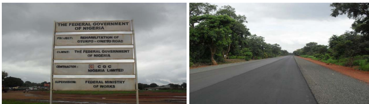
Picture 4.8: A portion of the asphalted binder course at Otukpo – Oweto road project
