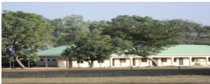
Picture 12: Renovated Staff Quarters at NITT, Zaria
