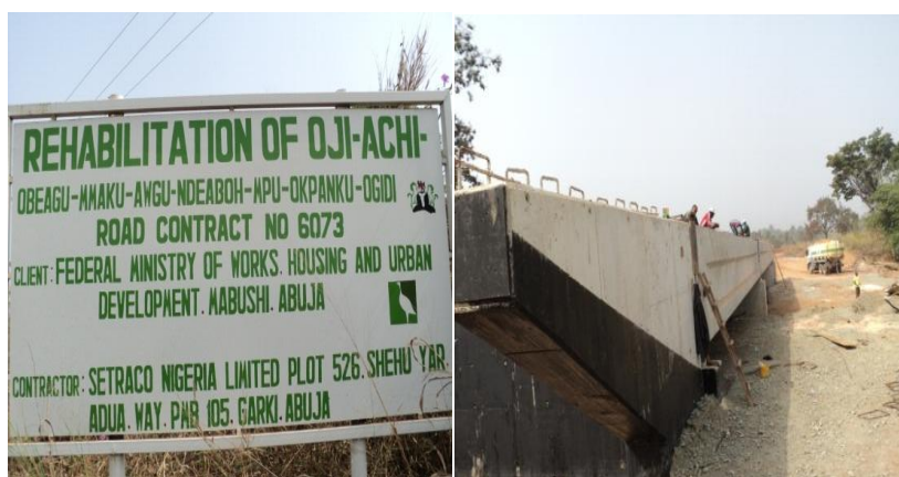
Picture 8: One of the bridges under construction
