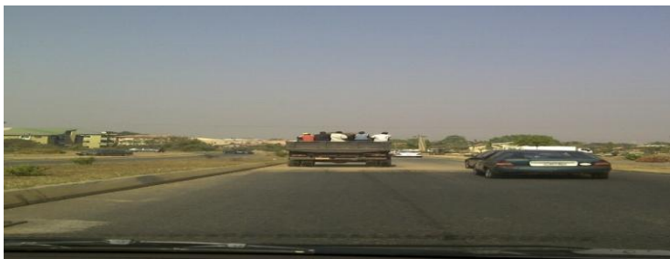
Picture 4: Completed portion of ONEX, Lot 11, Mpape junction.
