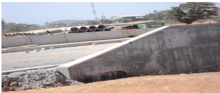
Picture 1: On-going construction of Bridge at Idu Engineering Infrastructure
