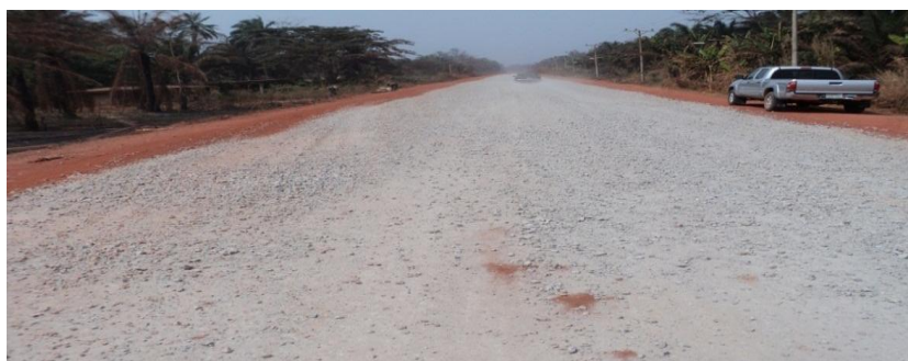
Picture 7: A section of the Nsukka–Obollo–Ikem–Ehamufu–Nkalagu Road under construction
