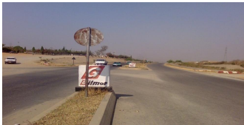
Picture 2: Completed access road at Guzape District Lot 11, Abuja
