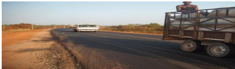
Picture 5: Asphaltting works in progress at Lafia – Obi – Awe road
