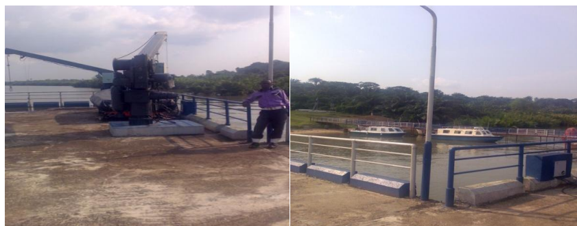
Picture 13: Completed Concrete Jetty & 20-seater Boat for cadet training
