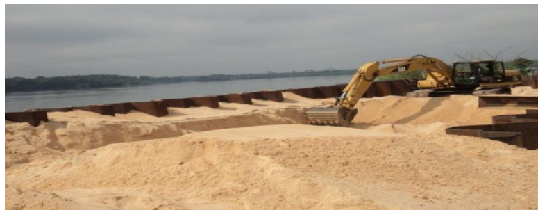
Picture 14 Construction of River Port, Oguta
