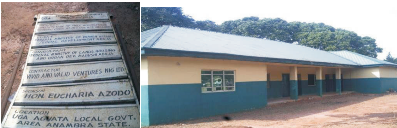
Picture 122: Ongoing renovation/construction of skill acquisition centre, Oye-Uga – Anambra state
