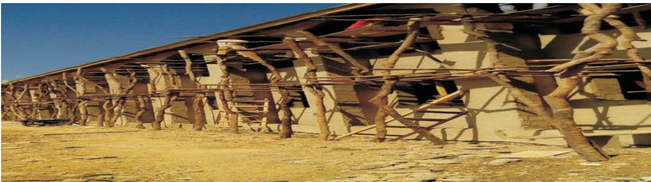
Picture 38: The On-going Construction of Trauma Centre, ATBUTH, Bauchi Main Campus.
