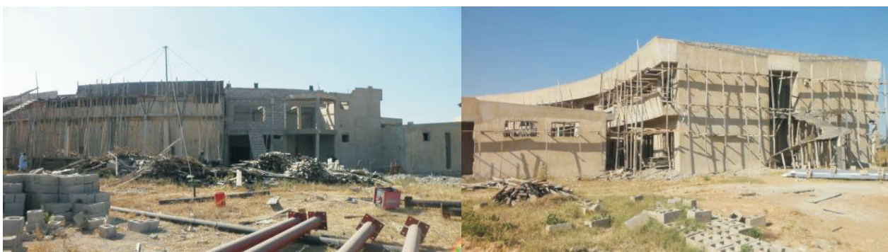
Picture 49: Ongoing completion of International Conference Centre & 40 no chalets
