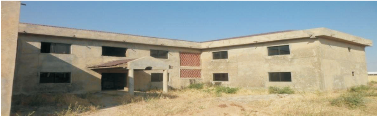
Picture 30: Ongoing construction of Katsina state Command
