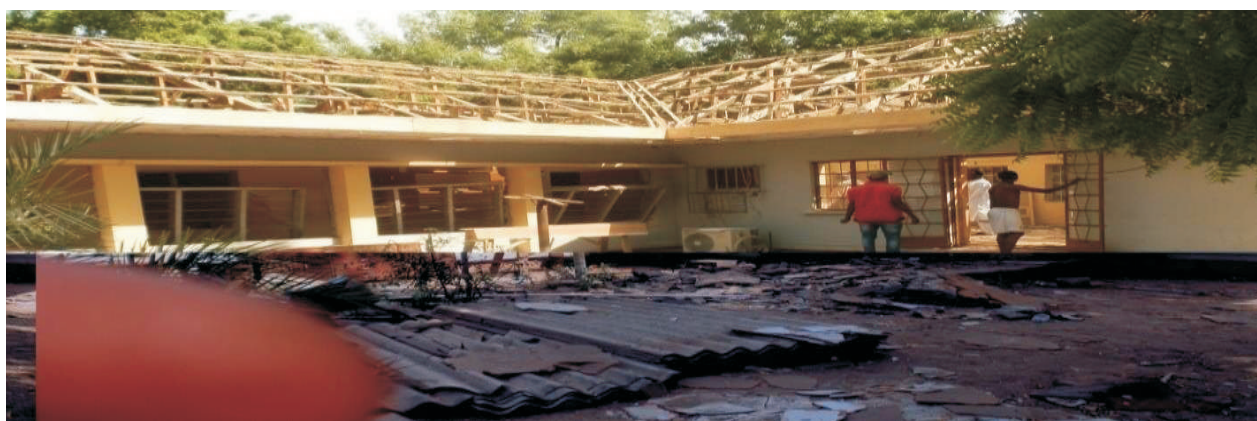
Picture 48: On-going rehabilitation/renovation of Staff quarters at University of Maiduguri
