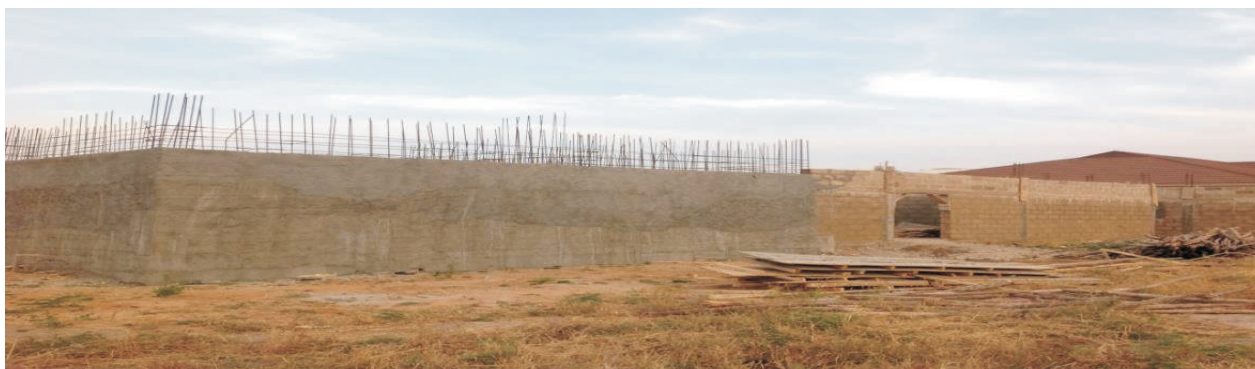
Picture 39: ongoing construction of Nuclear medicine phase II
