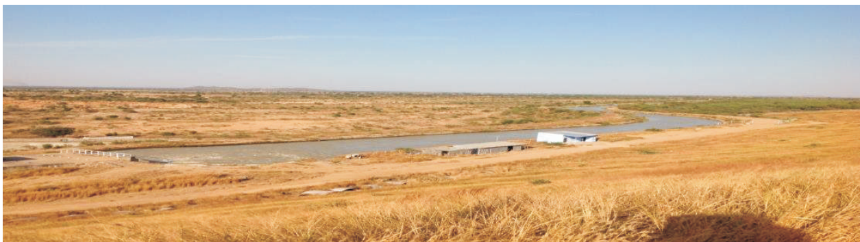
Picture 37: upstream and downstream dam cleared of weeds at Tiga Dam, Kano
