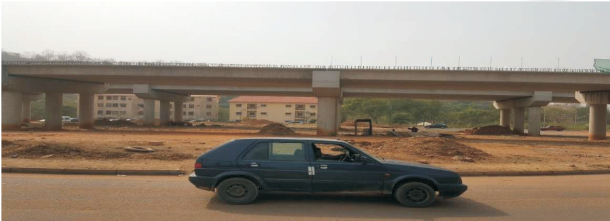
Picture: On-going bridge work at Villa roundabout (OSEX)
