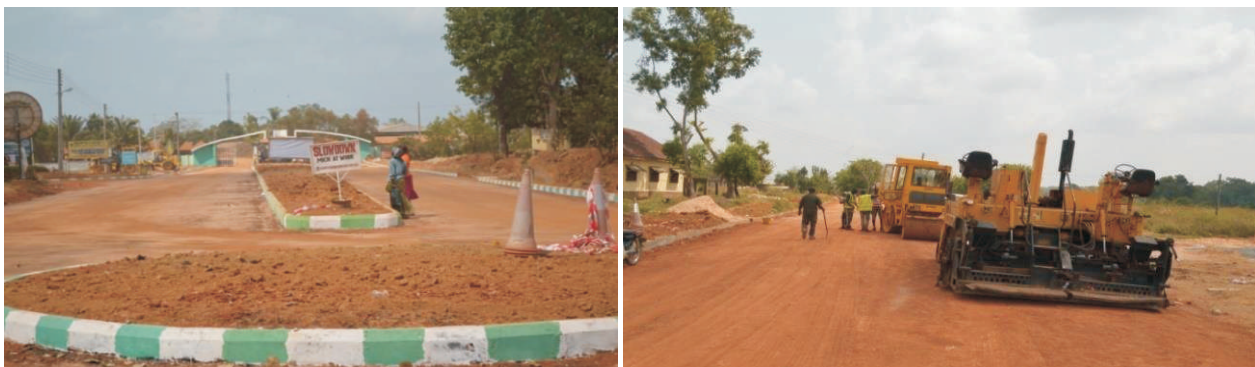
Picture 25: A portion of the completed earthworks and kerbs around the college entrance gate
