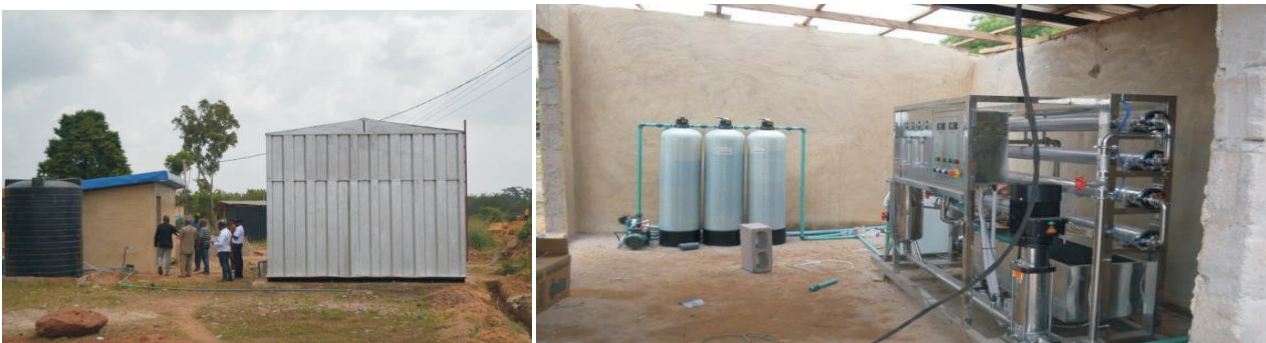
Picture 24: Completed Water Treatment Plant and Reservoir at the project site
