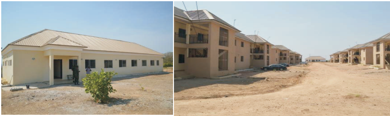
Picture 33: Completed Search & Rescue Company and Staff quarters at the Guards Batallion, Gwagwalada – Abuja.
