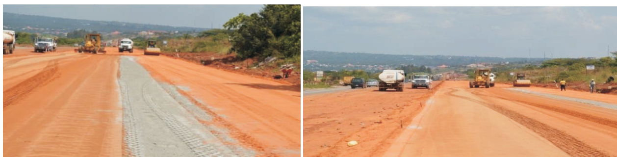
Picture 9: Ongoing cement stabilization works at the Enugu – Onitsha road
