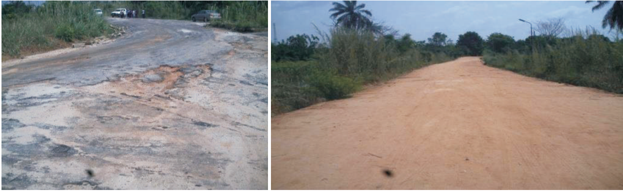
Picture 118: Part of the erosion ravaged road and the on-going earthworks/sand filling at the project site.
