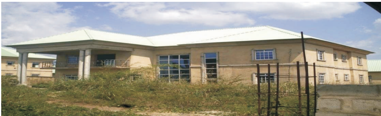
Picture 50: Ongoing construction of the Vice Chancellor’s lodge at the University
