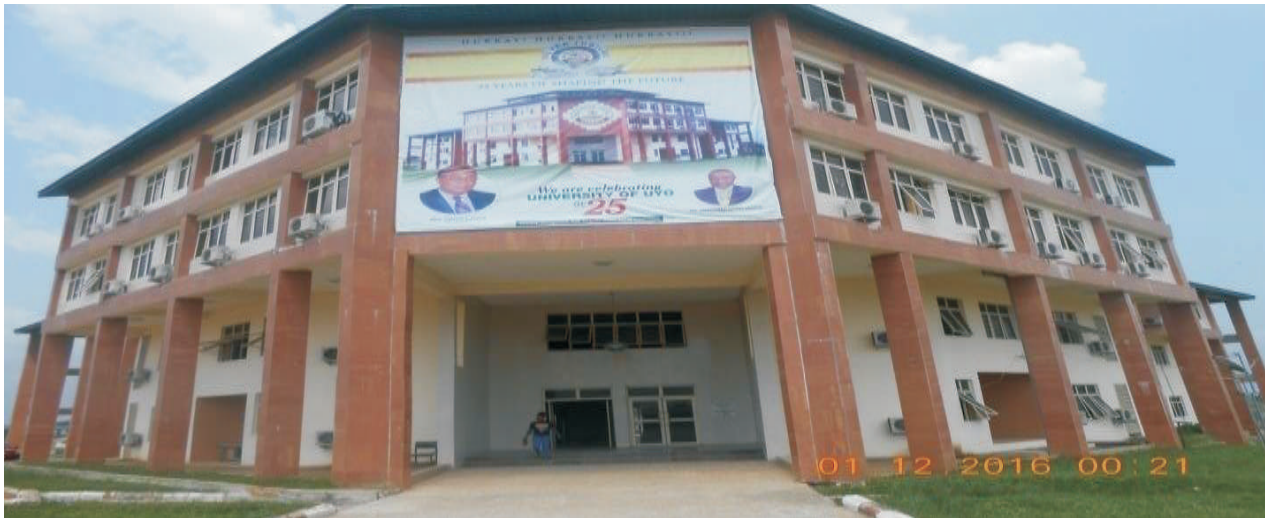
Picture 46: Completed Central Administrative Building at University of Uyo
