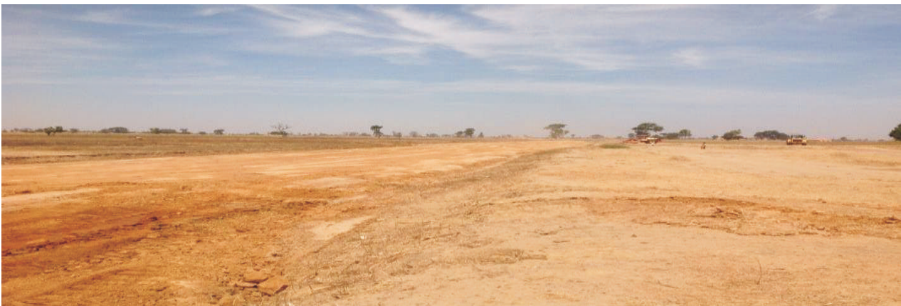
Picture 23: Ongoing construction of embankment at Jare Earth Dam, Katsina State
