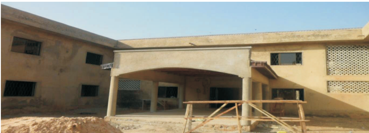
Picture 29: Ongoing construction of Kano state Command
