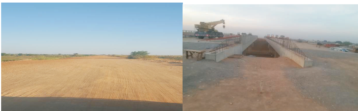
Picture 10: Ongoing road construction works at Kano Western By-Pass
