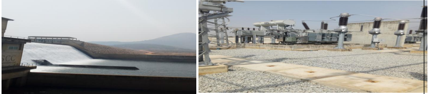
Picture26: The Completed Kashimbilla Dam and Hydro Power Station at Taraba State
