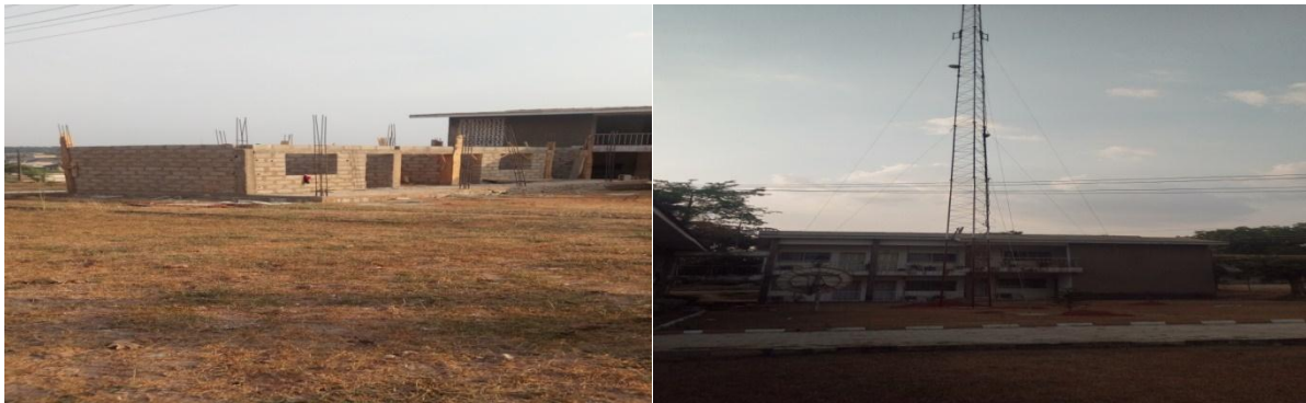
Picture 55: Ongoing Rehabilitation/Upgrading of Central Library Building and Internet facility at Forest Research Institute of Nigeria
