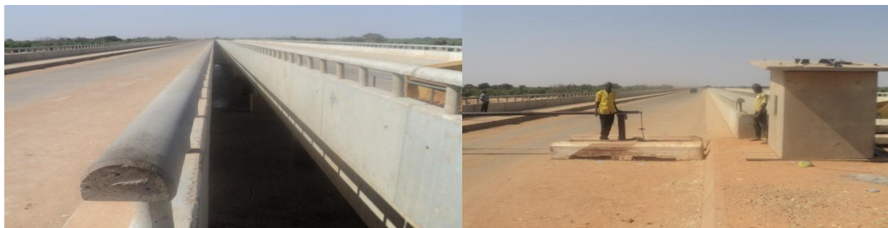
Picture 18: Completed Bridge No.1 at Kano-Wudil-Shuarin Road Project
