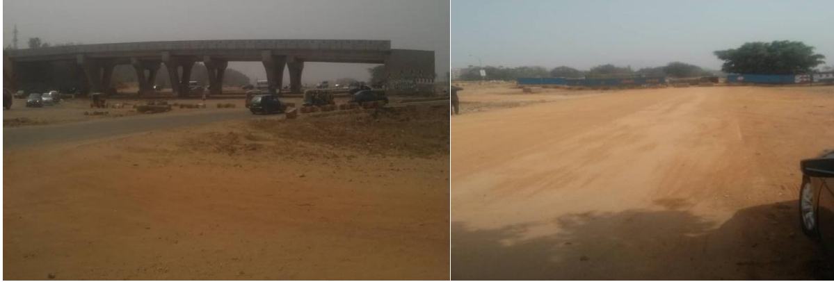
Picture 43: Ongoing Works At the Apo Bridge and Old CBN Sections of the Project
