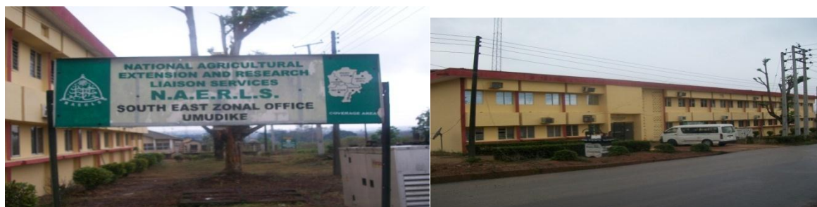
Picture5: The Renovated National Agricultural Extension and Research Service (NAERC) Complex Building at NRCRI, Umudike.
