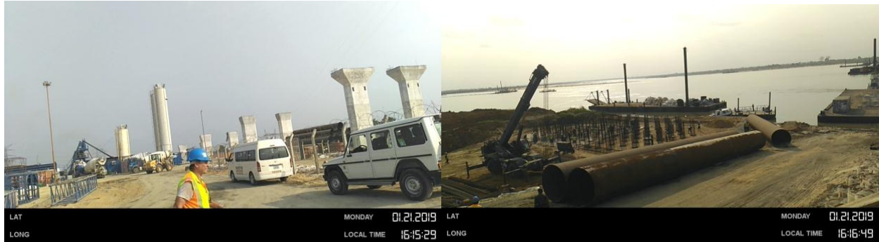
Picture 21: Construction of 2 nd Niger Bridge in progress at the Project Site
