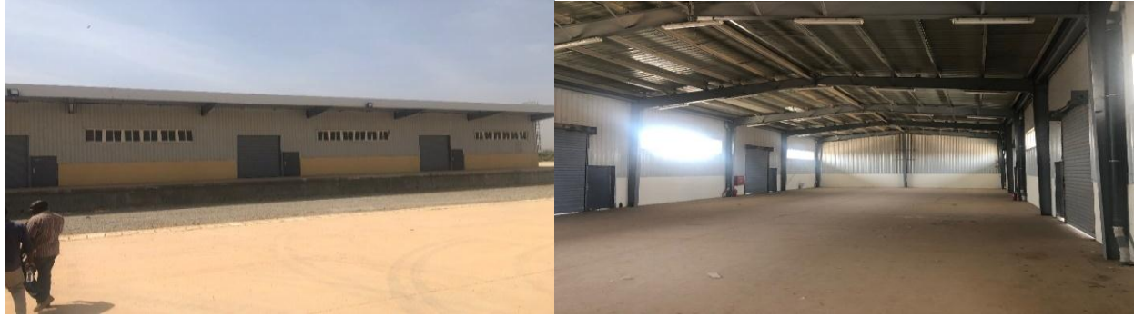
Picture 28: Completed Cargo Building at Idu-Kaduna Rail Project
