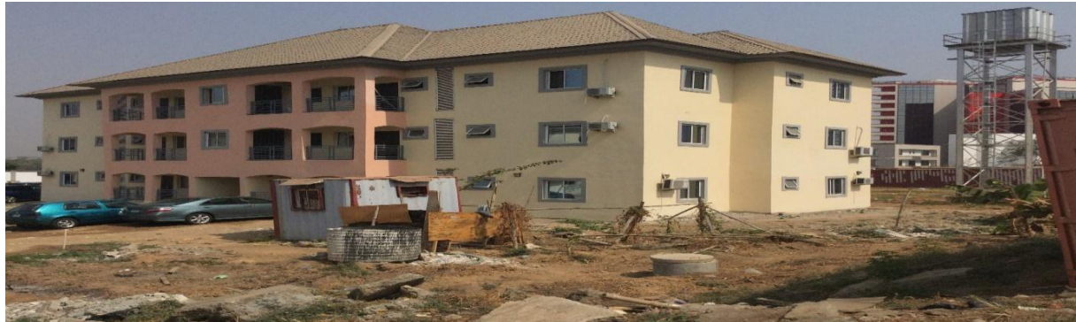
Picture 33: Completed and Furnished 1Unit Block of 6Nos.3 Bedroom Flats Doctors' Quarters at FMC, Jabi
