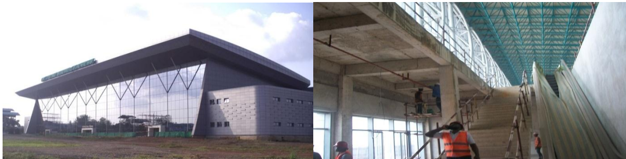
Picture 30: Ongoing Construction of New Terminal Building at Enugu Airport
