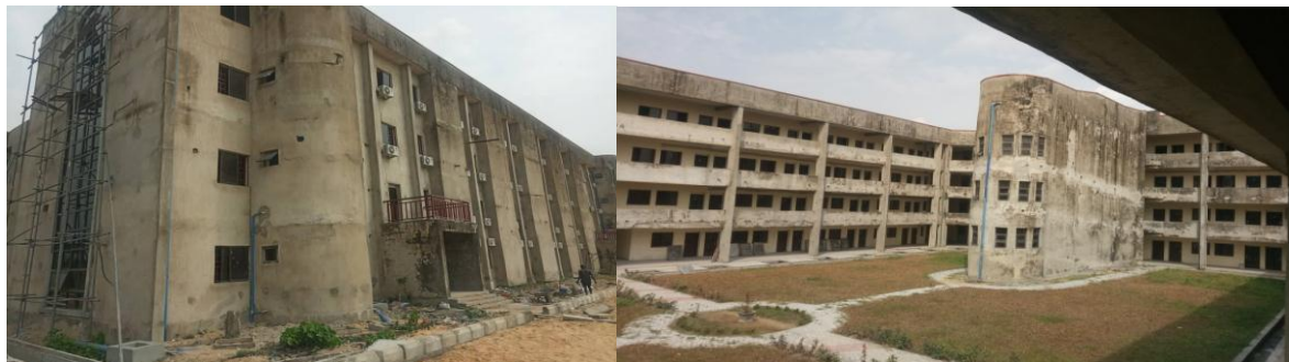
Picture 23: Ongoing Construction of Federal Secretariat Complex, Yenagoa, Bayelsa State
