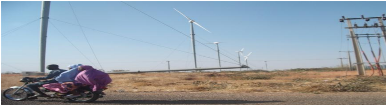
Picture 13: Part of the Installed Turbines at Katsina Wind Farm
