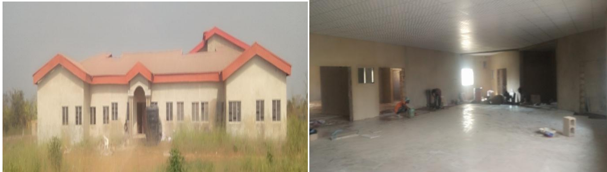
Picture 36: On-going Construction of Cardiac Centre at OAUTH, Ile-Ife
