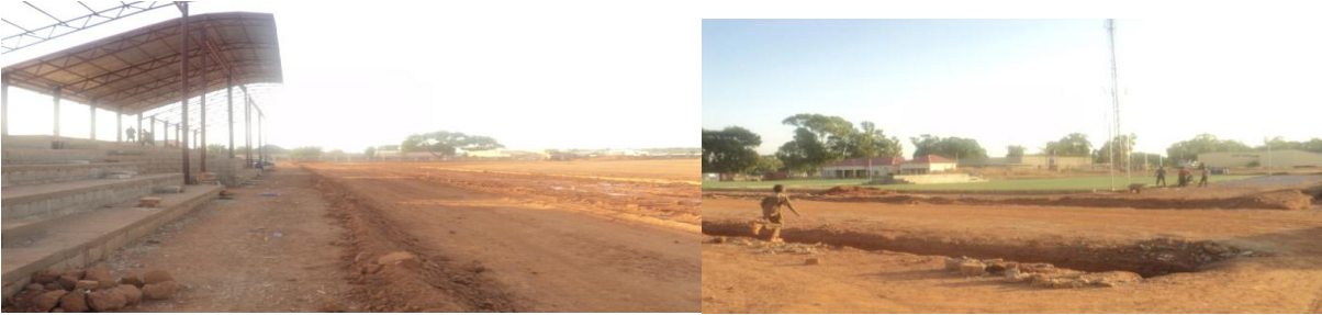
Picture 7: Ongoing Construction of Sport Complex at Armed Forces Command & Staff College, Jaji
