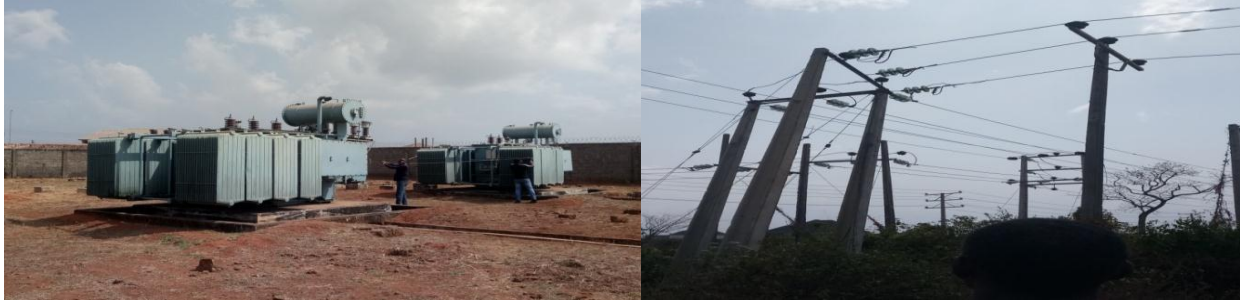
Picture 14: Ongoing Construction & Installation of 10KM of 33/11KV Lines and Associated 2x15MVA Injection Substation, Ibuzor, Delta State
