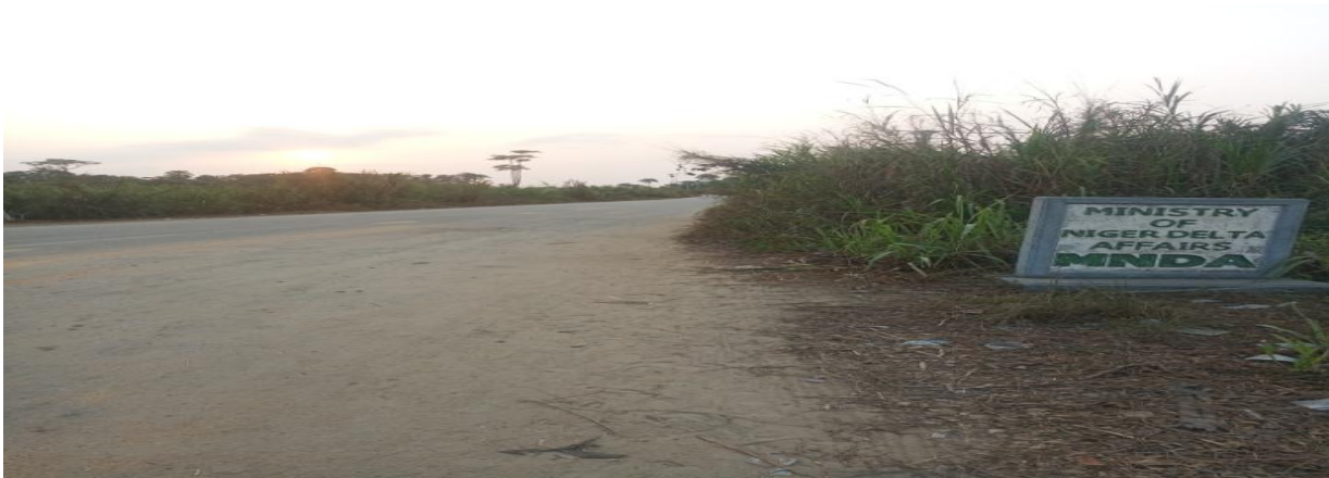
Picture 54: Ongoing Construction of Gberegolor-Ogriagbene Road, Delta State
