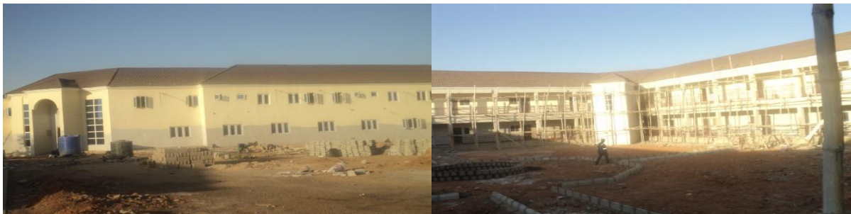
Picture 6: Exterior and Interior views of the 40Nos of 1-Bedroom Building in progress at Armed Forces Command & Staff College, Jaji
