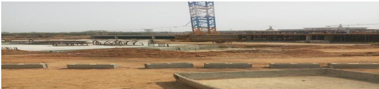
Picture 9: Ongoing Construction of Administrative Block at National Defence College Piwoyi
