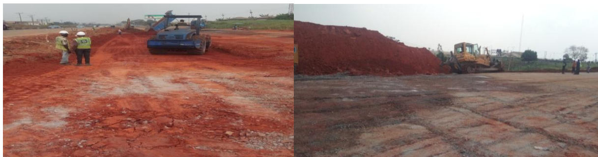
Picture19: On-going Construction of Lagos – Ibadan Expressway Section I
