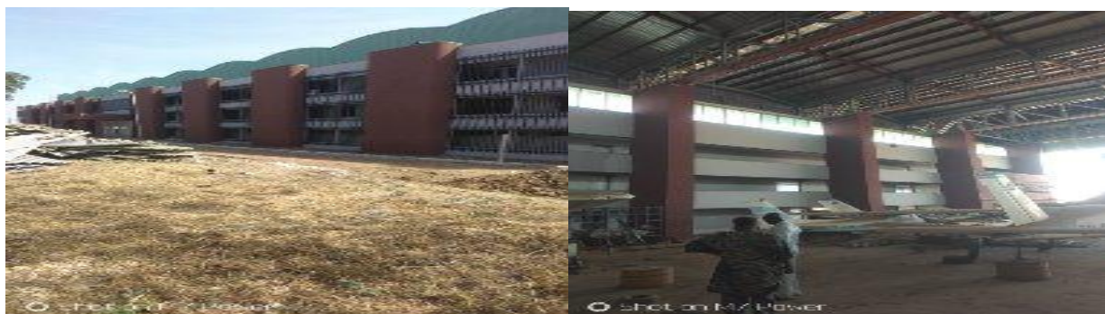
Picture 31: The rehabilitation of Third Hanger in progress at NCAT Zaria.
