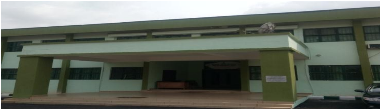
Picture 40: Ongoing Construction of the Faculty of Agriculture at University of Benin
