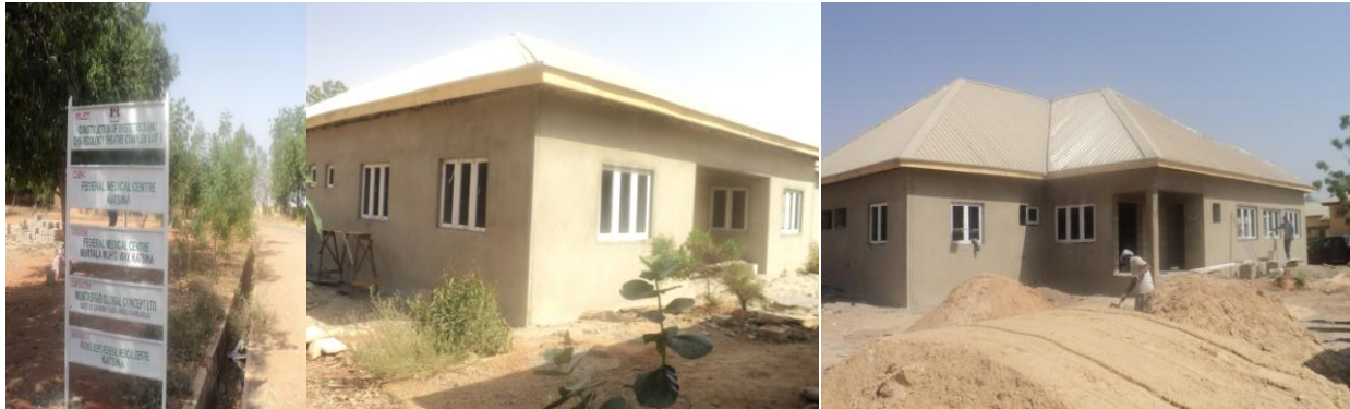
Picture 32: Ongoing Construction of Obstetrics/Gynecology Theatre Complex and a Laboratory at FMC Katsina
