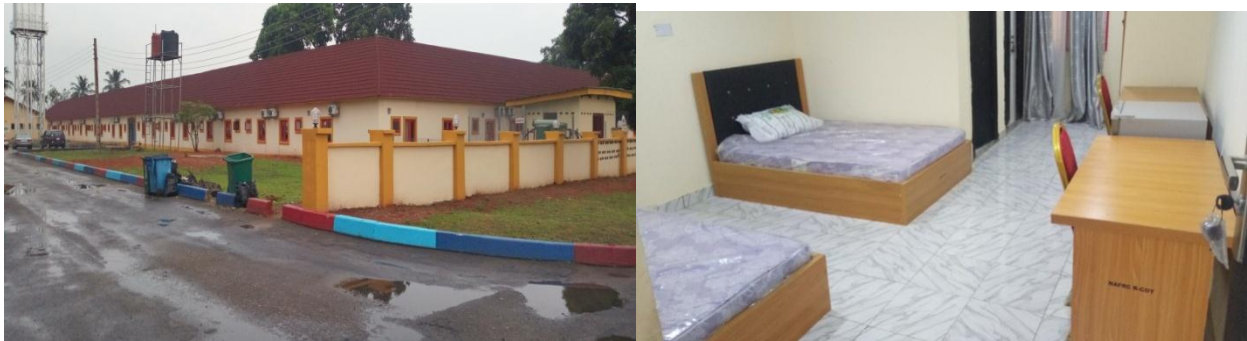
Picture 12: Part of the Construction/Renovation and Furnishing of Trainees Accommodation Coy-B at Armed Forces Resettlement Centre, Lagos
