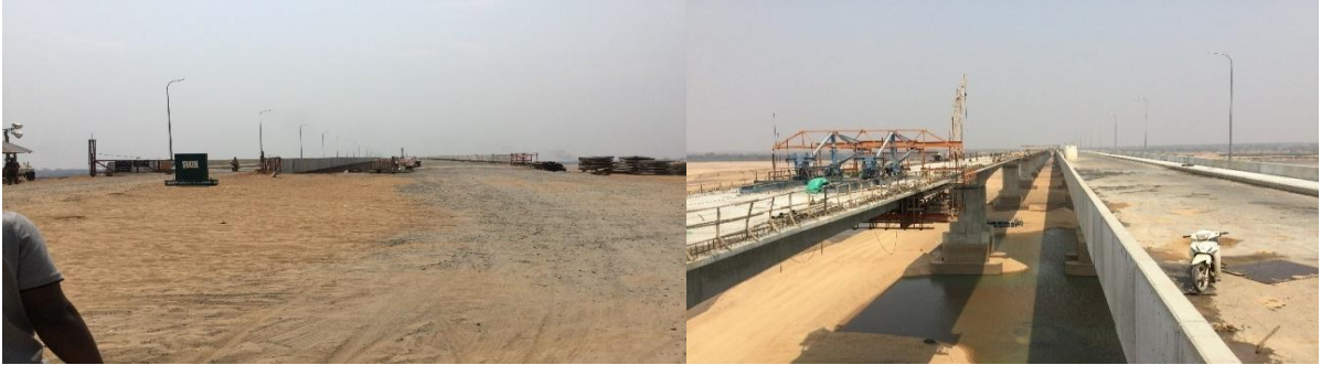
Picture16: Completed Portion & On-Going Construction Work on Loko-Oweto Bridge
