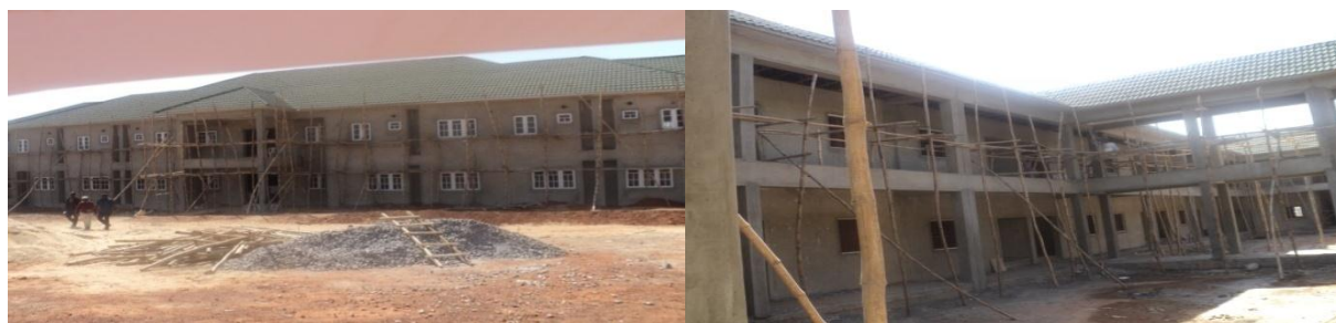
Picture 8: Ongoing Construction of 50-Bedrooms Complex at DICON, Kaduna
