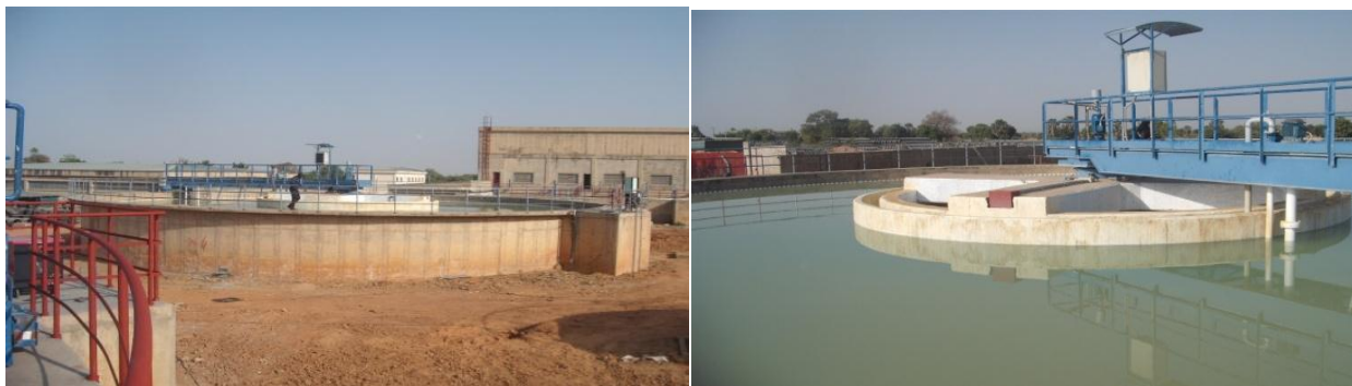
Picture 24: Installed Facilities at Zobe Water Project, Katsina State
