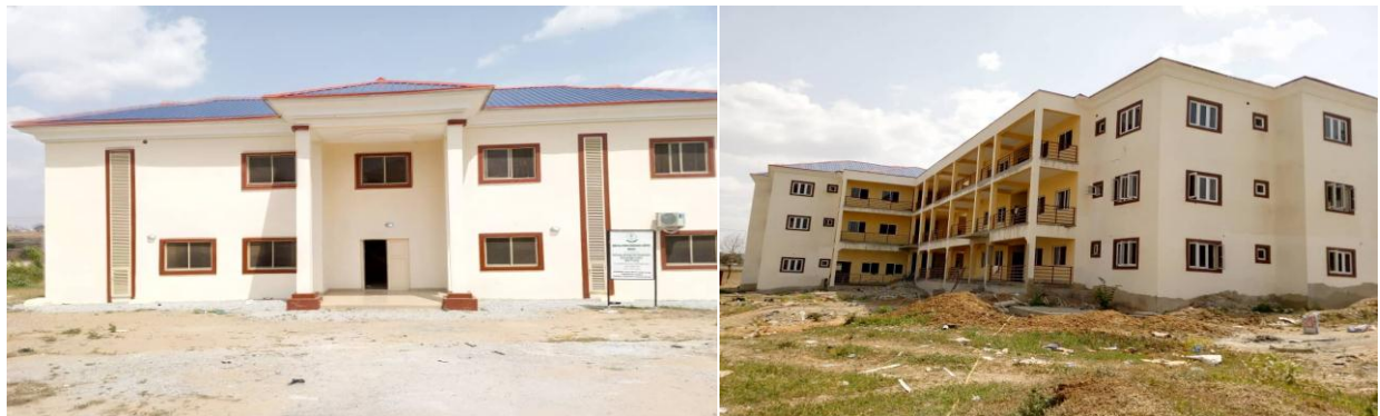
Picture 45: Ongoing Completion of Barracks at NSCDC Sauka, Abuja
