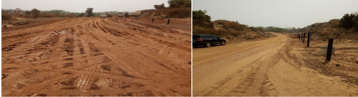
Picture 44: Earthworks in Progress at the Project Site (Guzape Lot II)
