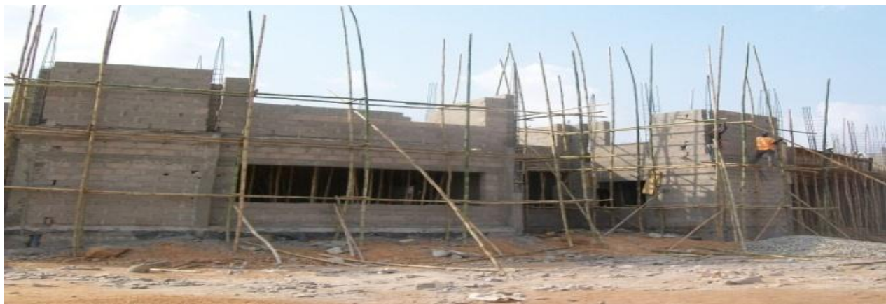
Picture 41: Ongoing Construction of College of Medicine Academic Block
