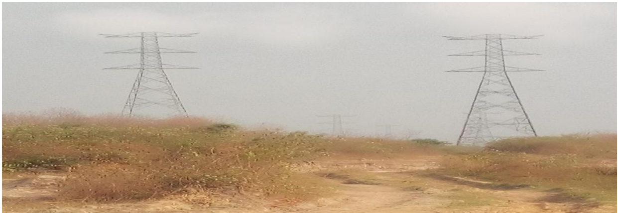
Picture 15: On-Going Installation of Towers for Power Evacuation of the Benin North – Oshogbo 33KV DC Line
