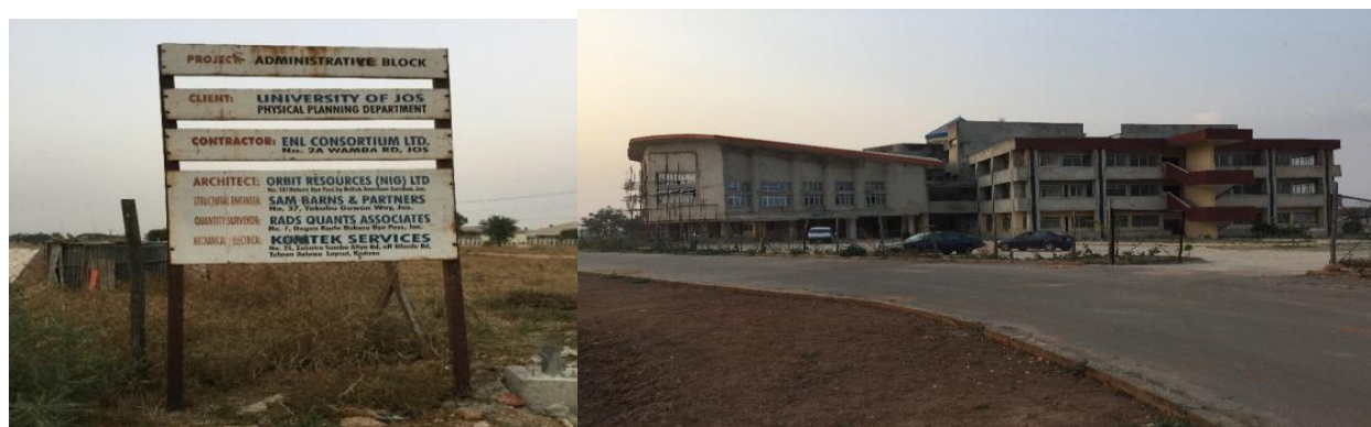
Picture 39: Ongoing Construction of Administrative Block/Senate Chamber at the University of Jos
