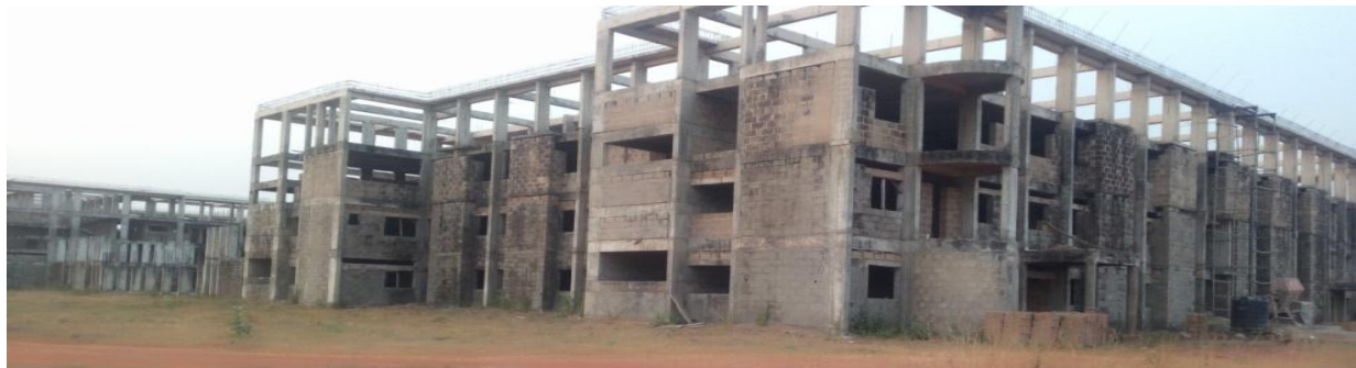
Picture 22: Ongoing Construction of Federal Secretariat, Osgogbo
