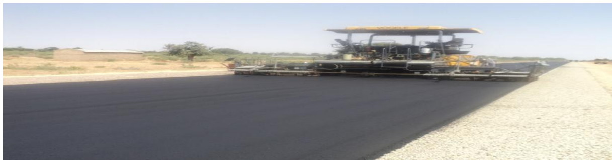
Picture 17: Ongoing Wearing Course at Gamoji and Bakin Ruwa Areas of Kano-Wudil-Shuarin Road
