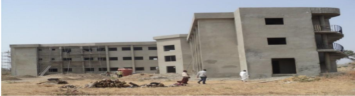
Picture 48: On-Going Completion of Administrative Building at NCPRD, Bauchi
