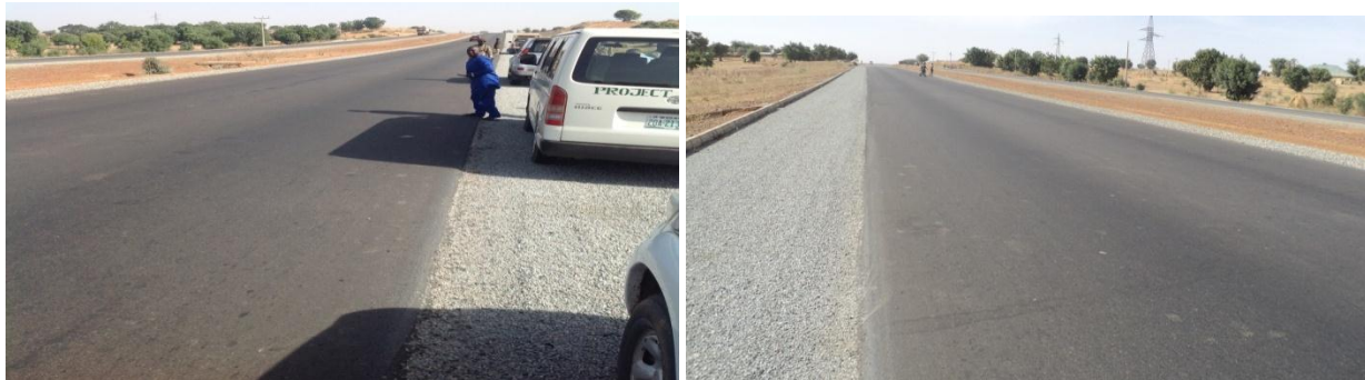
Picture 20: Completed Dualisation of Kano – Maiduguri Road, Section II (Shuwarin-Azare)
