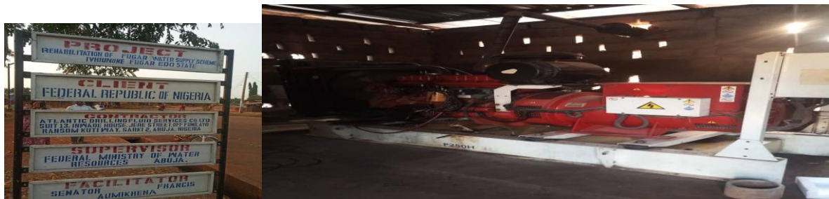
Picture 25: Part of the Rehabilitated Water Works Equipment at Etsako Central LGA, Edo State
