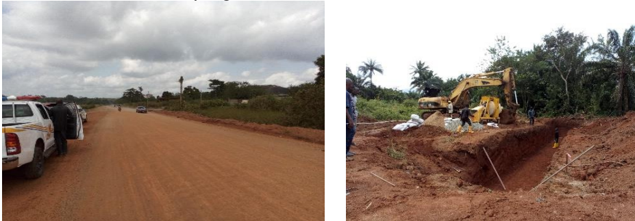
Picture 9: Ongoing palliative and culvert works at the Dualization of Akure – Ado Ekiti road project.
