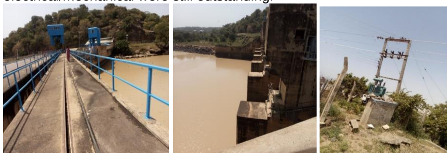
Picture 18: The construction of 90m Left-hand Dyke and Installation of 300KVA Transformer.
