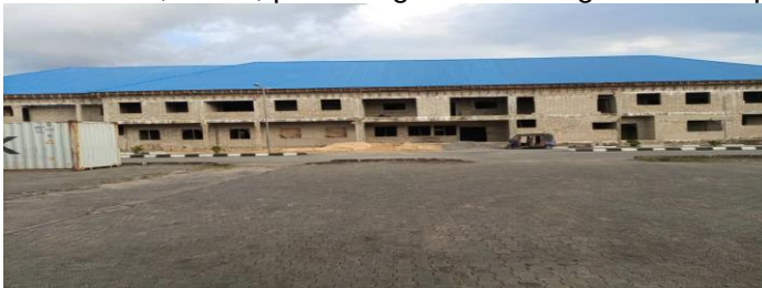
Picture 26: Ongoing construction of six (6) theatre suites facility at FMC, Yenagoa
