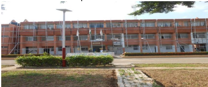
Picture 42: Ongoing remodelling of existing Administrative Building at NITT, Zaria
