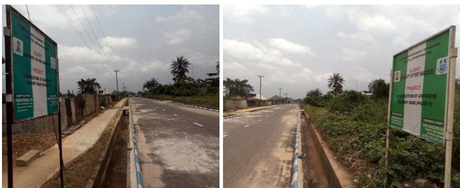
Picture 58: Completed Access Road (Phase I) and Ongoing Drainage Works (Phase II) at Ashgroove Academy of University of Port Harcourt
