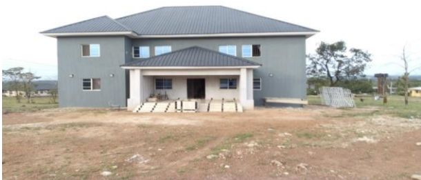
Picture 6: Completed construction of Student Resource Centre, at Federal Cooperative College, Orji – River.
