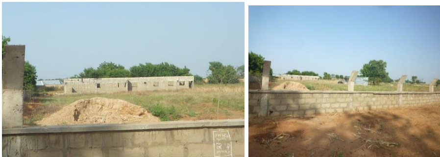
Picture 21: Ongoing construction of Poultry Building and Fencing at SRRBDA
