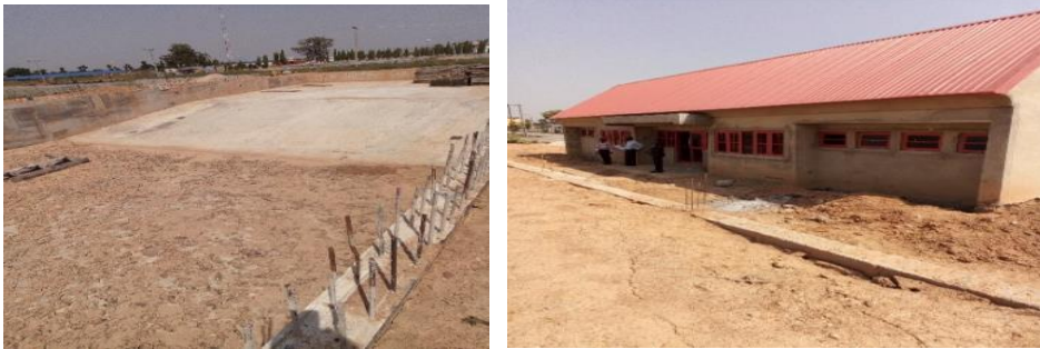
Picture 74: Ongoing Construction of Swimming Pool and a Pool House at FFS, Abuja
