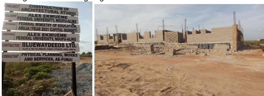
Picture 61: Ongoing Construction of Architectural Studio at Alex Ekweme Federal University, Ndufu-Alike, Abakaliki
