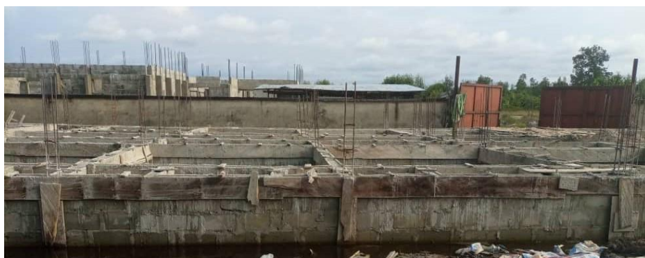
Picture 59: Ongoing Construction of Male Hostel at Nigeria Maritime University, Okerenkoko
