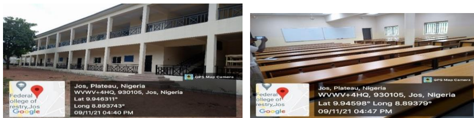
Picture 63: The Completed Building at College of Forestry, Jos
