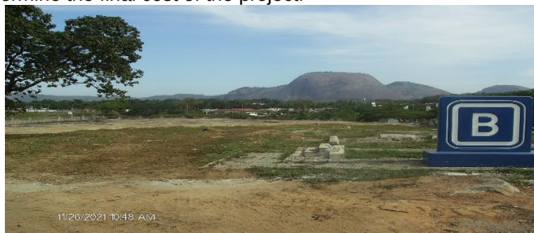
Picture 73: Ongoing Works at the VIP Clinic, State House - Abuja
