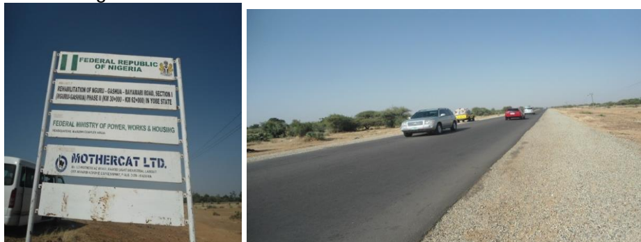
Picture 13: The completed portion of the Nguru-Gashua-Bayamari Road, Section I Phase II in Yobe State
