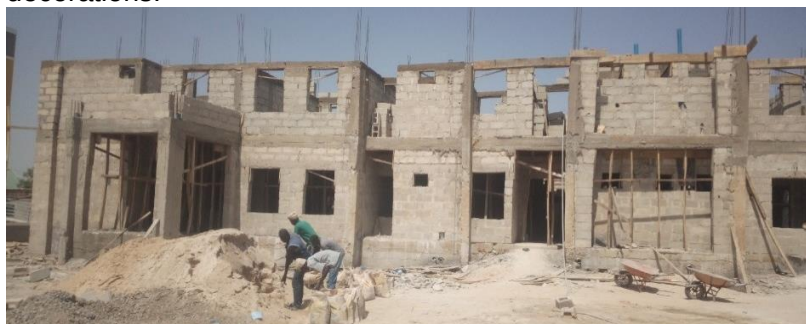
Picture 32: Ongoing Construction of Male & Female Drug Rehabilitation Ward at (FNPH), Maiduguri.
