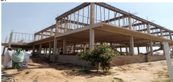
Picture 7: The ongoing construction of the Administrative Block at Federal College of Horticulture Dadin Kowa
