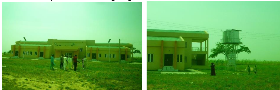
Picture 55: Ongoing Construction of Visiting Scholar Transit Camp at
