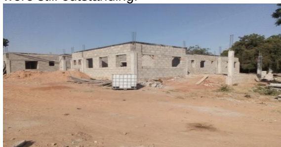
Picture 28: Ongoing Construction of Isolation Centre at Federal Teaching
