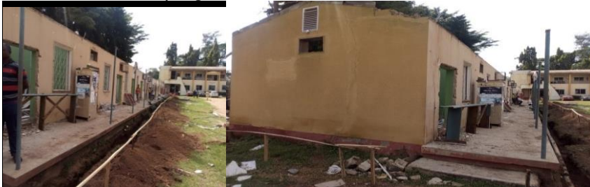
Pictures 60: On-going Rehabilitation/Construction of Computer Laboratory
