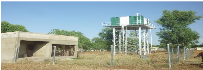
Picture 22: The Ongoing Water Project at SRRBDA, Sokoto
