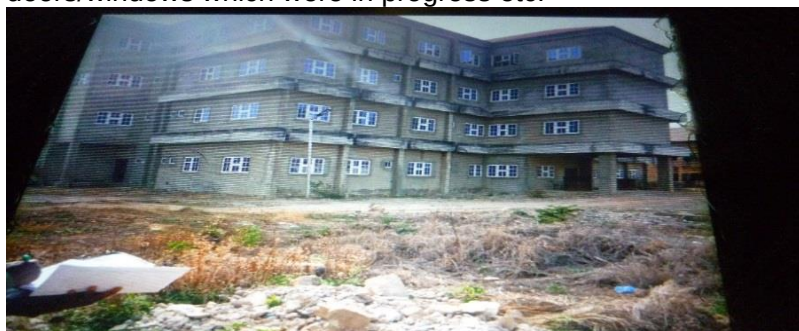
Picture 75: Ongoing Construction of Computer Aided Design Multipurpose Hall in Headquarter, Kaduna
