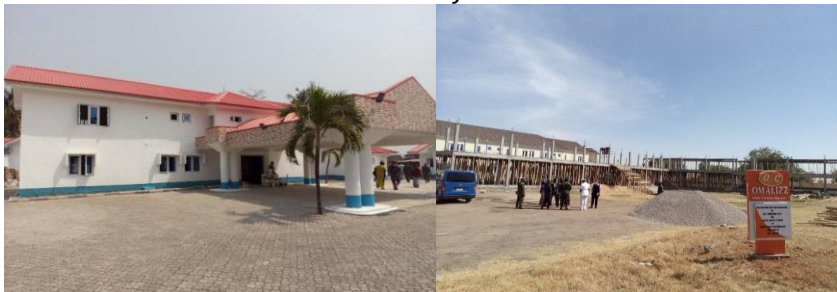
Picture 37: Completed Renovation of Air House at Ikoyi Lagos and Ongoing Construction and Furnishing of 30 x 1-Bedroom Flat for JC Students at Jaji, Kaduna state.
