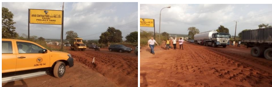
Picture 11: Ongoing rehabilitation of Old Enugu-Onitsha Road at Orji River, Enugu State
