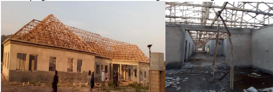
Picture 80: Ongoing Construction and Furnishing of Administrative Block and Conference Hall at NIOMCO
