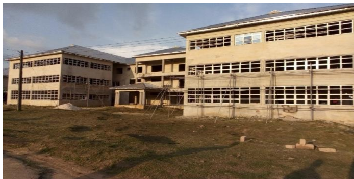
Picture 34: Ongoing Construction of 2 Storey Laboratory Building (Phase I)
