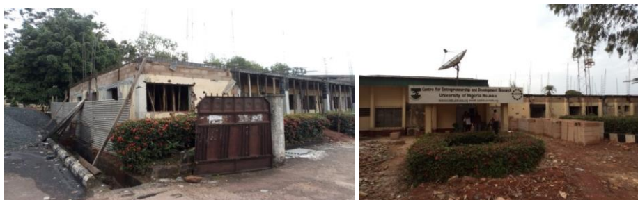
Picture 62: Ongoing Remodelling of Centre for Entrepreneurship and Development Research Centre at University of Nigeria, Nsukka
