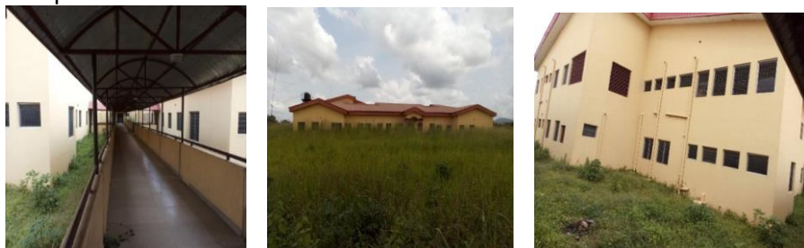
Picture 23: Ongoing construction of Cardiac Center at OAUTH, Ile – Ife.
