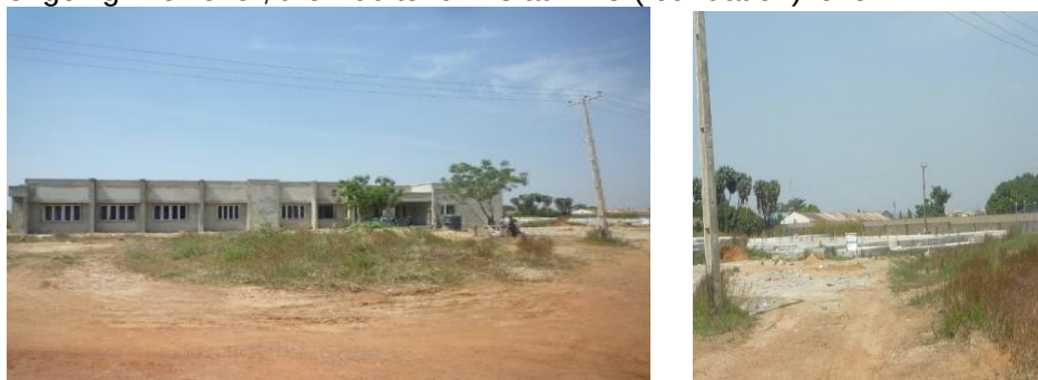
Picture 41: The Ongoing Construction of Library Hall and Auditorium Building at DICON, Kaduna
