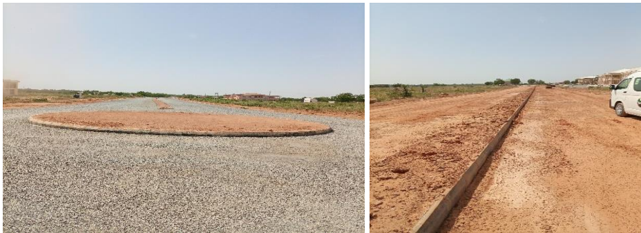
Picture 56: Ongoing dualization road at FCE, Katsina
