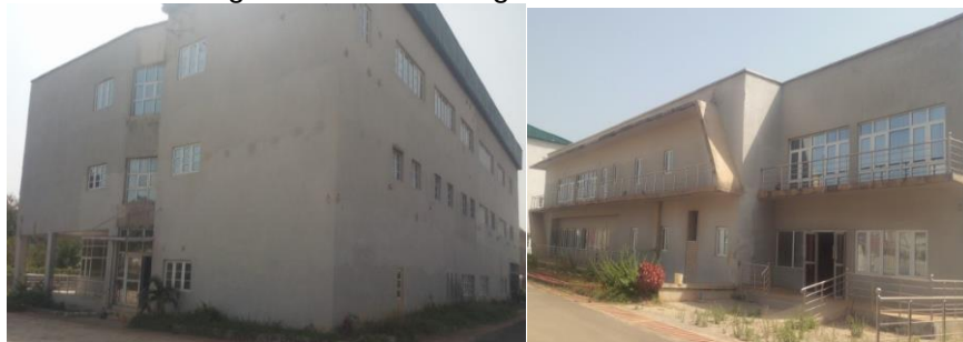
Picture 43: The completed Administrative Block and a Training Institute in Abuja
