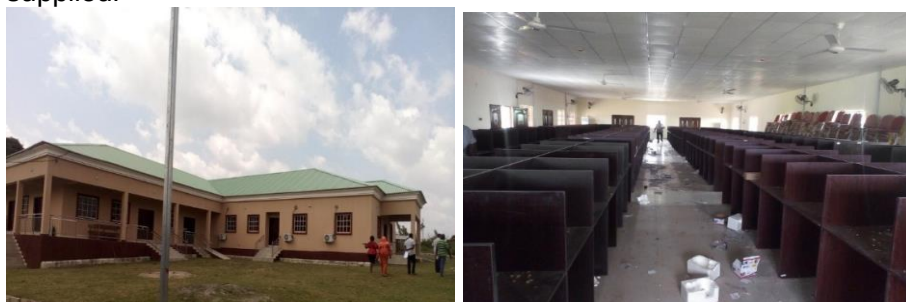
Pictures 64: Construction and Equipping of 250 Sitters Computer Laboratory nearly completed at Federal College of Forestry, Ibadan
