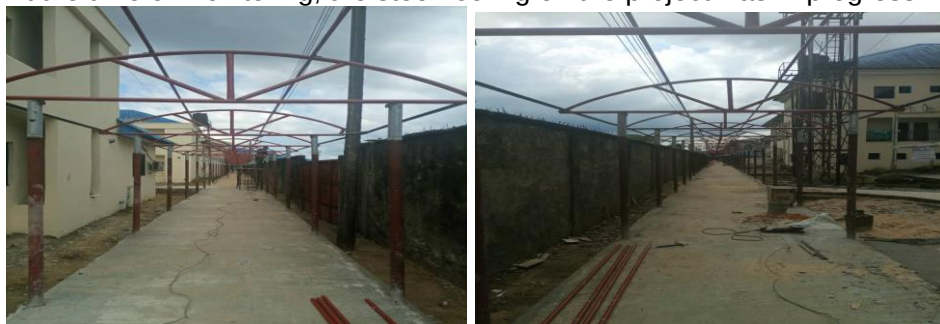
Pictures 27: On-going construction of gangways at the FMC, Yenagoa.
