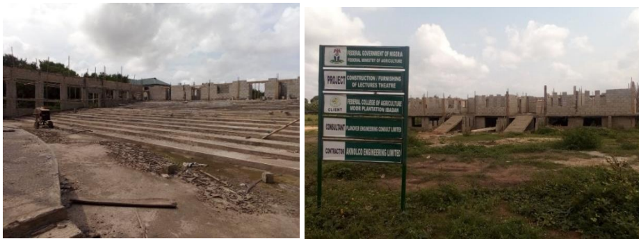
Picture 1: On-going construction of Lecture Theatre at Federal College of Agriculture, Ibadan
