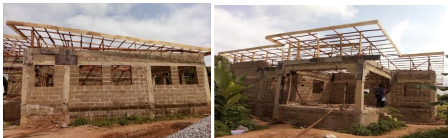
Picture 2: On-going construction of Modern Audio-Visual Building/Printing Press at Federal College of Agriculture, Ibadan.
