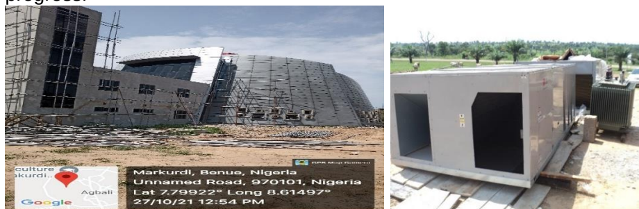
Picture 3: Ongoing Construction of Senate chamber at the University of Agriculture, Makurdi
