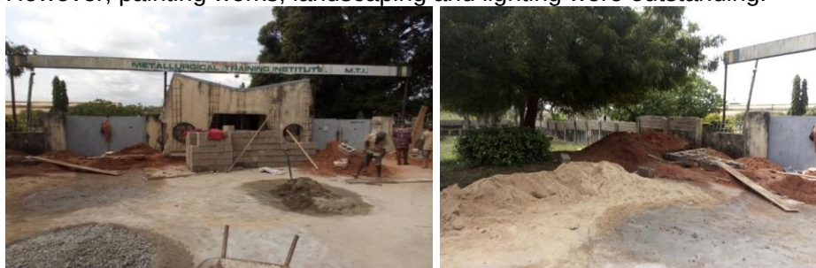
Picture 78: Ongoing Reconstruction of the Institute's Main Gate House and Perimeter Fencing at Metallurgical Training Institute, Onitsha
