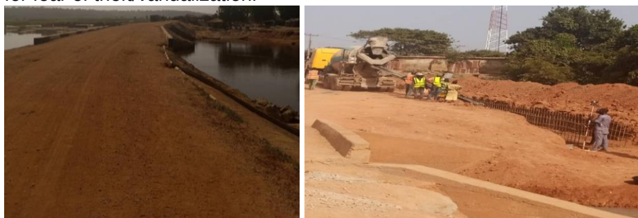
Picture 20: Ongoing Construction of Drainages and Dyke at the Tada - Shonga Irrigation Project.
