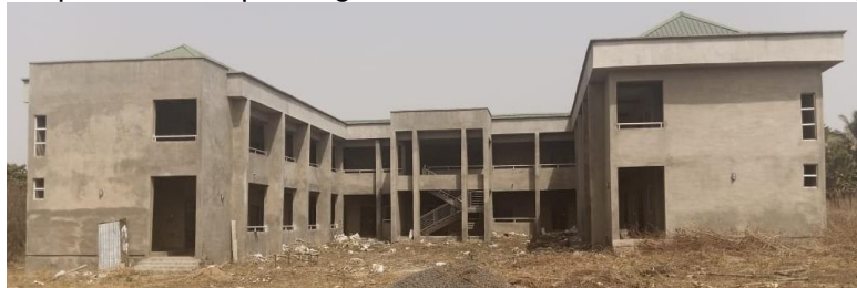
Picture 67: The ongoing Construction of Office Building at the Michael Imodu Institute of Labour Studies Ilorin, Kwara State
