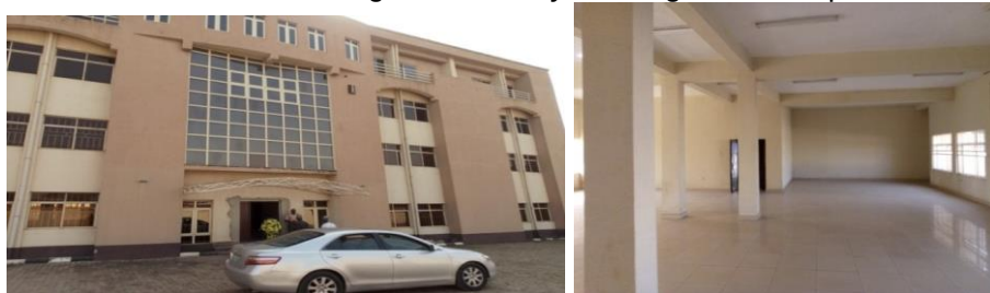
Picture 72: The Procured Office Accommodation Building for (NEITI), at Idu–Industrial Layout, Abuja
