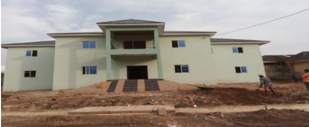
Picture 5: Completed Construction of Female Hostel, at Federal Cooperative College, Orji – River.
