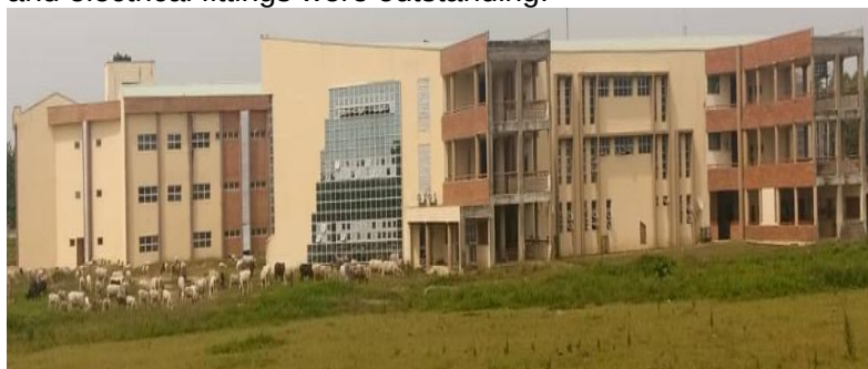
Picture 57: Ongoing Construction of Cyber Security Science Department at the FUT, Minna
