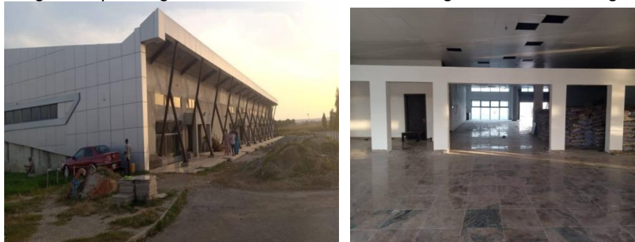
Picture 48: Ongoing Upgrade and Rehabilitation of Domestic Terminal Minna, Niger State
