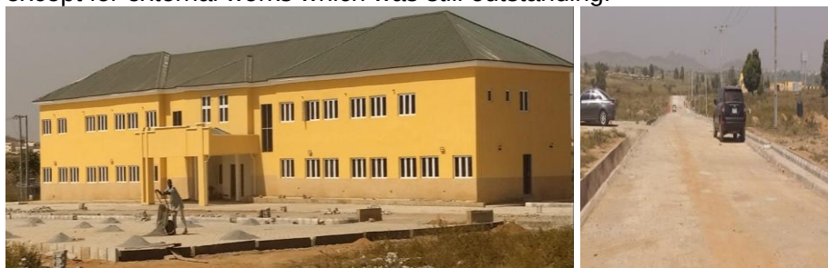
Picture 36: A Cross Section of Ongoing Works at Giri Cantonment Abuja (Phase 2), Nigerian Army.
