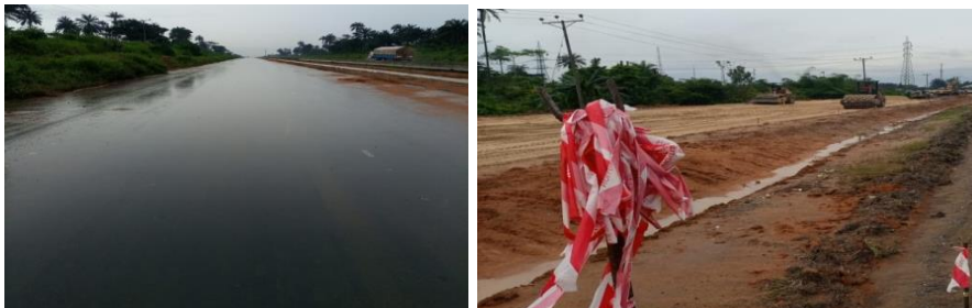
Picture 52: Ongoing Dualization of East-West Road Section II: (Ahoada-Kaiama) in River/Bayelsa State
