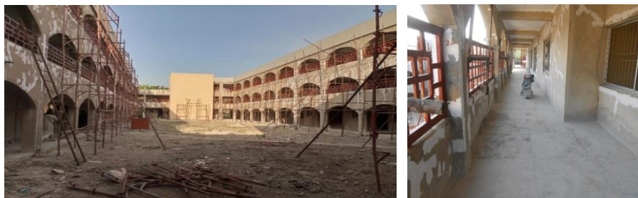
Picture 33: Ongoing Construction of 40nos. Flats for Resident Doctors at AKUTH, Kano.
