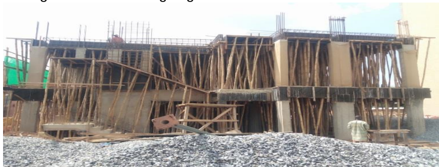
Picture 69: On-going Construction of ICT Centre at NYSC Directorate Headquarters
