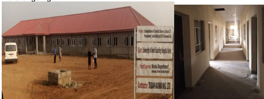
Picture 30: Completion of Central Stores/Procurement Department/ACTU Office
