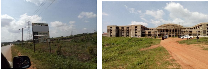
Picture 16: Construction of Federal Secretariat Complex at Oshogbo.
