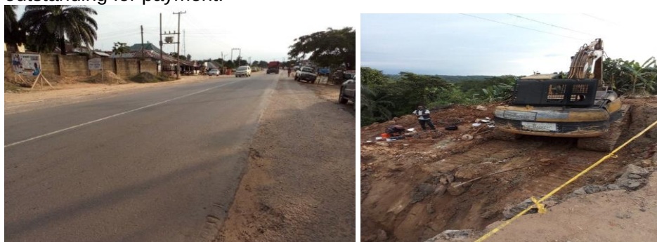
Picture 12: Ongoing rehabilitation works on Alesi-Ugep (Iyamoyung-Alesi) Road in Cross River State
