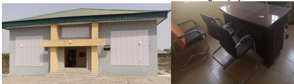
Picture 68: The Completed Entrepreneurship Building at the Michael Imodu Institute of Labour Studies Ilorin, Kwara State
