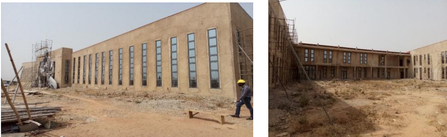
Picture 44: Ongoing Construction of AIB Training School in Abuja
