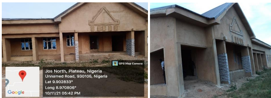
Picture 66: Front & Back Views of the Lecture Theatres and Classrooms at Nigerian Film Corporation's Permanent Site, Jos
