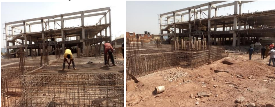
Picture 71: Ongoing Construction/Provision of Infrastructures (Pilgrims Heritage Camp) at the National Christian Pilgrims Board's Permanent Site
