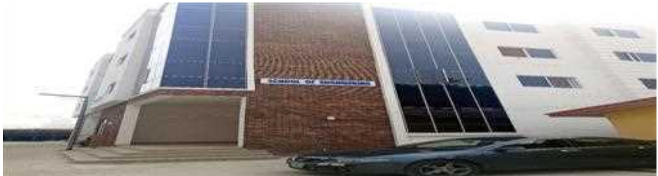
Picture 81: Constructed Marine Engineering Building at FCFMT Victoria Inland, Lagos.
