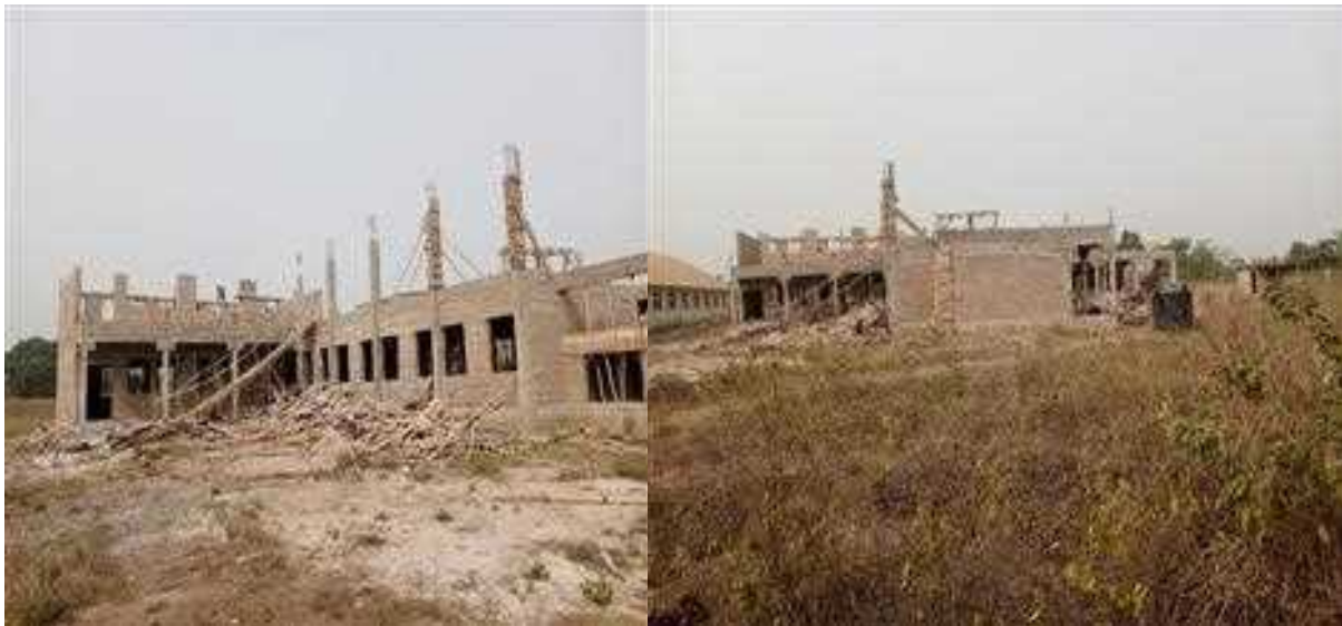
Picture 39: Ongoing construction of 1 no block of 6 classrooms with furnishing
