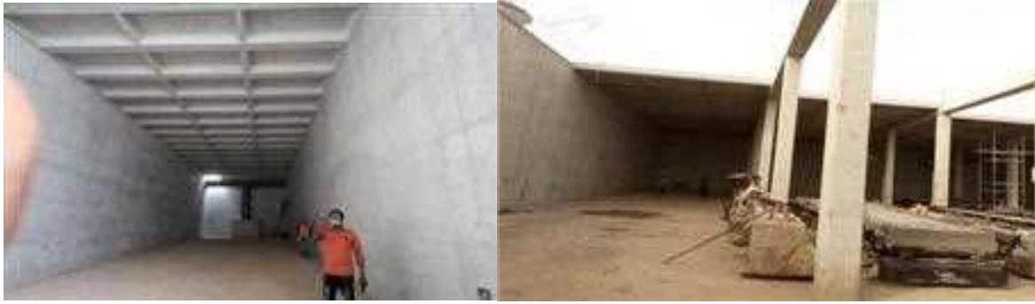
Picture 19: Ongoing Water Treatment Tank Reservoirs in Takum town.
