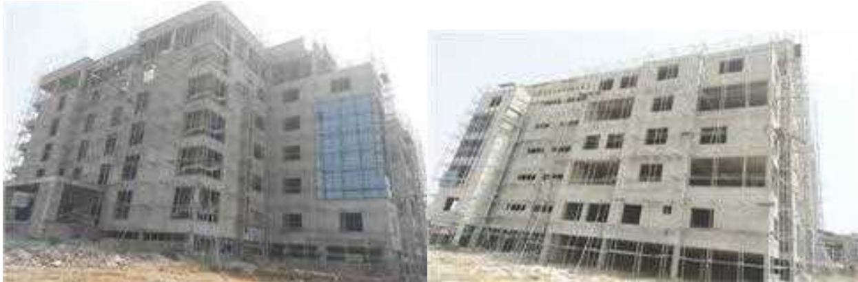
Picture 10: Ongoing construction/provision of office building at DRDB, Abuja.
