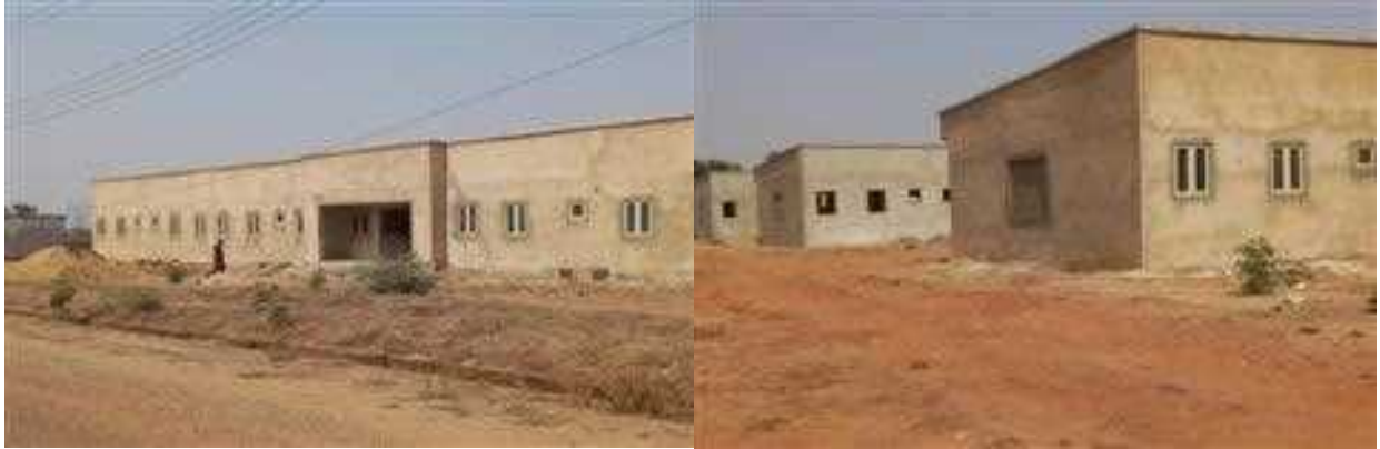
Picture 3: Ongoing construction of Hostel at DICON, Zaria
