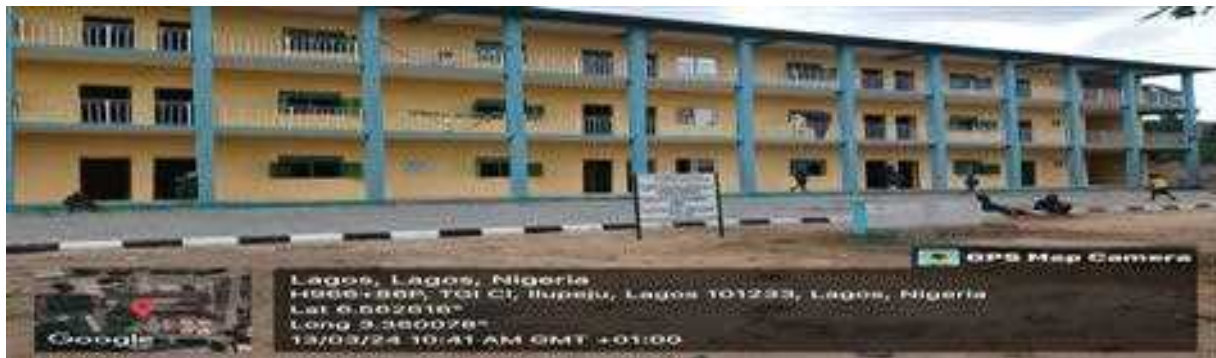
Picture 85: Completed three floors Class Rooms at Ikeja Cantonment, Lagos.
