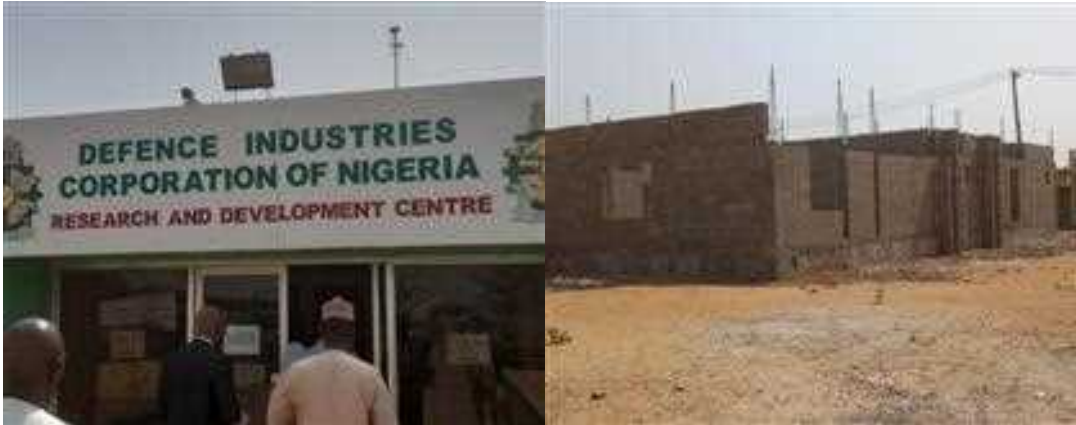
Picture 4: Ongoing construction of Quality Control building at DICON, Kaduna.
