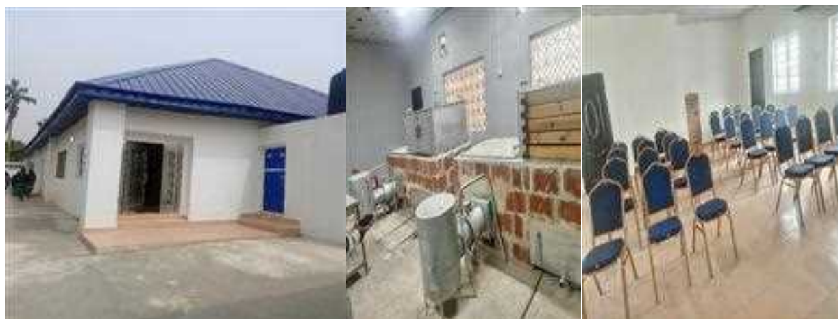
Picture 82: Completed Traore Laboratory and Provision for Prevention of Post-Harvest Loss and Public Health Safety for Farmers.
