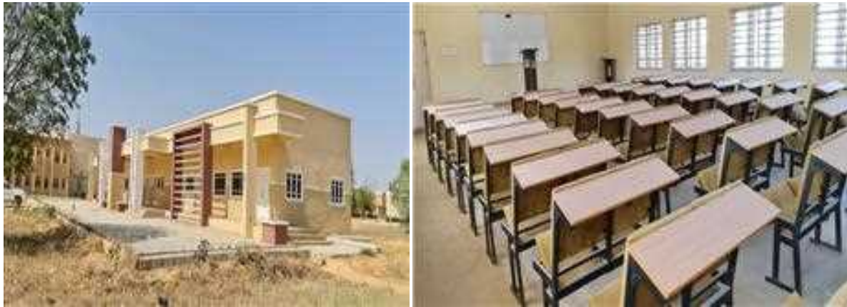
Picture 36: Completed Class Room Block at Federal university, Dutse.
