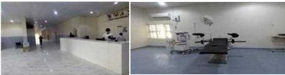
Picture 53: Ongoing Construction and Upgrading of Hospital Buildings and Wards.
