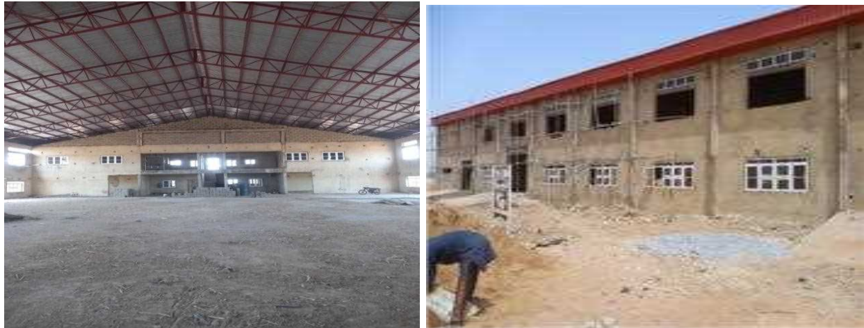
Picture 86: Ongoing construction of development of footwear workshop at NILEST, Zaria.
