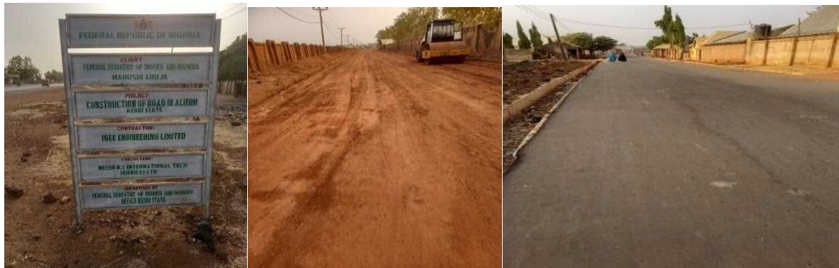
Picture 12: Ongoing construction of Aliero Road, Kebbi State.
