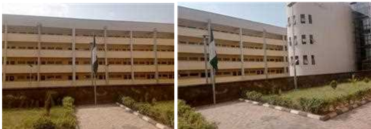
Picture 17: Completed Federal Secretariat Building Complex at Awka, Anambra State.
