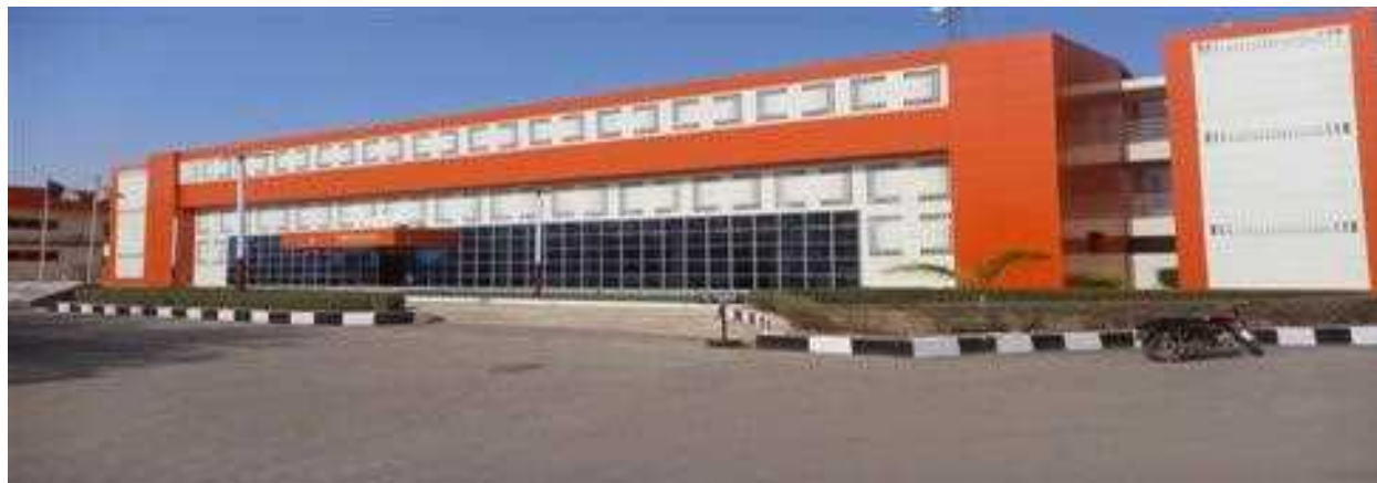
Picture 89: Remodelling of Admin. building at NITT, Zaria.
