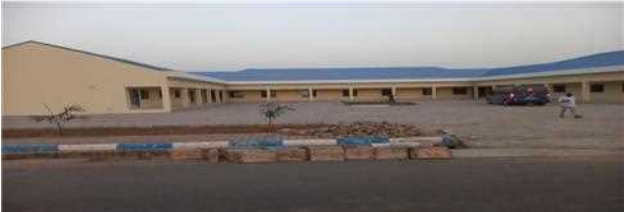
Picture 5: Ongoing construction of classrooms at AFIT, Kaduna
