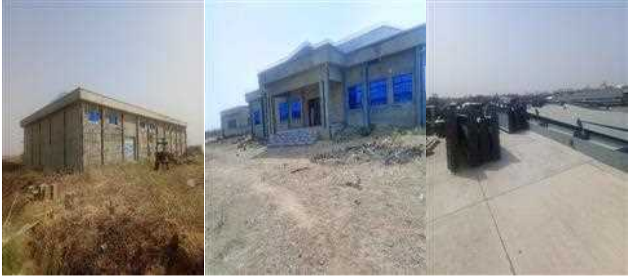
Picture 7: Ongoing completion of hanger project at Nigeria Airforce, Bauchi.
