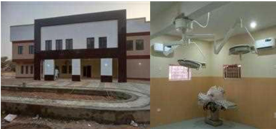
Picture 56: Ongoing construction of Trauma centre at ABUTH, Zaria.
