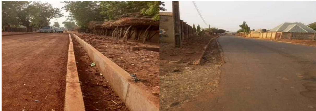
Picture 11: Ongoing construction of Jega Road at Kebbi State.
