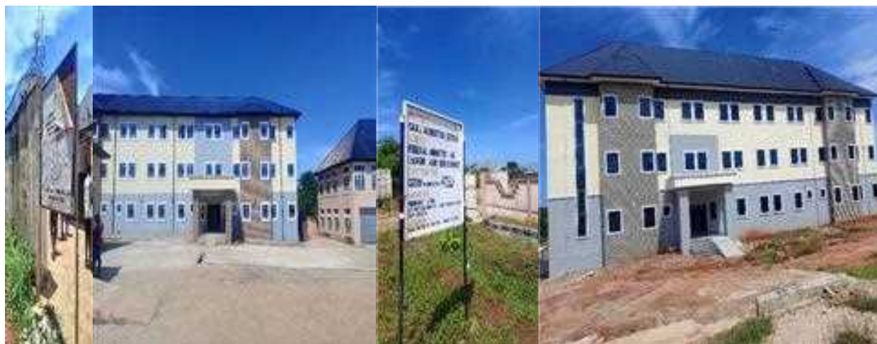
Picture 92: Completed Hostels for Specialized Skills Acquisition Centres in Ifitedunu and Alor in Anambra State.
