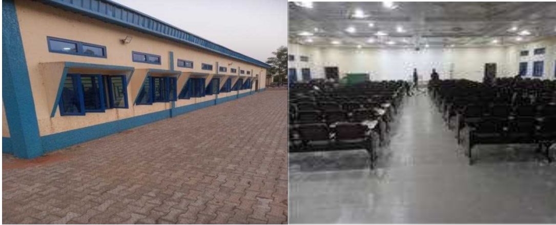
Picture 6: Completed maintenance hall at AFIT, Kaduna.
