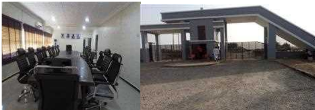
Picture 20: Ongoing Completion of Headquarters' Infrastructure Rehabilitation at URBDA, Yola.
