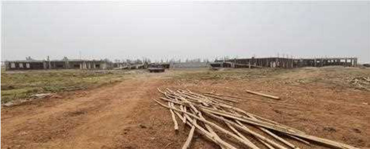
Picture 79: Ongoing Construction of Multi-Purpose Training Centre at ARMTI, Ilorin.
