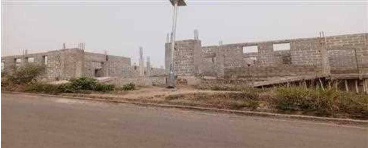
Picture 65: Ongoing Construction of catering building at FMC, Abeokuta.
