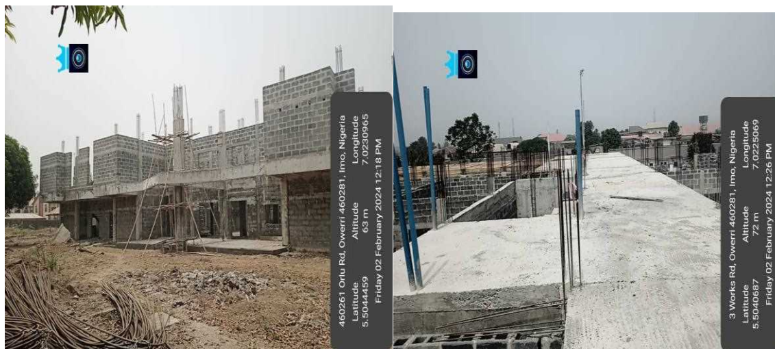
Picture 68: Ongoing completion of the trauma centre at FMC, Owerri.
