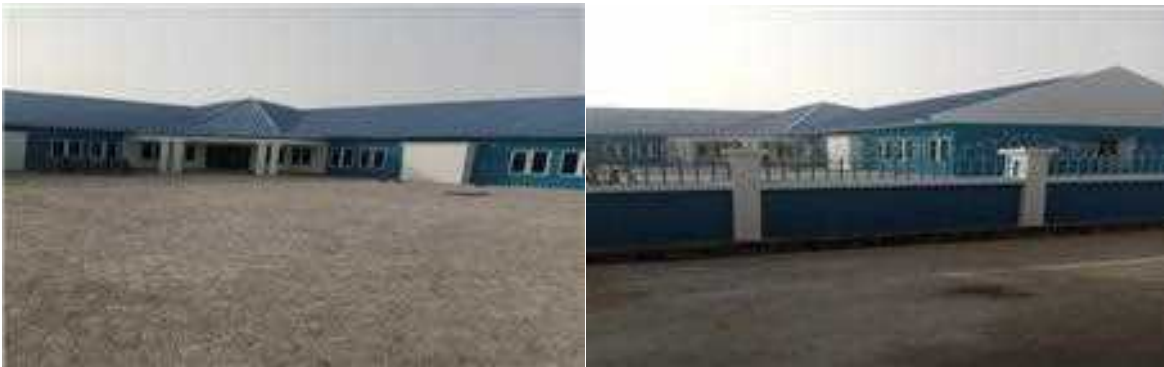
Picture 91: Completed Construction of FRSC, Zaria Unit Command.
