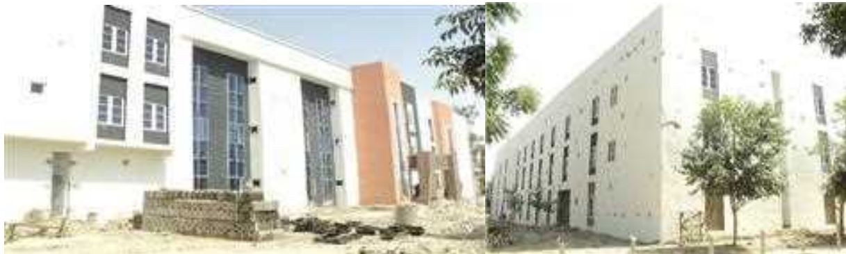
Picture 46: Completed radiology department extension at University of Maiduguri Teaching Hospital, Maiduguri.
