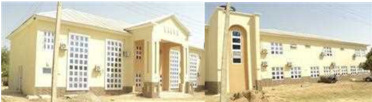
Picture 49: Completed rehabilitated and expansion of ENT complex at ATBUTH, Bauchi.
