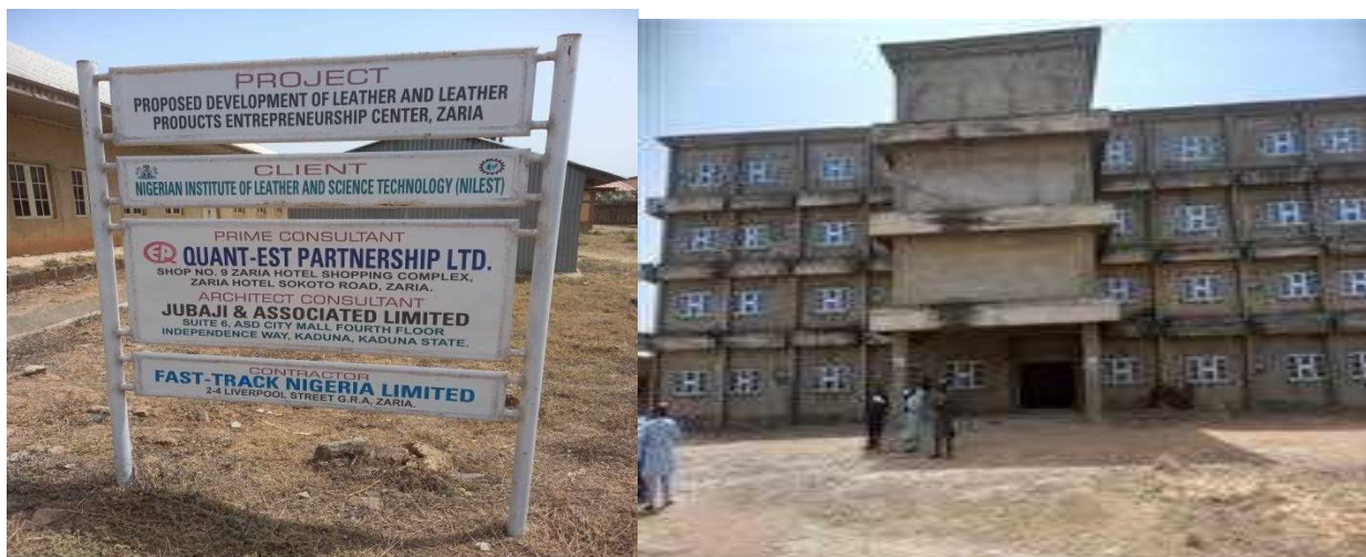
Picture 87: Ongoing construction of Leather Product entrepreneurship centre at NILEST, Zaria.
