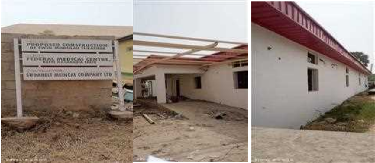
Picture 60: Ongoing Construction of Modular Theatre at Federal Medical Centre, Keffi.
