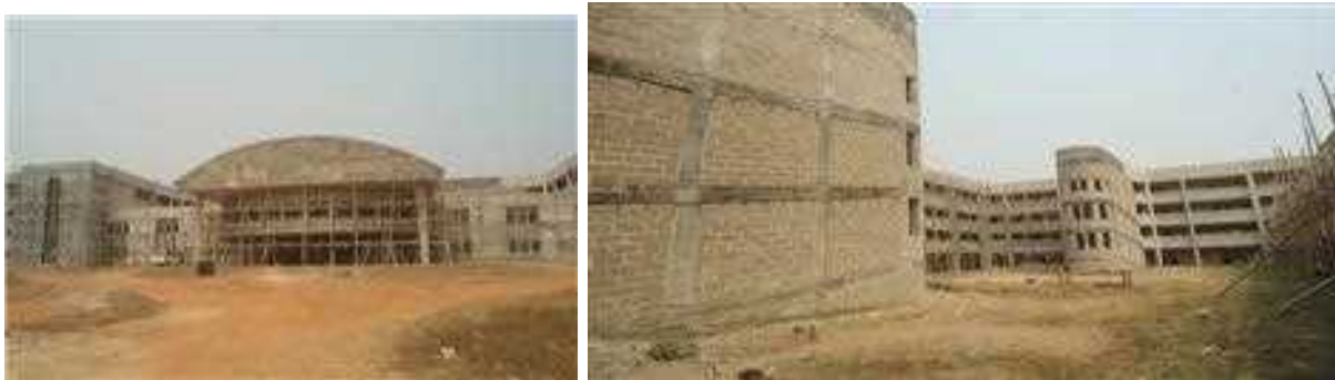
Picture 15: Ongoing Construction of Federal Secretariat Complex, Oshogbo.
