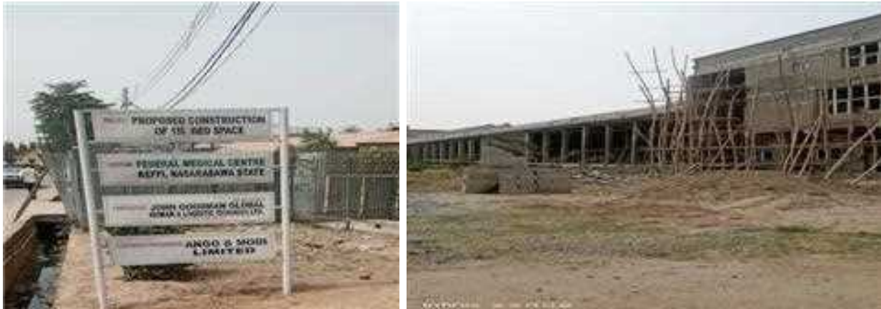
Picture 59: Ongoing Construction of Wards at the FMC, Keffi.
