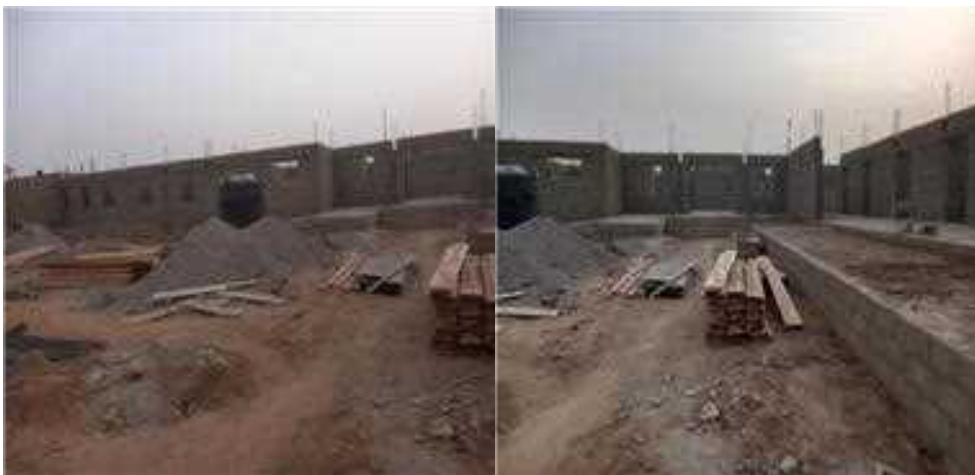
Picture 57: Ongoing Construction of Cardiology and Cardiothoracic Complex at ABUTH, Zaria.
