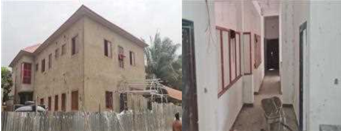
Picture 58: Ongoing Conversion of Existing Male Ward at Ear Centre, Kaduna
