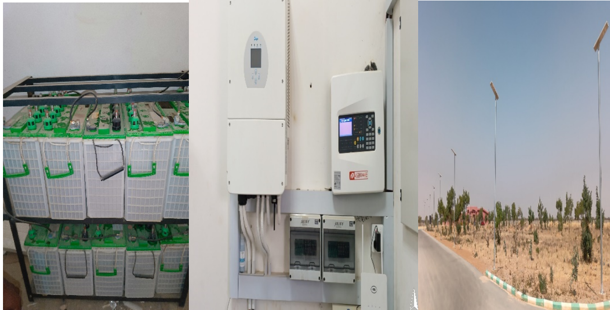
Picture 211: Supply & Installation of 3in1 Solar Street Light in FUT, Daura, Kastina State.
