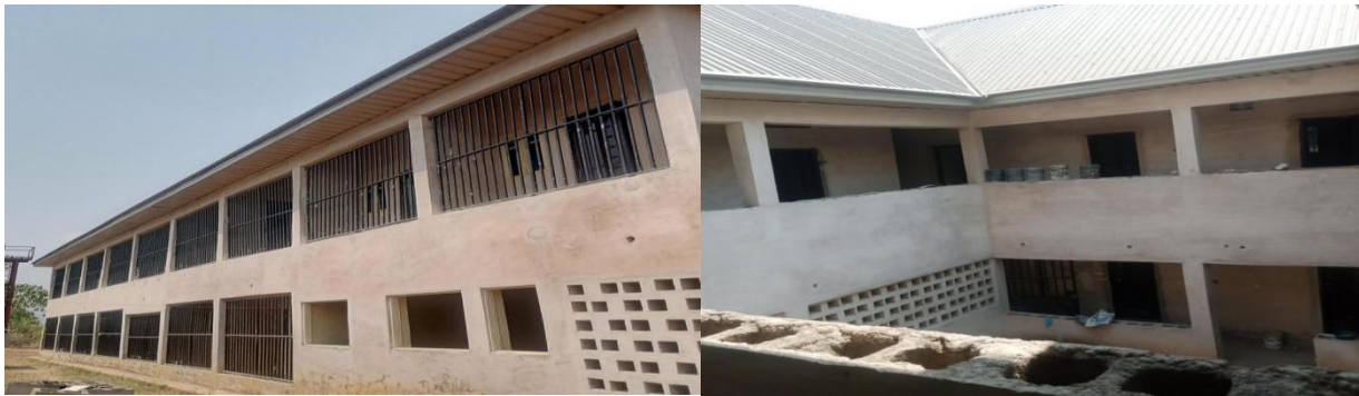
Picture 123: Ongoing Construction of Hostel Phase II at Akanu - Ibiam Federal Polytechnic Uwana - Afikpo.
