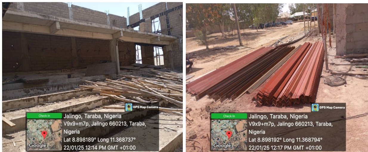
Picture 109: Ongoing Construction/Equipping and furnishing of Auditorium Hall FMC, Jalingo
