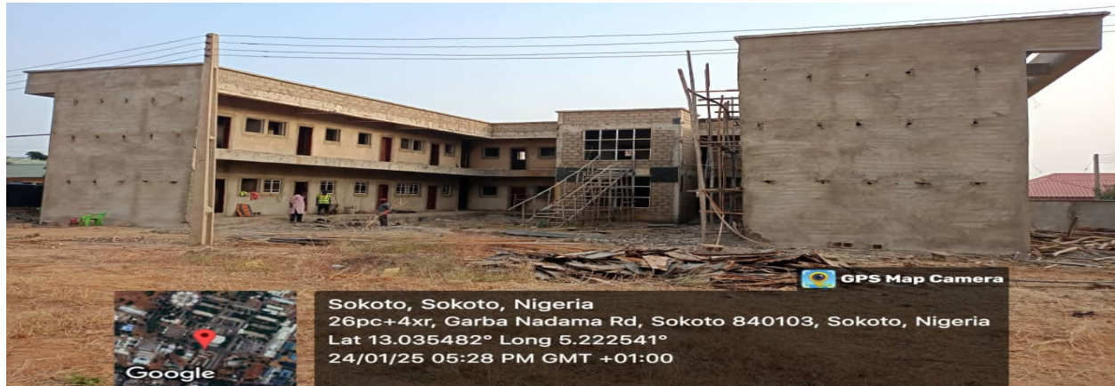
Picture 52: Ongoing construction and furnishing of a storey building multipurpose students' hostel at FNPH, Kware - Sokoto.
