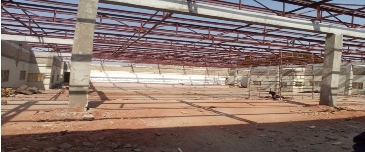
Picture 180: Ongoing Rehabilitation of Academic Building at Federal Polytechnic, Bida.
