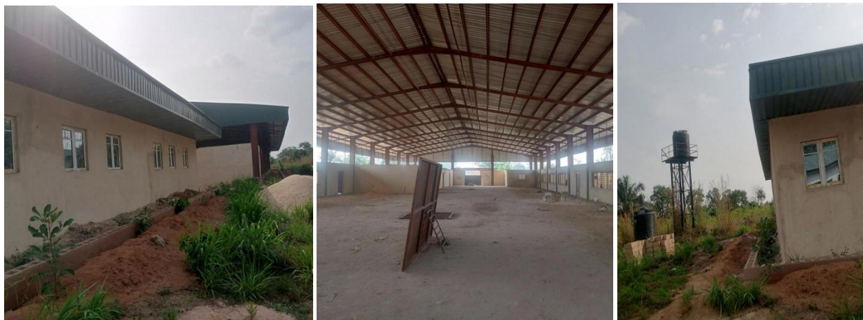
Picture 226: Ongoing Construction of Engineering and Welding workshop at National Metallurgical Training Institute (MTI), Onitsha.
