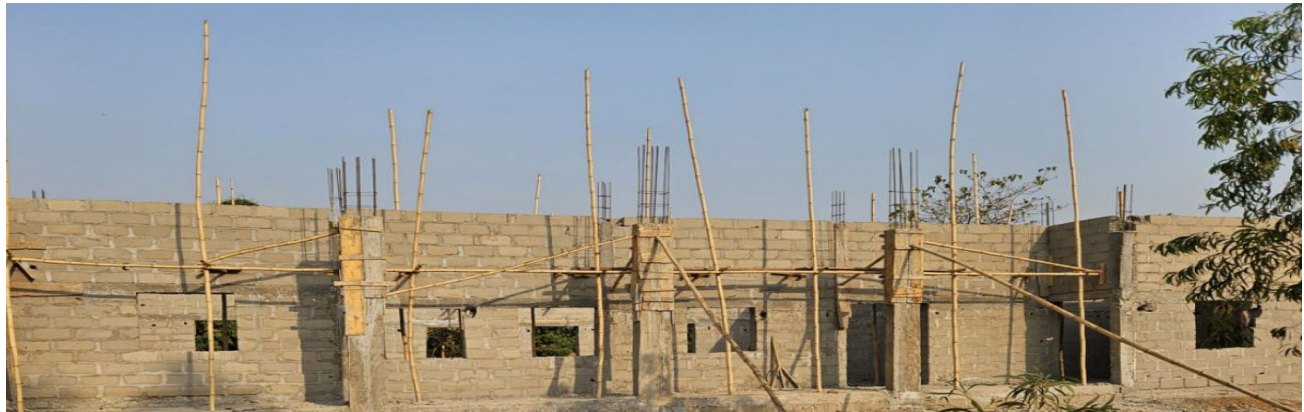
Picture 126: Ongoing Construction of lecture theatre at Faculty of Social Sciences, Alex Ekwememe Federal University, Ndufu Alike, Ebonyi State.
