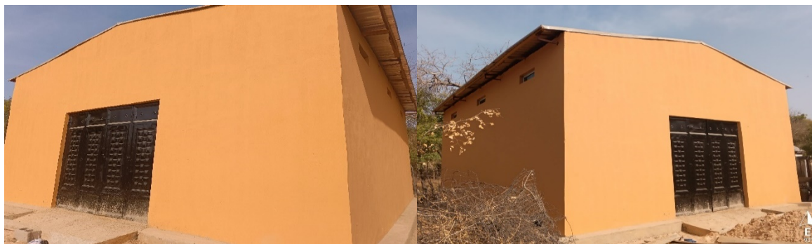
Picture 190: Completed central store at Bayero University New Campus, Kano State.
