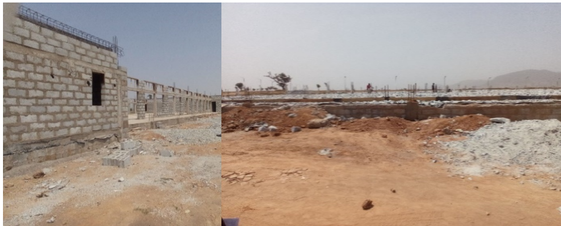
Picture 213: Ongoing Construction of multipurpose hall, Research Centre, Synoptic Laboratory, Fencing and Gate House at the permanent site of AAAU, Abuja
