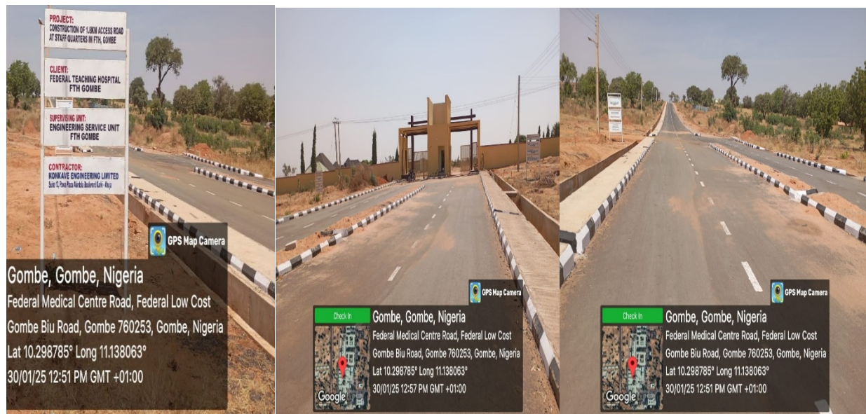
Picture 107: Constructed 1.8 km Access Road at Staff Quarters, FTH Gombe.
