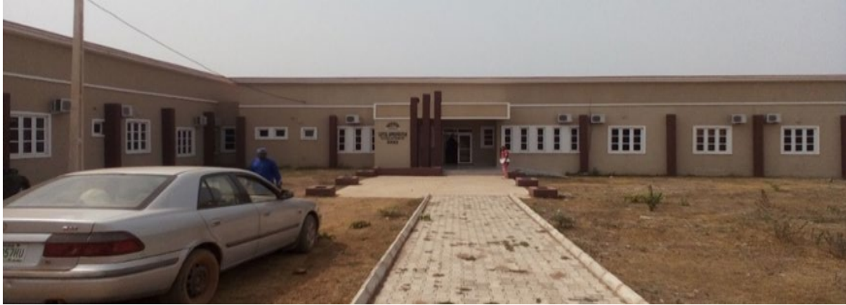
Picture 186: Completed construction and furnishing of 30nos offices at Federal Polytechnic, Offa.
