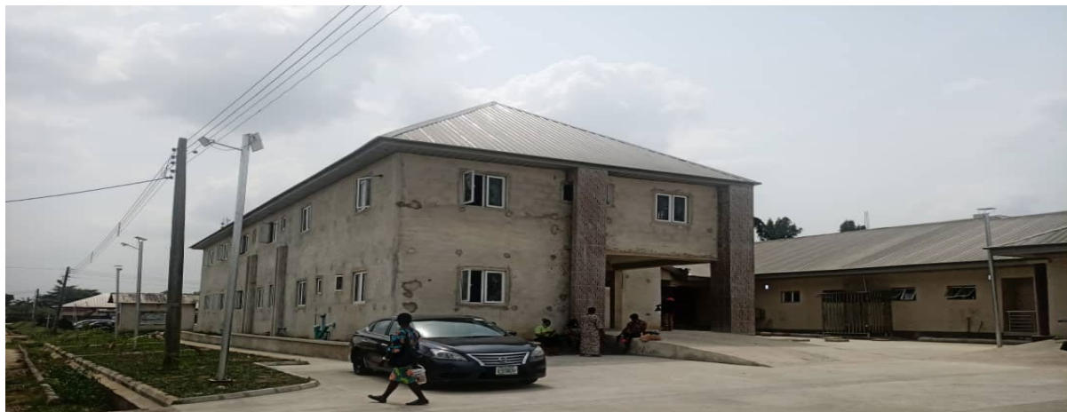
Picture 76: Ongoing Expansion of Accident and Emergency Block at Uyo Teaching Hospital.
