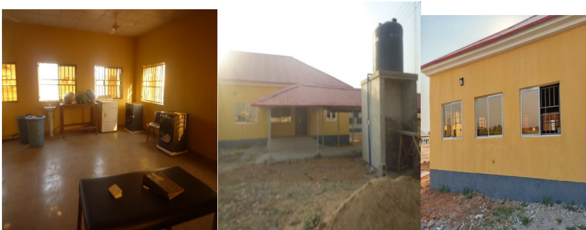
Picture 116: Constructed/equipped laundry unit at FMC, Makurdi.
