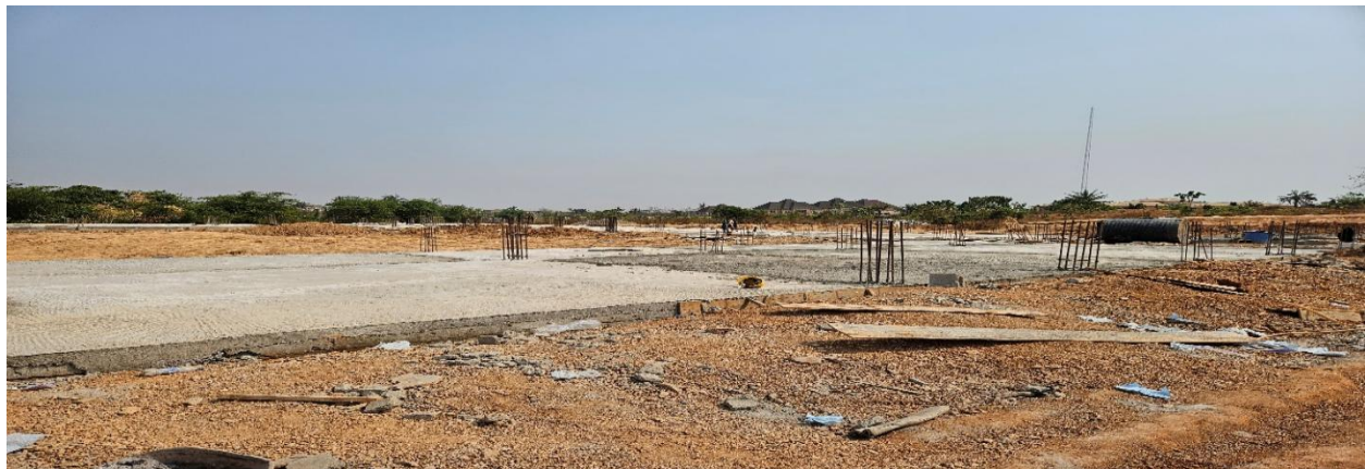
Picture 20: The Ongoing Construction of Federal Secretariat, Abakaliki, Ebonyi State.
