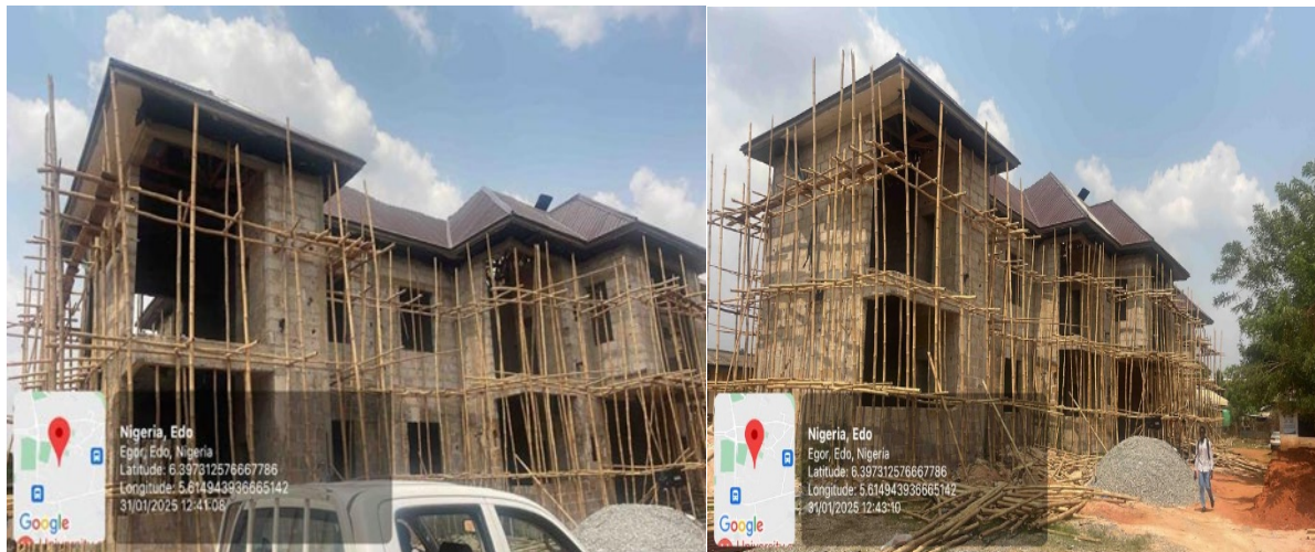
Picture 138: Ongoing Construction of Internal Audit Building at University of Benin, Edo State.
