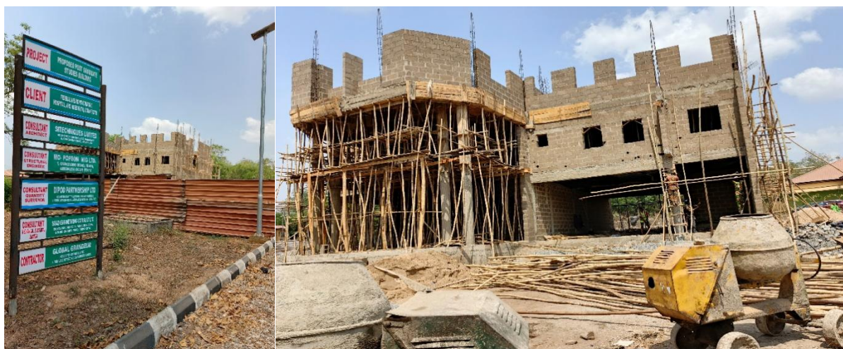
Picture 98: Ongoing Construction of 2-Storey Building at Post Graduate Complex of Federal Neuro psychiatric Hospital, Aro, Abeokuta.
