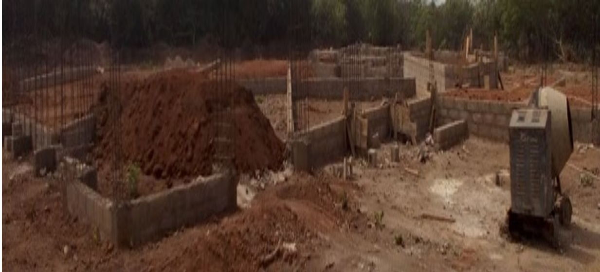
Picture 185: Ongoing construction of 500-seat capacity lecture theatre at Federal Polytechnic, Offa
