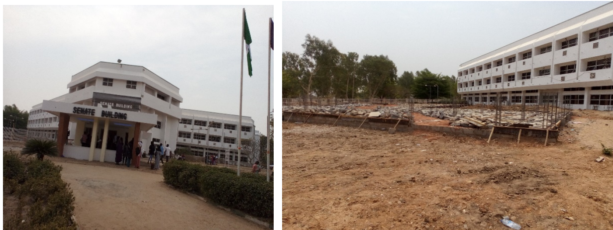
Picture 167: Construction of Senate building extension and entrance extension/ remodelling at FUT, Minna.
