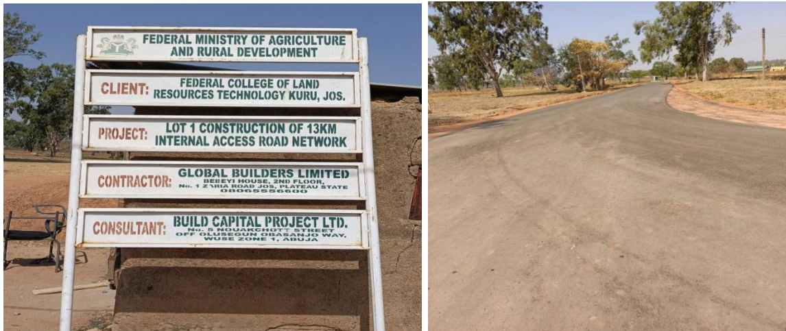
Picture 29: The ongoing Construction of 13km internal access road network at FECOLART,Jos
