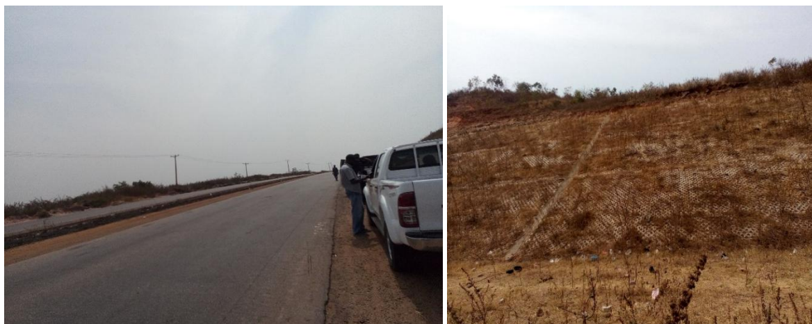
Picture 14: Abuja – Lokoja Road Section IV (Koton-Karfe – Lokoja)
