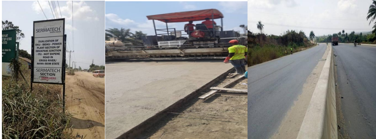
Picture 3: Ongoing Dualization of Oku Iboku- power plant section of the Odukpani Junction- Itu- Ikot Ekpene Road in Cross River / Akwa States.
