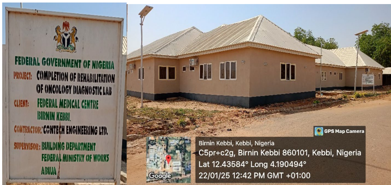
Picture 44: Completed extension of the existing oncology laboratory
