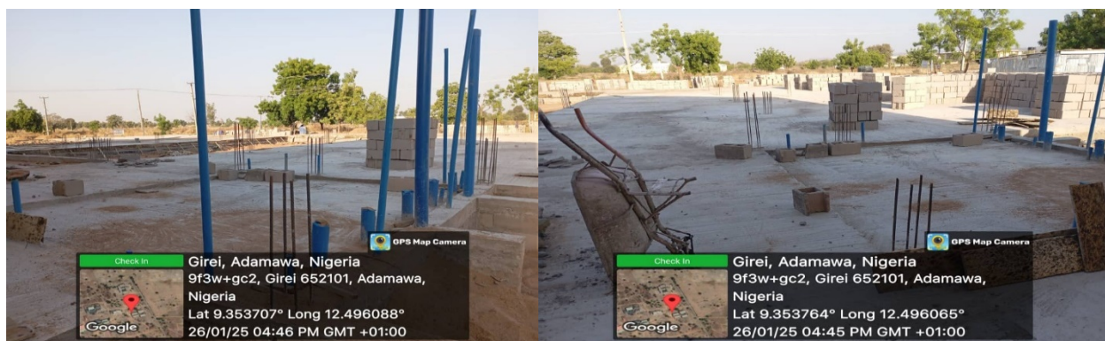
Picture 155: Ongoing Construction of the Department of Electrical Engineering and Electronics Laboratory at Modibbo Adama University, Yola.
