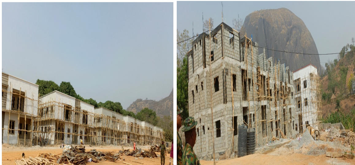
Picture 205: Ongoing construction of barracks building for officers at Niger Barracks, Abuja.
