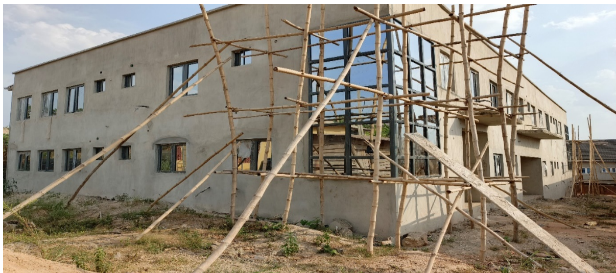
Picture 97: Ongoing Construction of Anatomic Pathology Building at Federation Medical Centre Abeokuta
