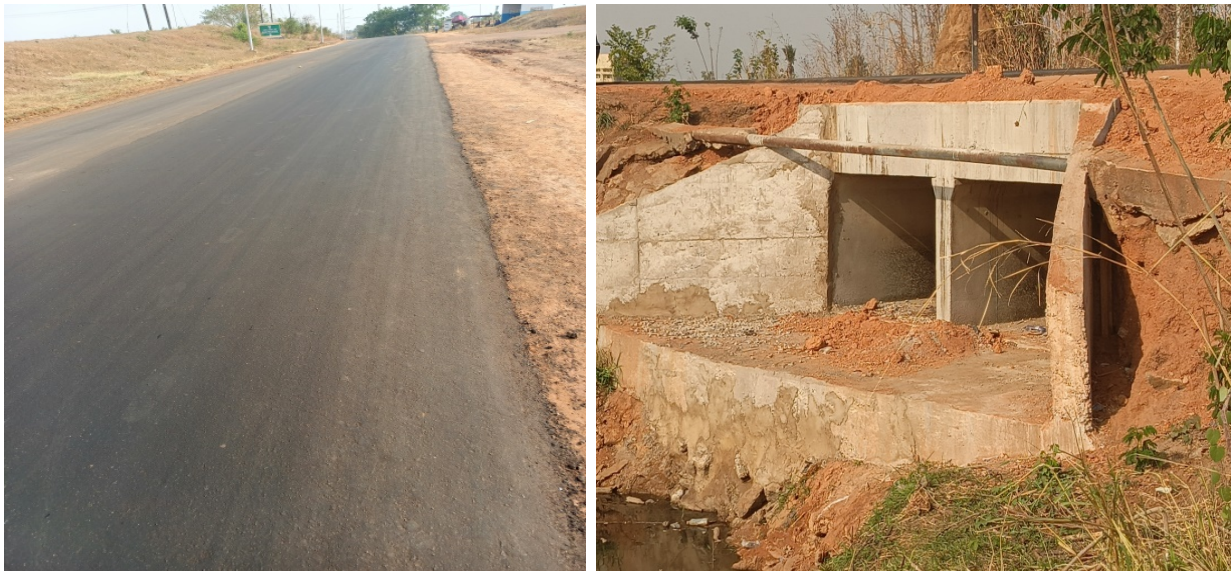
Picture 27: Construction of 2.3km Asphaltic Road at Federal University of Agriculture, Makurdi.
