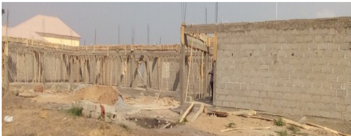
Picture 183: Ongoing construction of 4nos classroom at FCE, Okene.
