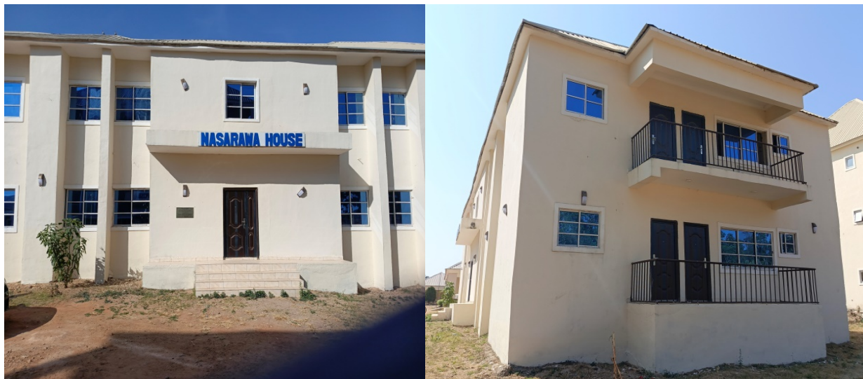
Picture 222: Completed rehabilitation of participant's quarters at NIPSS, Jos.
