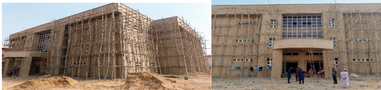
Picture 192: Ongoing Construction of Advanced Laboratory for Science and Technology at Federal Polytechnic, Kaduna.
