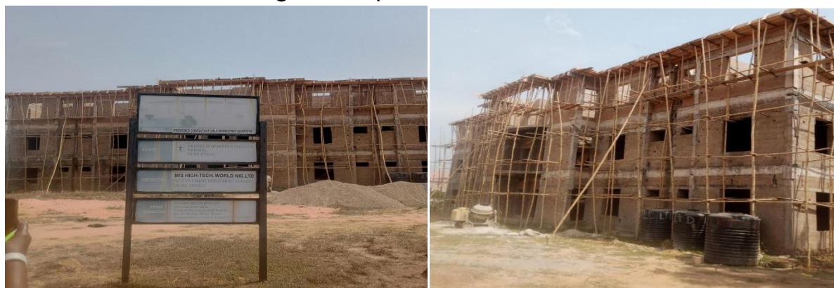
Picture 62: Ongoing Construction of a 2-Storey Building for Doctors' Quarters at University of Nigeria Teaching Hospital, Enugu.
