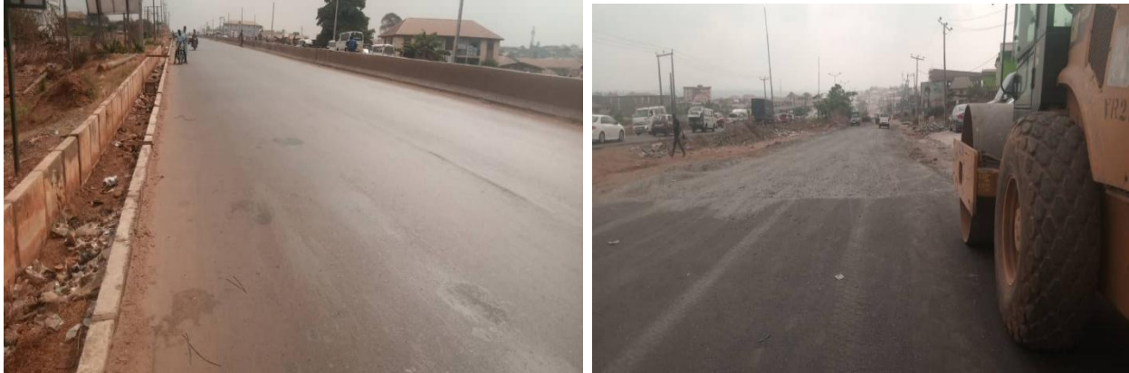
Picture 6: Ongoing Reconstruction of Ibadan Ife-Ilesha dual carriageway in Oyo – State, C/No.6631.
