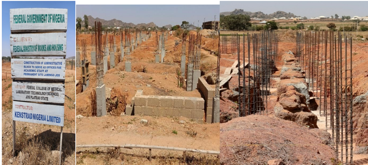
Picture 117: Ongoing construction of Admin Block for Academic Staff in FMLT, Jos.
