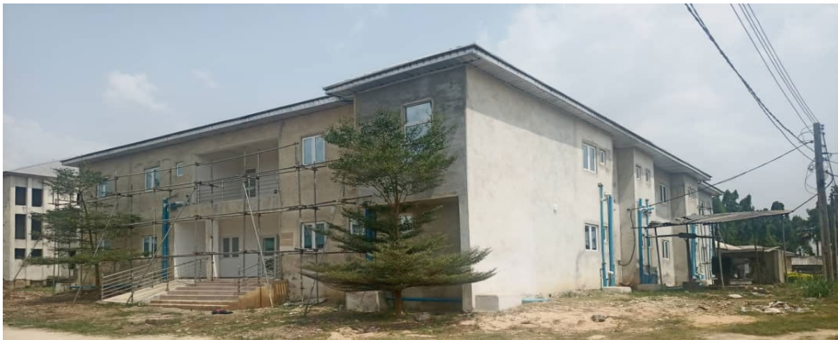
Picture 77: Completed expansion of ante-natal block at University of Uyo Teaching Hospital.
