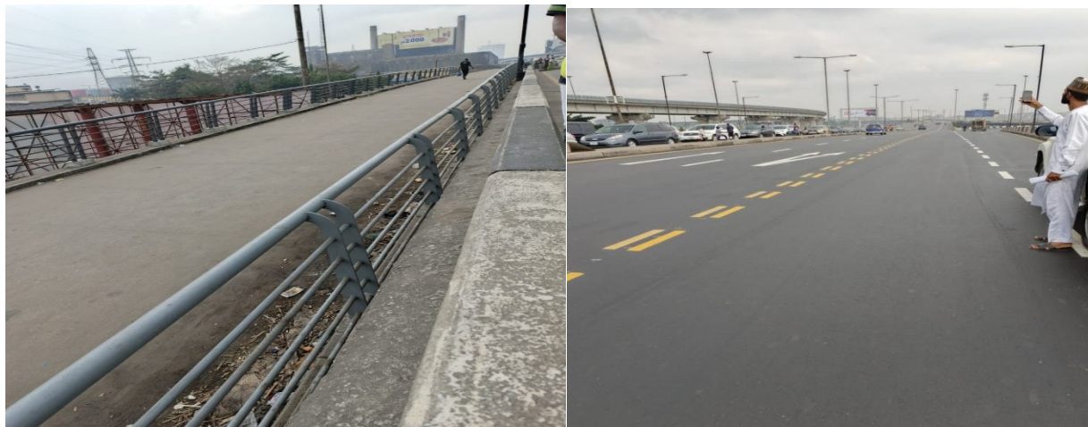
Picture 7: Emergency Comprehensive Repairs of Eko Bridge in Lagos State.
