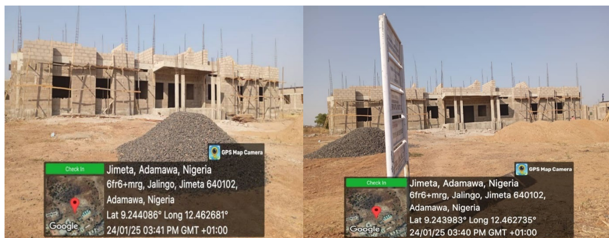
Picture 161: Ongoing Construction of Nomadic and Entrepreneurship Centre at FCE, Yola.
