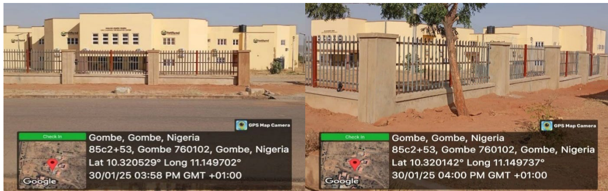
Picture 159: Ongoing Construction and Fabrication of 450m Fence at ECCE Complex and Other Structures.
