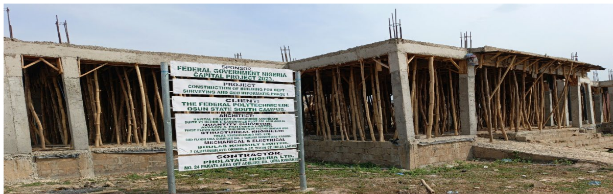
Picture 144: Ongoing Construction of Surveying and Geo-informatic Department at Federal Polytechnic, Ede, Osun State.
