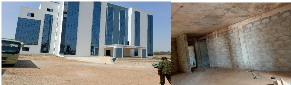
Picture 206: Ongoing construction of Administrative Building at Defence Research & Development Bureau, Abuja.
