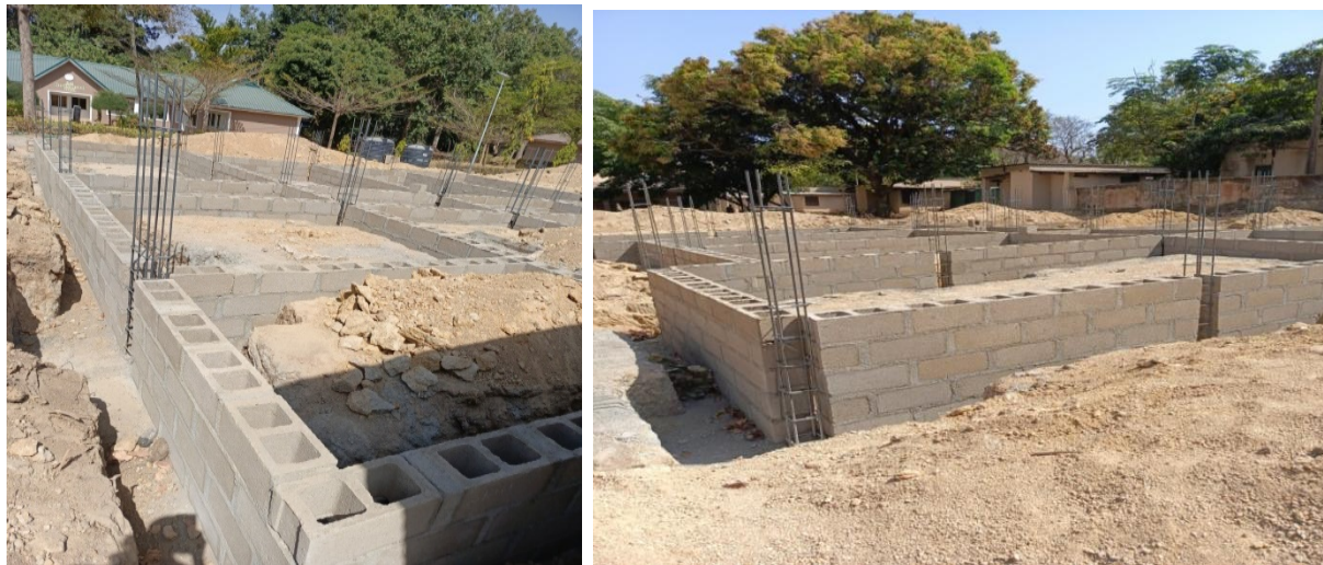
Picture 229: The Ongoing construction of CBT Centre at Federal College of Forestry, Jos.
