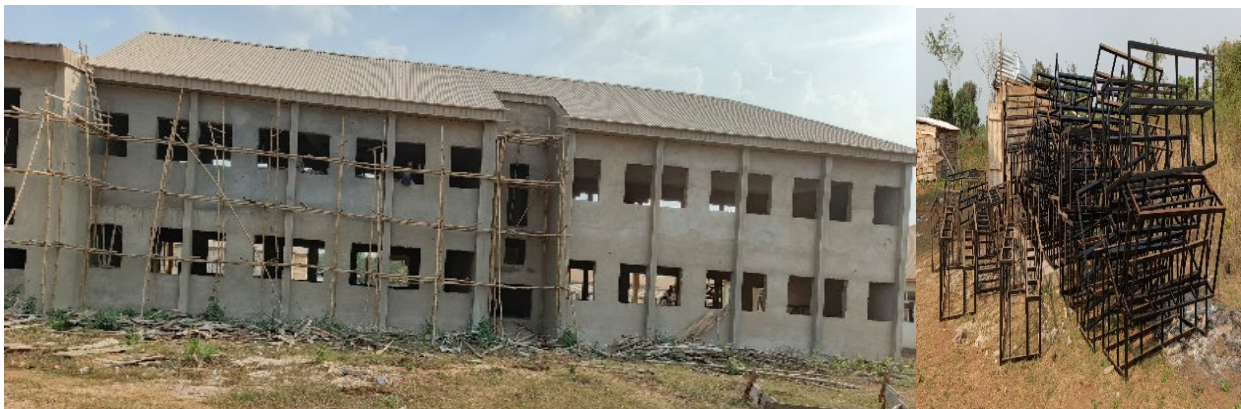
Picture 151: Ongoing Construction of 1no Block of 6 Classrooms at Federal Polytechnic Ilaro.
