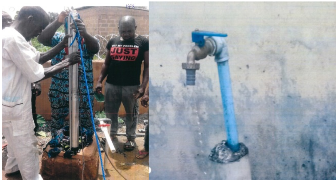
Picture 38: Ongoing Integrated Water Scheme for the new layout area of the Ogu community in Ogu Bolo LGA, Rivers State.
