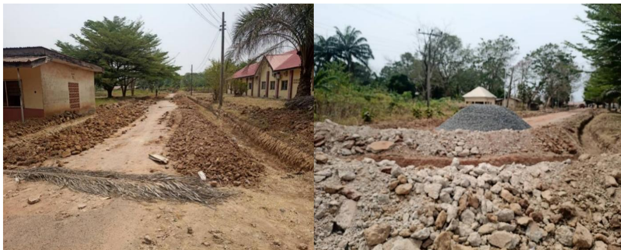
Picture 132: Ongoing Rehabilitation of 1km internal Road Network at the Main Campus Phase II FCE Obudu
