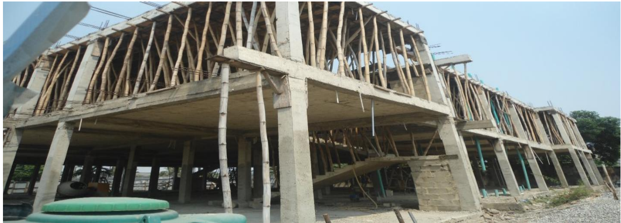
Picture 92: Ongoing Construction of Tele-Psychiatric Centre at Federal Neuro psychiatric Hospital, Lagos.
