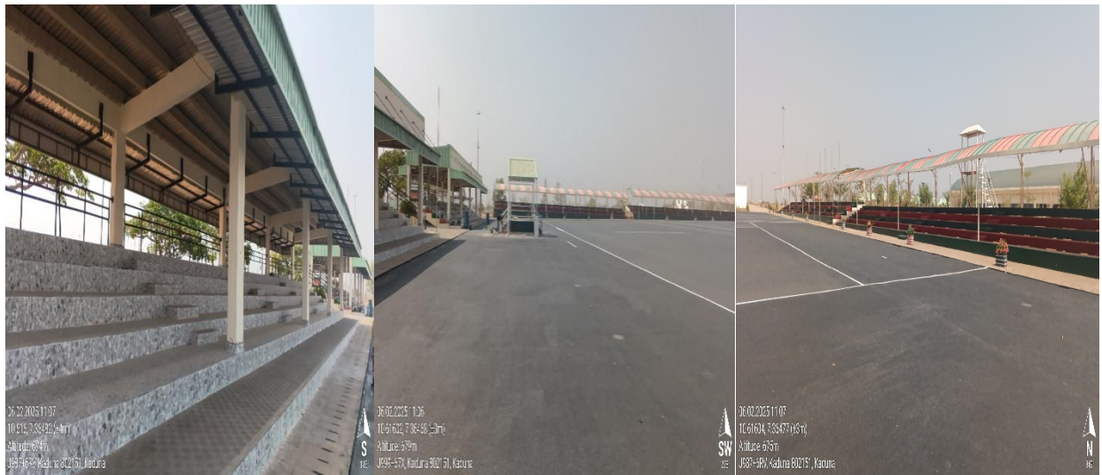
Picture 201: Completed Upgrade of Parade Ground at NDA Afaka, Kaduna State.
