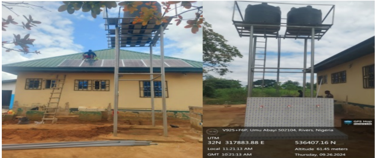
Picture 37: Ongoing Rehabilitation of Umuagbai Water Project including reticulation, Oyigbo LGA Rivers, State
