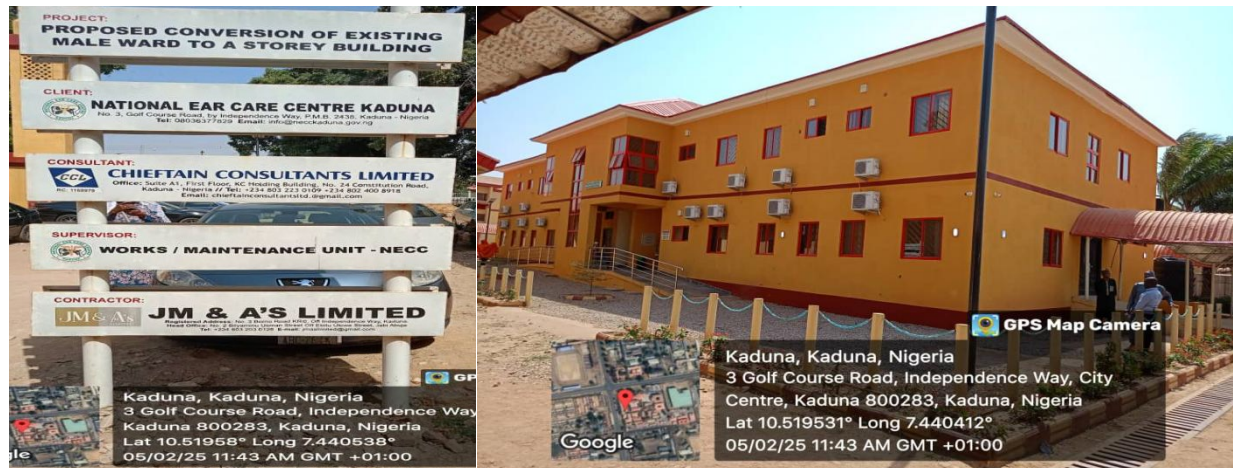
Picture 47: Completed Conversion of Existing Male Ward at National Ear Care Centre (NECC), Kaduna
