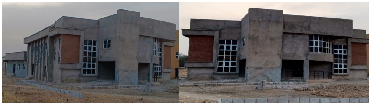
Picture 176: Ongoing construction & furnishing of multi-purpose lecture theatre complex at Federal University Dutse, Jigawa State.
