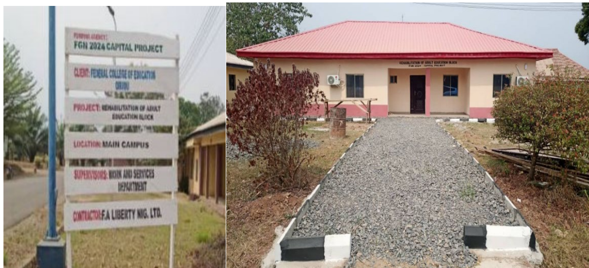
Picture 130: Completed Rehabilitation of Adult Education Block at FCE, Obudu
