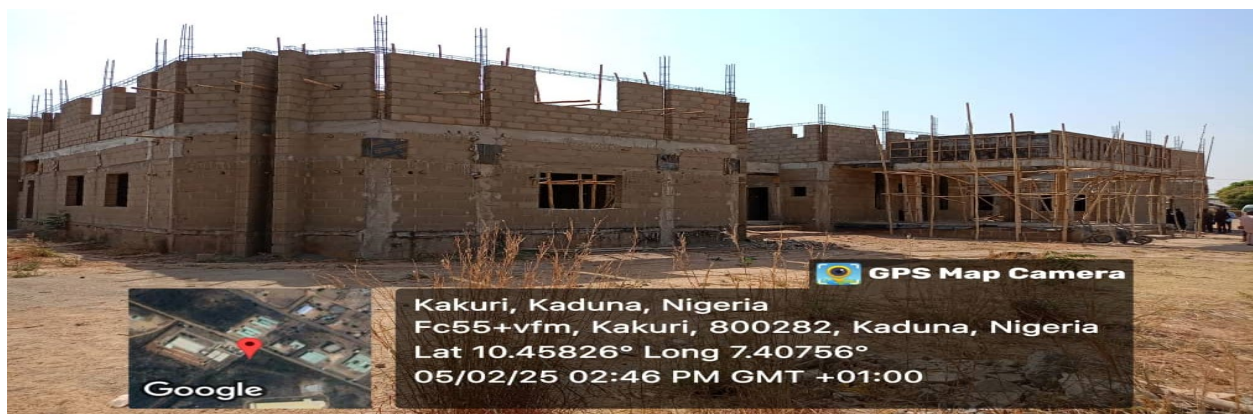
Picture 197: Ongoing construction of Quality Control Administrative Block at DICON, Kaduna.
