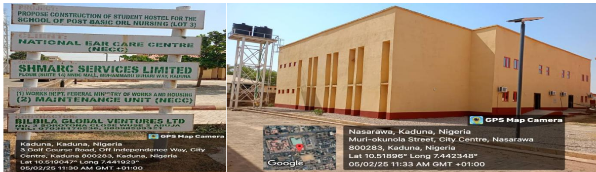
Picture 48: Constructed School of Post Basic ENT Students Hostel at NECC, Kaduna.
