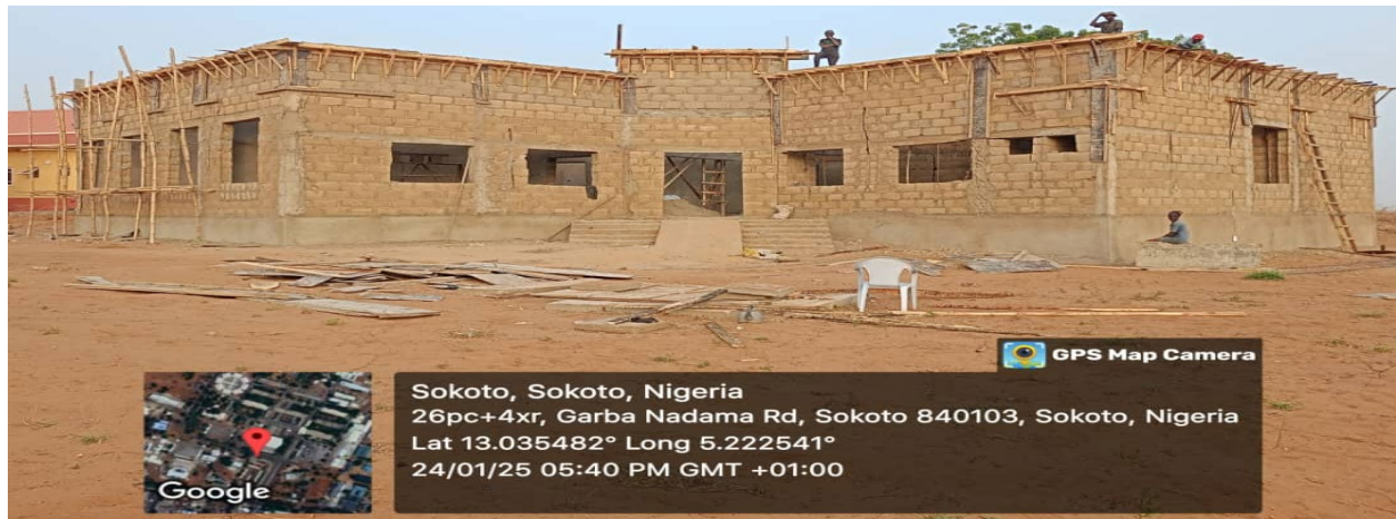
Picture 51: Ongoing Construction of the School of Post Basic Nursing at FNPH Kware - Sokoto.
