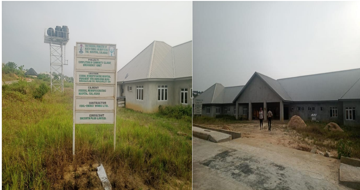
Picture 74: Ongoing Completion of Community Clinic/Emergency unit at permanent site of Federal Psychiatry Hospital, Calabar
