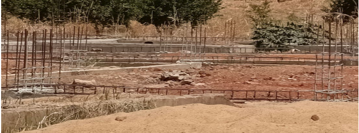
Picture 178: Ongoing construction of Engineering Studio at FCE, Wannune.
