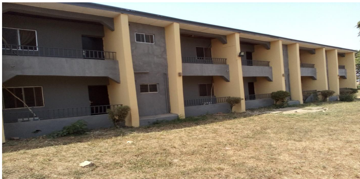
Picture 220: Rehabilitation of hostel at Micheal Imodu Institute, Ilorin
