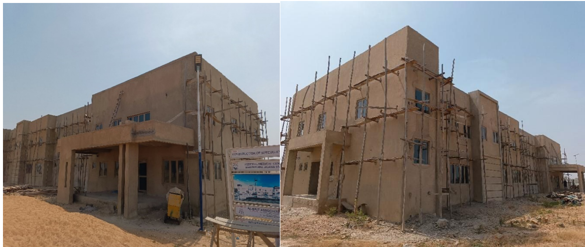
Picture 57: Ongoing Construction of Specialty Building at FMC, Birnin Kudu
