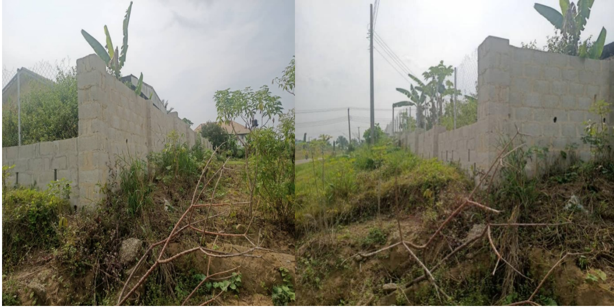
Picture 35: Ongoing Rehabilitation of broken portion of the fence at CRBDA Headquarters Calabar Cross River State
