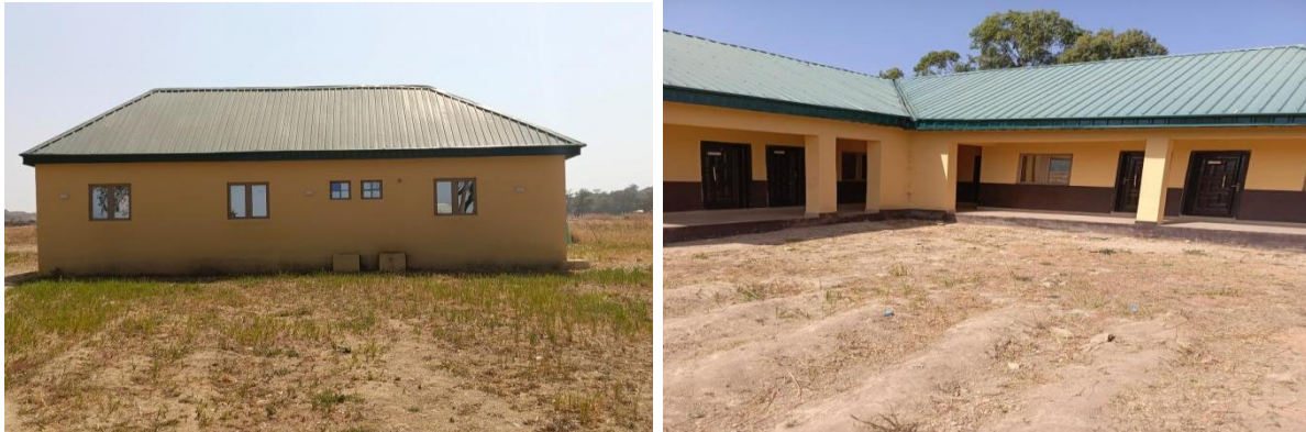
Picture 30: The ongoing construction of 25 Lecture offices at FECOLART, Jos
