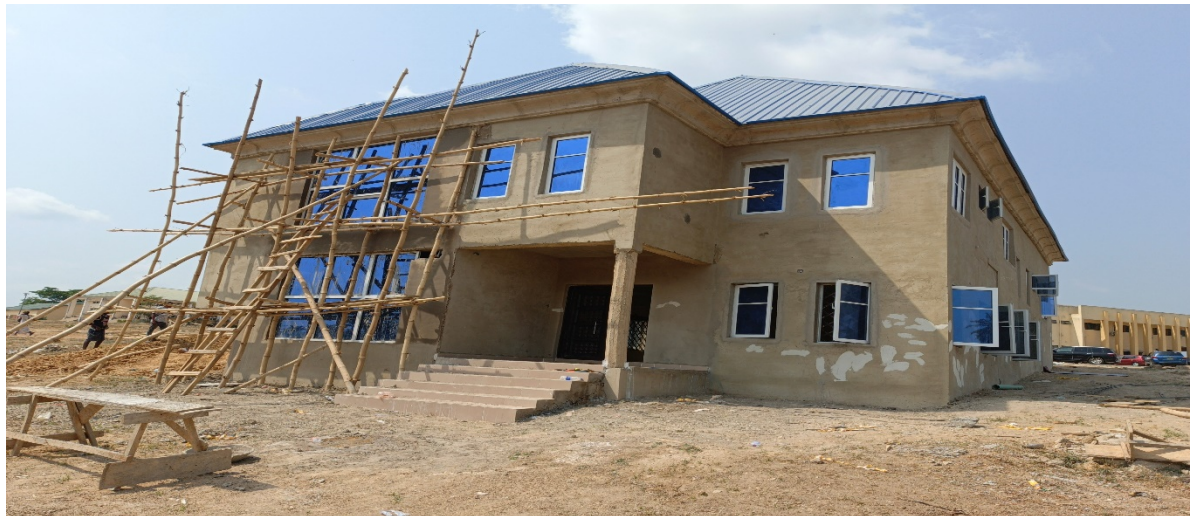
Picture 142: Ongoing Construction of academic office and classrooms at Federal University, Oye – Ekiti.
