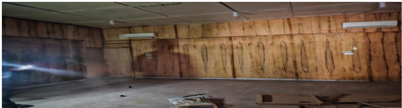
Picture 64: Completed base for the CT-Scan Machine at Federal Teaching Hospital, Abakaliki, Ebonyi State.
