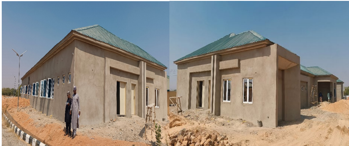
Picture 61: Completed intensive care unit at NOFIC, Kastina State.
