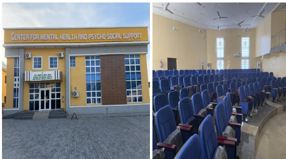
Picture 102: Completed Mental Health Psychological Support and Drug Rehabilitation Centre at Federal Neuro-Psychiatric Hospital, Maiduguri.
