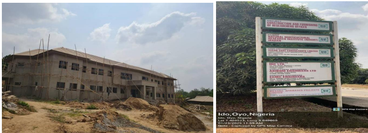
Picture 23: Ongoing Construction of new research office building Ibadan at NIHORT, Ibadan.
