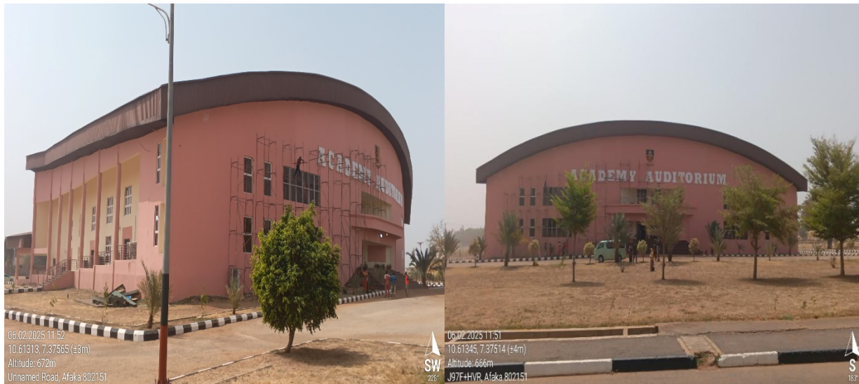
Picture 202: Renovated Auditorium at NDA Afaka, Kaduna.
