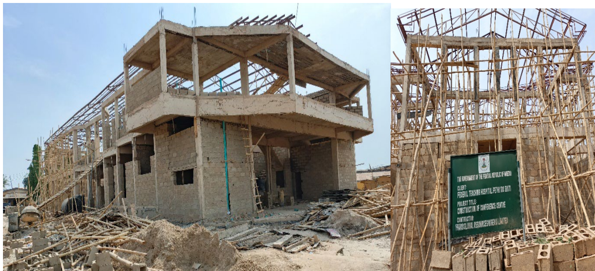
Picture 95: Ongoing Construction of Conference Centre at Federal Teaching Hospital, Ido – Ekiti.
