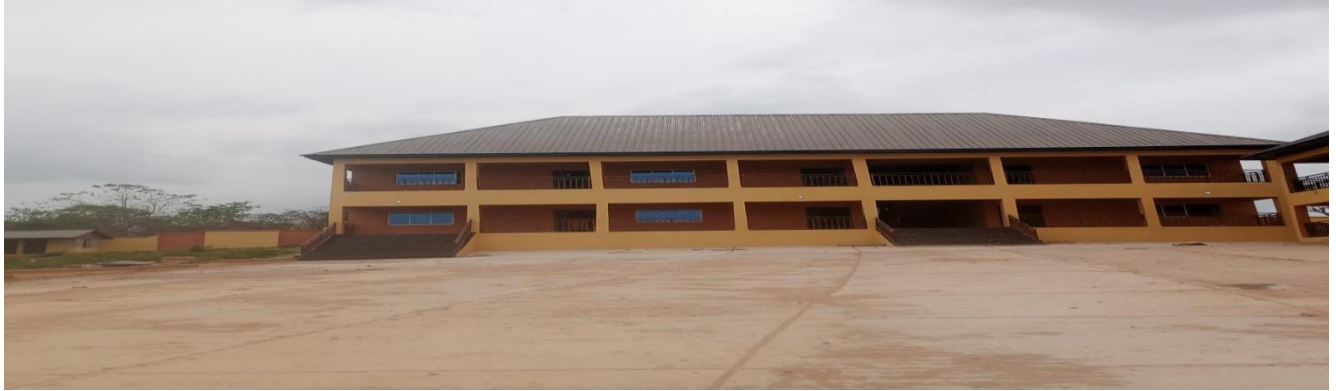
Picture 21: Completed 1-Storey Building Lecture Hall, at Federal Cooperative College, Orji – River.
