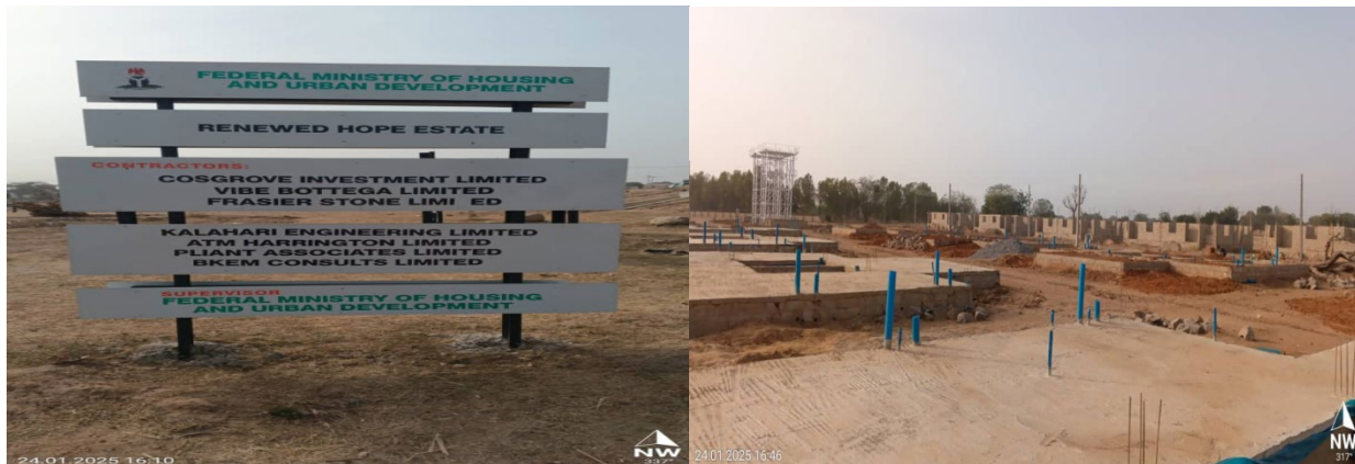
Picture 18: Ongoing Construction of 250 Housing Units at Kano State
