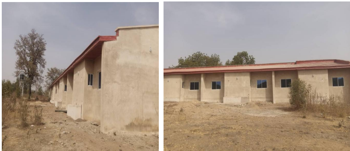
Picture 32: Ongoing Construction/ Provision of Residential Building at Fisheries, New Bussa.
