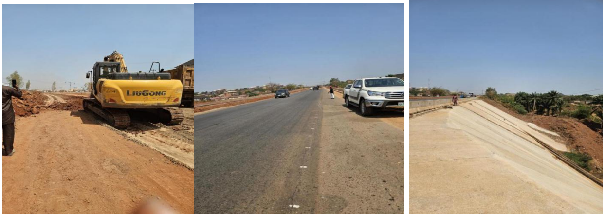
Picture 1: Ongoing Rehabilitation of Enugu - Port Harcourt Expressway Section III: Lokpanta - and Part of Erosion Control at Independence Layout in Enugu State.
