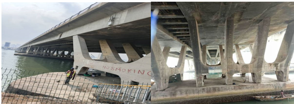
Picture 8: Ongoing Comprehensive Repairs of Marine Bridge in Lagos State, Contract No: 7479
