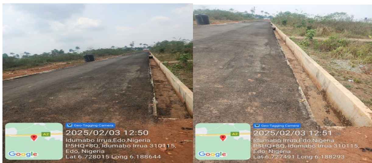
Picture 80: The Constructed 2.5 Kilometer Road and Landscaping with Drainages for Erosion control at Irrua specialist Hospital at Irrua.
