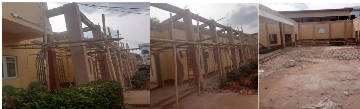
Picture 121: Ongoing Remodeling Centre for Entrepreneurship at University of Nigeria Nsukka.
