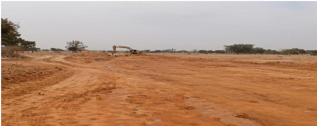
Picture 16: Ongoing Construction of Kano Northern Bypass Road
