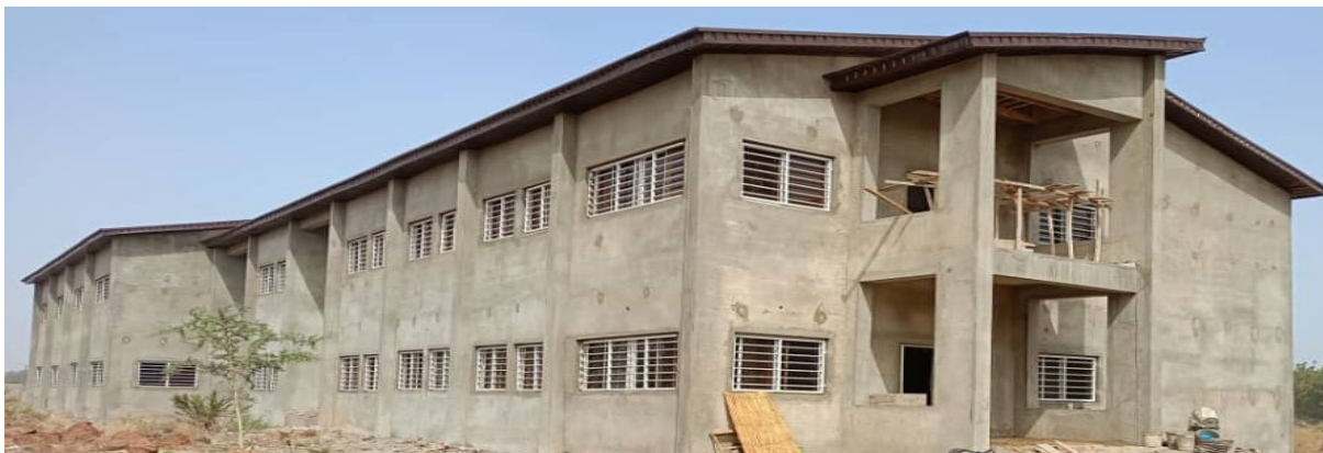
Picture 41: Ongoing Construction of Eye Centre at Usmanu Danfodio University Teaching Hospital (UDUTH), Sokoto.
