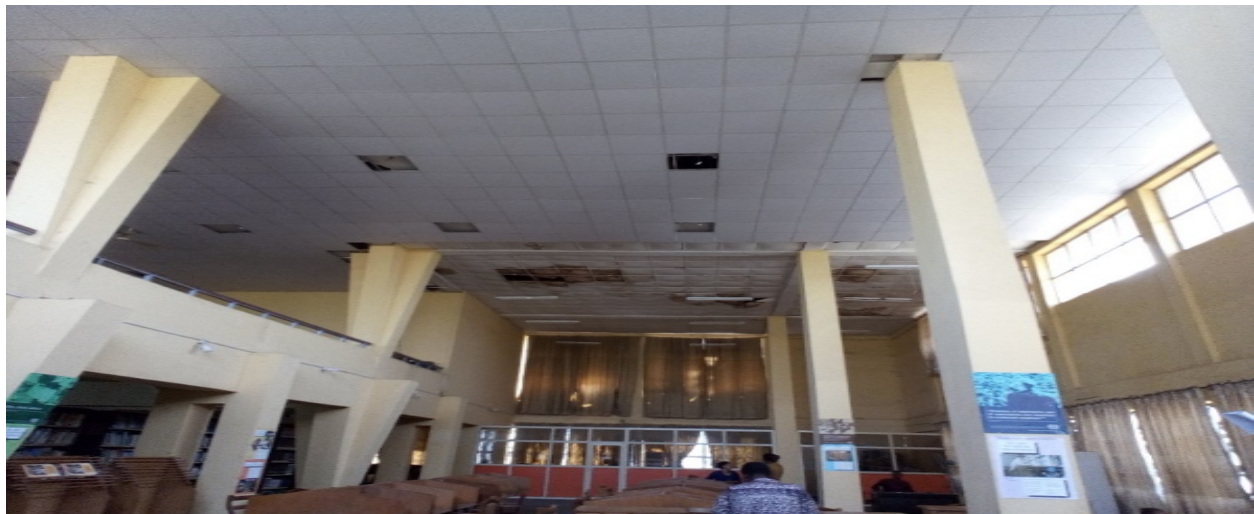
Picture 219: Rehabilitation of Auditorium / library at Micheal Imodu National Institute for Labour Studies.
