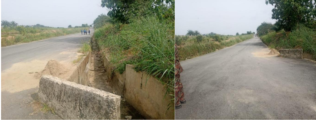
Picture 34: Completed Construction of Basin Town Community Erosion Control Works, Calabar
