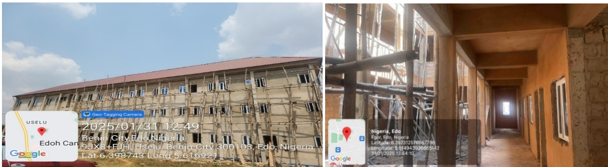
Picture 139: Ongoing Construction of Optometry Building at University of Benin, Edo State.
