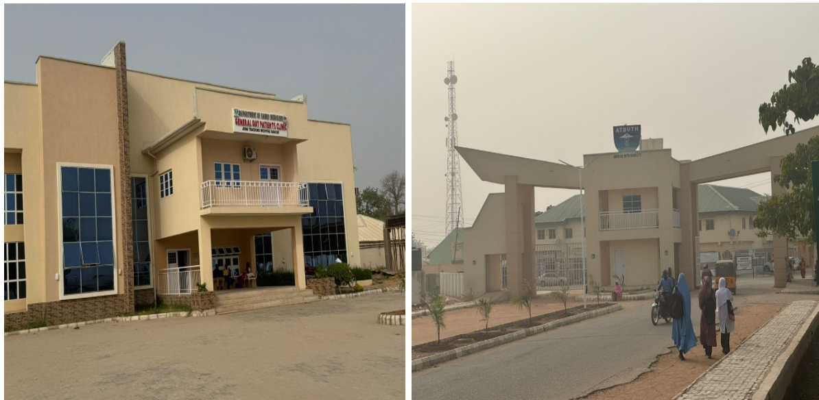
Picture 99: Completed Family Medicine Complex at the ATBU Teaching Hospital, Bauchi.
