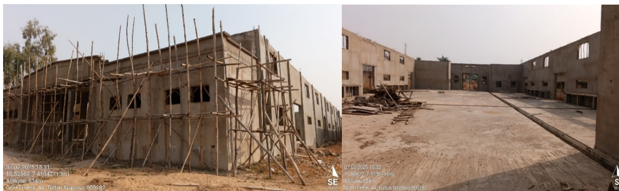
Picture 193: Ongoing Construction and Equipping of Central Workshop for College of Engineering at Federal Polytechnic, Kaduna.
