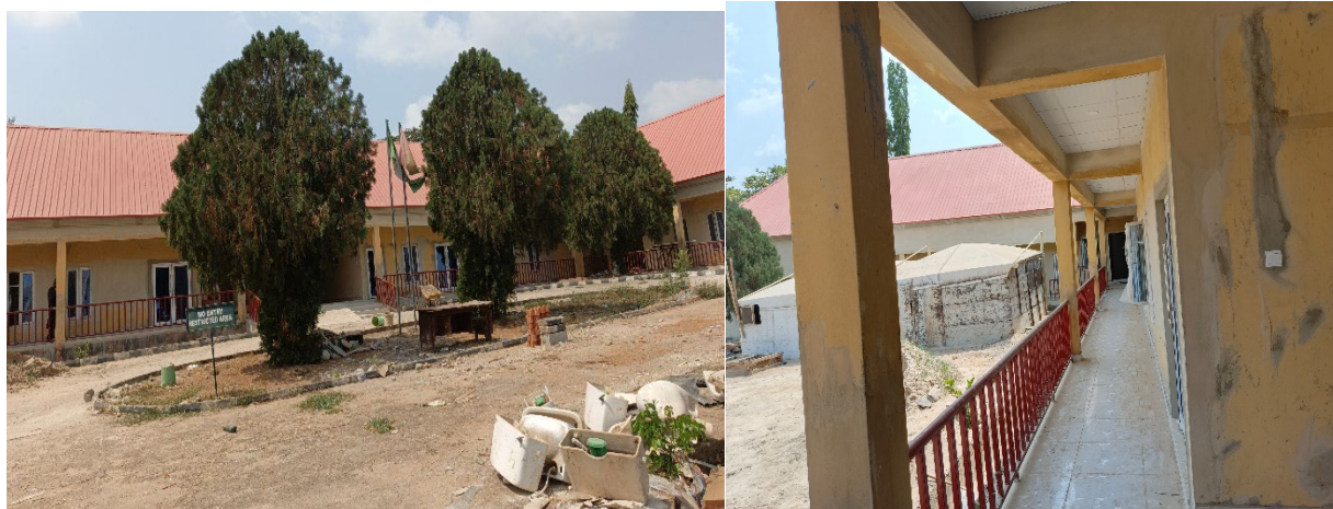
Picture 146: Ongoing Remodelling and Construction of Old Administrative staff offices (phase II) at FCE Abeokuta
