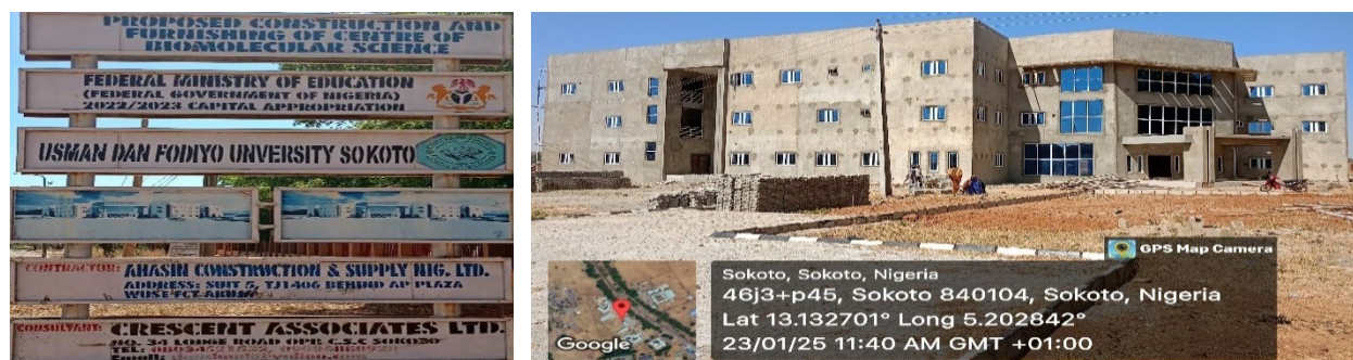
Picture 169: Ongoing construction and furnishing of centre of biomolecular science building at Usman Danfodio University, Sokoto.
