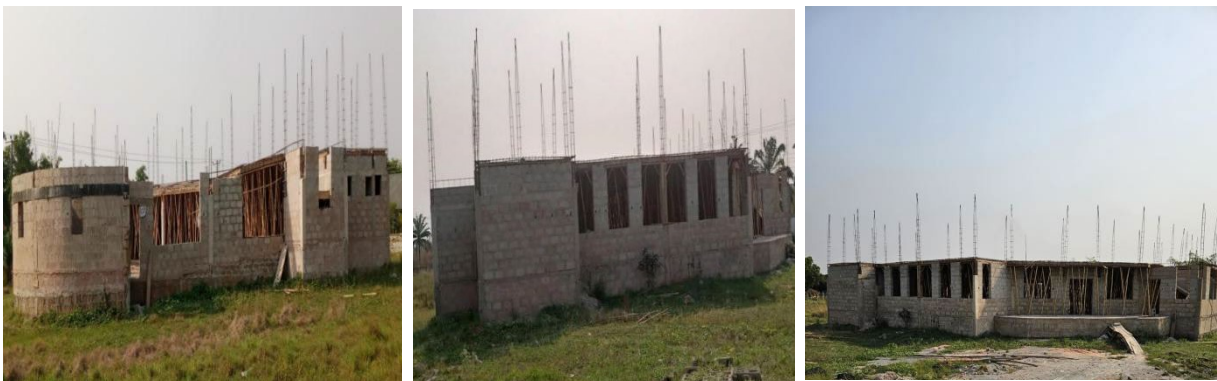
Picture 22: Ongoing Construction of State of the Art" College Lecture Theatre at Federal College of Agriculture, Ishiagu, Ebonyi State.
