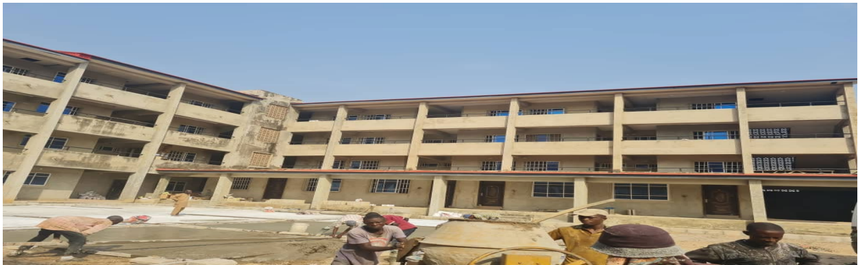
Picture 93: Completed House Officers Residence at University College Hospital, Ibadan.
