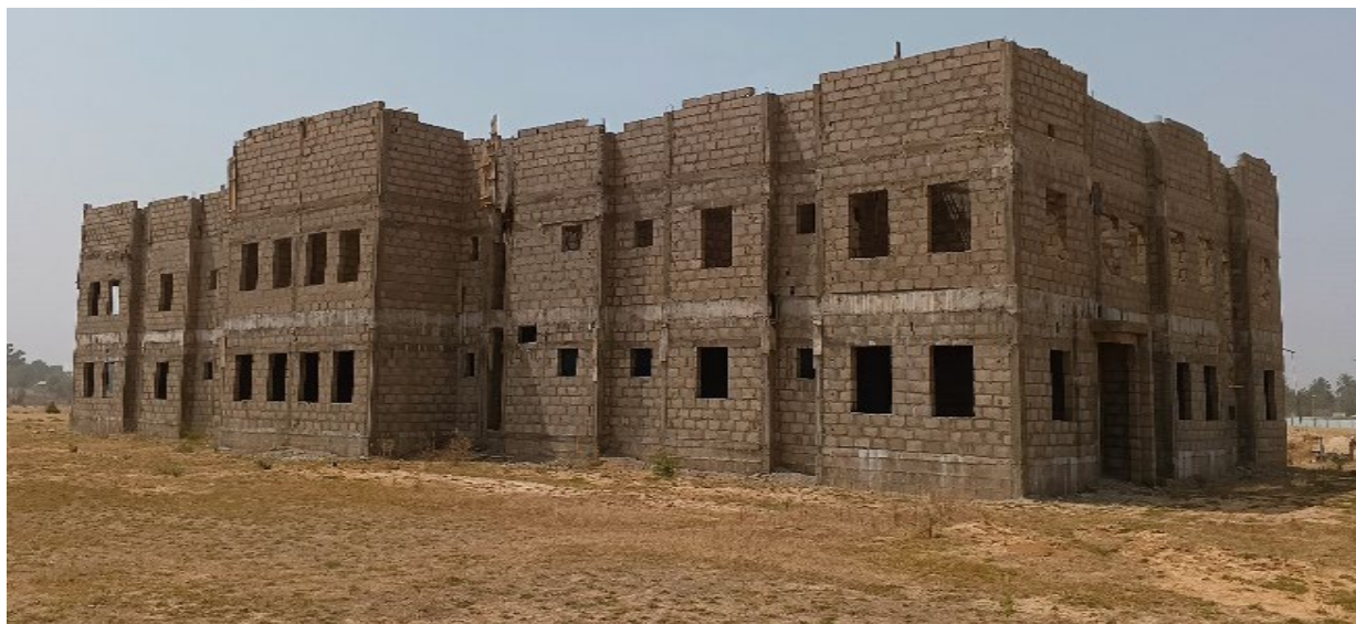
Picture 58: Ongoing Construction of General Administrative Block at FMC, Birnin Kudu
