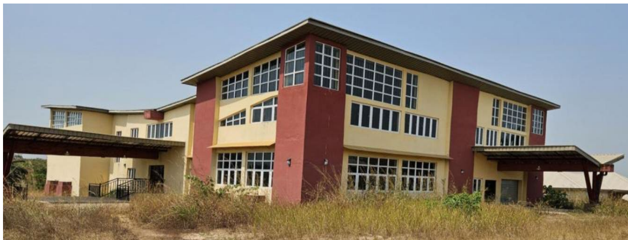
Picture 124: Ongoing Construction of Mechatronics Workshop at Akanu - Ibiam Federal Polytechnic Uwana, Afikpo.
