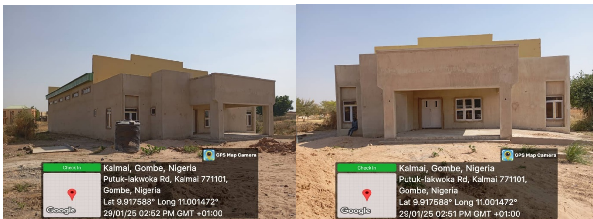
Picture 156: Completed University Main Store at Federal University Kashere, Gombe State.
