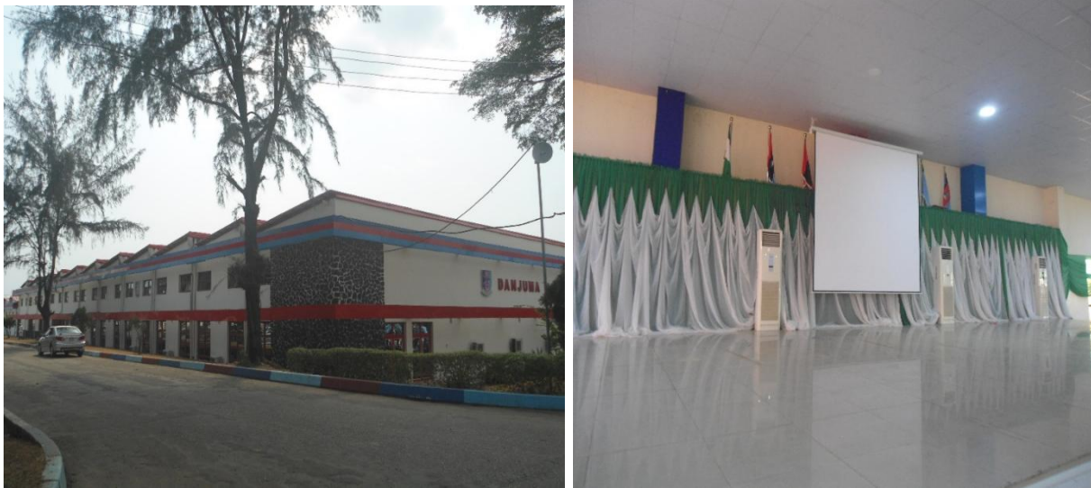
Picture 203: Reroofing /lightening of the Danjuma Hall at NAFRC, Oshodi, Lagos State.
