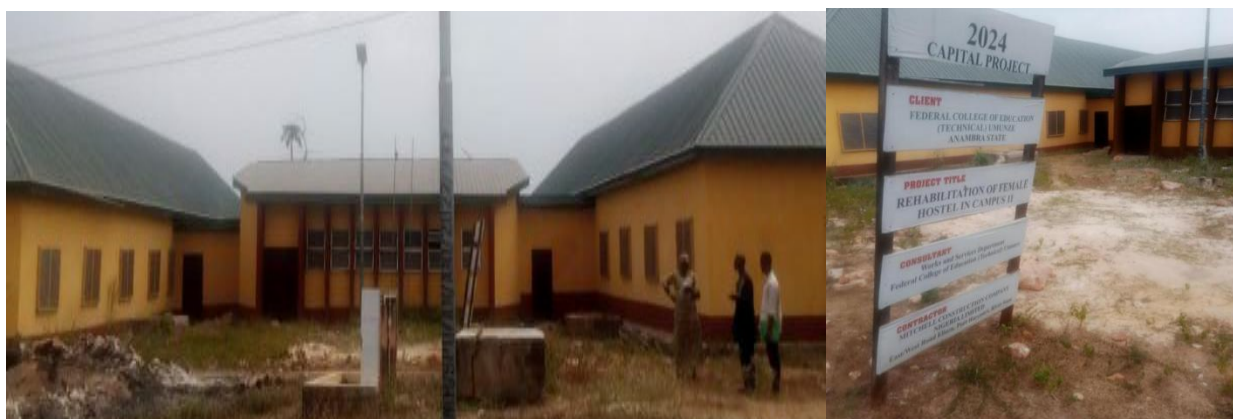
Picture 196: Ongoing Rehabilitation of Female Hostel at Federal College of Education (T), Umunze, Anambra State.
