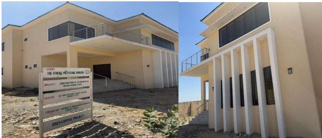
Picture 154: Ongoing Construction of Federal Polytechnic, Monguno Liaison Office, Maiduguri, Borno State.
