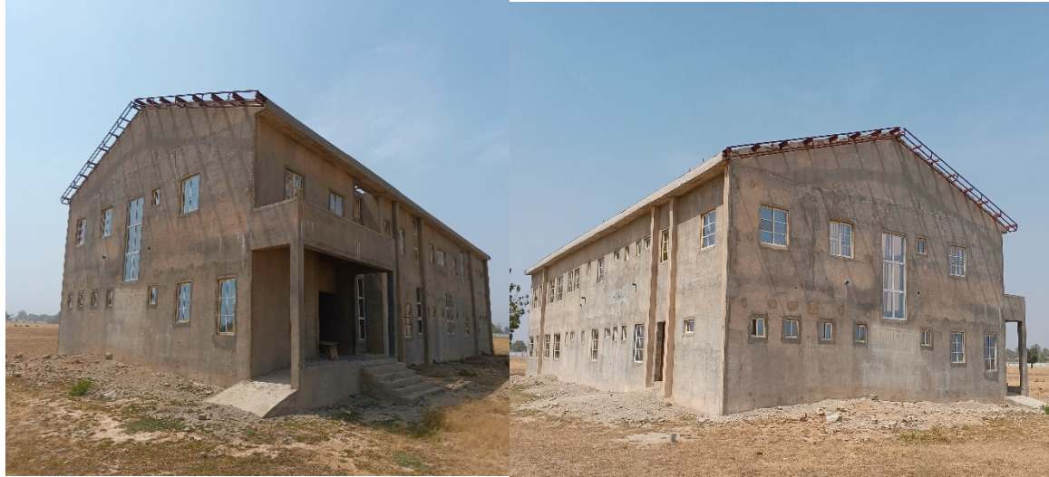
Picture 56: Ongoing Construction of Pediatric Clinic/Ward at FMC Birnin Kudu.
