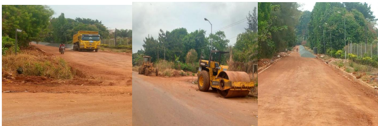
Picture 122: Ongoing Rehabilitation of Louis Mbanefo Street Road at University of Nigeria Nsukka.
