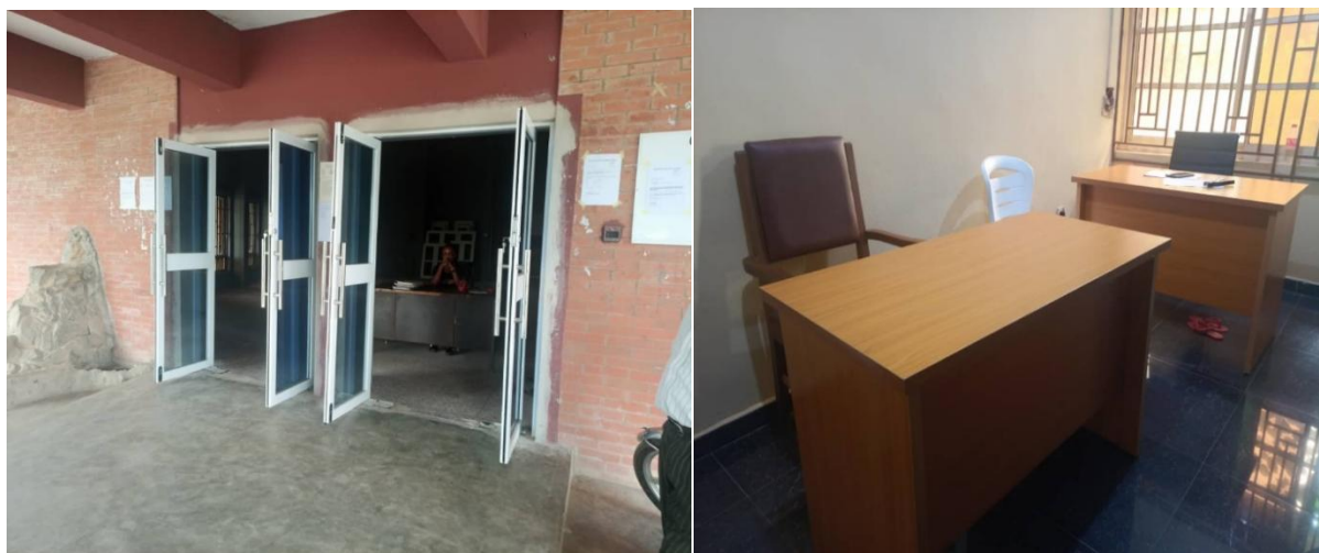
Picture 36: Completed replacement of aluminum swing doors at the CRBDA Headquarters
