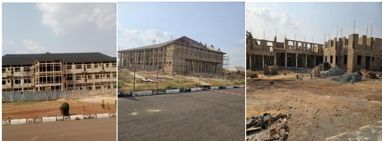
Picture 67: Ongoing Upgrade of Administrative Block and Auditorium at Federal College of Dental Technology and Therapy, Enugu.
