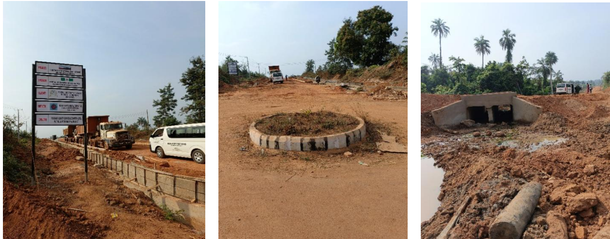
Picture 150: Ongoing Construction of Internal Roads Network, Drainages and Land Scaping at the Federal University of Health Sciences, Ila-Orangun permanent site.
