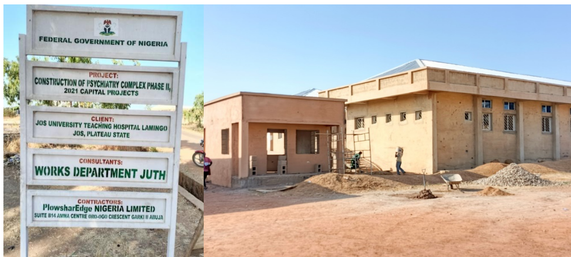
Picture 114: Ongoing Psychiatric Complex at Jos University Teaching Hospital.
