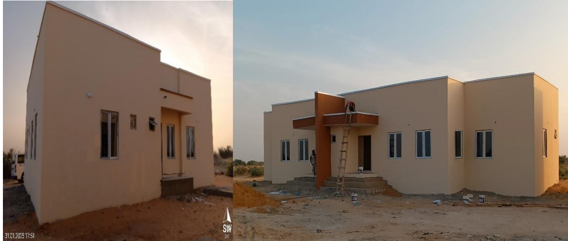
Picture 168: Completed Staff Housing Units at Federal University of Technology Babura, Jigawa State.
