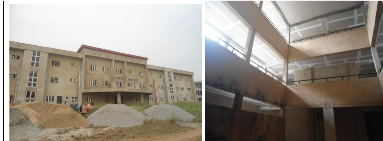
Picture 91: Ongoing Construction of Accident and emergency block at National Orthopedic Hospital, Igbobi, Lagos State.
