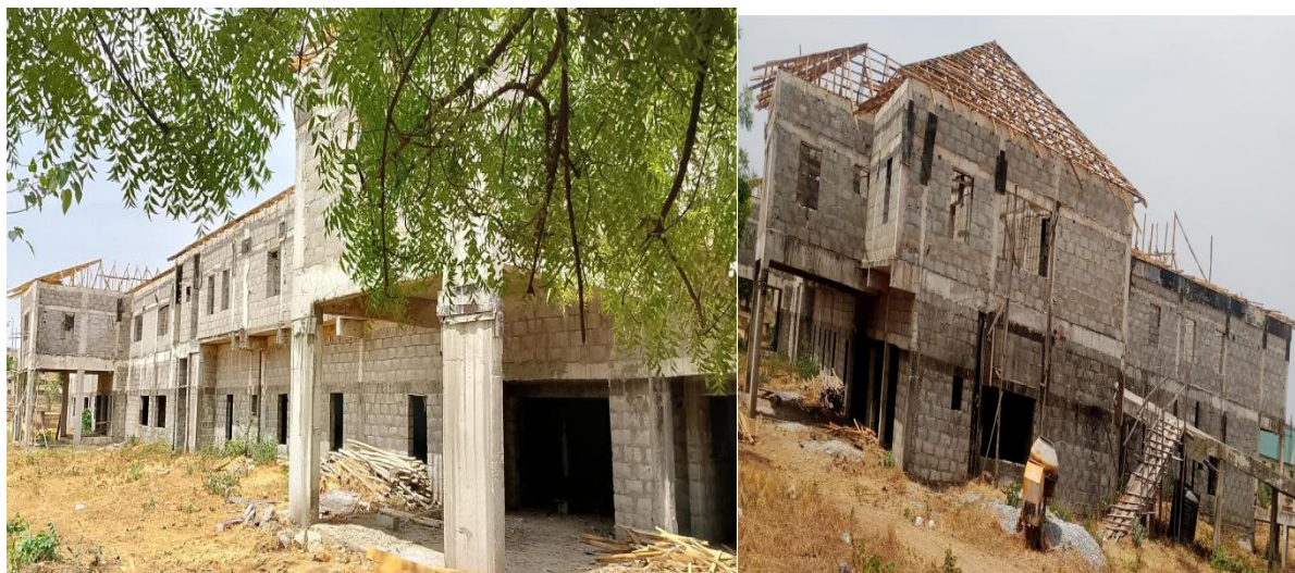
Picture 232: Ongoing Construction and Equipping of Clinic at Nigeria Immigration Service Headquarters, Abuja.
