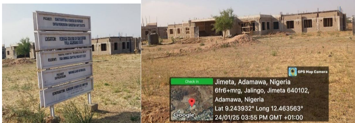
Picture 162: Ongoing Construction of Centre for Basic Entrepreneurship Education at FCE, Yola.
