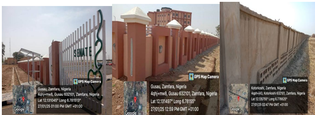
Picture 171: Completed Senate Fence/Gate and ongoing construction of 9km perimeter fencing wall at Federal University, Gusau.
