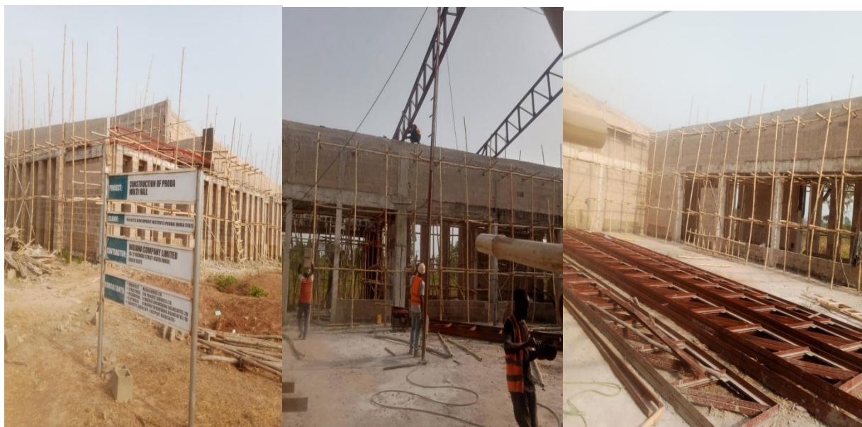
Picture 214: Ongoing Construction of PRODA Multipurpose Hall at Project Development Institute, Enugu State.
