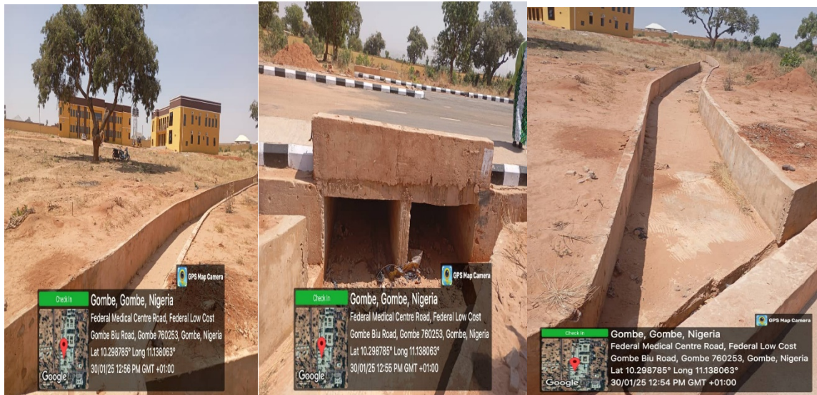
Picture 108: Completed Construction of Erosion Control and Drainage at FTH Gombe.
