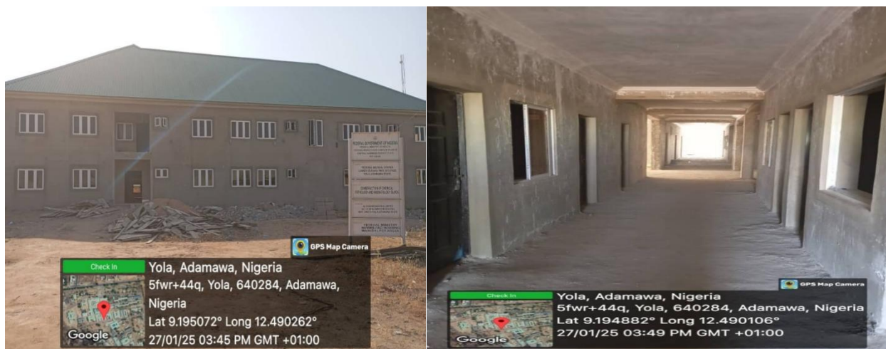
Picture 110: Completed Hematology and chemical pathology laboratory block at Teaching Hospital, Yola.
