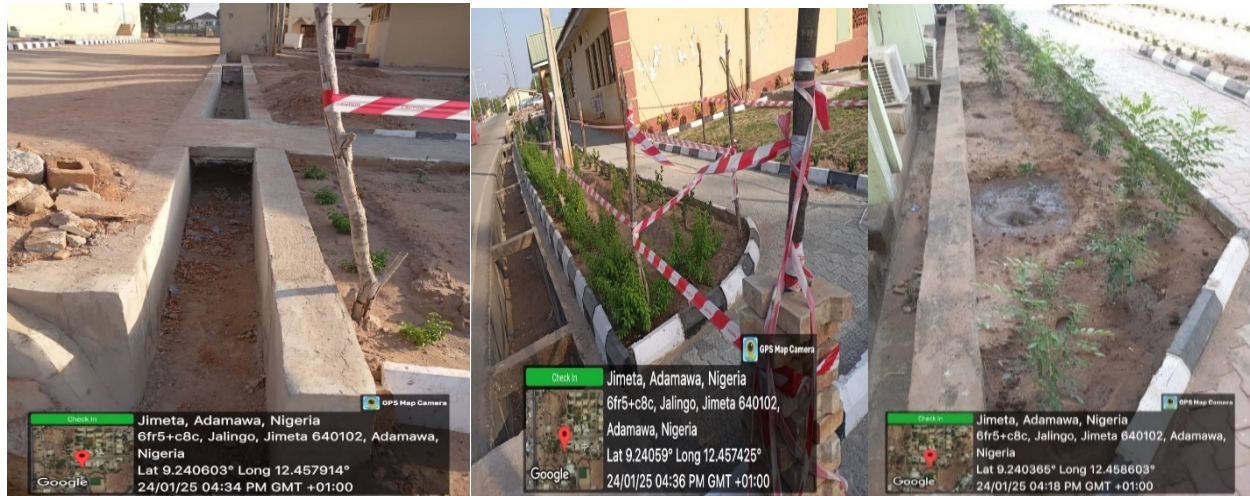
Picture 160: Constructed portion of drainage for erosion control at FCE, Yola.
