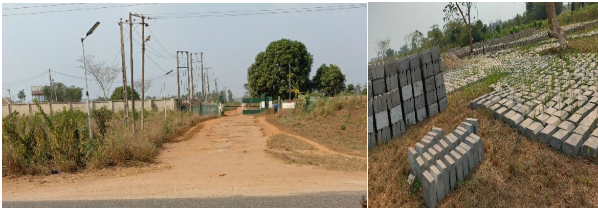
Picture 152: Moulded Blocks and Kerbs for Rehabilitation of 1000m Gbokoto Road at Federal Polytechnic, Ilaro
