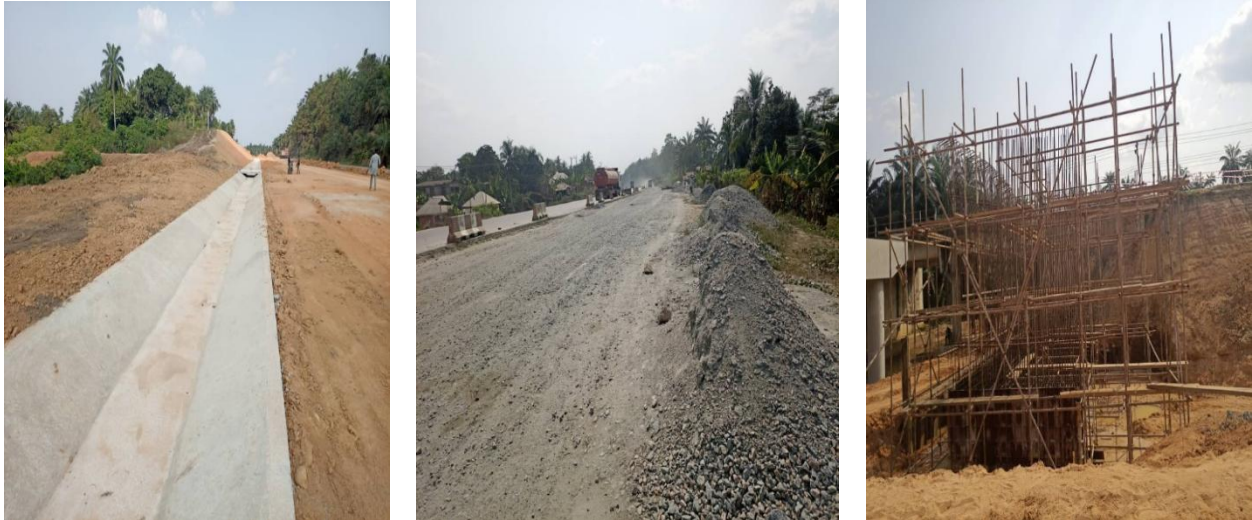
Picture 4: Ongoing Dualization of the Oku Iboku- power plant section of the Odukpani Junction- Itu- Ikot Ekpene Road in Cross River / Akwa Ibom States.
