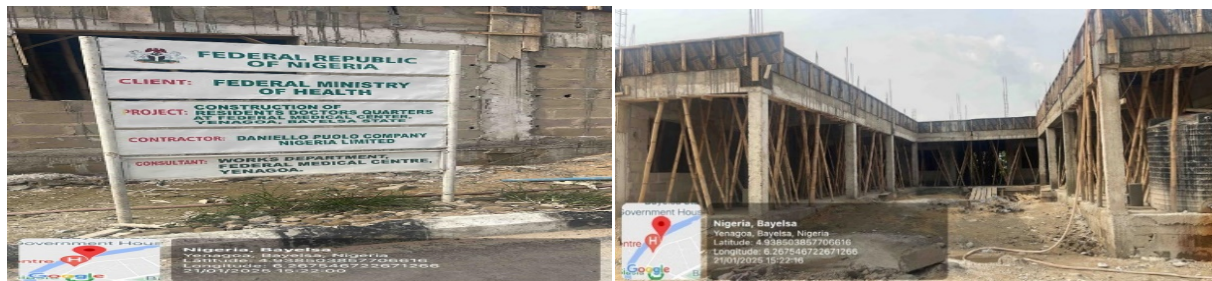
Picture 82: Ongoing Construction of Resident Doctors' Quarters at Federal Medical Centre, Yenegoa, Bayelsa State.
