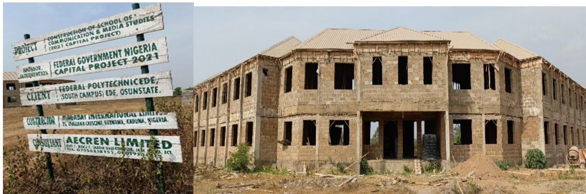
Picture 145: Ongoing Construction of Communication and Media Studies Department at Federal Polytechnic, Ede, Osun State.
