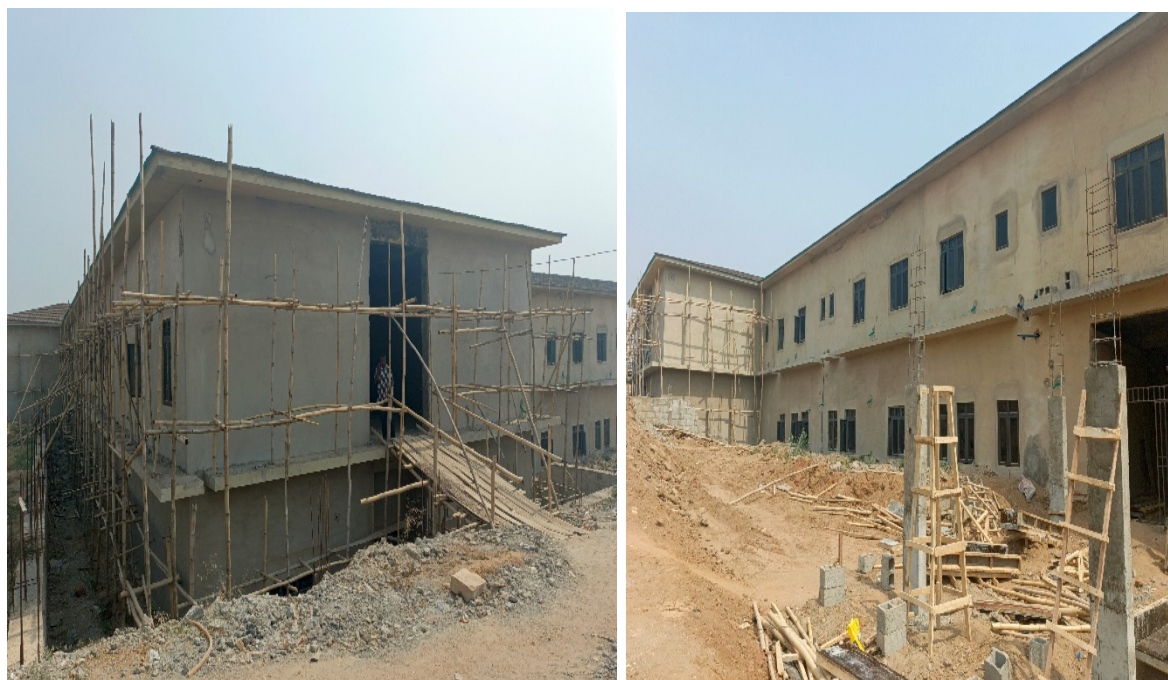
Picture 204: Ongoing Construction of Defence Reference Hospital at Abacha Barracks, Abuja.
