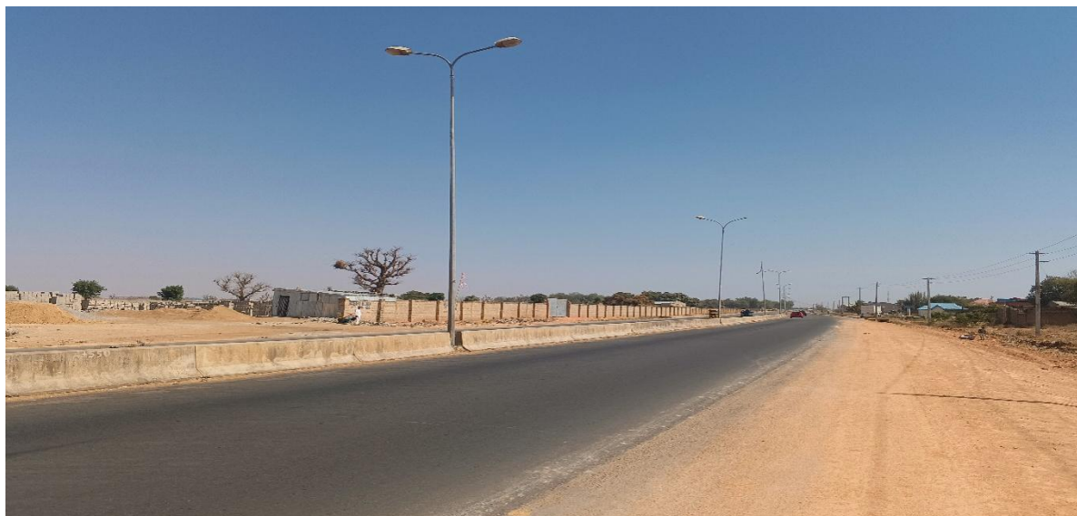
Picture 15: Dualization of Kano-Katsina Road Phase 1
