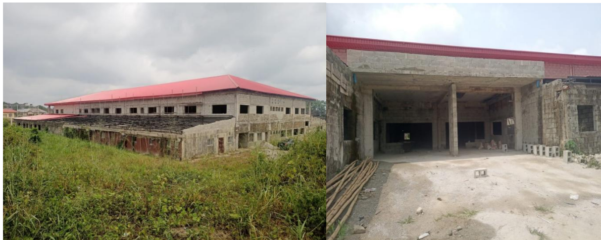
Picture 72: Ongoing Completion of Accident and Emergency (A&E) at University of Calabar Teaching Hospital.
