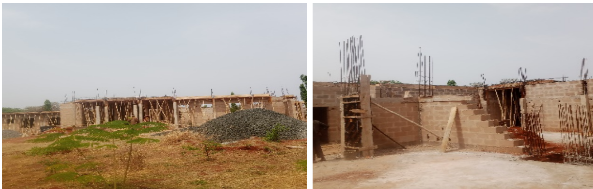
Picture 63: Ongoing Construction of Theatre at National Orthopedic Hospital, Enugu.
