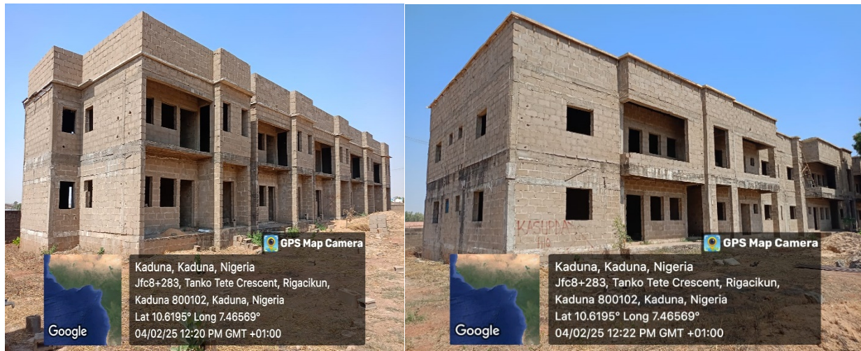
Picture 50: Ongoing Construction of Post Graduate Hostel at National Eye Centre, Kaduna.
