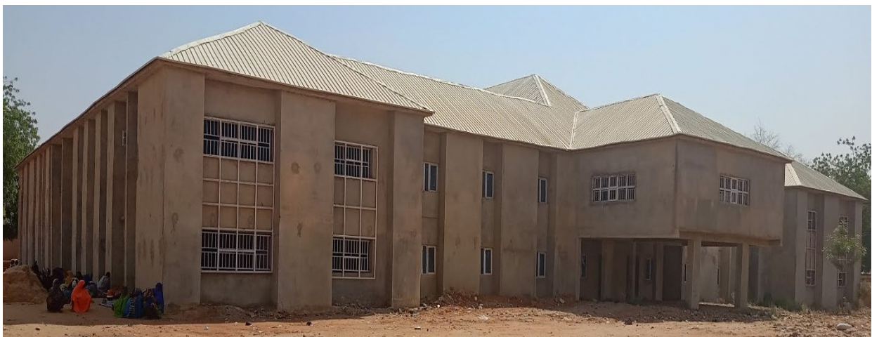
Picture 43: Ongoing construction and finishing of a-storey Administrative block at the FMC, Birnin Kebbi
