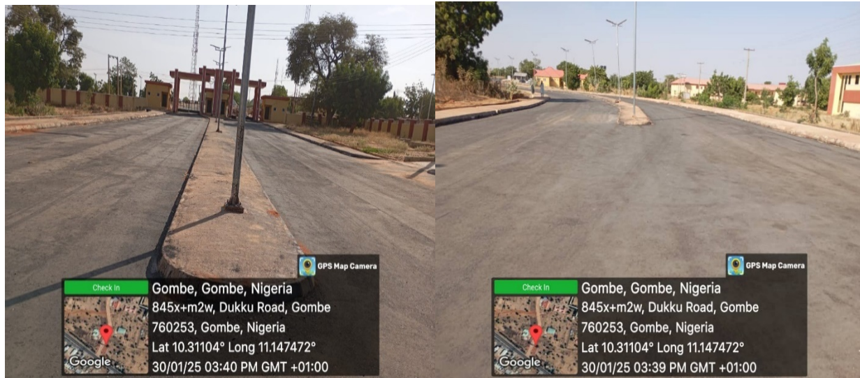
Picture 158: Completed 1.6km asphalt road with drainages at the Federal College of Education, Gombe.
