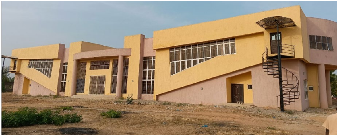
Picture 175: Constructed & Furnishing of 250 Twin Theatre at Federal University Dutse, Jigawa State.
