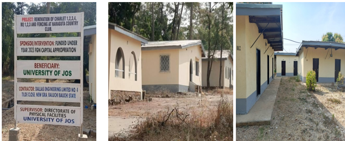
Picture 166: Completed Renovation of Naraguta Country Club at UniJos.
