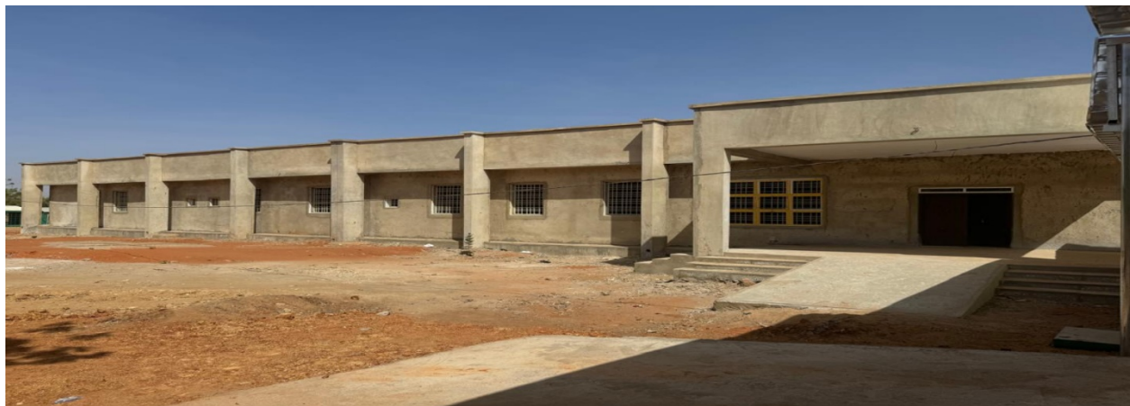
Picture 104: Completion of Specialty Clinic & GOPD at Permanent Site at Federal University of Health Sciences Teaching Hospital, Azare, Bauchi State
