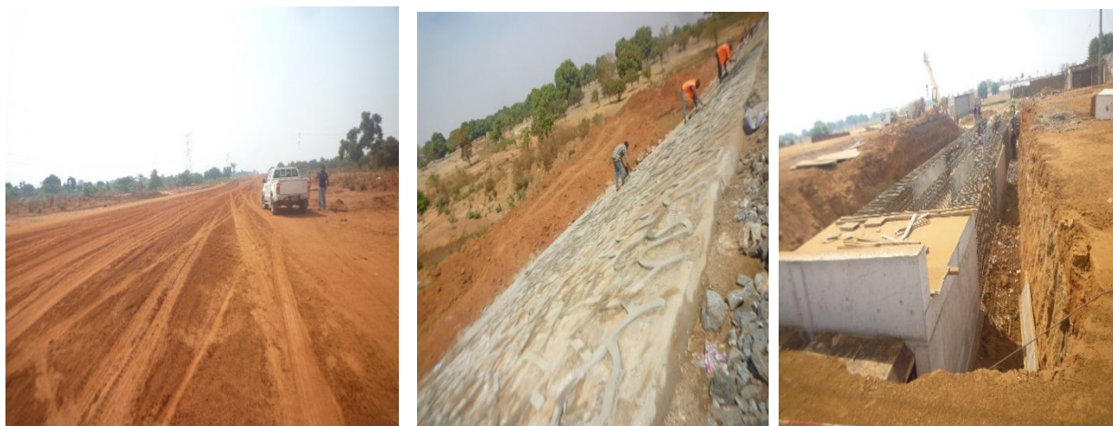
Picture 12: Ongoing Construction of Lafia Bypass from Nasarawa to Benue State.
