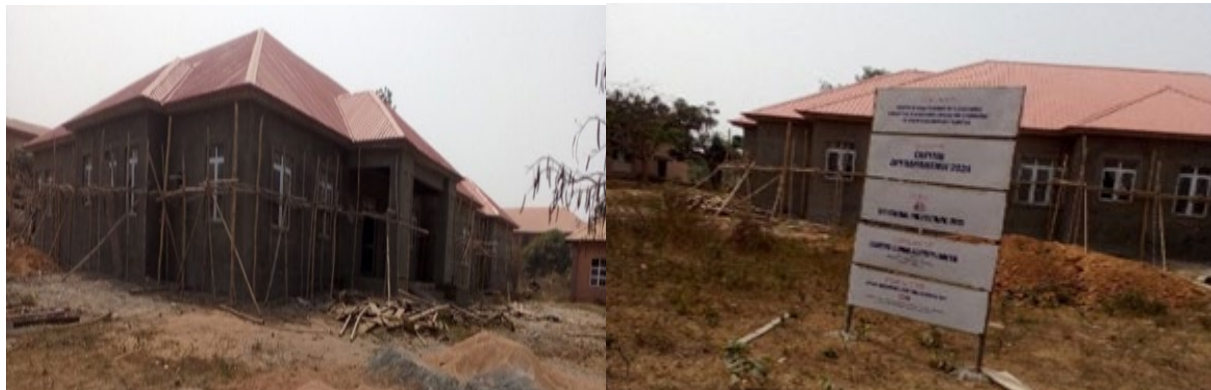
Picture 184: Ongoing construction of Classroom and Office Accommodation at Federal Poly, Offa.
