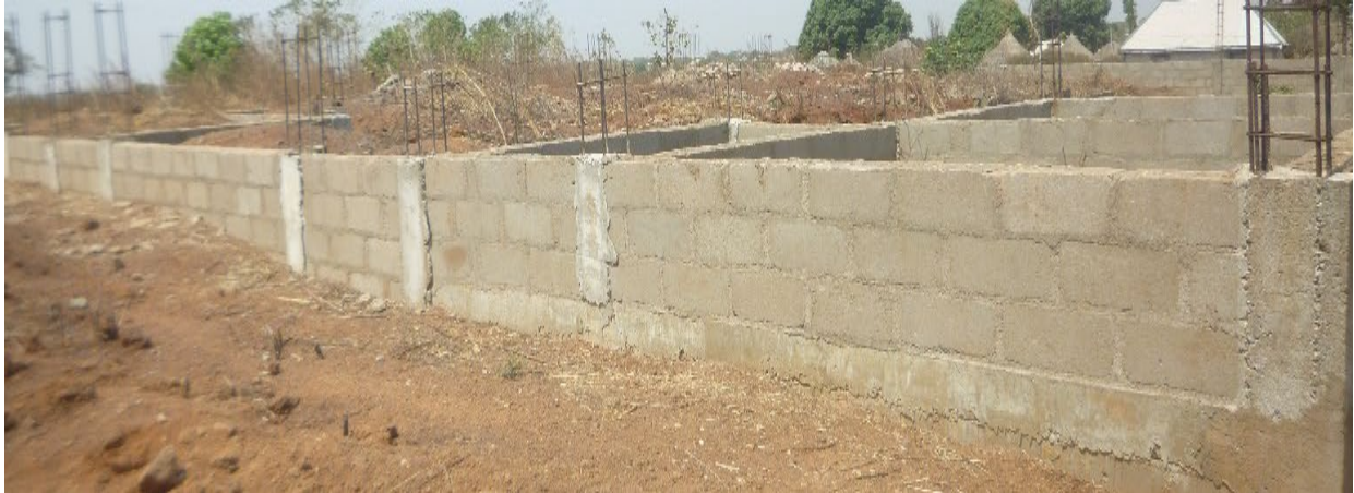
Picture 177: Ongoing Construction of Skill Acquisition Workshop at Federal Polytechnic, Wannune.
