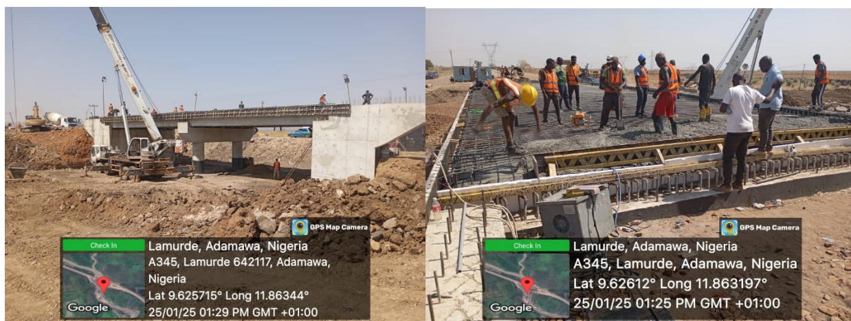
Picture 10: Rehabilitation of Cham-Numan section of Gombe - Yola roads in Adamawa State Contract No. 6300
