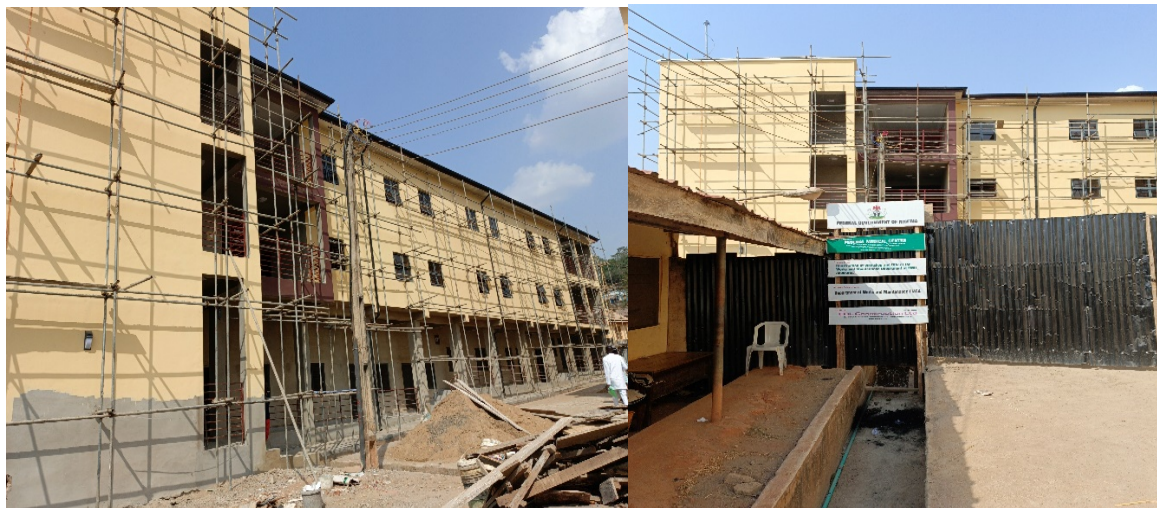
Picture 96: Ongoing Upgrading of Workshop and Offices for Works and Maintenance Unit at Federal Medical Centre, Abeokuta.
