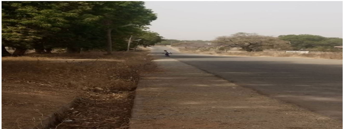
Picture 33: Ongoing rehabilitation/ repair of access road and drainages
