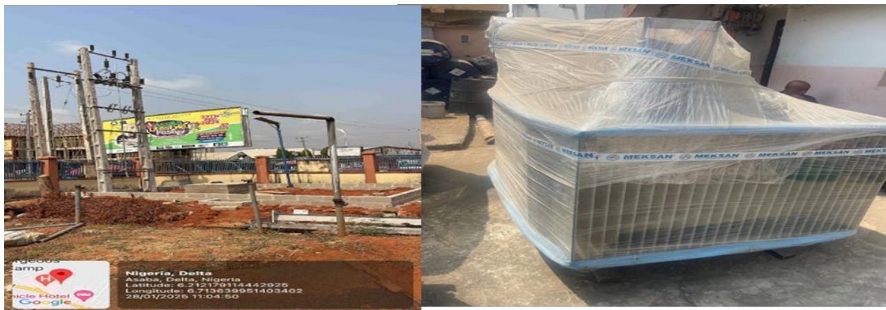
Picture 85: Ongoing construction of 1.5mva Power Sub-Station at FMC, Asaba, Delta State
