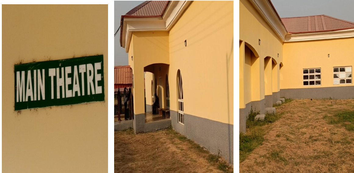
Picture 115: Completed renovation of Male /Female Surgical/theatre at FMC, Makurdi.
