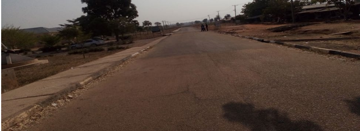
Picture 179: Completed 3km road network at Federal Polytechnic, Bida
