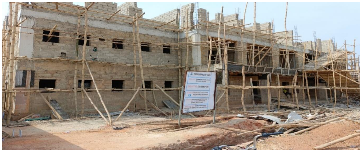
Picture 94: Ongoing Construction of 150 bedded ward at Federal Teaching Hospital, Ido – Ekiti.
