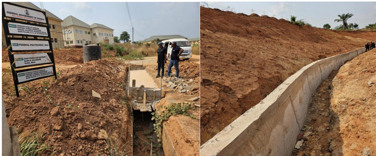
Picture 129: Ongoing Construction of Retaining Walls for Erosion Control at New Extension site, Federal Polytechnic, Oko.
