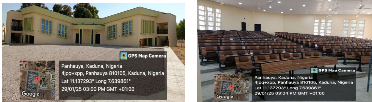
Picture 170: Completed 500-Seater Student Lecture Hall at Ahmadu Bello University, Zaria.
