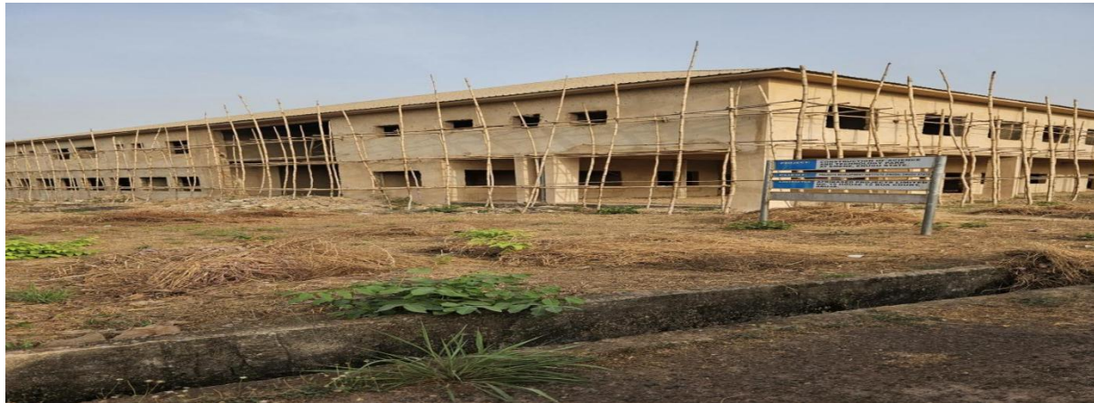
Picture 215: Ongoing Construction of PRODA Science and Technology Park, at PDI, Enugu State.
