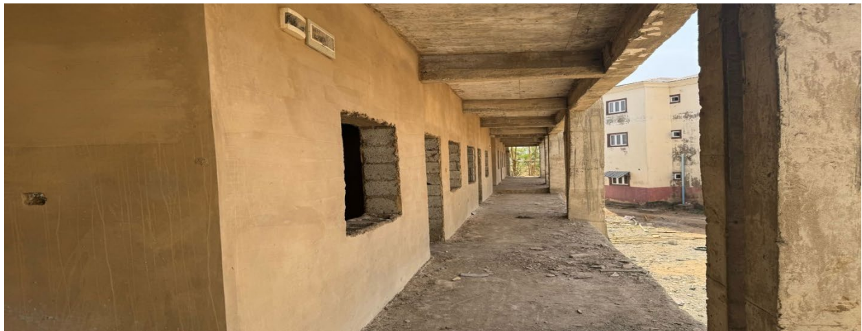
Picture 231: Ongoing Construction of Barracks at NSCDC Headquarters, Abuja.
