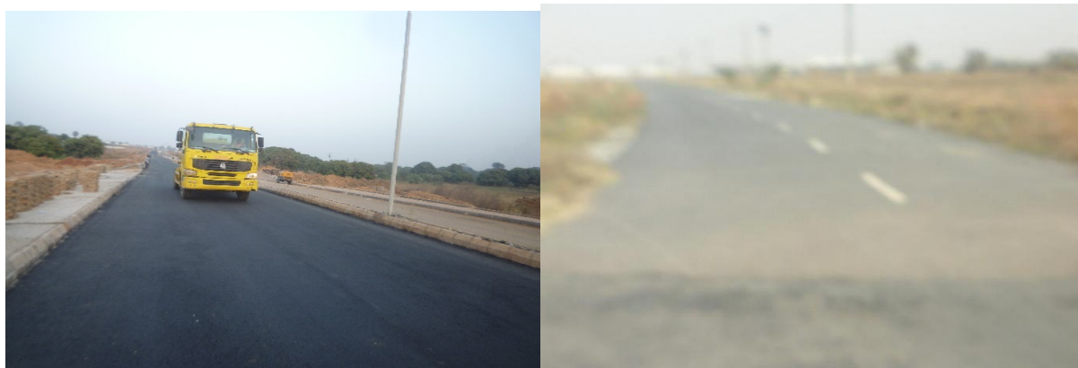
Picture 13: Completed Keffi-Akwanga-Lafia Makurdi Road in Nasarawa and Benue States.
