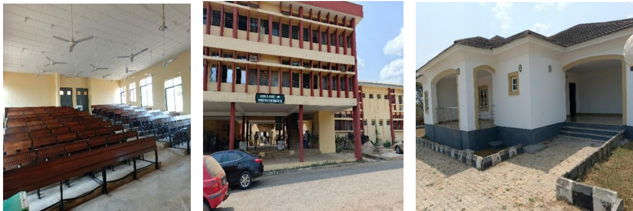
Picture 24: Rehabilitated School Building at Federal University of Agriculture Abeokuta.
