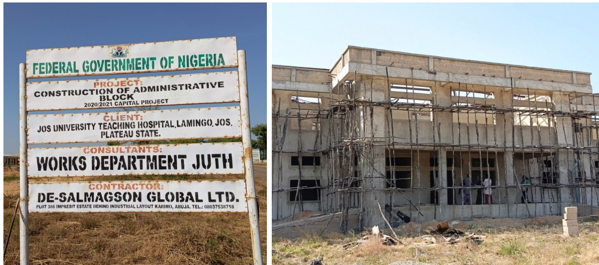
Picture 113: Ongoing construction of Admin. block at Jos University Teaching Hospital.
