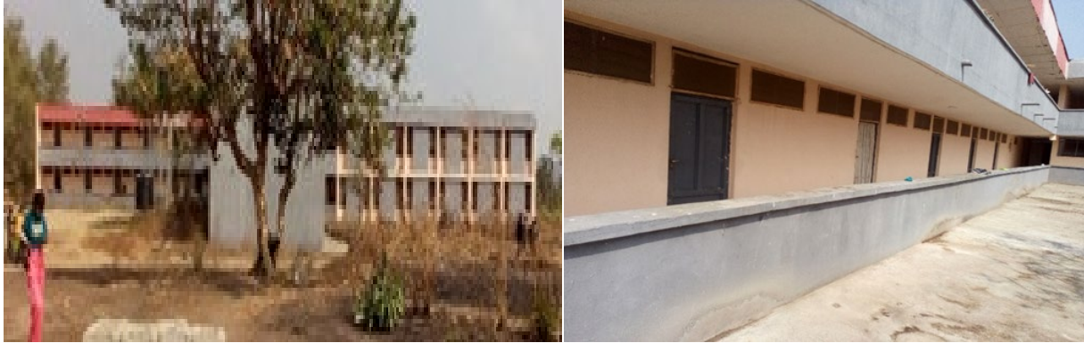
Picture 182: Completed renovation of Male Hostel C and D at FCE, Okene.
