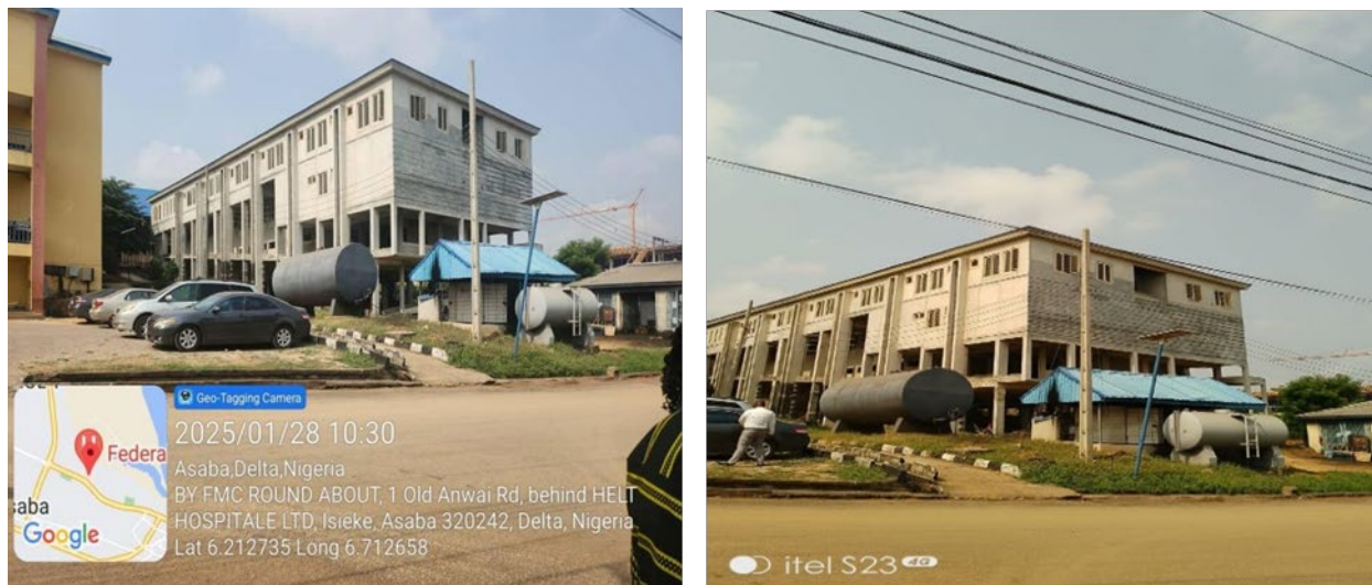
Picture 88: Ongoing construction of Male and Female ward at FMC, Asaba, Delta State
