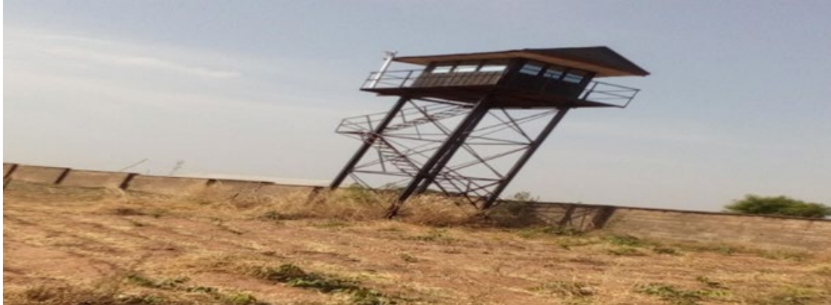
Picture 181: Constructed Security Watch Tower at the Federal Polytechnic, Bida.
