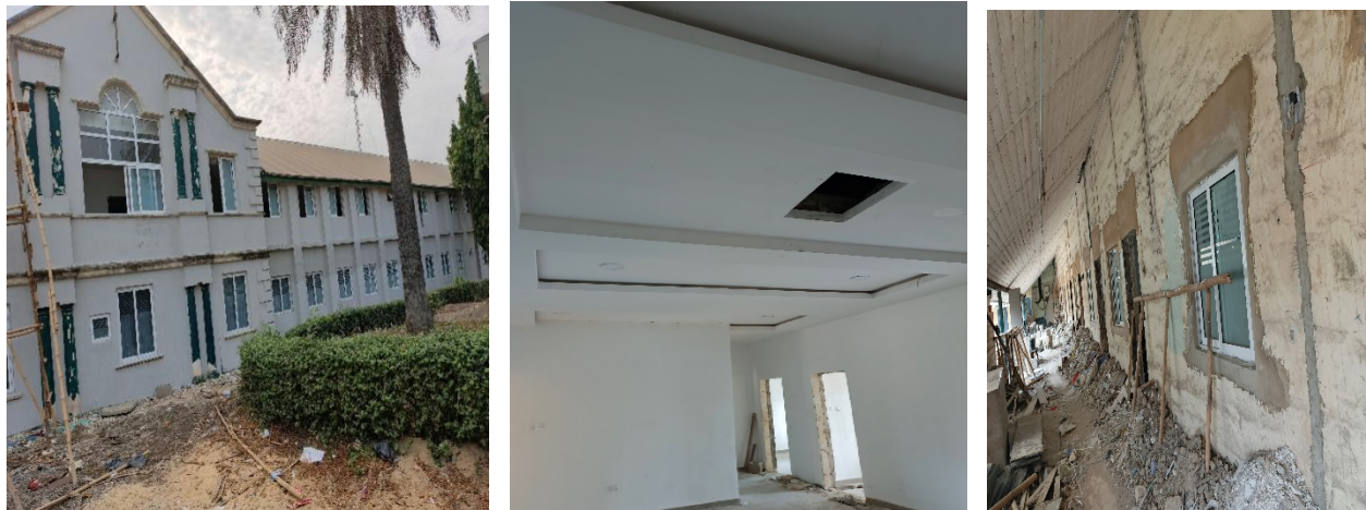
Picture 208: Ongoing rehabilitation of railway building at Nigerian Railway corporation Headquarters, Ebute-Metta, Lagos.
