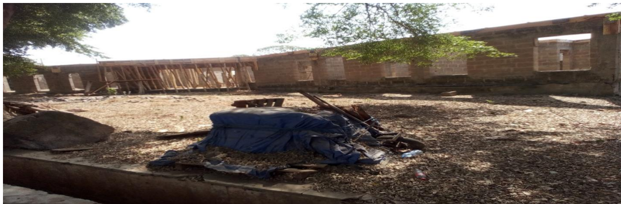
Picture 218: Ongoing Completion of admin block at Michael Imodu Institute, Ilorin
