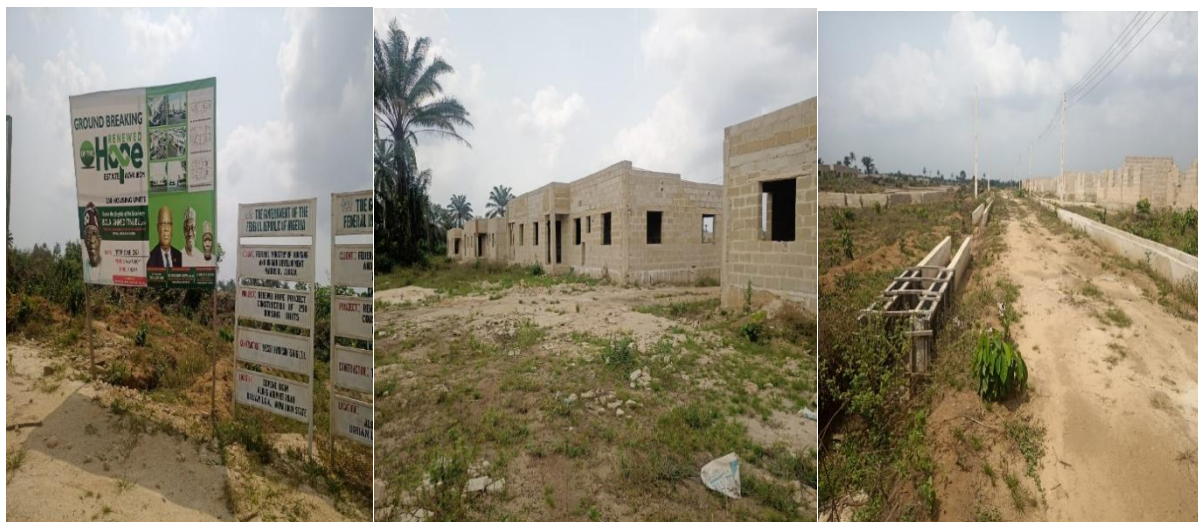
Picture 19: Ongoing Renewed Hope Agenda Housing Scheme at Uyo Cross Rivers.
