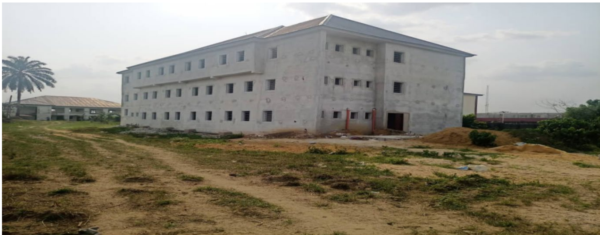
Picture 71: Ongoing Completion of Interns hostel at University Port-Harcourt Teaching Hospital, River State.
