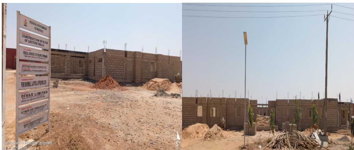
Picture 212: Ongoing Construction of Lecture Halls at Federal University Technology, Daura, Katsina State.
