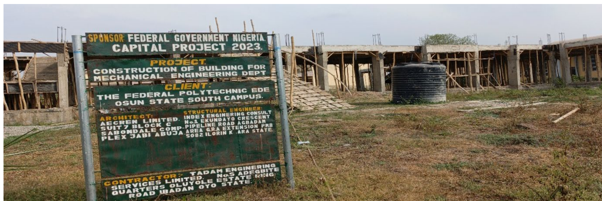
Picture 143: Ongoing Construction of Building for Mechanical Engineering Department at Federal Polytechnic, Ede, Osun State.
