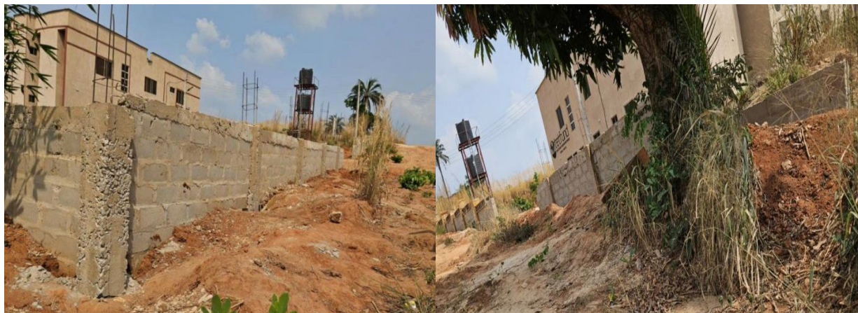
Picture 128: Ongoing Construction of 2km Perimeter Fence for Male and Female Hostel at New Extension site, Federal Polytechnic, Oko.
