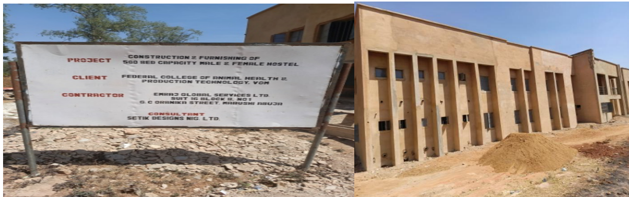
Picture 31: Ongoing construction and furnishing of 500 bed Capacity for Male and Female Students hostel.
