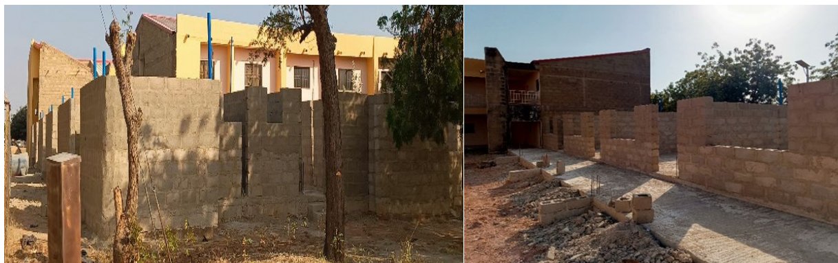
Picture 189: Ongoing Construction of Administrative Block at Federal College of Education, Kastina.
