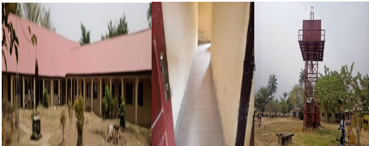
Picture 131: Ongoing rehabilitation of bursary and registry wing of old administrative block at the main campus phase II Obudu
