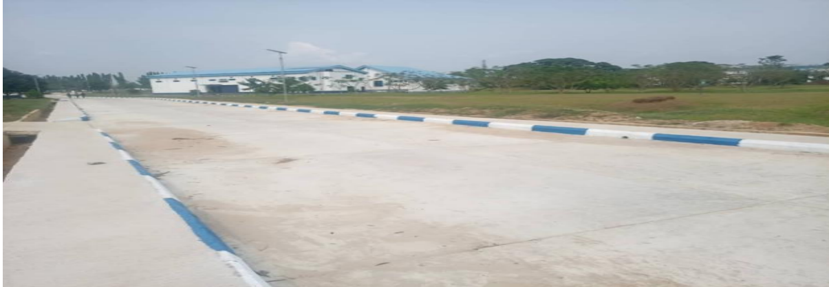
Picture 224: Completed Internal Road with streetlights at the Maritime Academy Oron.
