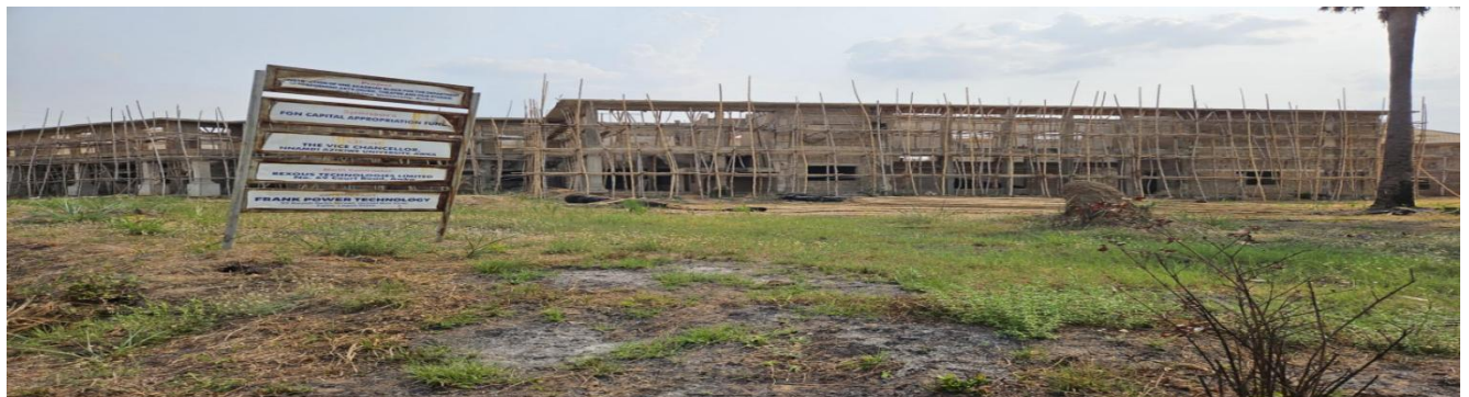
Picture 127: Ongoing Construction of Performing Arts, Music theater and film studies Department at Nnamdi Azikwe University, Awka.
