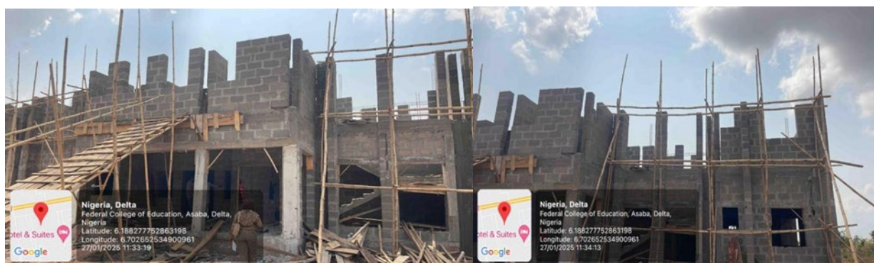
Picture 140: Ongoing Construction of Administrative Department Office at Federal College of Education (Tech.), Asaba, Delta State.
