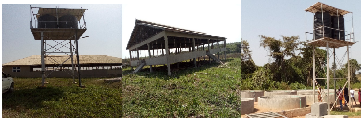
Picture 76: Constructed goat ranch, layer's pen, fish ponds and boreholes
