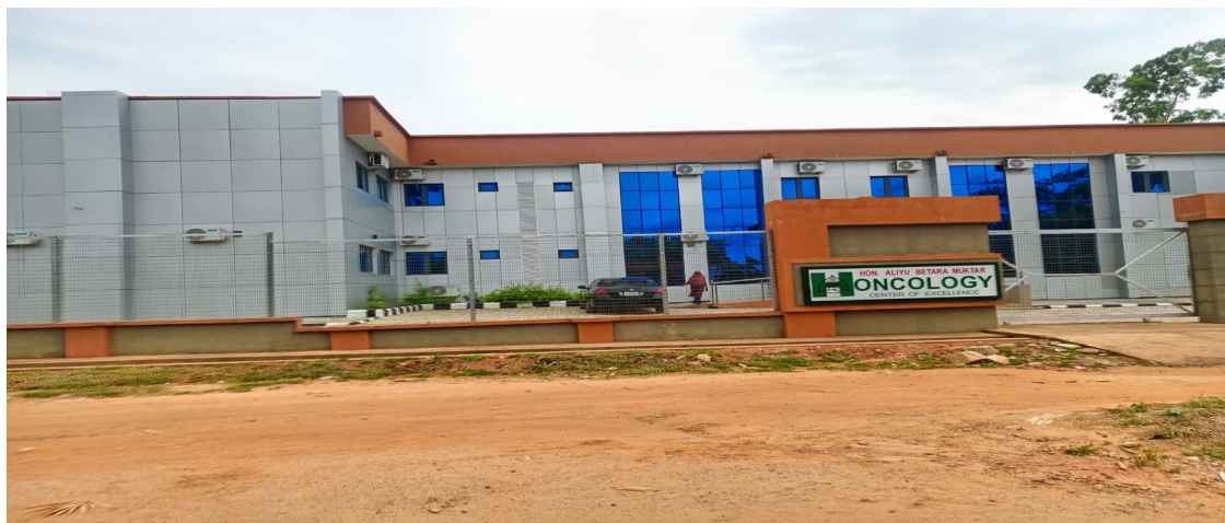
Picture 48: Constructed oncology/radiotherapy Centre at ABUTH, Zaria.
