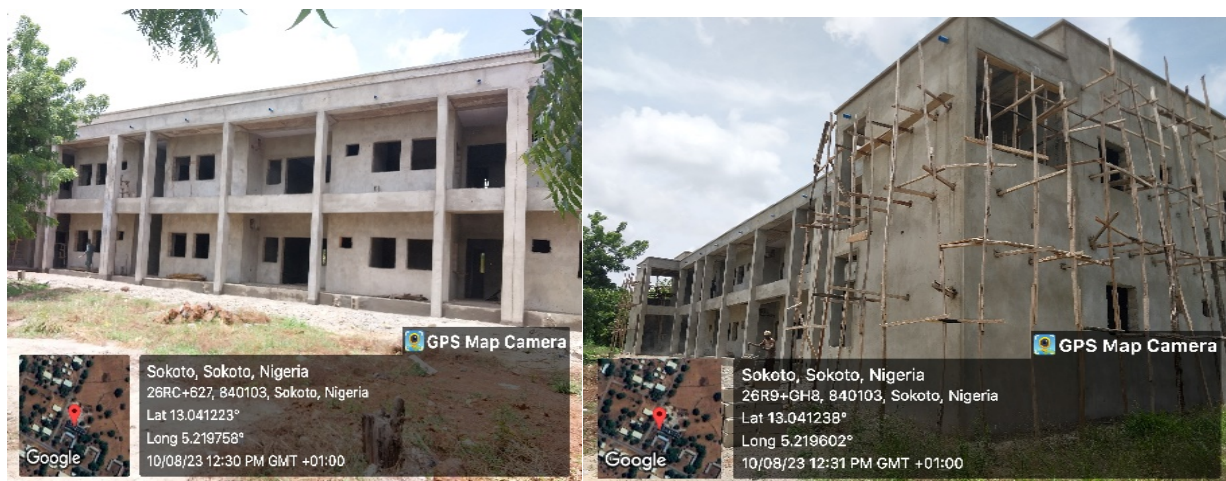
Picture 39: Ongoing Construction and Furnishing of House Officers Quarters At UDUTHS.
