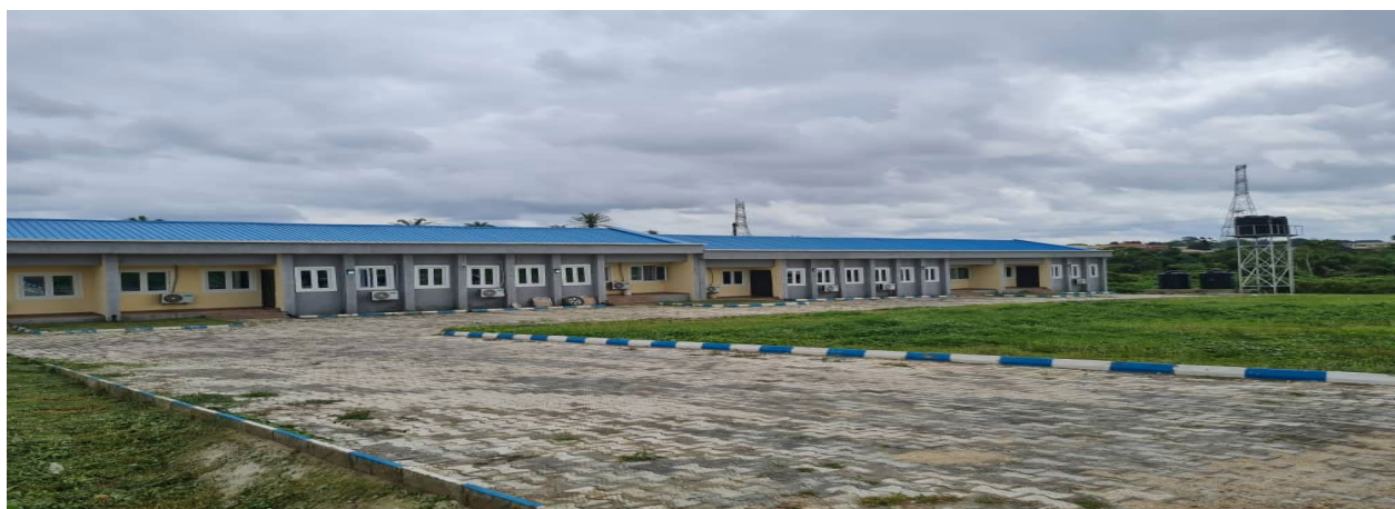
Picture 68: ongoing construction of 2 block of commanders' accommodation with at NAF base Oshogbo.
