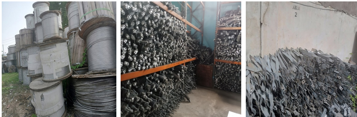
Picture 80: Supplied Materials for the Construction of 33KV Double Circuit Line for Emergency Power Supply from Damaturu to Maiduguri.
