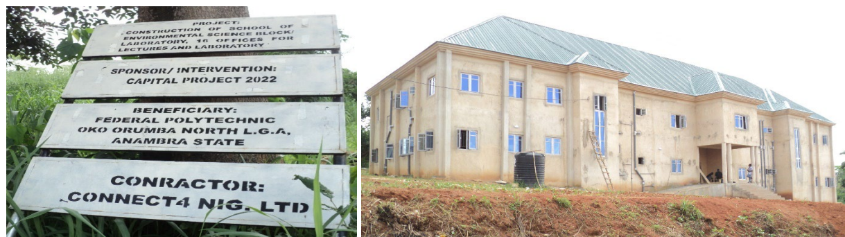
Picture 12: Ongoing Construction of School of Environmental Science Block at the Federal Polytechnic, Oko.
