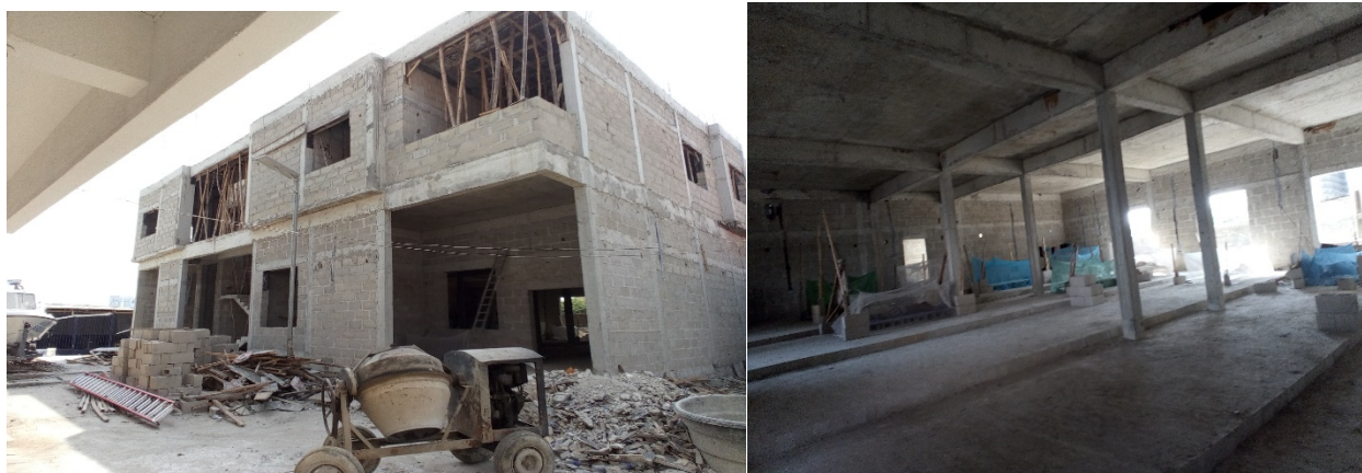
Picture 34: Ongoing construction of marine engineering laboratory extension building
