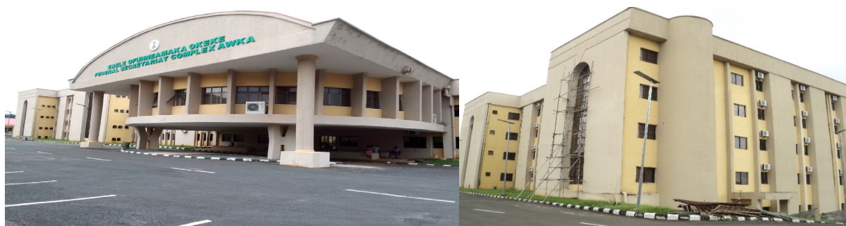
Picture 9: Completed Front and Side View Federal Secretariat Complex at Awka, Anambra State.
