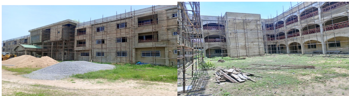
Picture 50: Ongoing construction of 40 flats for nurses and other essential staff at AKTH.
