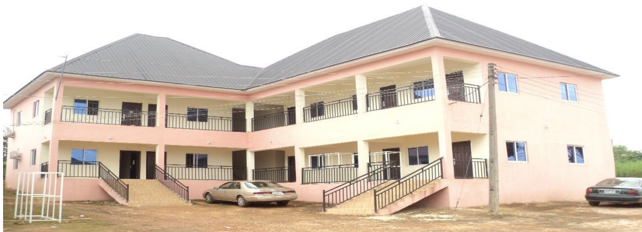
Picture 26: Constructed Lecturers' Office at Federal Cooperative College, Orji – River, Enugu State.
