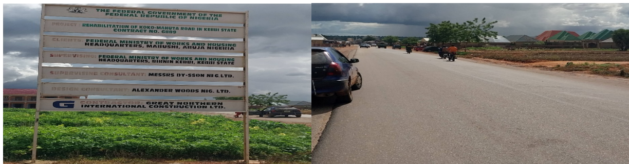
Picture 3: Ongoing Rehabilitation of Koko Mahuta Road (87km) in Kebbi State
