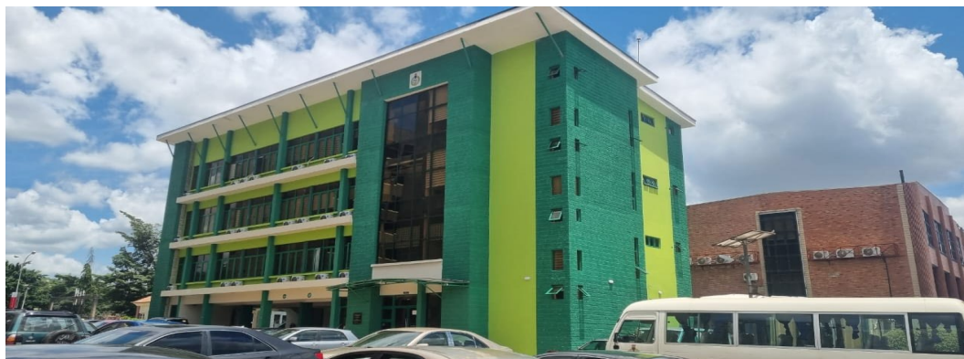
Picture 73: Completed ICT Centre at NYSC Headquarters, Abuja.
