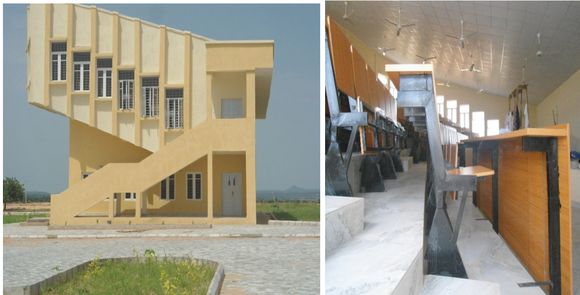
Picture 28: Constructed Lecture theatre at Federal College of Horticulture Dadin Kowa, Gombe.
