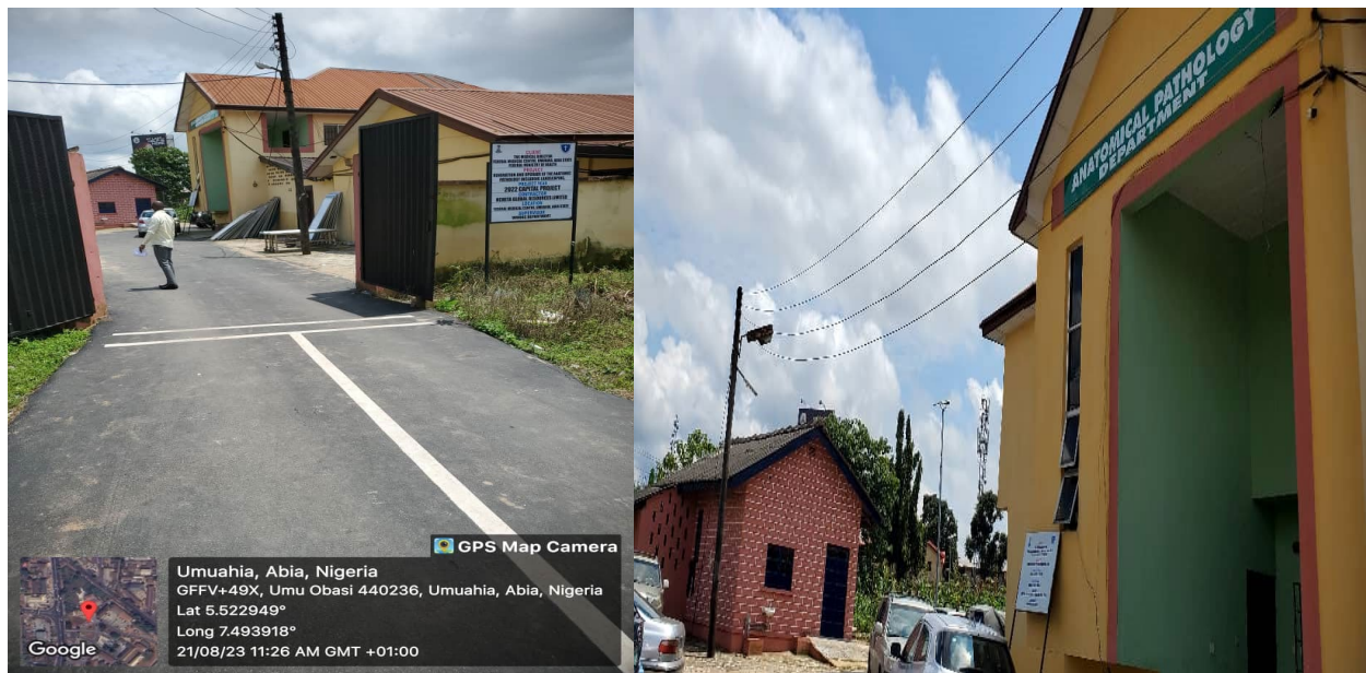
Pictures 36: Completed renovation of the Anatomic Pathology building at FMC, Umuahia
