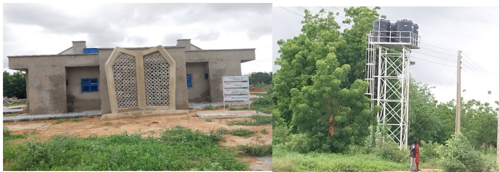
Picture 18: Ongoing Construction of 150 seats capacity lecture theatre for Faculty of Law at the Federal University, Birnin Kebbi.
