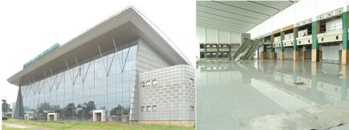
Picture 24: Ongoing Construction of New Terminal Building at Enugu Airport
