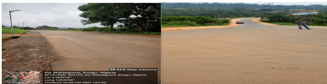
Picture 1: Rehabilitated portion of Old Enugu- Port-Harcourt Road (Agbogugu – Abia Border Spur to Mmaku), Enugu
