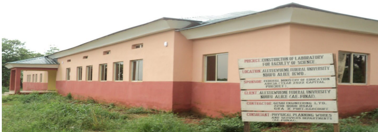
Picture 11: Constructed Bungalow Building for Faculty of Science Laboratory at Alex Ekwueme Federal University, Ebonyi State.
