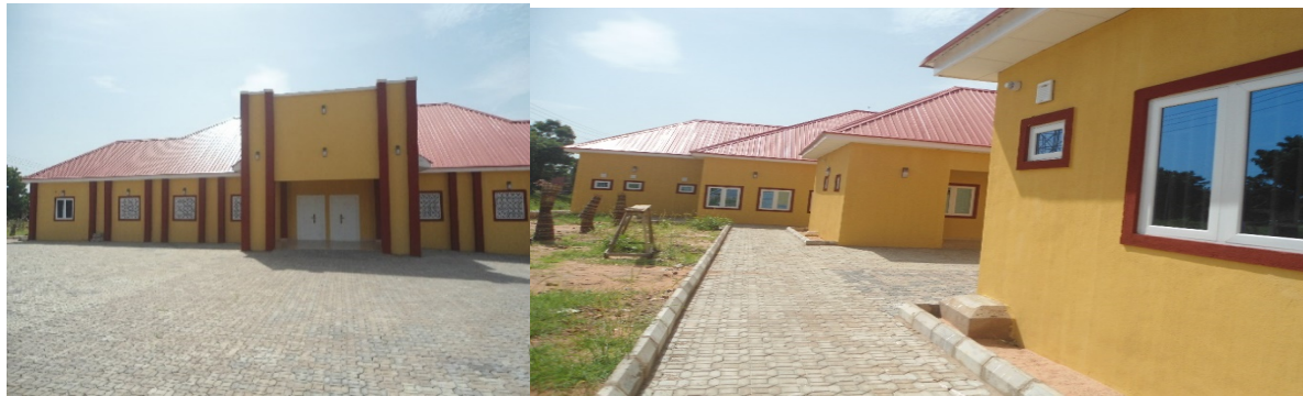
Picture 19: Completed student health centre at FCE (T) Gombe.
