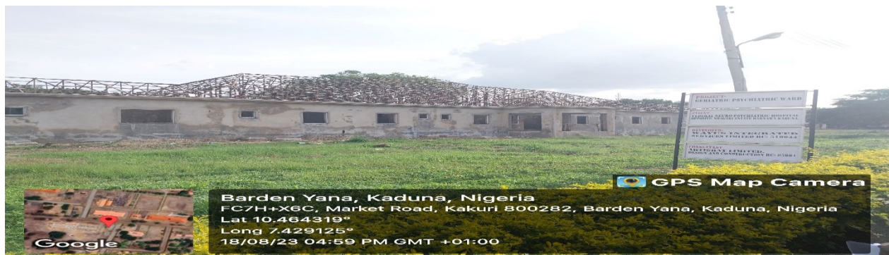
Picture 41: Ongoing Construction and furnishing of Geriatric Psychiatric ward at the Neuro-Psychiatric Hospital Kaduna.
