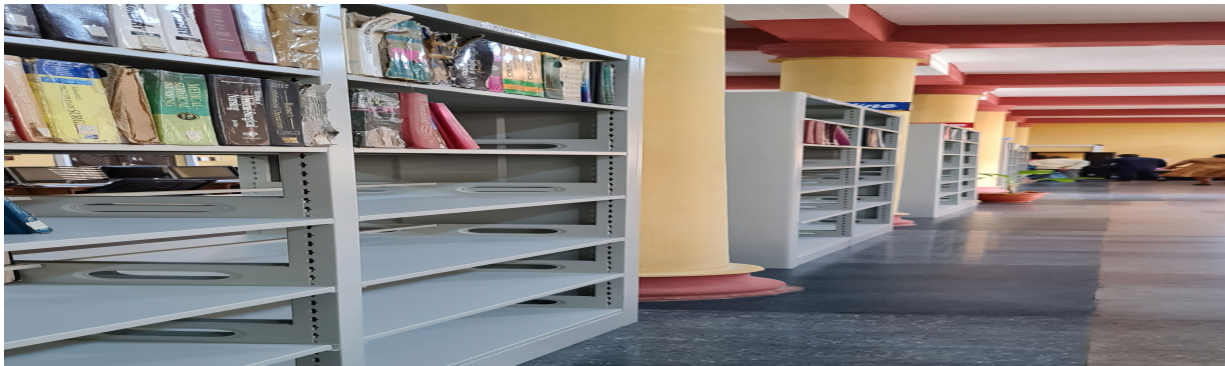
Picture 13: The completion section of E-library building at FUTO, Owerri
