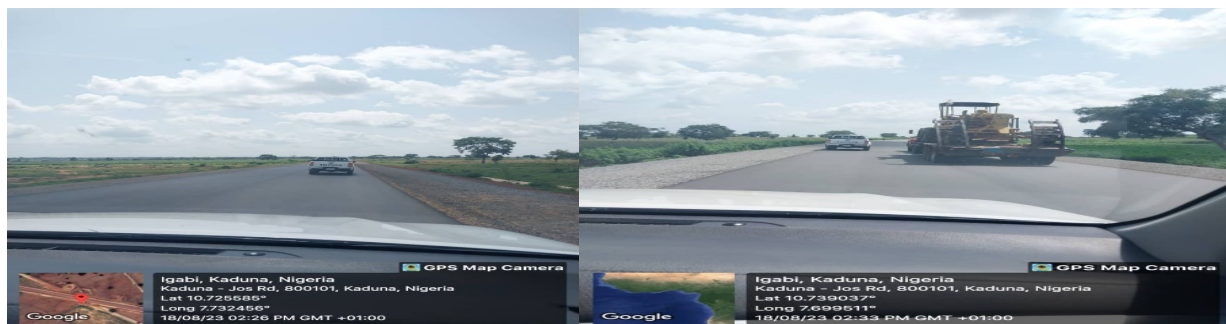
Picture 2: Ongoing Rehabilitation of Kaduna-Pambeguwa-Jos Road in Kaduna and Plateau States.
