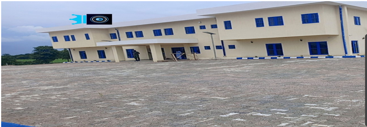
Picture 65: Constructed 2 blocks of 45 Rooms Student's hostel at Airforce Institute of Technology (AFIT), Kaduna.
