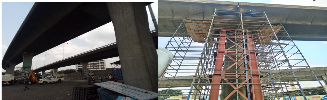
Picture 8: The strengthened and fixed finger bearing of Eko bridge
