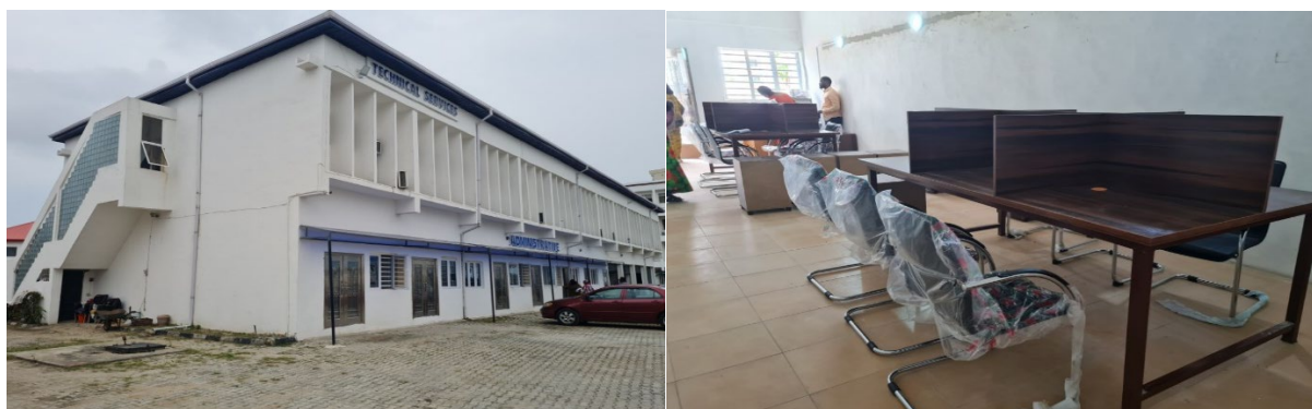
Picture 32: Completed Repairs and reroofing of dilapidated lecture building and provision of equipment at the institute of Oceanography.
