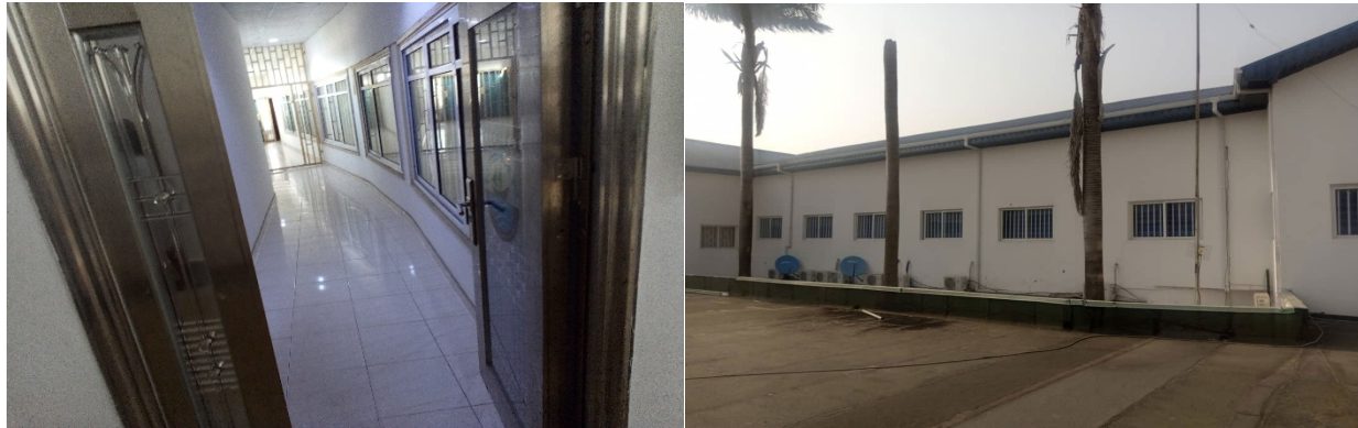
Picture 31: Renovated fish technology building office at Nigerian Institute of Oceanography and Marine Research, Lagos.
