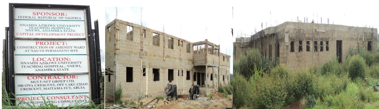
Picture 38: On-going construction of Amenity Wards (Male and Female) at Nnamdi Azikiwe University Teaching Hospital, Nnewi.
