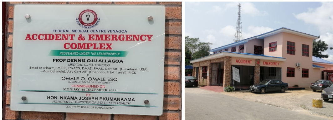
Picture 55: Completed Remodelling of Adult A&E Building at FMC, Yenegoa, Bayelsa State
