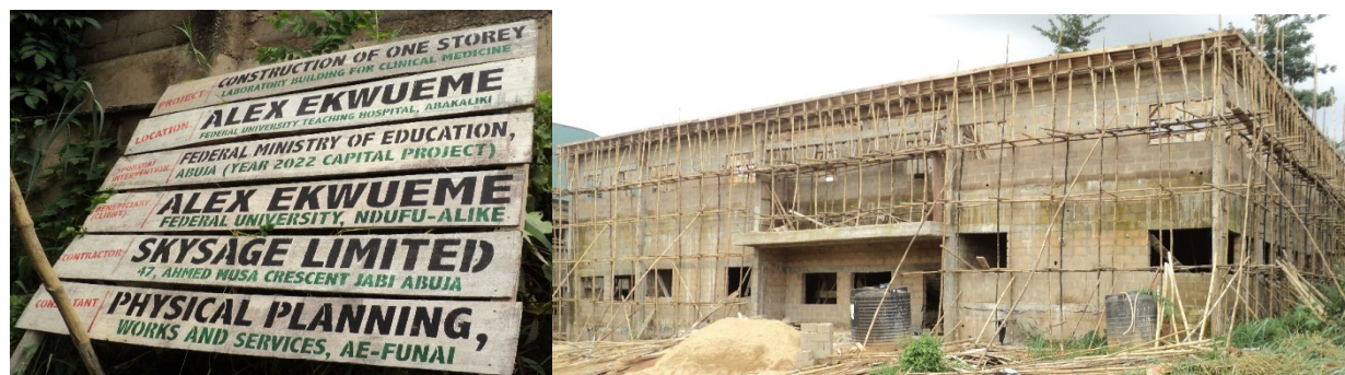
Picture 10: Ongoing Construction of Laboratories Block for Clinical Medicine at the Federal Teaching Hospital, Abakaliki.
