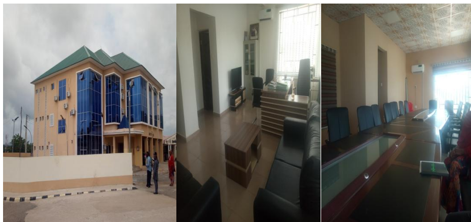
Pictures 44: Completion of Extension of Central Administrative Building & Furnishing at Federal Medical Centre Lokoja, Kogi State.
