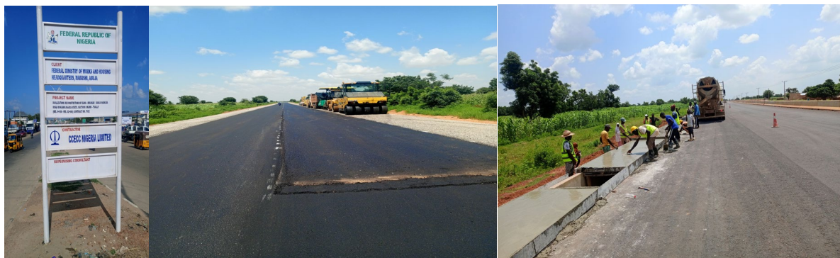
Picture 4: Ongoing dualization/reconstruction of kano-kwanar-danja-hadeija road
