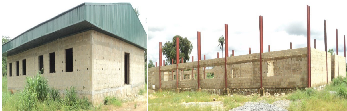
Picture 58: Ongoing Construction of Steel Fabrication and Welding Engineering Workshop at the MTI, Onitsha.
