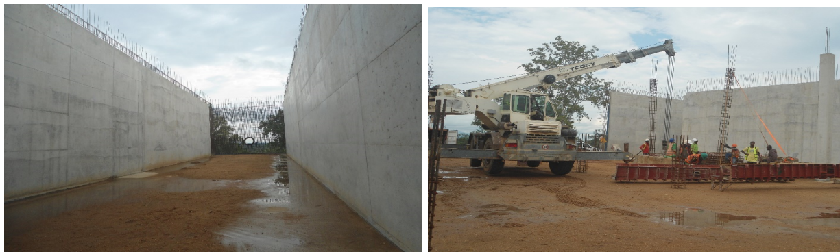
Picture 74: On going Intake reservoir construction work at Takum, Taraba State.
