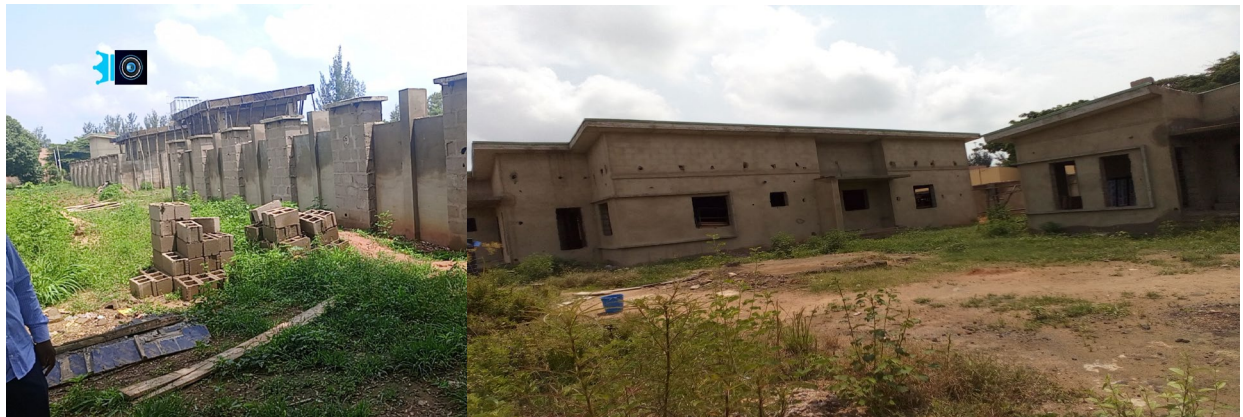
Picture 78: Ongoing Construction of Bursar house and other Directors houses at NITT, Zaria.
