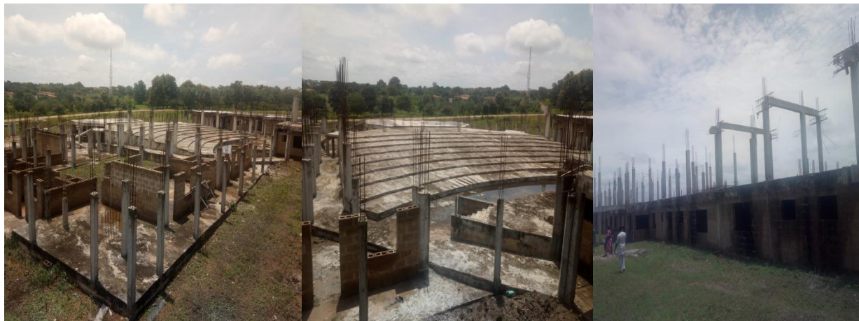
Pictures 29: On-going Construction of a 1000 Capacity Multi-Purpose Training Centre at ARMTI campus Ilorin, Kwara State
