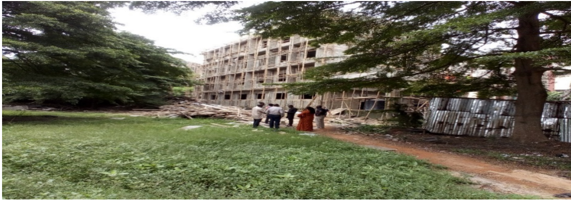
Picture 17: Ongoing Upgrade of Academic Building at the University of Lagos.
