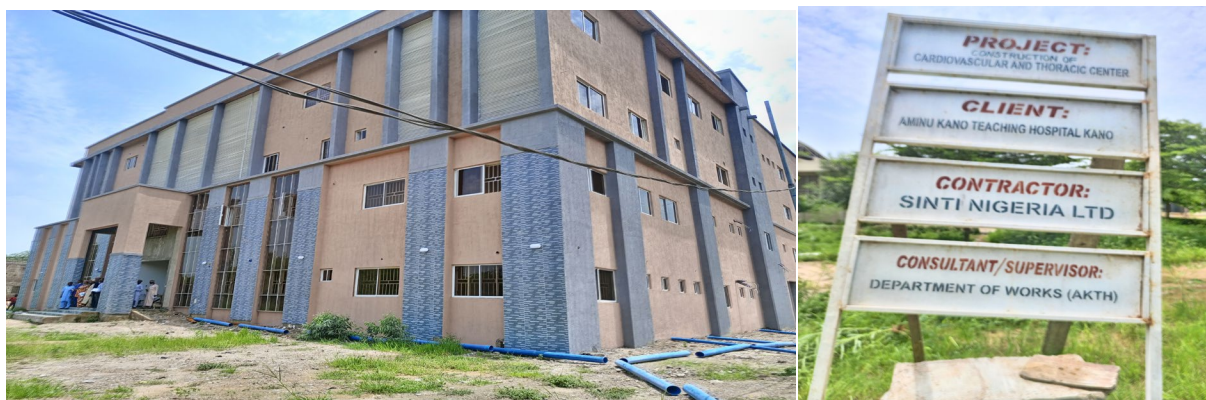
Picture 51: Constructed cardio vascular and thoracic Centre at AKTH, Kano.
