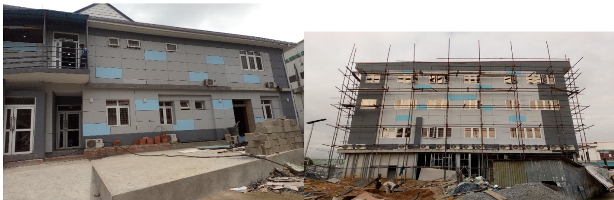
Picture 53: Completed phase A and ongoing phase B of the hospital complex
