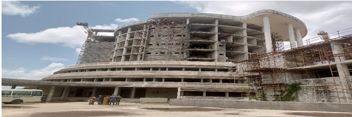
Picture 63: Ongoing Construction of Administrative Block at Permanent site Piwoyi, Phase I.
