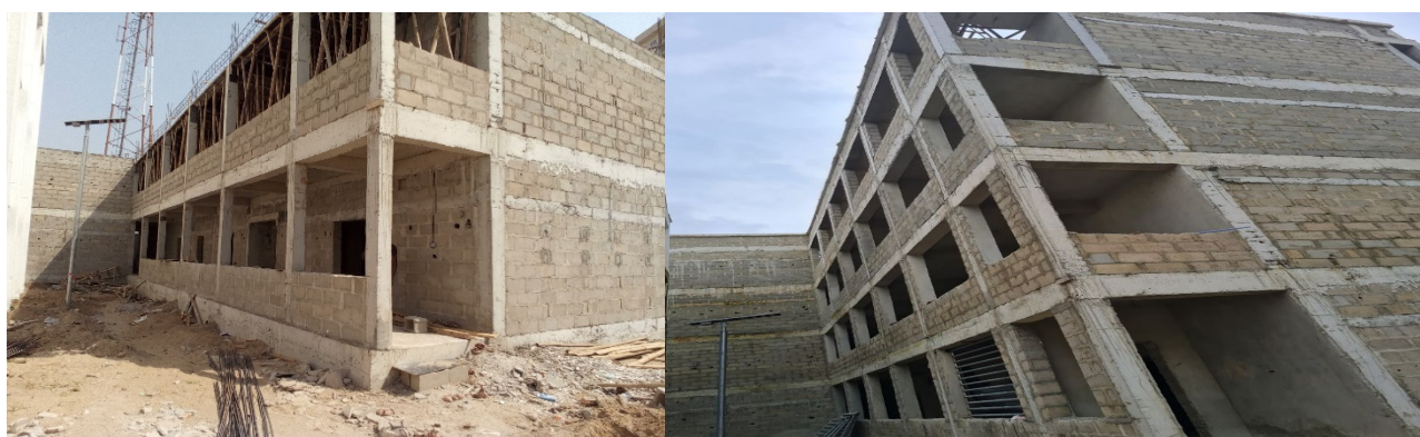
Picture 33: Ongoing construction of 56 rooms capacity hostel at Federal College of Fisheries and Marine Technology, Lagos.
