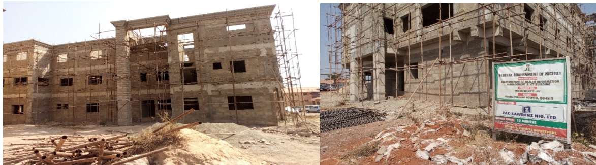
Picture 52: Ongoing construction of ICT and health information management Centre
