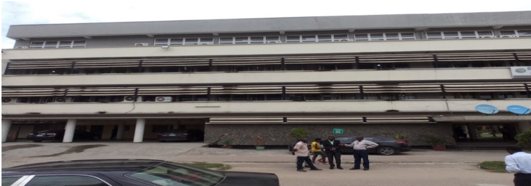
Picture 16: Completed Administrative building for College of Medicine University of Lagos, Idi-Araba.
