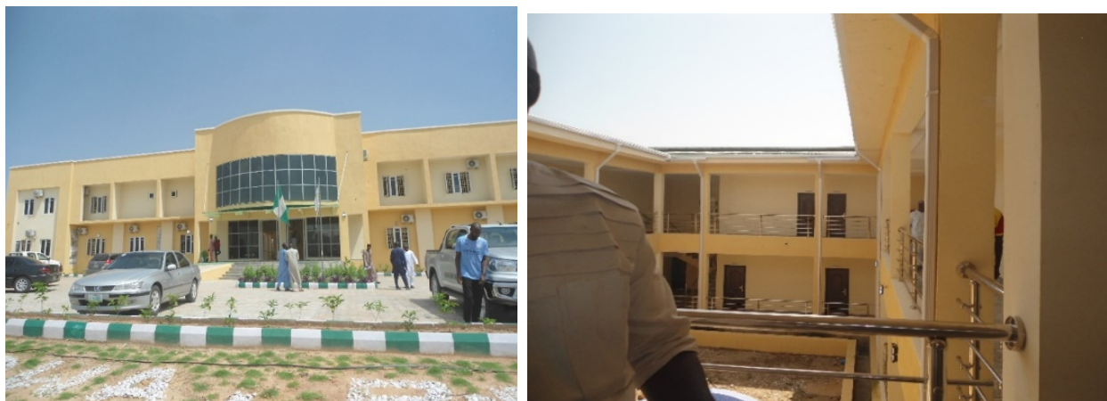
Picture 27: Completed Provost Office Complex at Federal College of Horticulture Dadinkowa, Gombe.
