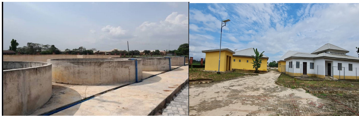
Pictures 14: The completed fish ponds, processing centre & staff quarters at Polytechnic, Nekede.
