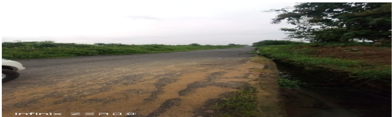
Picture 79: Ongoing Construction of Internal Road (16B) at Maritime Academy, Oron.
