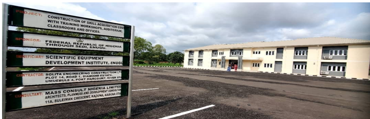
Picture 71: The Completed Construction and Equipped Skill Acquisition Centre at SEDI, Enugu.
