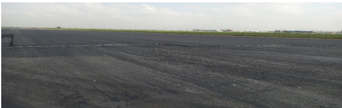
Picture 25: Extension and Asphalt Overlay of MMIA Runway 18L/36R at Lagos Airport
