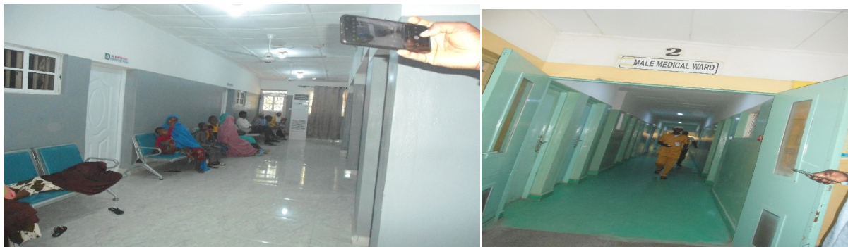
Picture 42: Completed expansion of clinics/wards works at Federal Teaching Hospital Gombe.
