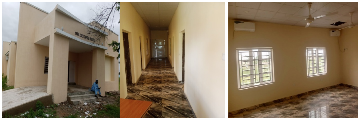
Picture 23: The Completed Construction of Works and Services Department.
