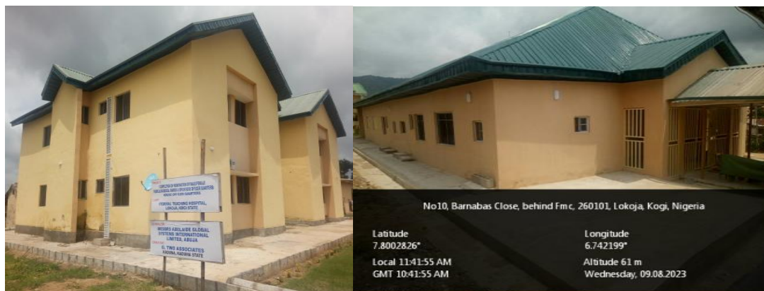
Pictures 45: Complete Renovation of Male/Female Medical/Surgical Wards Epu/House Officer Quarters at Federal Medical Centre Lokoja, Kogi State.
