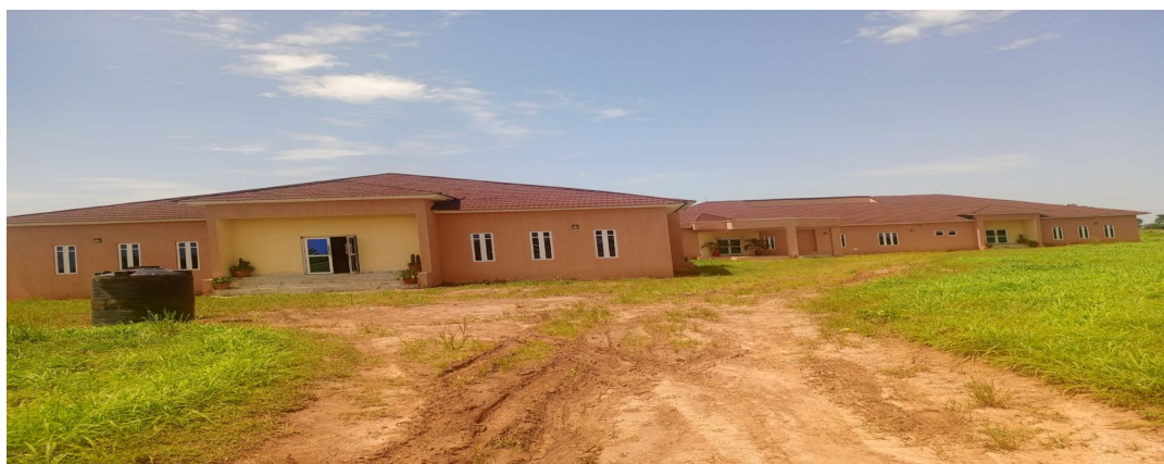
Picture 66: completed officers' mess at NDA Afaka, Kaduna.
