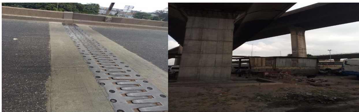
Picture 7: Repaired portion of the Marine bridge in Lagos State.
