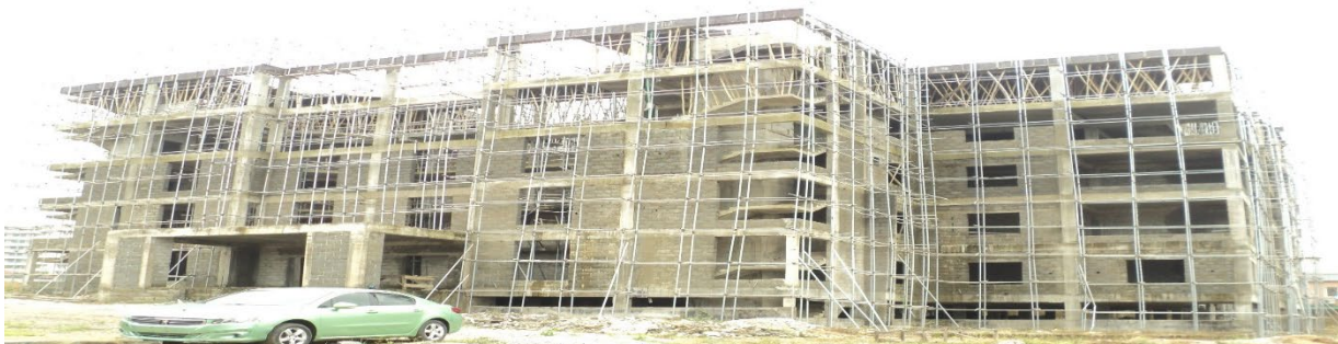
Picture 61: Ongoing construction and provision of a 5-storey office building at DRDB Headquarters, Abuja.
