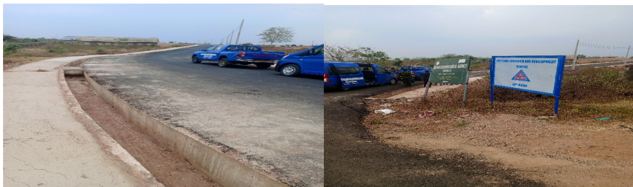
Picture 69: completed 2km flexible road pavement at air force research and development Centre, Oshogbo
