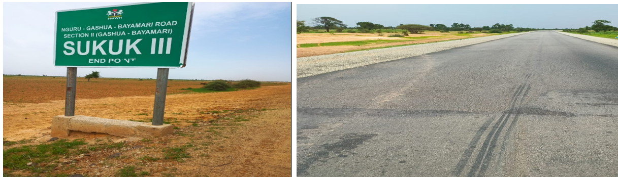
Picture 5: Completed portion and on-going works at Nguru-Gashua-Bayamari Section II Phase II:(Gashua-Bayamari) Road in Yobe State Contract No. 6479.
