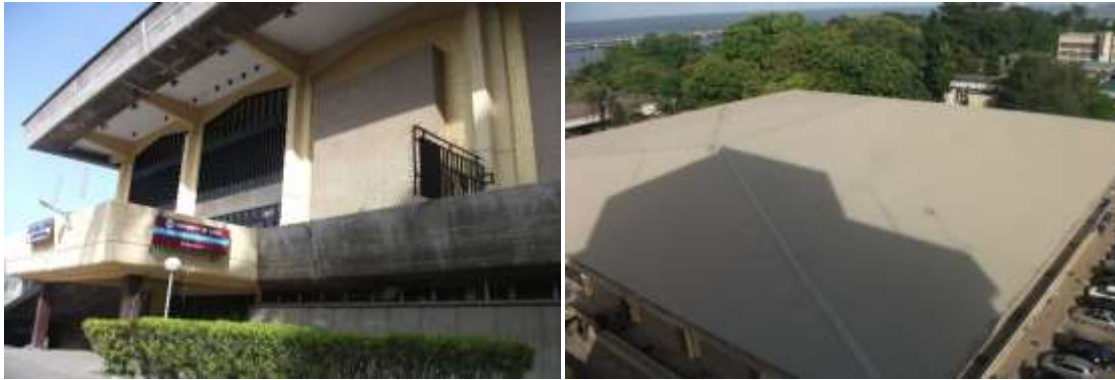
Picture 44: Rehabilitated Auditorium building at University of Lagos
