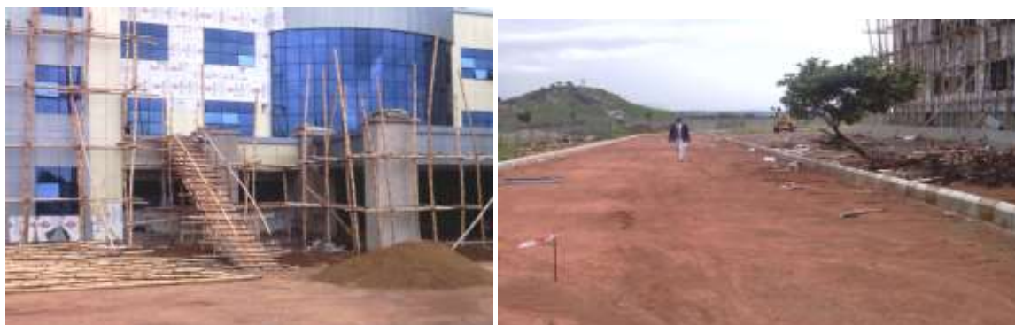
Picture 36: On-going construction works of Defence Space Agency Complex
