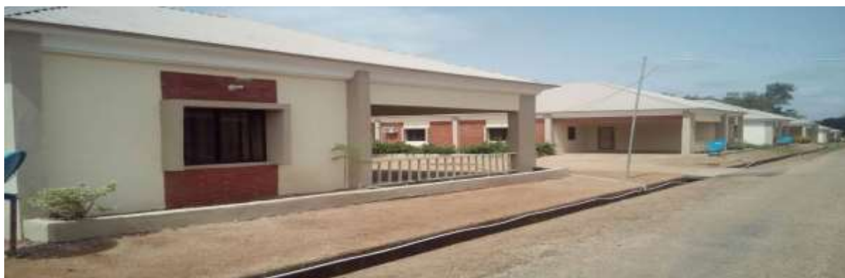
Picture 53: Completed Renovation Works of a Section of the 12Nos Participants Chalets in NIPSS, Jos.
