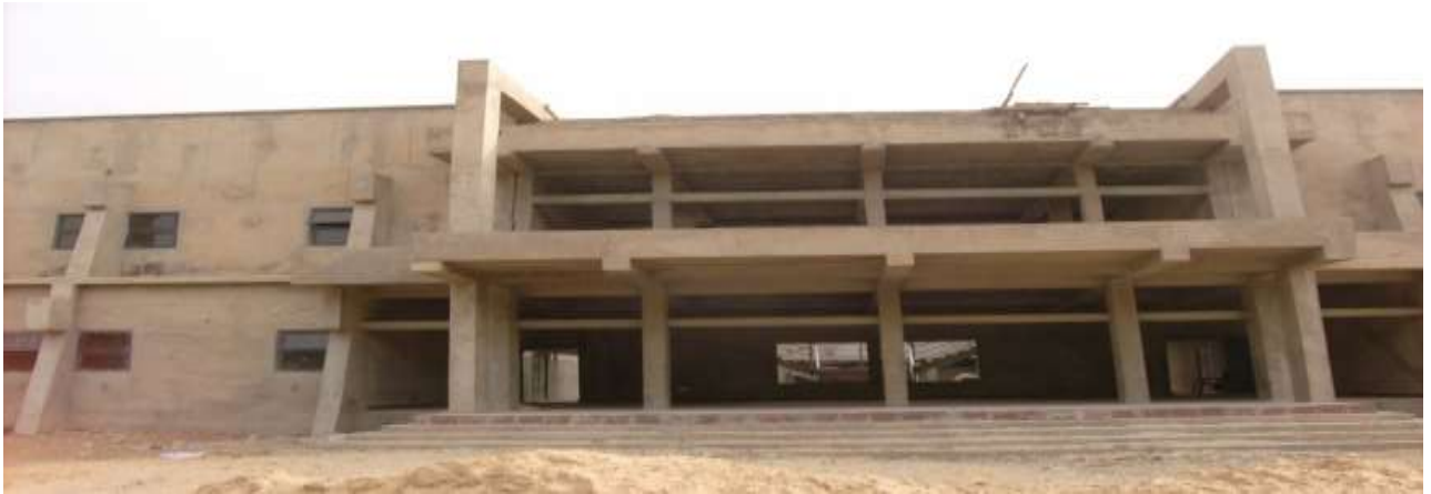
Picture 45: On-going construction of Faculty of Civil Engineering complex at Usman Danfodio University, Sokoto
