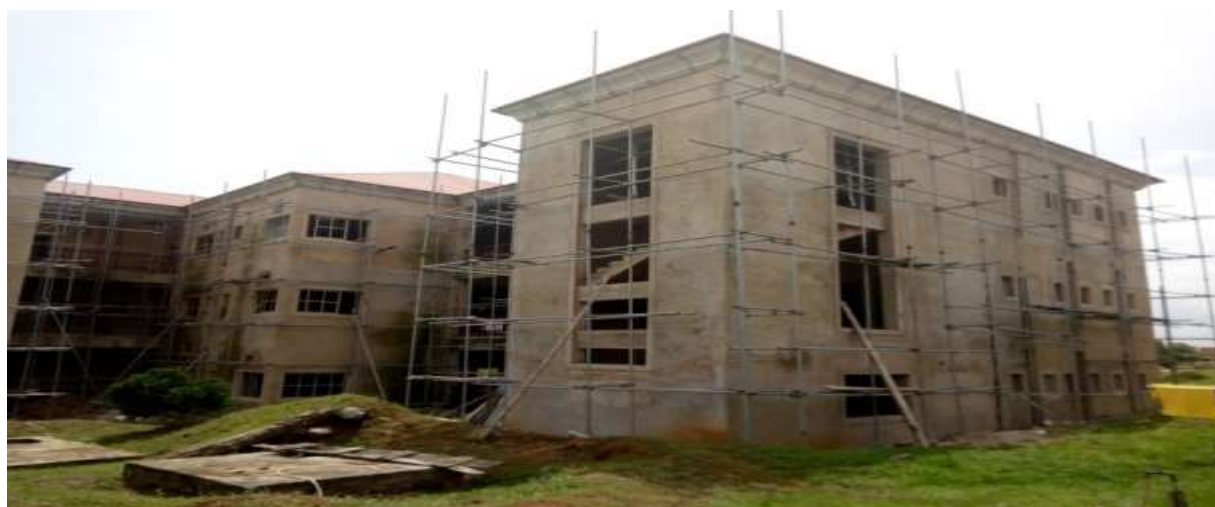
Picture 26: On-going Upgrading of ward 10 to 2 storey building at FMC Owerri
