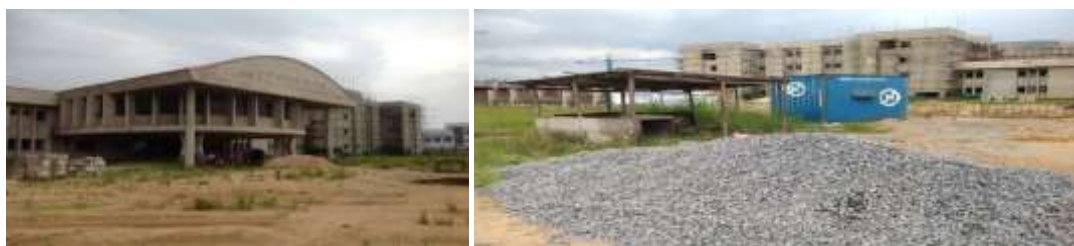
Picture 17: Ongoing Construction of Federal Secretariat Complex, Yenagoa, Bayelsa State
