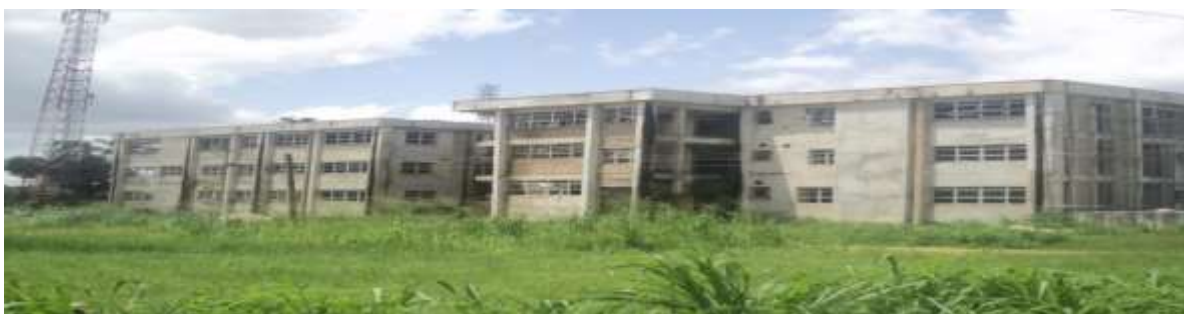
Picture 25 : Ongoing Construction of 2-storey General Outpatient Block, Phase II
