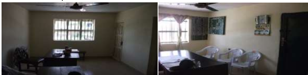
Picture 5: Completed renovation of administrative offices at Ilaro Prison
