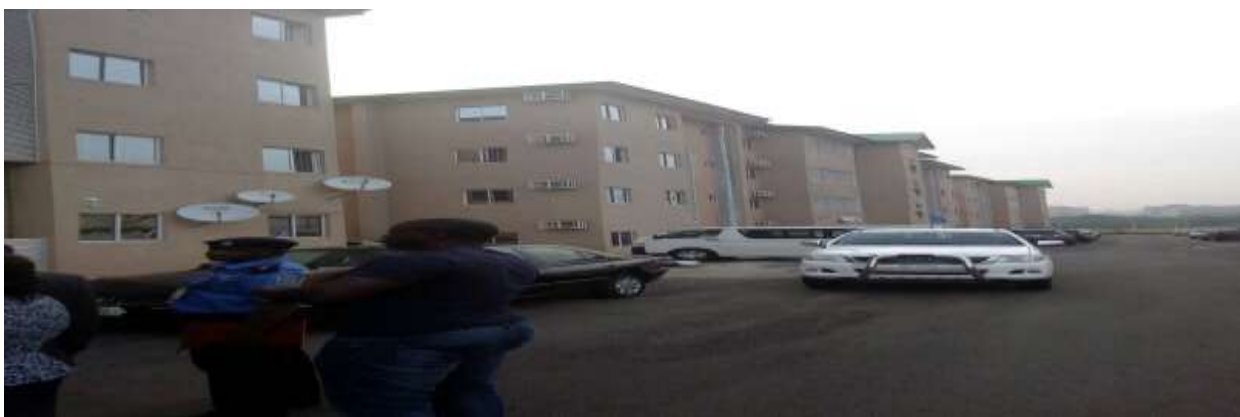
Picture 7: Completed 4nos Blocks of 8 flats at FHQ, Abuja
