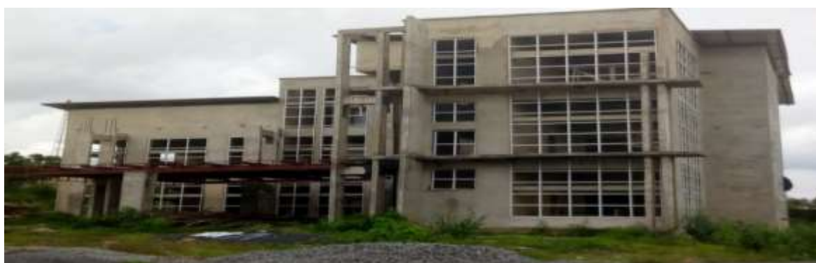
Picture 50: Ongoing construction of South East Zonal office for NEMA, Enugu
