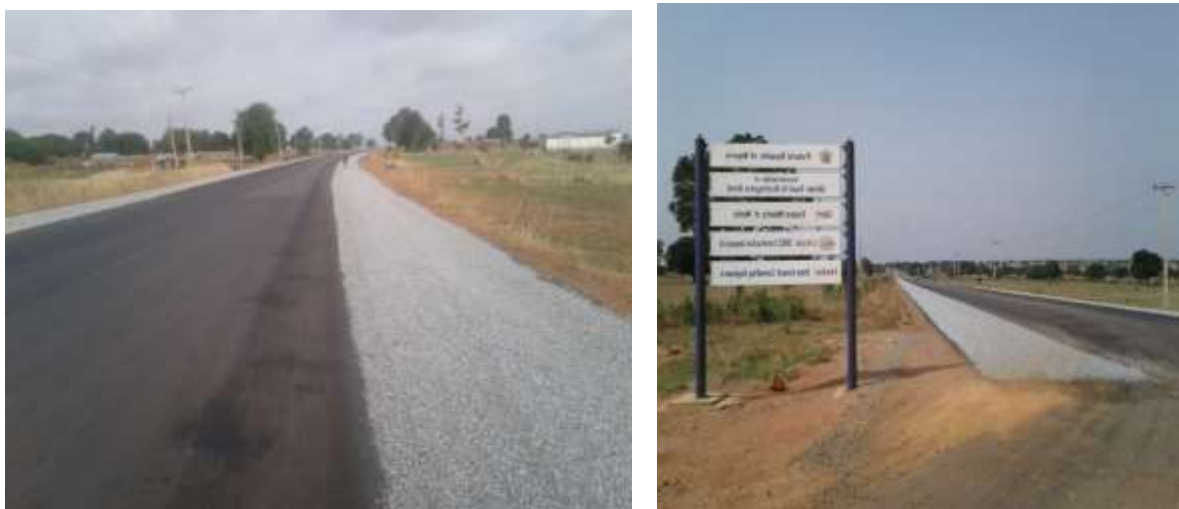
Picture 15: Completed portion and on-going works at Reconstruction of Sokoto-Tambuwal-Jiga-Kontagora-Makera Road, Section 11, Niger State.
