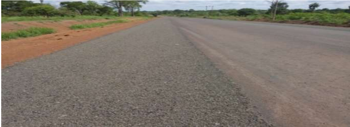
Picture 14: On-going construction of Oshegbudu-Oweto Road in Benue State
