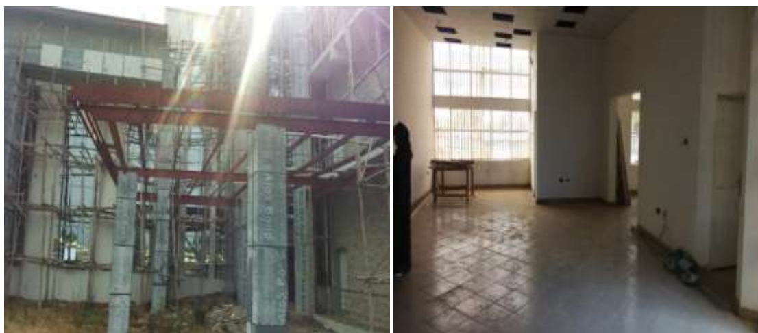
Picture 51: On-going Construction of NEMA North West Zonal Office, Kaduna
