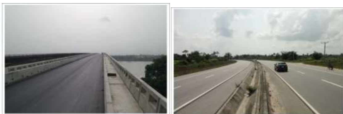
Picture 46: Completed dualisation of East-West Road, Section I
