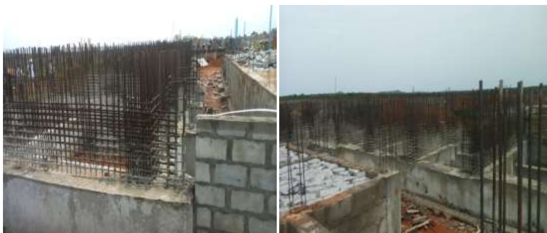
Picture 38: On-going DICON project of construction of Primer Cap Production Line at Kachia, Kaduna State
