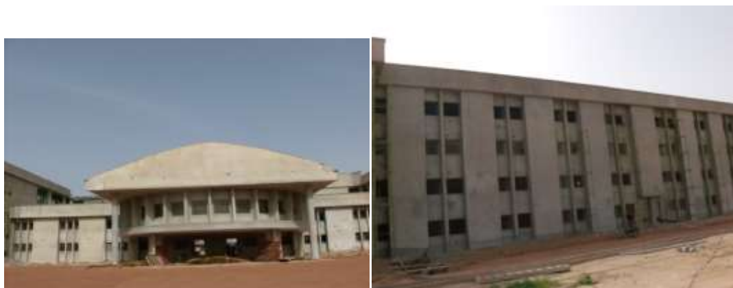
Picture 18: Ongoing Construction of Federal Secretariat in Zamfara State
