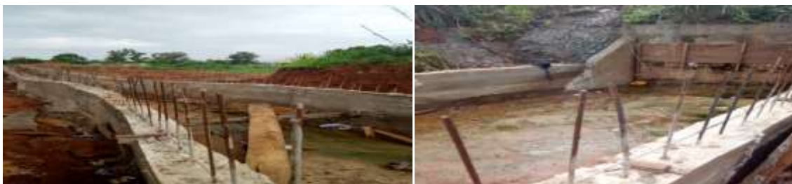
Picture 49: On-going Flood and Erosion Control at Metallurgical Training Institute, Onitsha.
