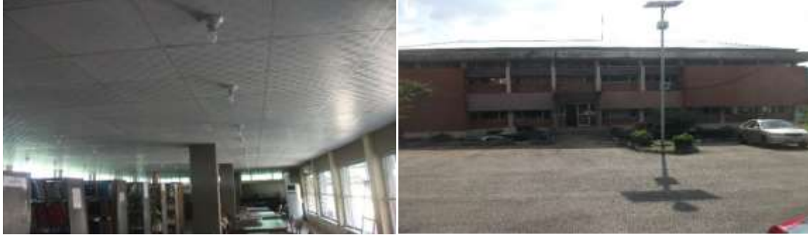
Picture 56: Completed re-roofing of NISER library
