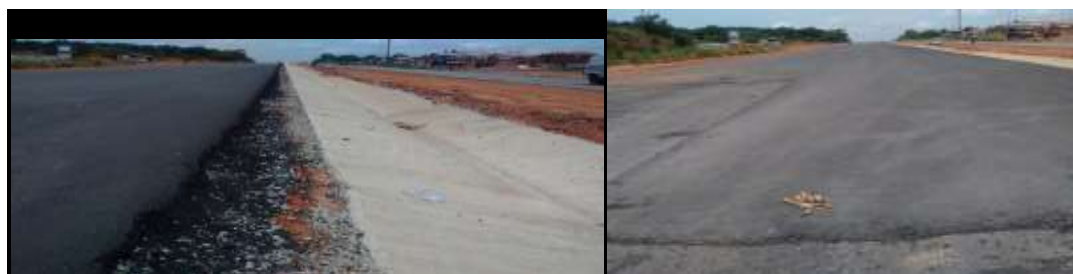
Picture 10: Ongoing rehabilitation of outstanding portion of Onitsha – Enugu Expressway Amansea – Enugu Road
