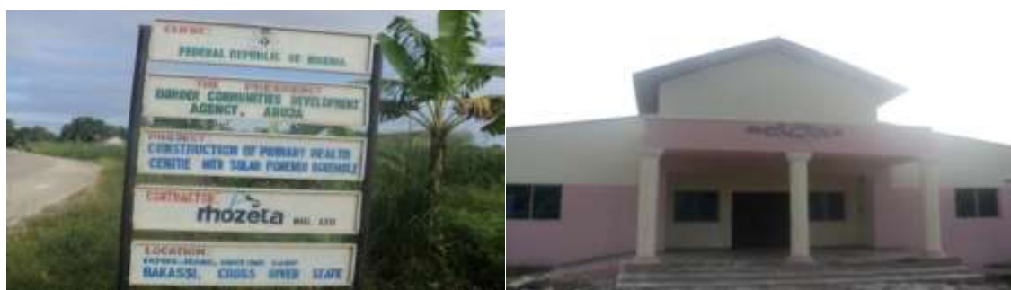
Picture 33: Completed Medical Health Care at Ekpiri-Ikang, Obutong camp- Bakassi, Cross River State
