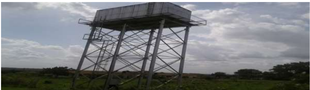
Picture 24: Completed borehole at ARMTI Ilorin
