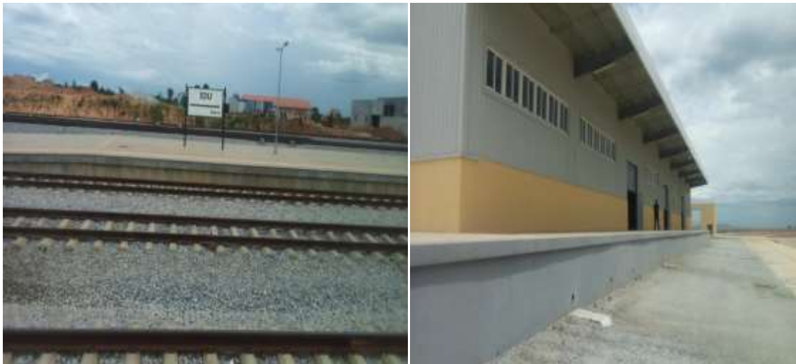
Picture 29: Completed rail track and on-going construction of Idu cargo freight yard and warehouse at Idu, rail station.
