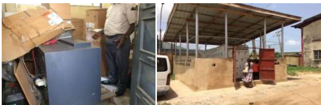
Picture 21: Storage for uninstalled Equipment and 350KVA Sound-proof Power Generating Set
