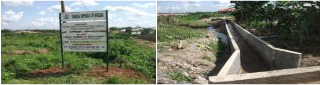
Picture 40: Completed drains and box culverts at Irepodun, Olorunda, Osogbo, Orolu, Osun State
