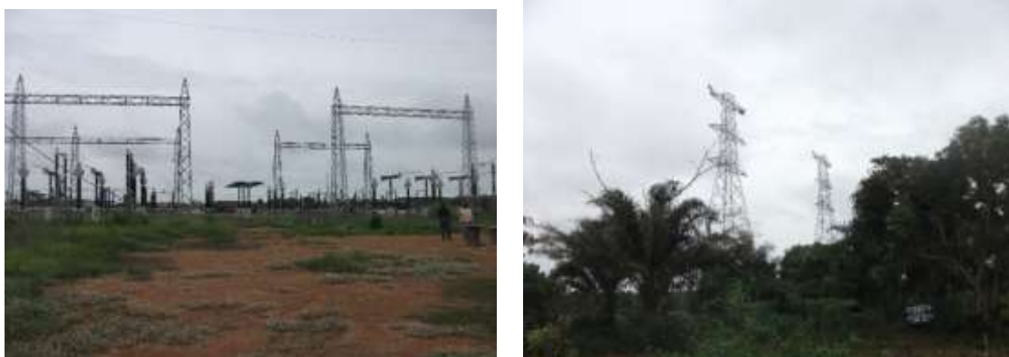
Picture 8: Benin North-Oshogbo 330KV DC Line with one SC turning in and out to new Akure Sub-Station.
