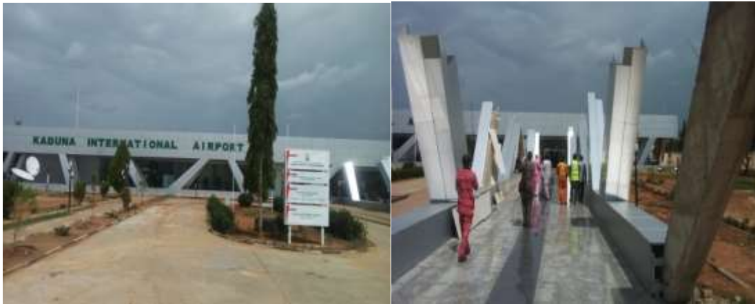
Picture 31: Completed Arrival & Departure sections and on-going construction of Slippers at Kaduna International Airport, Kaduna
