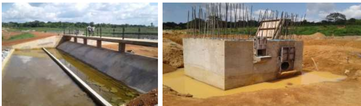
Picture 3: The Ongoing Construction of Orin irrigation project
