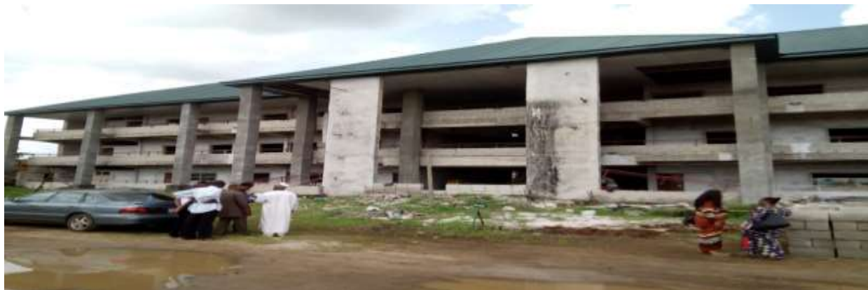
Picture 43: On-going Construction of 2 Storey (Senate) Building at FCE, Owerri.
