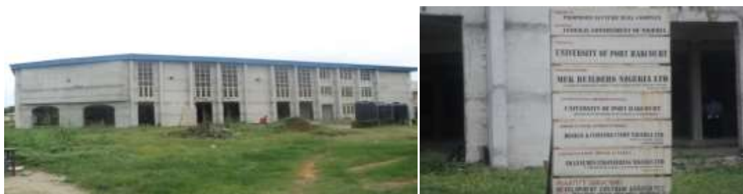
Picture 42 : Ongoing Construction of Pharmacy Lecture Complex at UniPort.
