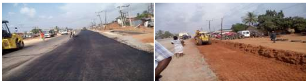
Picture 12: On-going dualization of Obajana Junction to Benin Section IV, Ehor –Benin Road.
