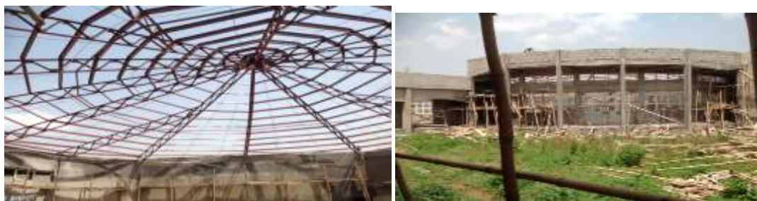
Picture 22: On-going completion of Space Technology Incubation Centre
