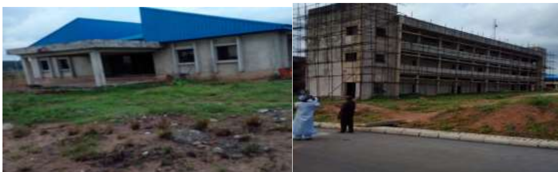
Picture 35: Ongoing Construction of medical centre & hostel at FRSC Academy, Enugu State
