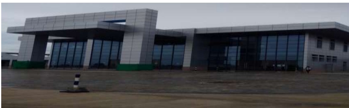
Picture 54: Completed Idu Station at Abuja Rail Mass Transit
