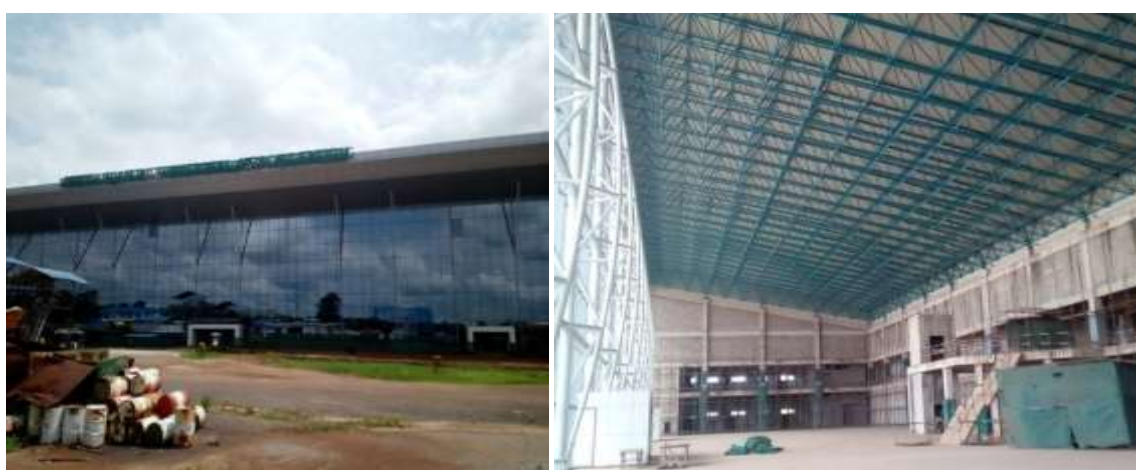
Picture 30: On-going construction of new terminal building at Akanu-Ibiam International Airport, Enugu
