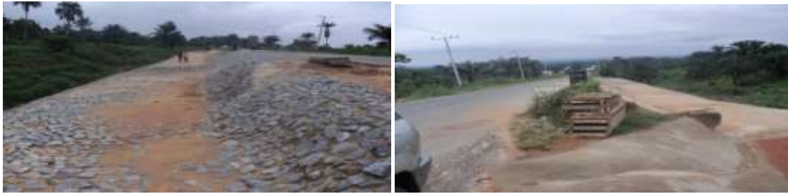
Picture 39: Completed Erosion Control works at Mbia Bong and IkpeEketNkom, Akwa- Ibom State
