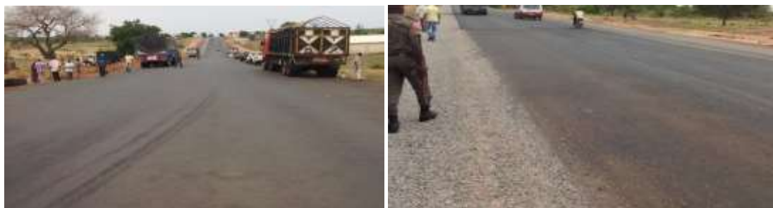
Picture 13: On-going Construction work of Gombe – Numan – Yola road Section II,
