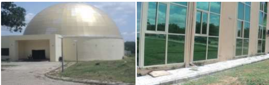
Picture 19: The electronic dome and completed portion of landscaping works at NASRDA, Abuja.
