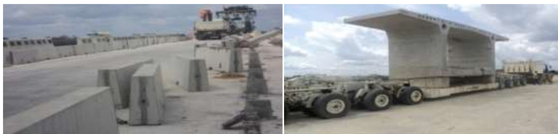
Picture 47: Concrete works/a bridge segment being conveyed at Kaiama Bridge
