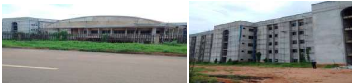
Picture 16: On-going Construction of Federal Secretariat Complex, Awka, Anambra State.
