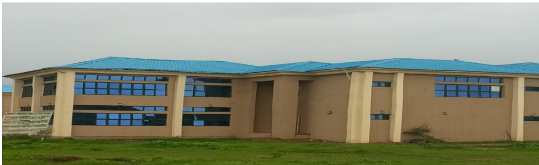
Picture 31: Completed 4No. 100 Seat Capacity Lecture Rooms at Federal University, Birnin-Kebbi
