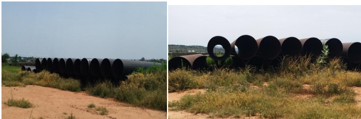
Picture 34: Part of the Steel Pipes on ground at the Chouchi Irrigation Project
