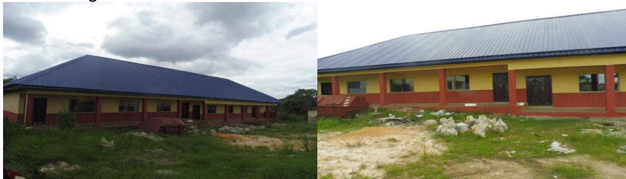
Completed 27: Completed Students' Lecture Halls at UNICAL Teaching Hospital, Calabar
