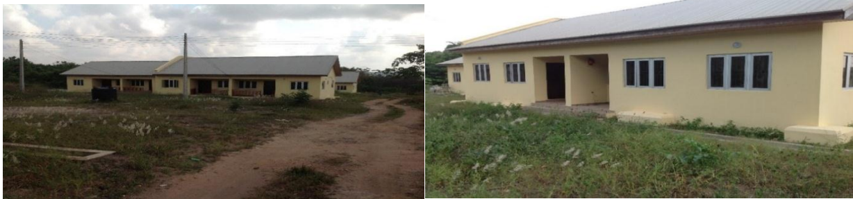
Picture 24: Completed Block of Flats at Neuropsychiatric Hospital, Aro, Abeokuta
