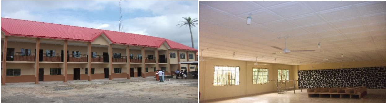
Picture 30: Completed Administrative Block at Adeyemi College, Ondo State
