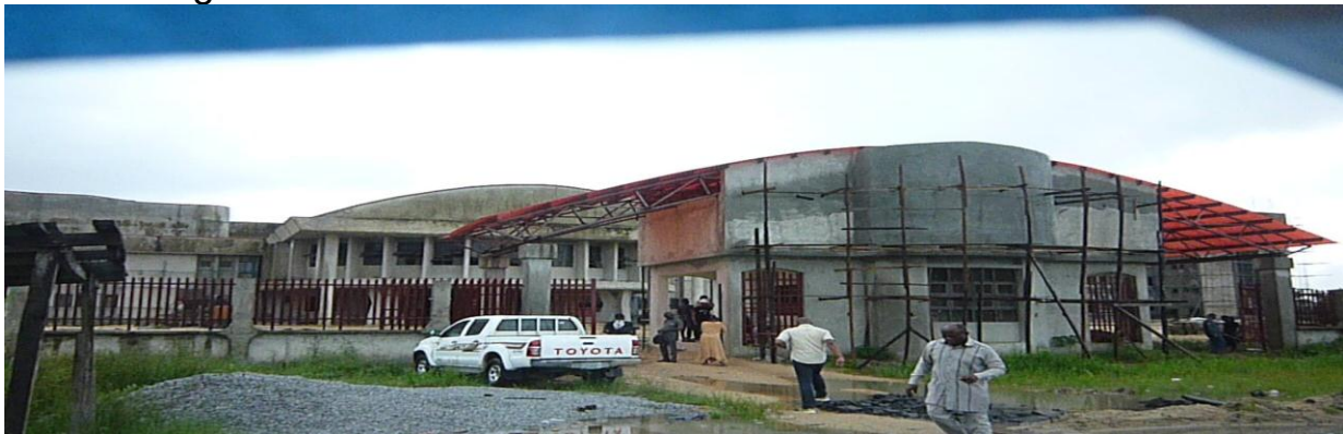
Picture 16: On-going Construction of Federal Secretariat Complex, Yenagoa, Bayelsa State
