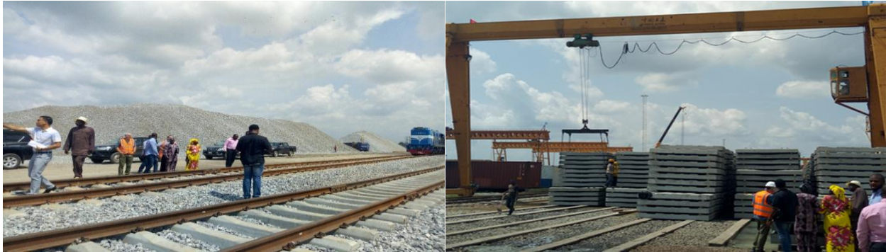
Picture 3: On-going Construction of Rail Line/Tracks Slippers at Lagos – Kano Railway Project
