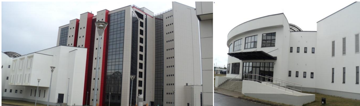
Picture 21: Completed Admin Block and Female Detention Block at the EFCC New Head Office, Abuja
