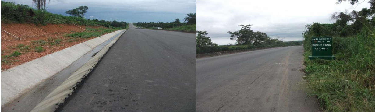
Picture 9: Completed Portion of Benin-Ofosu-Ore-Ajebandele-Shagamu Expressway, Phase III
