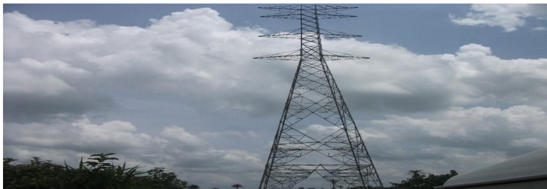
Picture 12: Completed Tower Erection at Omotosho-Erukan (Ogijo) Transmission line
