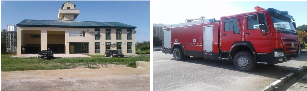
Picture 5: The Constructed Workshop and Fire Fighting Equipment
