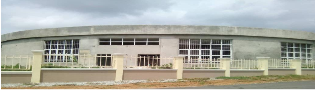
Picture 36: On-going Construction of Space Technology Incubation Centre at Centre for Satellite Technology Development (CSTD) Abuja
