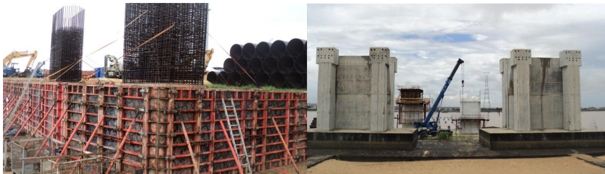
Picture 8: Ongoing Construction of 2 nd Niger Bridge at Onitsha
