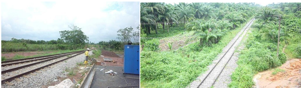
Picture 2: Completed Portion of Rail Tracks at Ajaokuta-Itakpe-Warri Rail Lline
