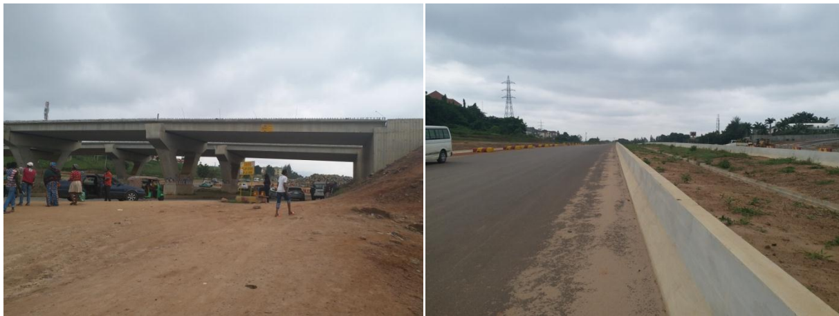
Picture 38: The Interchange Structure at the Apo Roundabout/Crash Barrier at the Deeper Life Axis
