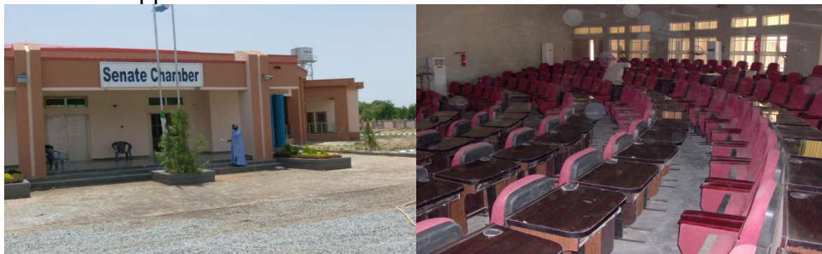
Picture 32: The Construction and Furnishing of the Senate Chamber, University of Maiduguri.
