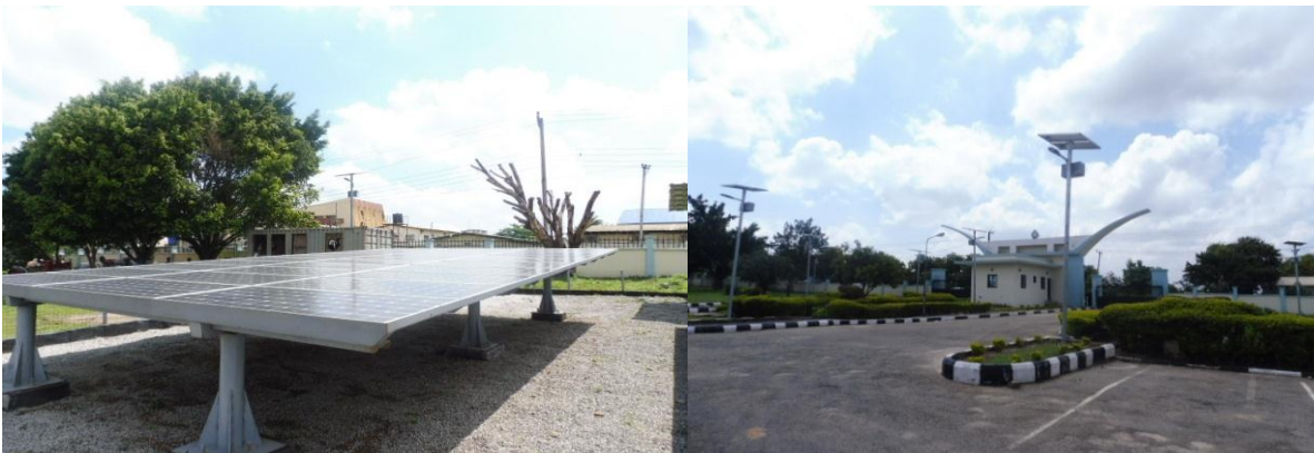
Picture 35: Renovation work at NASENI Headquarters, Abuja
