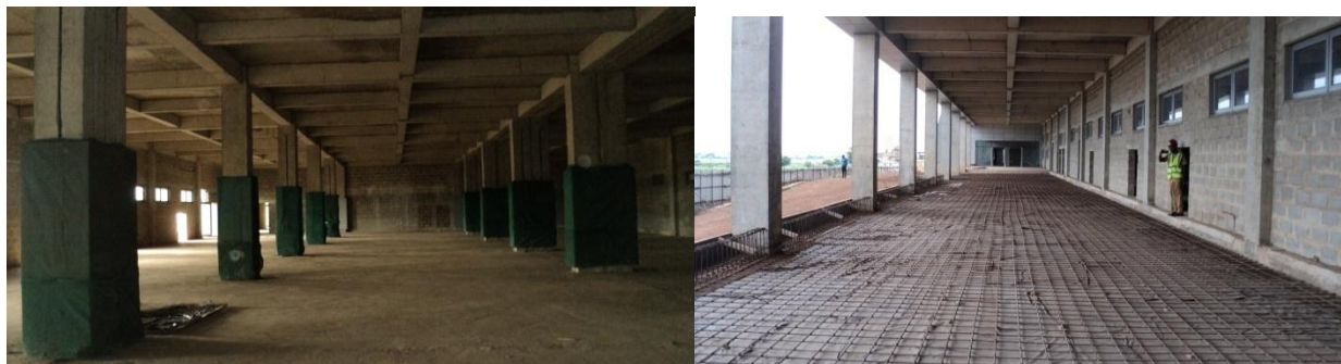
Picture 7: On-going Arrival Hall and Re-enforcement Works of External Passage at Akanu Ibiam International Airport, Enugu
