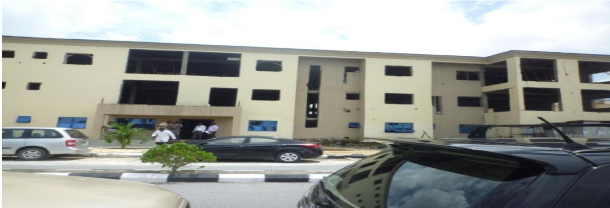
Picture 25: Construction of Surgical Ward Block almost completed at FMC Yenegoa
