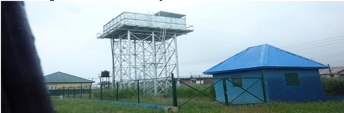
Picture 33: Completed Water Scheme and control room at Isiokolo Irrigation Projects, Delta State
