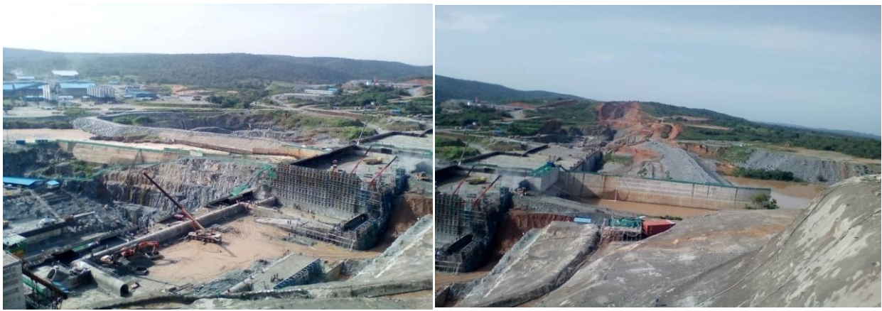
Picture 13: Excavation/Foundation Grounding Works at Zungeru Hydroelectric Power Project
