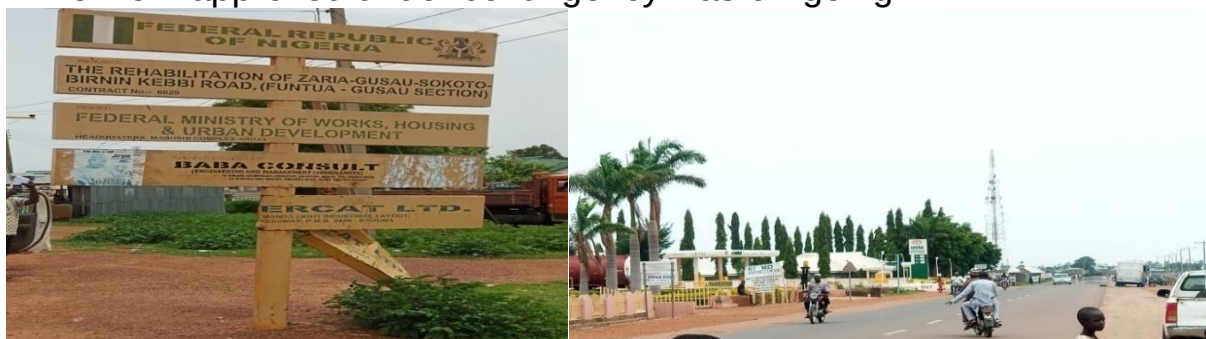
Picture 11: On-going work on Rehabilitation of Zaria-Gusua-Sokoto – Birnin Kebbi Road
