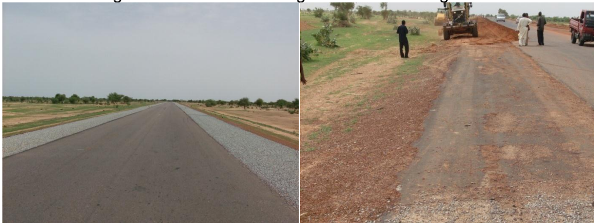
Picture 10: Rehabilitation of Hadejia-Nguru-Gashua-Bayamari Road Project with Ongoing Works on the Road Shoulder
