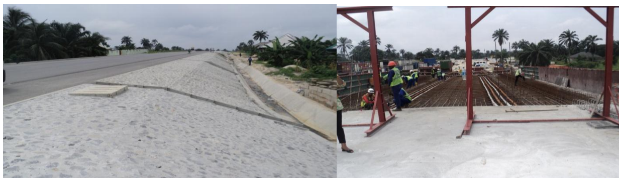
Picture 3: Ongoing Construction of Bodo–Bonny Road with Bridge accross Opobo Channel, Route 430 in Rivers – State
