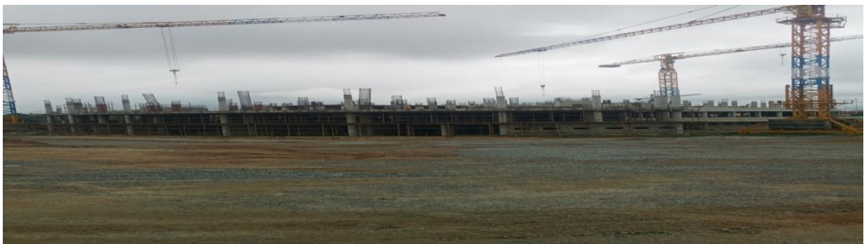
Picture 35: On-going Construction of Administrative Block at National Defence College Piwoyi-Abuja
