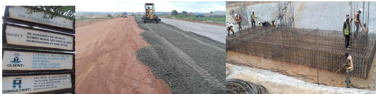
Picture 2: Ongoing Stone Base at KM46, Piles/Abutment and Reinforcement for Pile Caps and Piers in progress at Bridge 17
