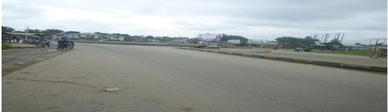
Picture 57: Completed Portion of Dualization of East –West Road , (Section IV) Eket-Oron in Akwa-Ibom State
