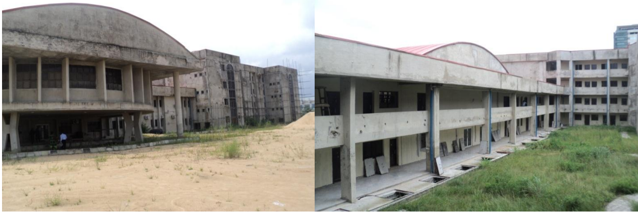
Picture 11: On-going construction of Federal Secretariat Complex, Yenegoa
