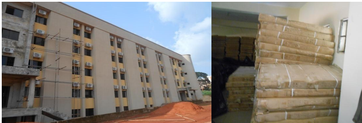
Picture 9: On-going Construction of Secretariat Complex at Awka in Anambra State
