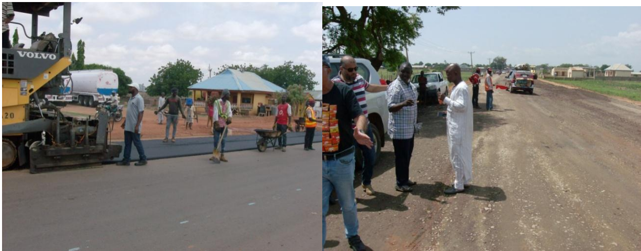
Picture 4: Laying of Asphalt and Scarification Works at Yauri Town of the Road Project
