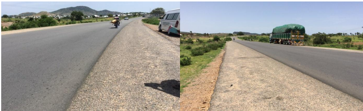
Picture 5: Ongoing completion of Gombe-Numan-Yola Road Phase II (Gombe-Kaltungo)
