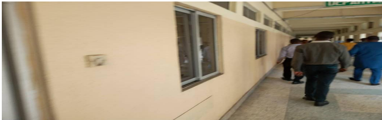
Picture 27: Ongoing Renovation of Block A (Lot 2) at UPTH
