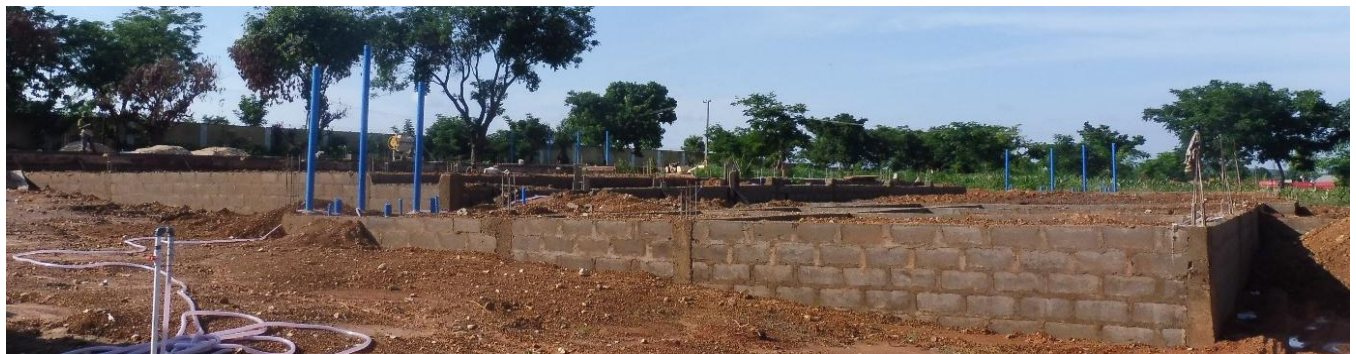
Picture 32: Ongoing Construction of a New Conference and Library Hall at National Cereal Research Institute, Badeggi, Niger State
