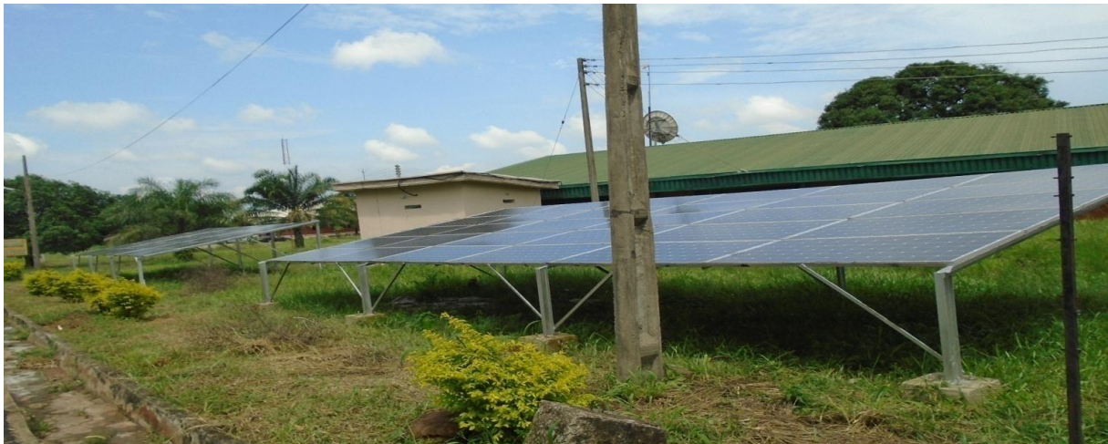
Picture 51: Installation of Solar Energy Panel at Metallurgical Training Institute, Onitsha
