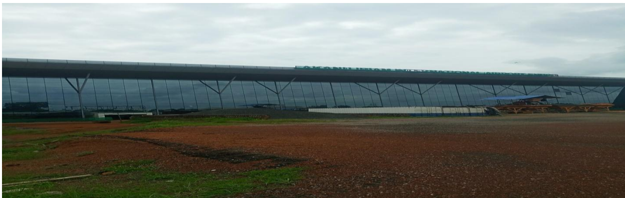
Picture 14: On-going Construction of the New Akanulbiam International Airport, Enugu Terminal Building
