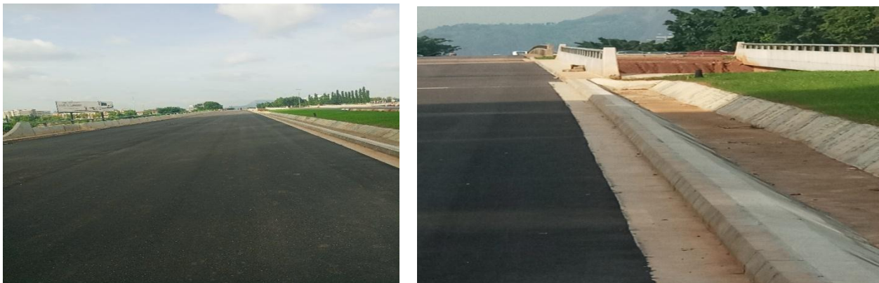
Picture 58: Ongoing Completion of Road B6, B12, and Circle Road at Independence Avenue, Abuja
