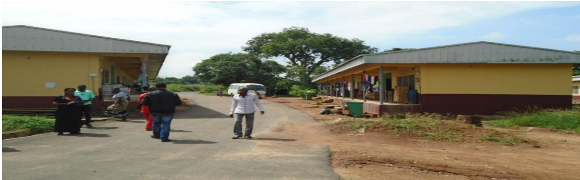
Picture 50: Some of the Renovated Hostel Blocks at the MTI, Onitsha
