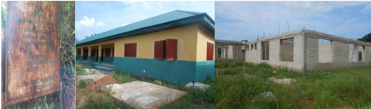
Picture 6: Ongoing construction of Classrooms and Administrative Building at the Model Building Craft Training School, Ikeduru – Imo state
