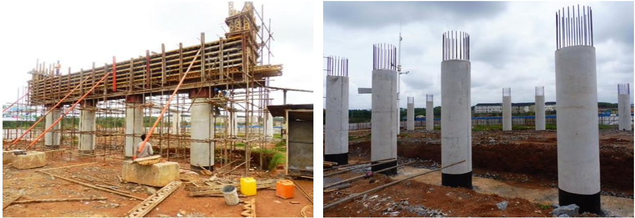
Picture 59: On-going Construction of Bridge Superstructure at the Galadimawa Interchange of the Extension of Inner southern Expressway Abuja
