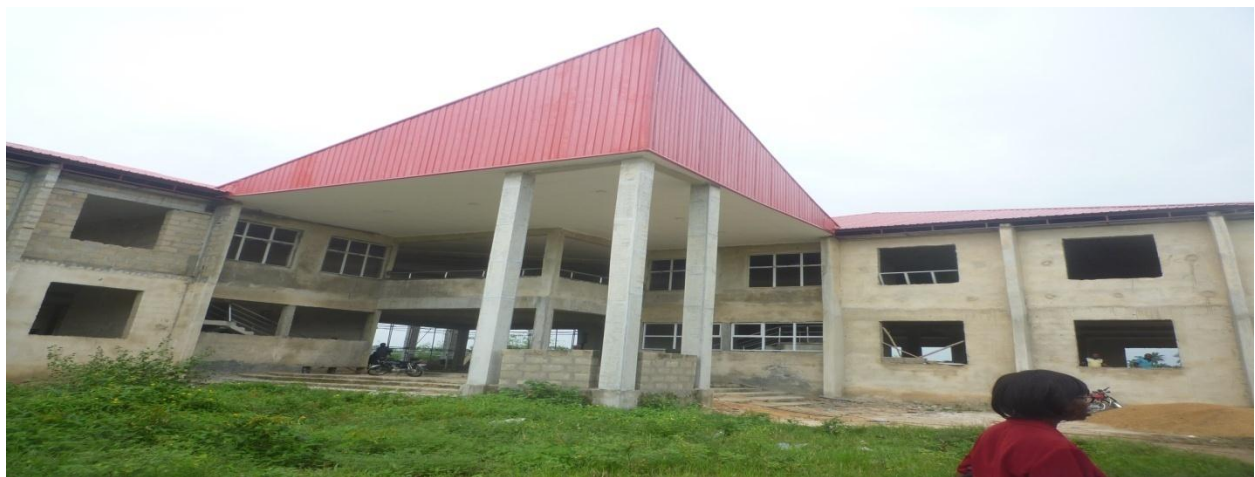
Picture 45: Ongoing Construction of Library Complex Federal Polytechnic Ukana
