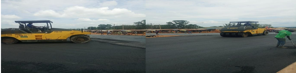
Picture 1: On-going Rehabilitation and Reconstruction of Enugu to Port-Harcourt Dual Carriageway Section I
