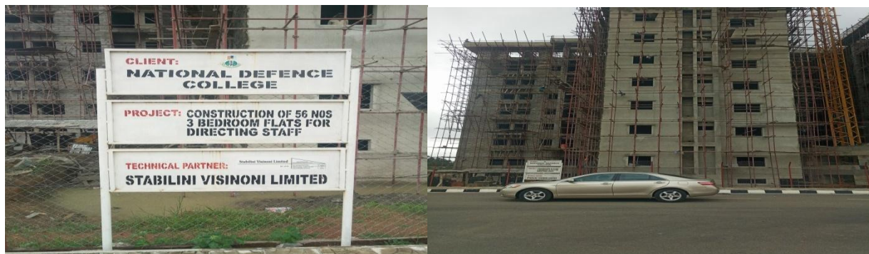
Picture 34: On-going Construction of DS Quarters at Piwoyi (NDC Permanent Site)
