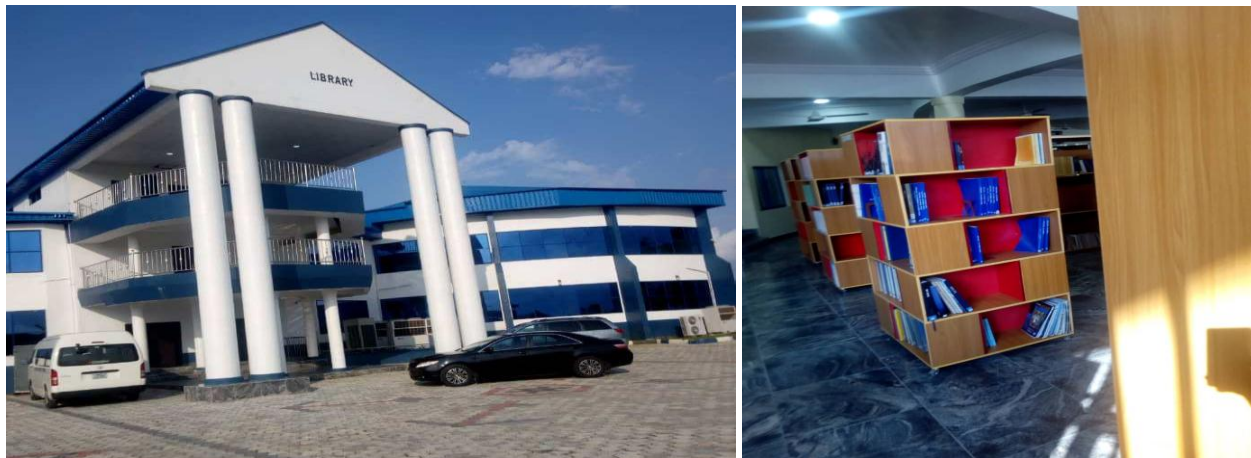
Picture 13: Completed Library/Resource Centre at the Maritime Academy, Oron
