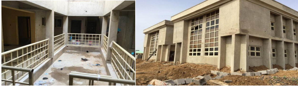
Picture 29: Construction of Office Complex, Classes and Laboratory at the College
