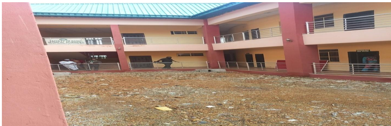
Picture 41: Completed College of Medicine Academic Block Federal University, Ndufu-Alike, Abakaliki
