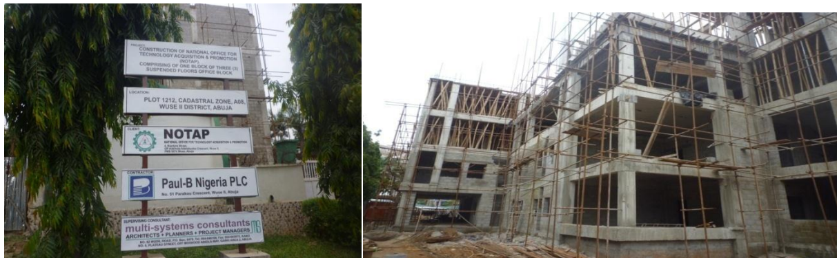
Picture 47: Construction of Headquarter Office Building at NOTAP, Abuja
