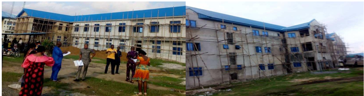
Picture 12: Completion Works of Male Cadet's Hostel at MAN, Oron
