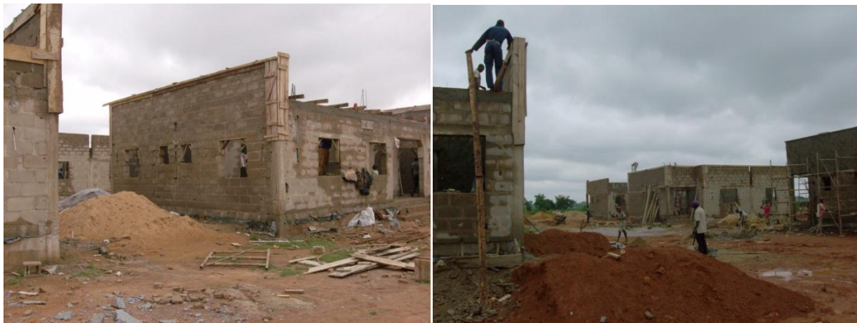
Picture 40: Ongoing Construction of Residential Quarters for Corporals at NDA, Kaduna
