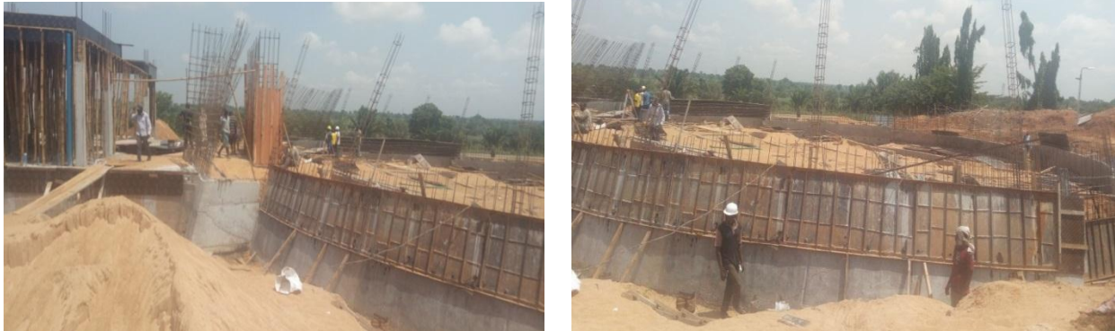
Picture 33: Ongoing Construction of Senate Chamber at the FUA, Makurdi
