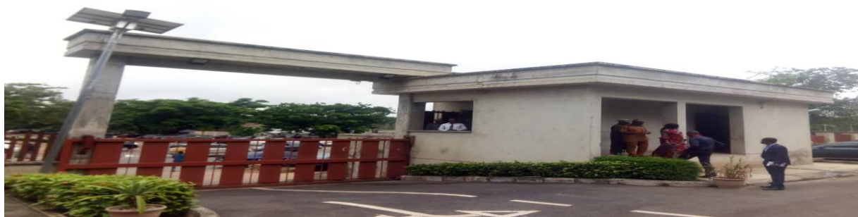
Picture 55: Completed Security Out-Post and a Motorized Gate at the Nigeria Export Promotion Council, Abuja
