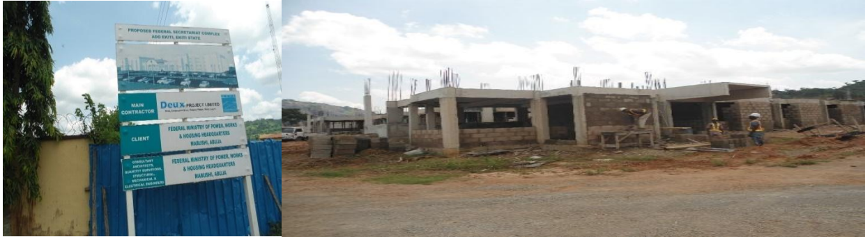
Picture 7: On-going Construction of Federal Secretariat Building, Ekiti, Ekiti State
