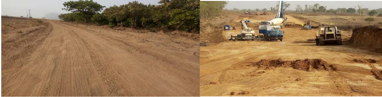
Picture 54: Completed Portion of the Earth Works and Ongoing Piling Work at Bridge Nos 4 at CH 16+000
