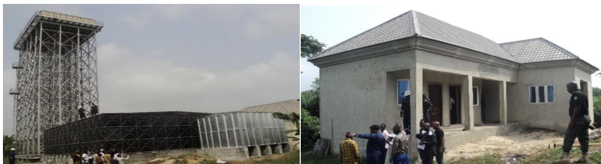
Picture 59: Some of the Borehole Facilities at the Petroleum Training Institute, Effurum
