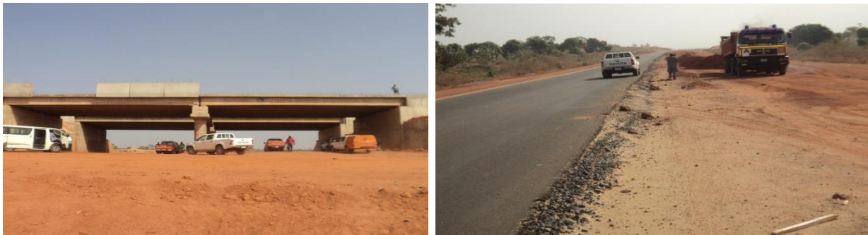
Picture 11: Ongoing Construction Works at the Kaduna Eastern Bypass
