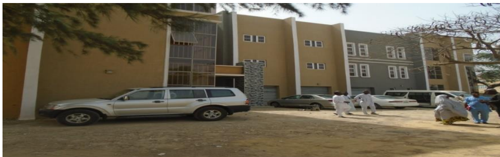
Picture 42: Completed Library Complex at the School of Continuous Education (SCE), Kano
