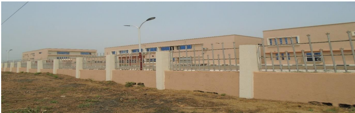
Picture 26: Completed Zonal Outreach Learning Centre at Eddah, Afikpo L.G.A, Ebonyi State
