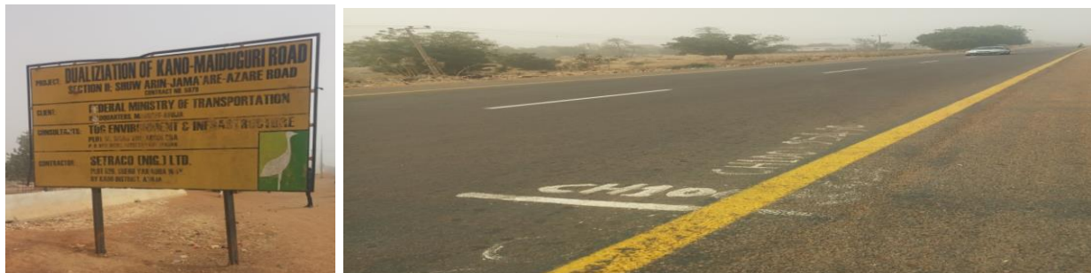
Picture 13: Completed Portion of Dualization of Kano – Maiduguri Road, Section II (Shuwarin-Azare)
