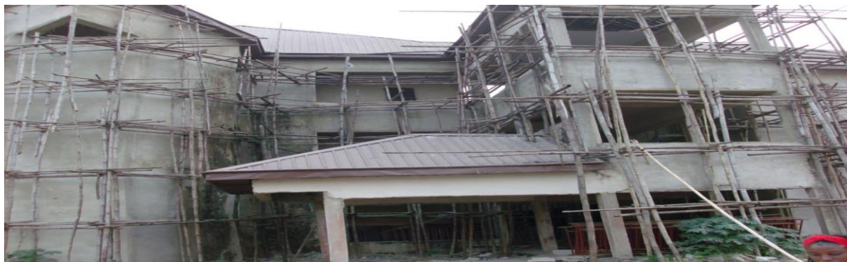
Picture 38: Ongoing Construction of School of Science Phase-I Complex at FUTO, Owerri
