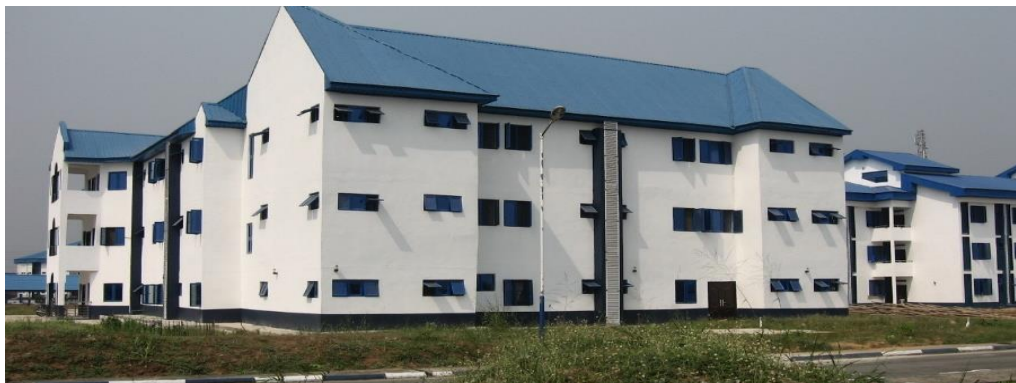
Picture 28: Completed 200 Capacity Male Cadet Hostels at MAN, Oron
