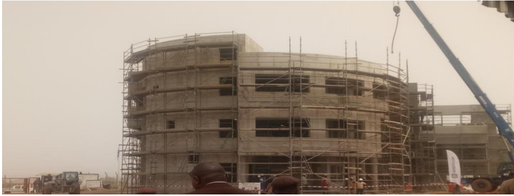
Picture 57: On-going Construction of Technology Building at Nigerian Immigration Service Headquarters, Abuja
