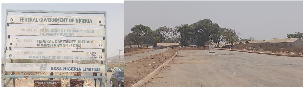
Picture 56: Provision of Primary Road to Mass Housing (Phase I) at Kabusa, Apo District, Abuja
