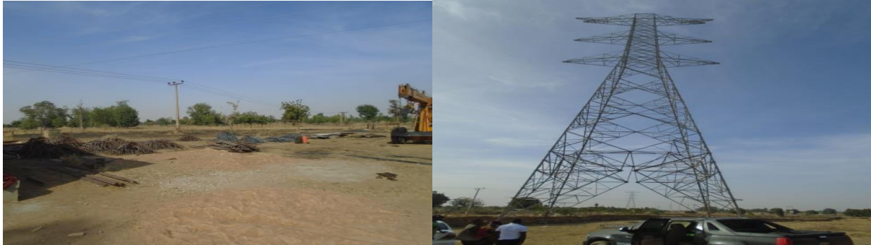
Picture 9: Ongoing Transmission Line of 33KV DC from Kano – Katsina
