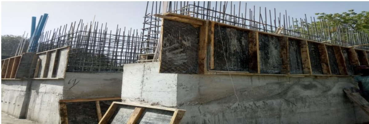
Picture 37: Ongoing Construction of Radiotherapy Centre at University of Maiduguri Teaching Hospital
