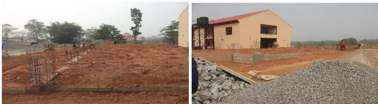
Picture 45: Ongoing Construction of School of Information and Communication Technology Building at FUTA Phase II
