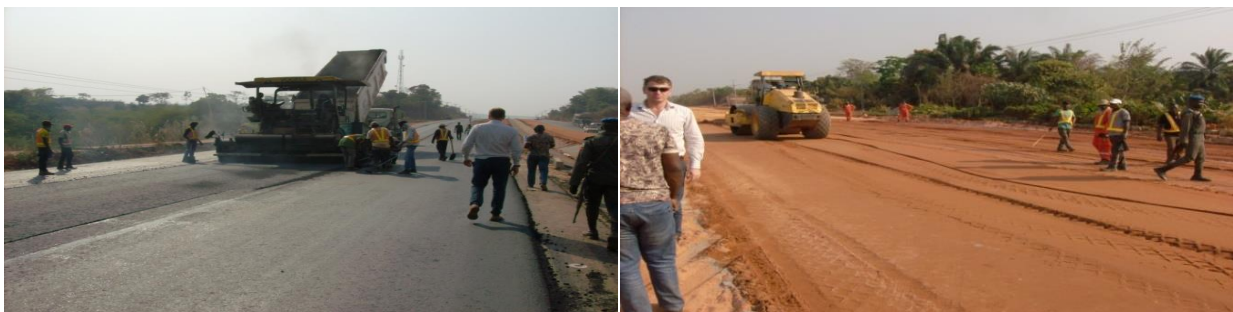
Picture 14: On-going Rehabilitation of an outstanding section of Onitsha – Enugu Expressway
