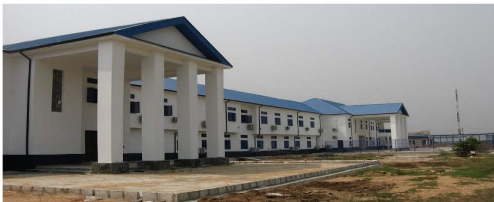
Picture 27: Completed Nautical Complex at MAN, Oron
