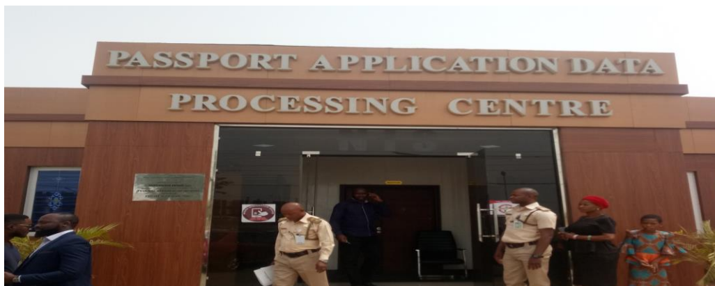
Picture 58: The Constructed Passport Application Data Processing Centre at NIS Headquarters, Sauka - Abuja
