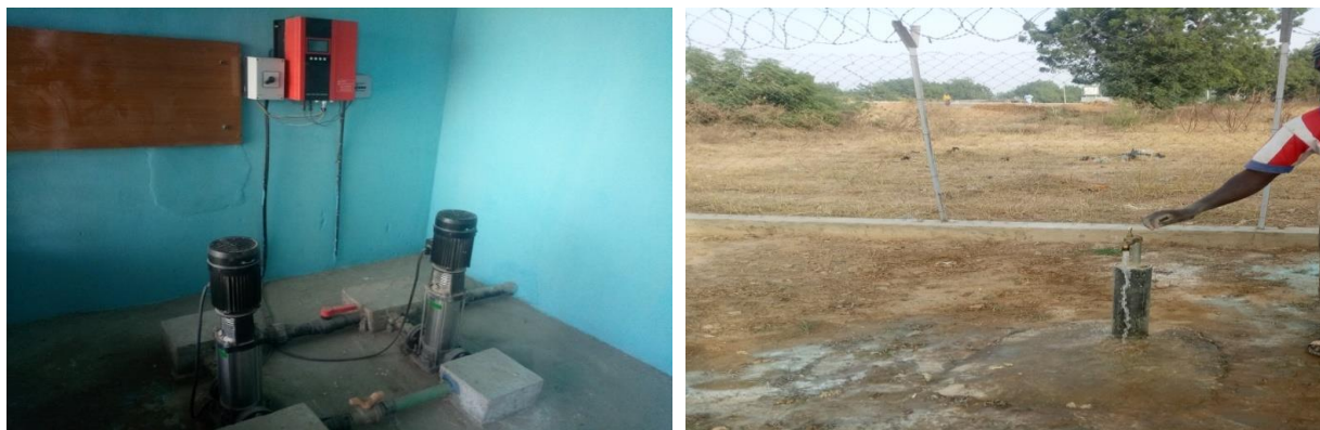
Picture 24: Completed Solar Powered Borehole at Gambaki Water Supply Scheme, Bauchi State
