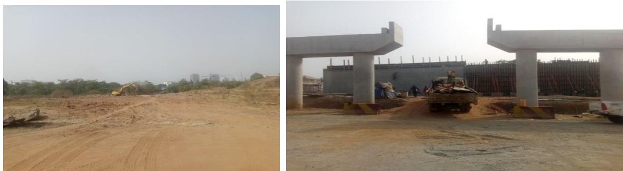
Picture 53: On-Going Excavation Works for River Parapata Bridge and Casting of Retaining Wall at Galadimawa Bridge
