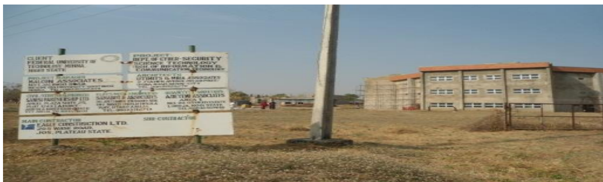
Picture 39: On-going Construction of Cyber Security Science Department at FUT Minna
