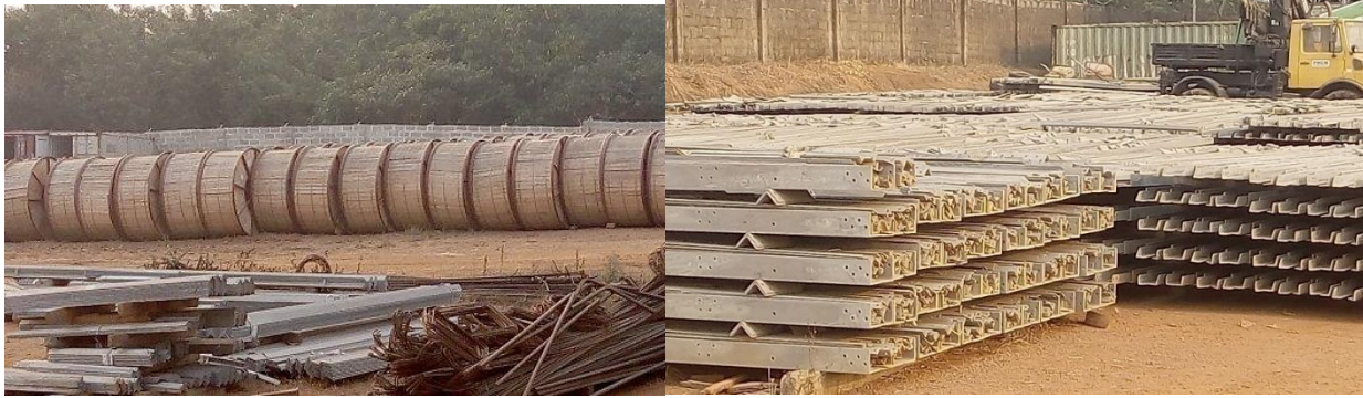
Picture 8: Some of the Materials Procured for 330KVA Double Circuit Transmission Line at the Energo Yard in Ijebu-Ode, Ogun State
