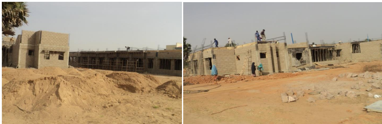
Picture 40: Ongoing construction of Venom, Anti-Venom and Natural Toxin Research Centre at ABU, Zaria.
