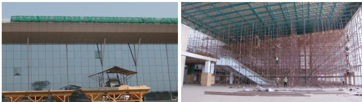
Picture 32: On-Going Construction of Terminal Building and a Cargo at Akanu – Ibiam International Airport, Enugu
