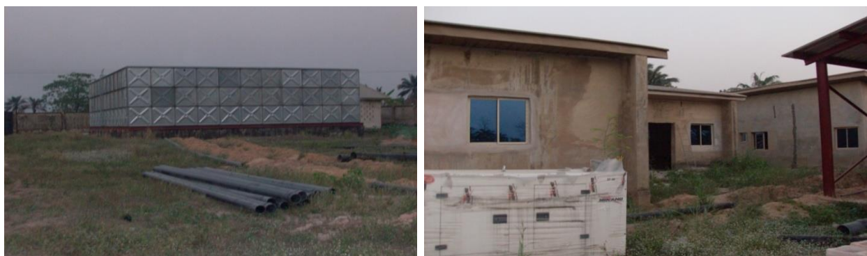
Picture 25: Water Tank and the Administrative Block almost completed at The Ivo Water Supply Scheme
