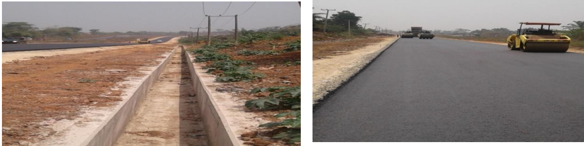
Picture 12: On-going Rehabilitation/Reconstruction of Enugu-Port Harcourt Dual-Carriage Section II
