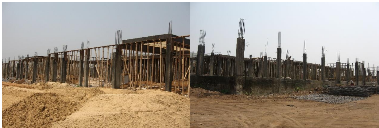
Picture 44: Ongoing Construction of Faculty of Agriculture Complex (Phase I), University of Uyo
