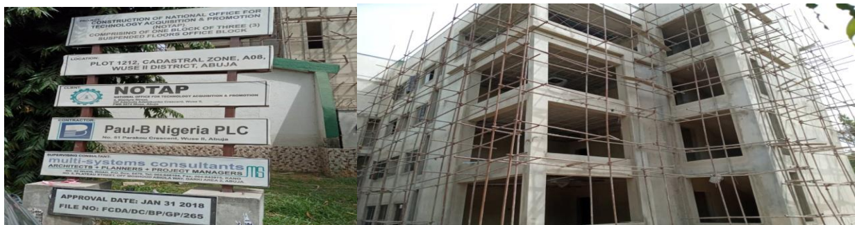
Picture 46: Ongoing Construction of the NOTAP Headquarters office building, Abuja
