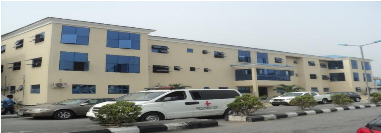
Picture 34: Completed Construction of Surgical Ward Block
