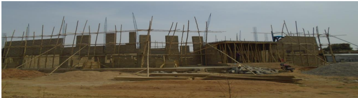
Picture 47: Construction of Leather and Computer Aided Design Multipurpose Hall
