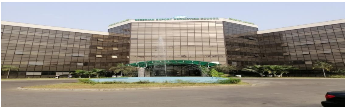
Picture 68: Completion of Headquarters Building at NEPC, Abuja.
