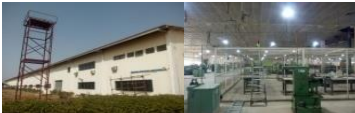
Picture 1: Some of the Rehabilitated Facilities at DICON, Kaduna
