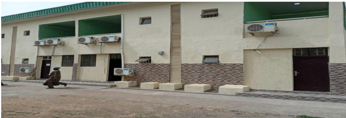
Picture 48: The Renovated Temporary Administrative Building at NASRDA, Abuja
