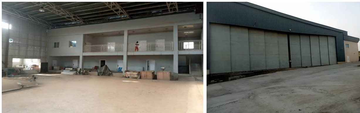
Picture 31: The Completed Wreckage Hangar at Nnamdi Azikiwe International Airport, Abuja
