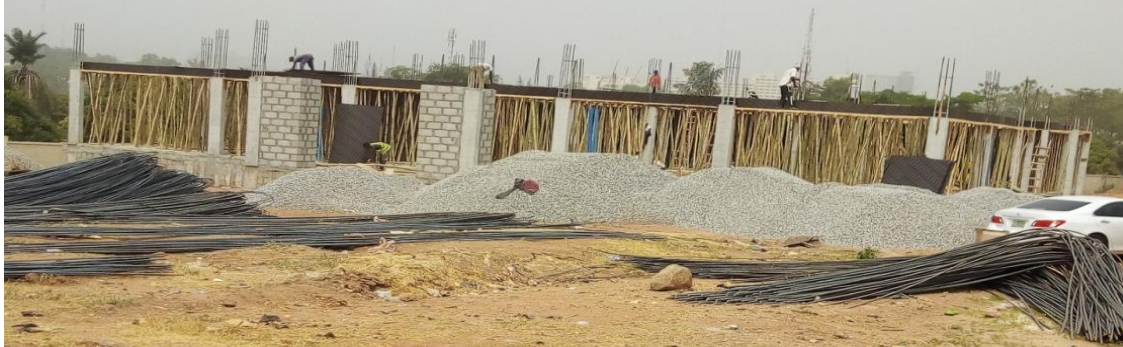
Picture 3: Ongoing construction of DRDB Headquarters Annex Building
