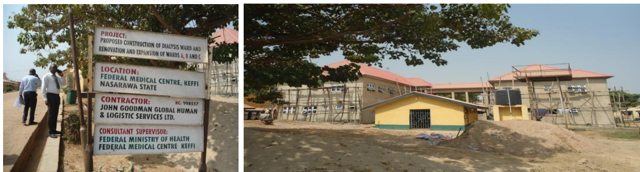
Picture 35: On-going Renovation/Expansion Works of Patient's Ward and Dialysis Centre at FMC Keffi
