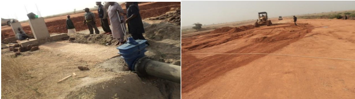
Picture 21: Water Intake Works and Construction of Dam Axis in Progress at Bangola Earth Dam in Kebbi State
