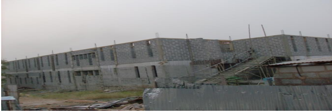
Picture 36: Ongoing Construction of Out Patient Building Complex at FMC, Owerri.
