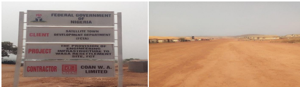
Picture 55: Ongoing Road Construction at Engineering Infrastructure To Wasa Resettlement Site I
