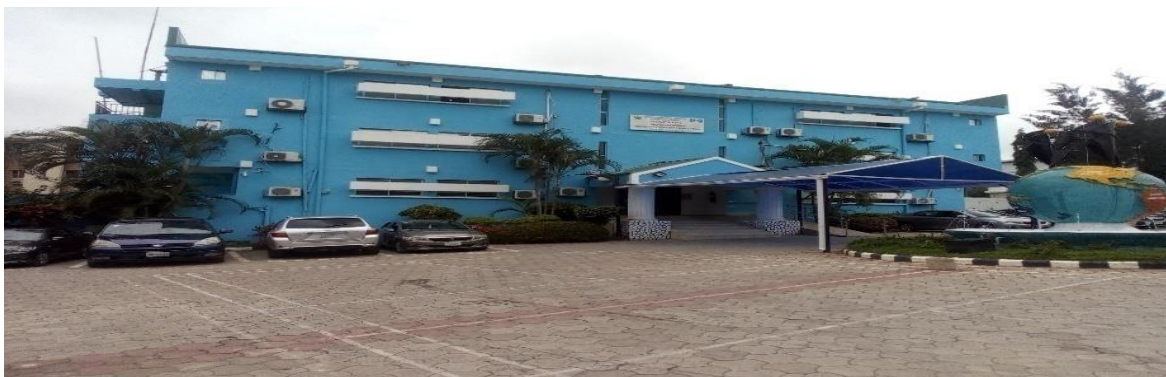
Picture 89: Renovated Headquarters Main Building at NATIP
