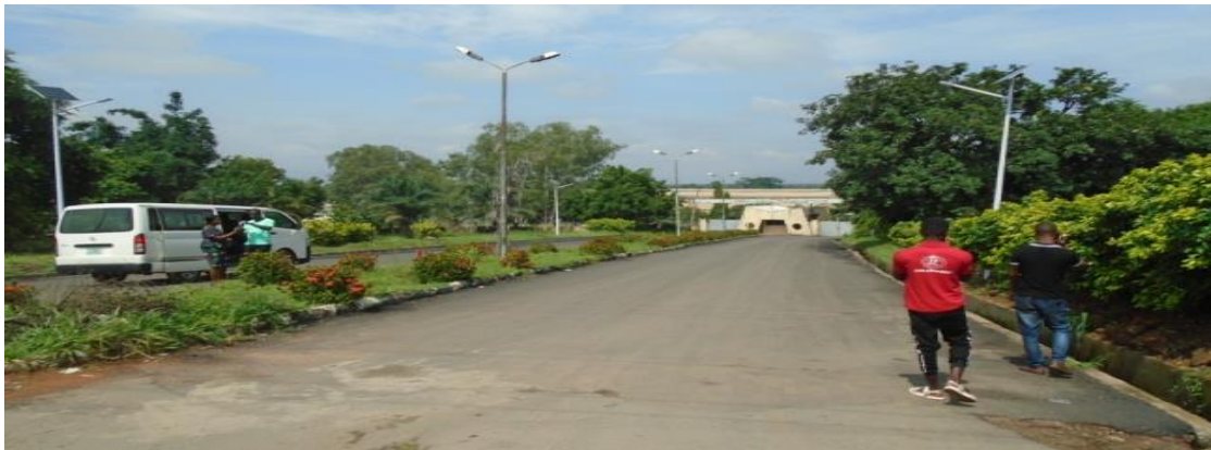
Picture 80: The Completed Rehabilitation of Internally Ravage Road at MTI, Onitsha
