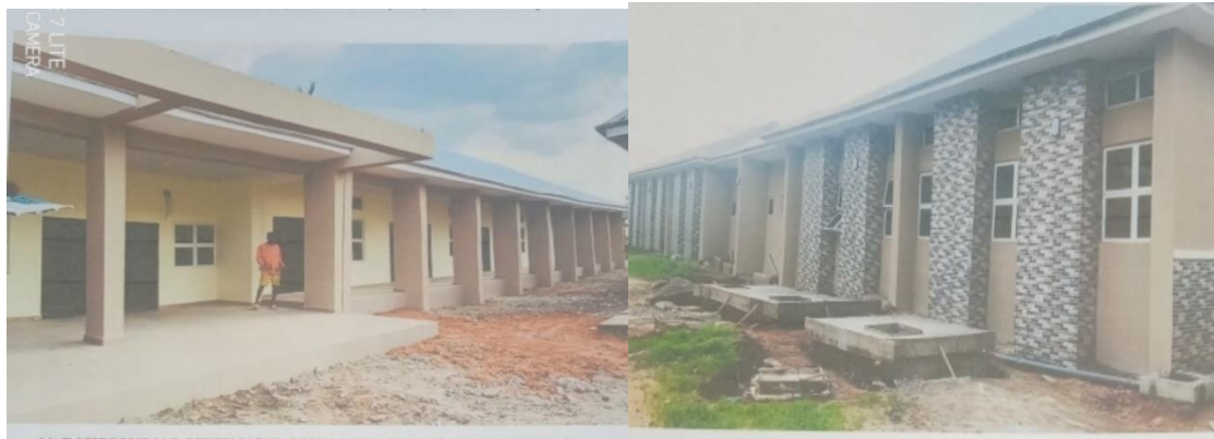
Picture 33: The completed construction of classrooms at the University
