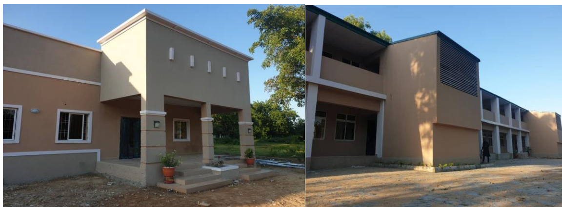
Pictures 37: Rehabilitated of College of Veterinary Medicine and School of Sciences at Federal University of Agriculture, Zuru
