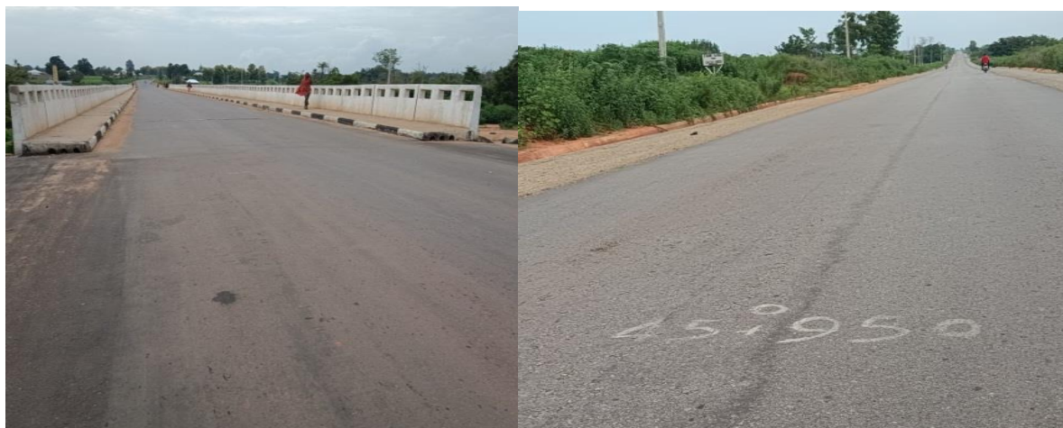
Picture 4: Ongoing Construction of Loko-Oweto Road in Nasarawa State
