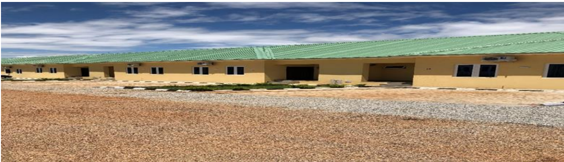
Picture 49: Completed 8NR, 2-Bedroom Bungalow for Officers at Nigeria Defence Academy, Kaduna
