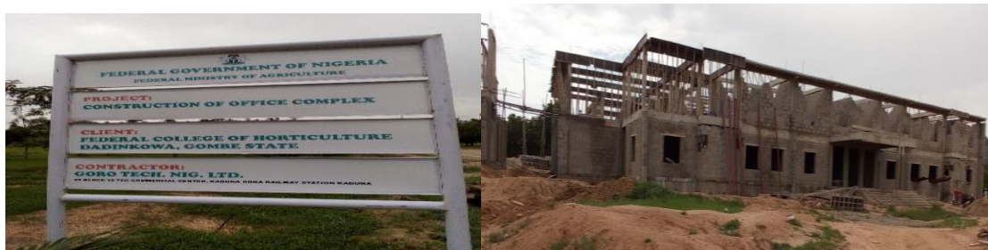
Picture 39: Ongoing Construction of Office Complex at the Federal College of Horticulture Dadin Kowa, Gombe State
