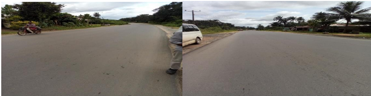
Picture 3: Constructed Portion at Abak-Ekparakwa-Ette-Ikot Abasi Road in Akwa Ibom State
