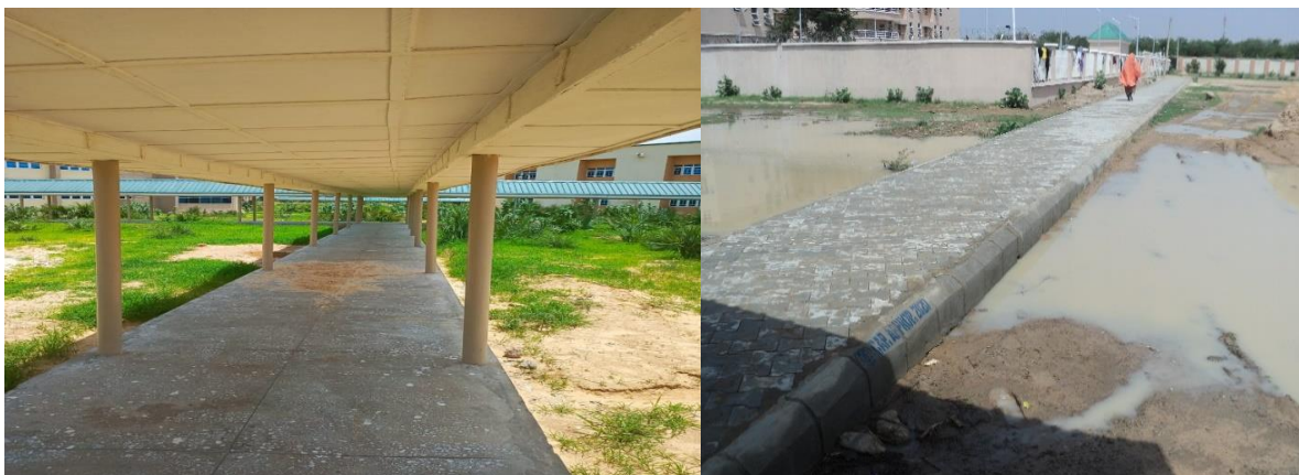
Picture 28: Completed Construction of Walkway at the Federal University, Gashua
