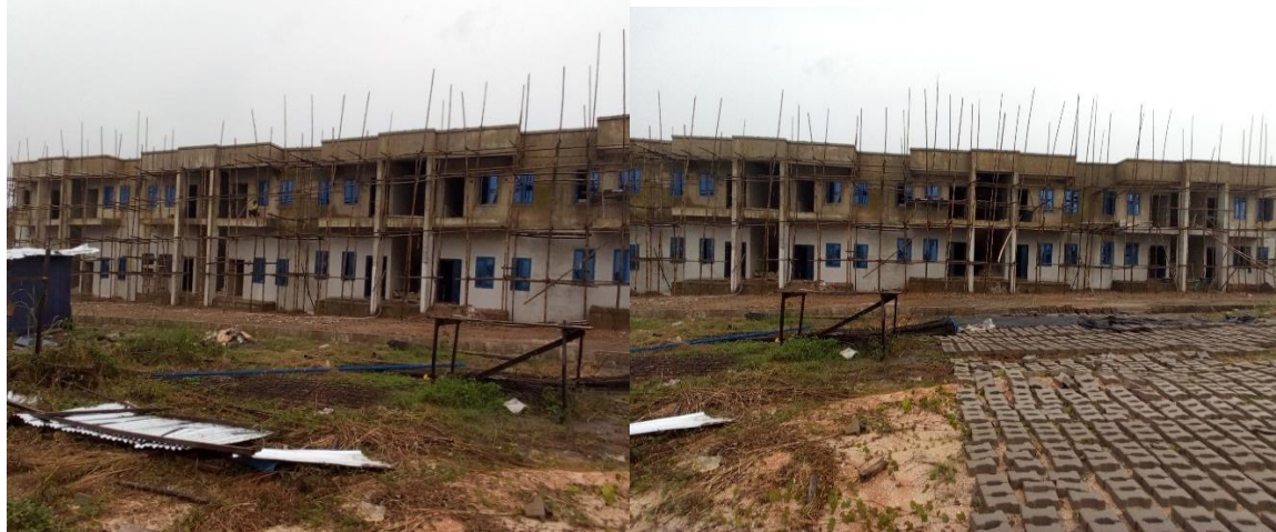
Picture 71: Ongoing Completion of 200-Capacity Male Cadets' Hostel at Maritime Academy, Oron
