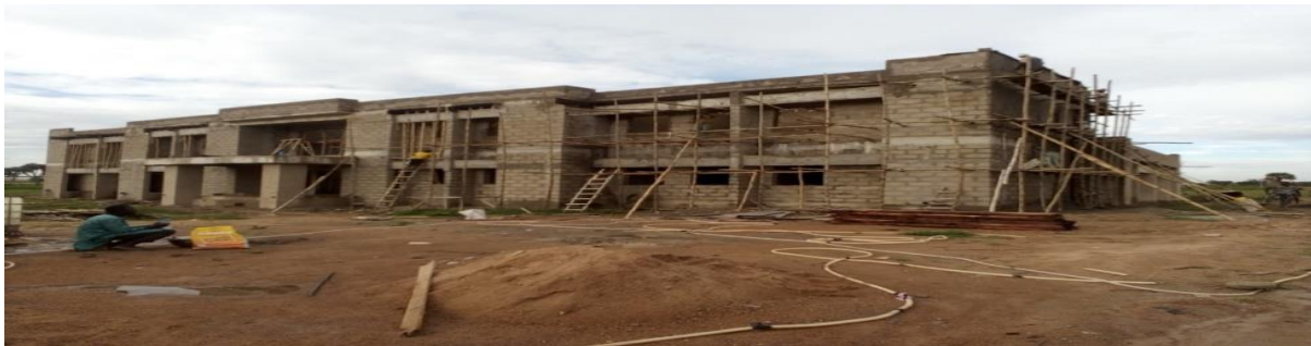
Picture 22: Ongoing Construction of Faculty of Veterinary Medicine at BUK
