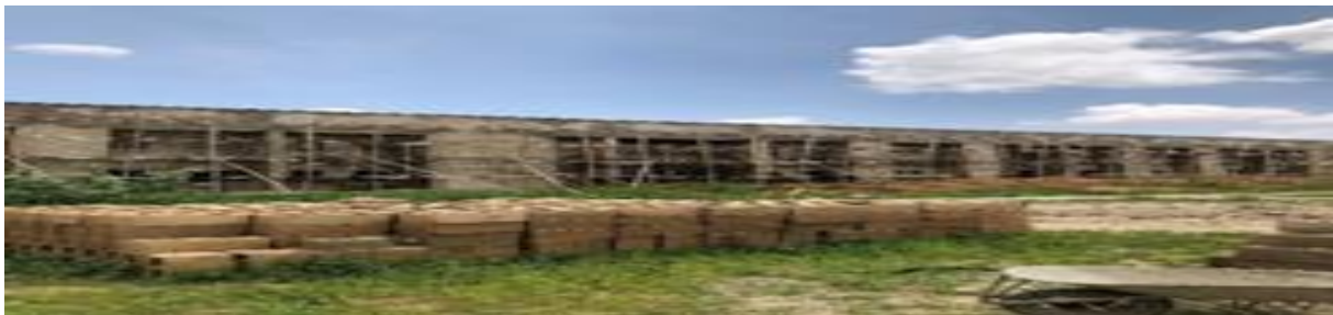
Picture 19: Ongoing Construction of Veterinary Medicine at UDU, Sokoto
