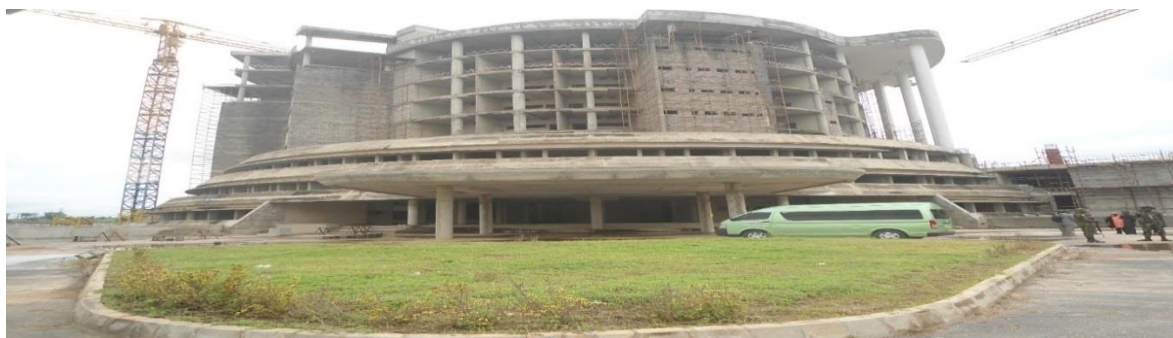
Picture 52: Ongoing Construction of Administrative Block at Permanent Site Piwoyi (Phase I), NDC Headquarters, Abuja
