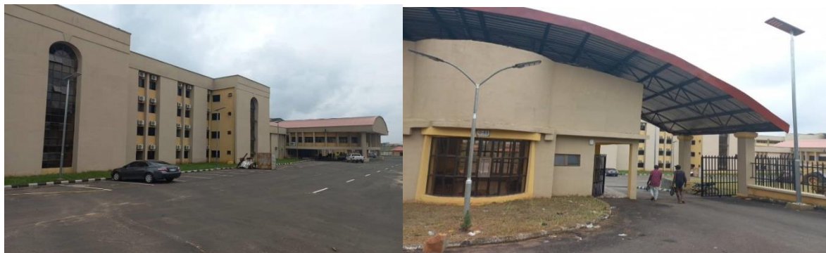
Picture12: Completed Federal Secretariat Building at Awka, Anambra
