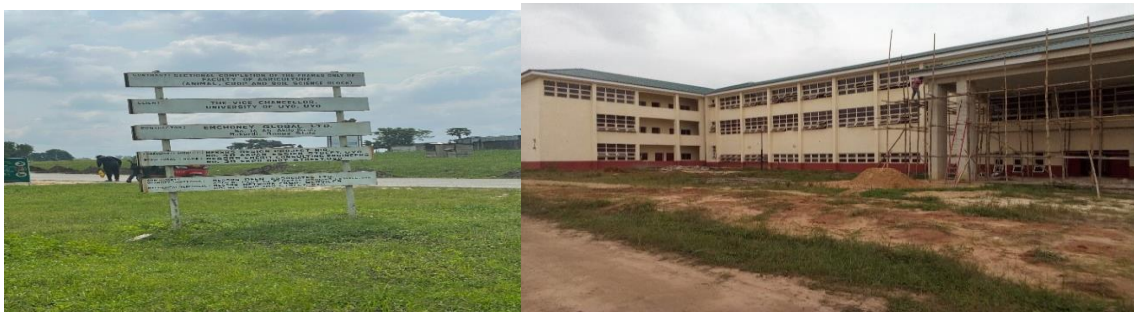
Picture 23: Ongoing Completion of Faculty of Agriculture Laboratory Block (Phase I) at University of Uyo
