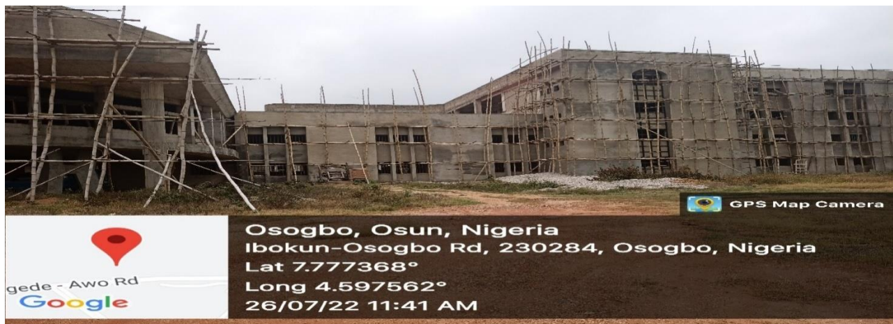
Picture 10: Ongoing Construction of Federal Secretariat Complex at Oshogbo, Osun State
