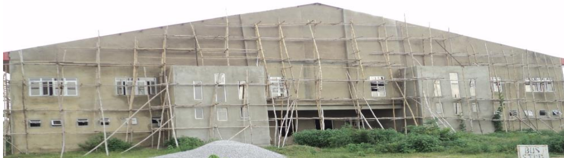
Picture 35: On-going construction of auditorium at Federal College of Education (Special), Oyo
