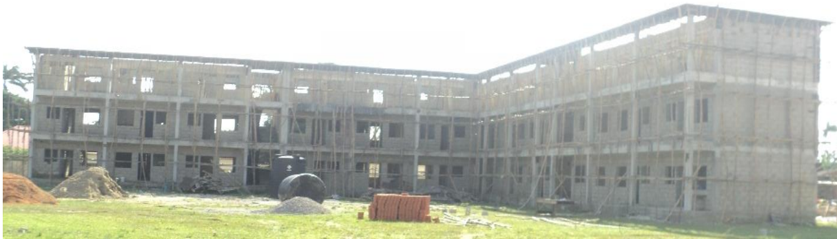
Picture 52: Ongoing Construction of Transit Flats for Corporal and Below Officers of NAFRC, Oshodi
