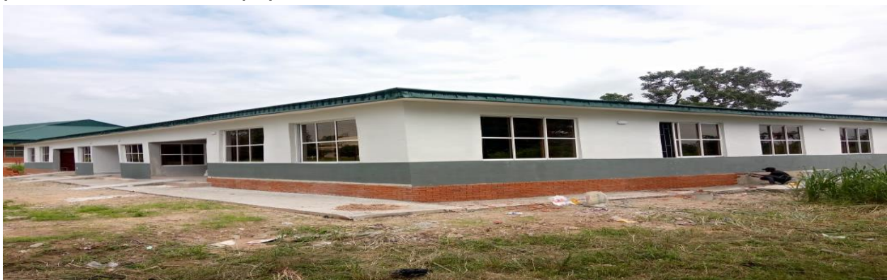
Picture 79: Completed Engineering Laboratory at MTI, Onitsha
