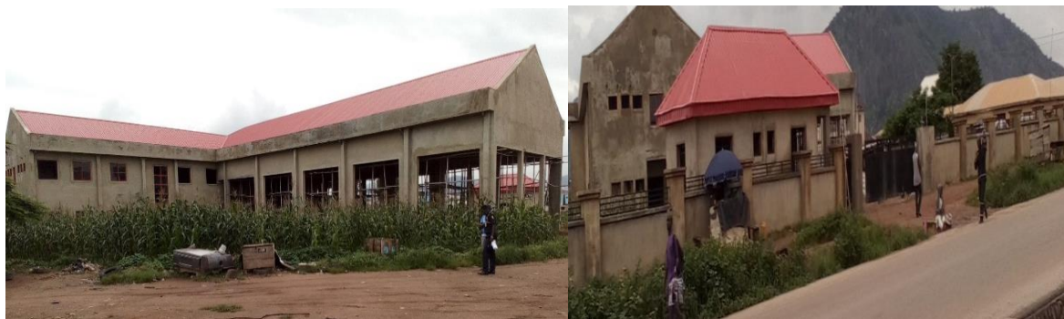
Picture 81: Metropolitan Fire Station, Gate House and Perimeter Fencing at the Federal Fire Service
