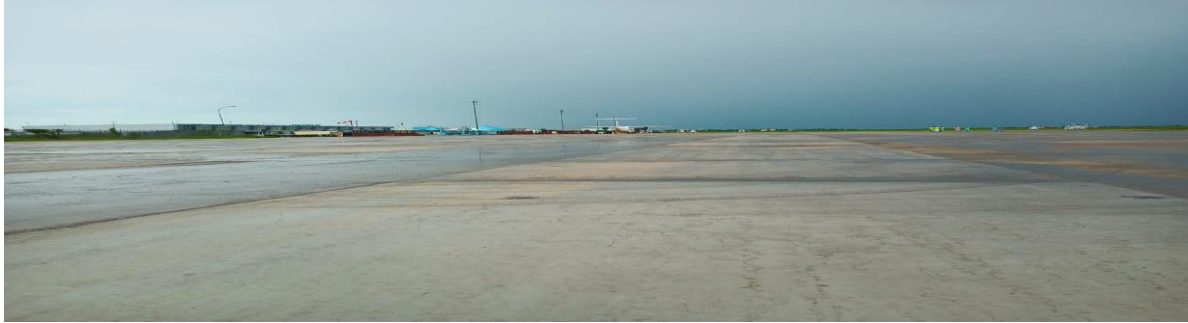
Picture 45: Ongoing completion of Maiduguri Apron Expansion at Maiduguri International Airport
