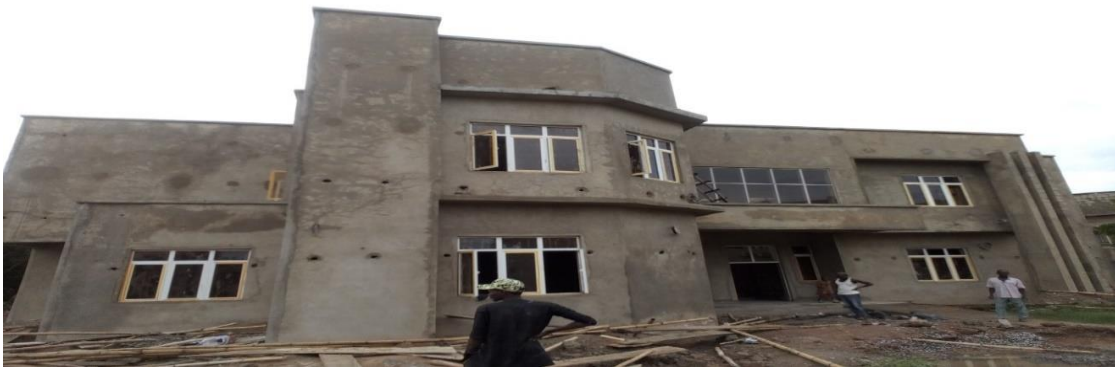
Picture 21: Ongoing Completion of centre for Teaching and Learning at BUK
