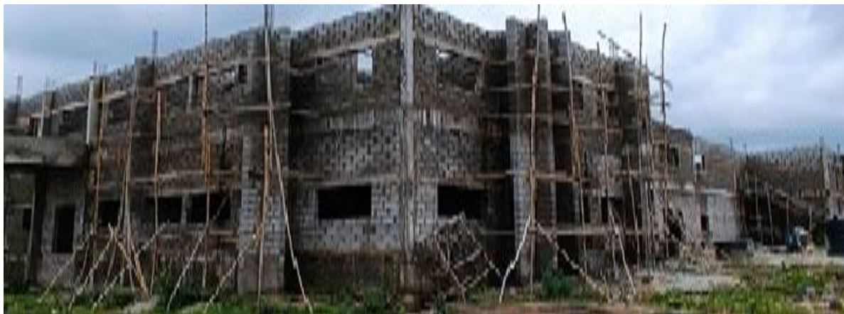
Picture 30: Ongoing Construction of the Pharmaceutical Department at University of Abuja
