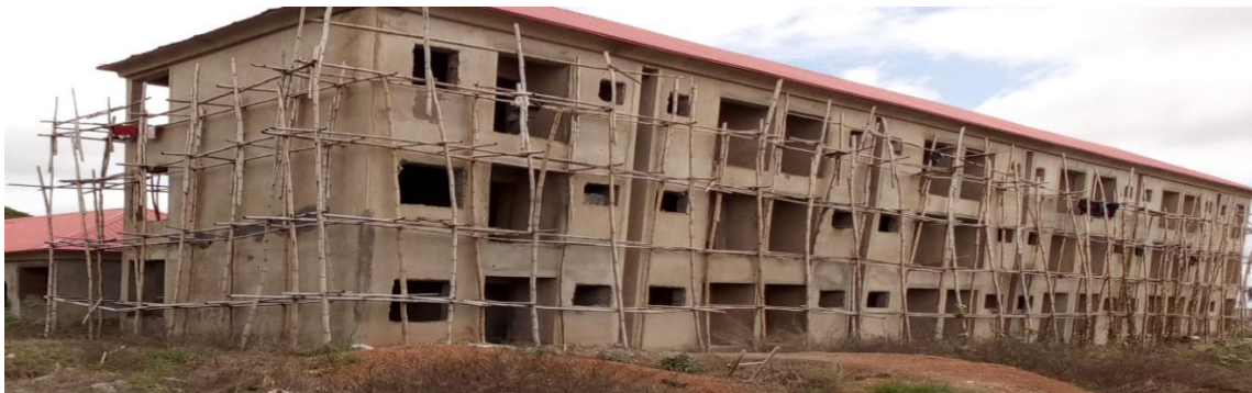
Picture 82: Ongoing Construction of Female Hostel at Federal Fire Service Academy, Sheda, Kwali Area Council
