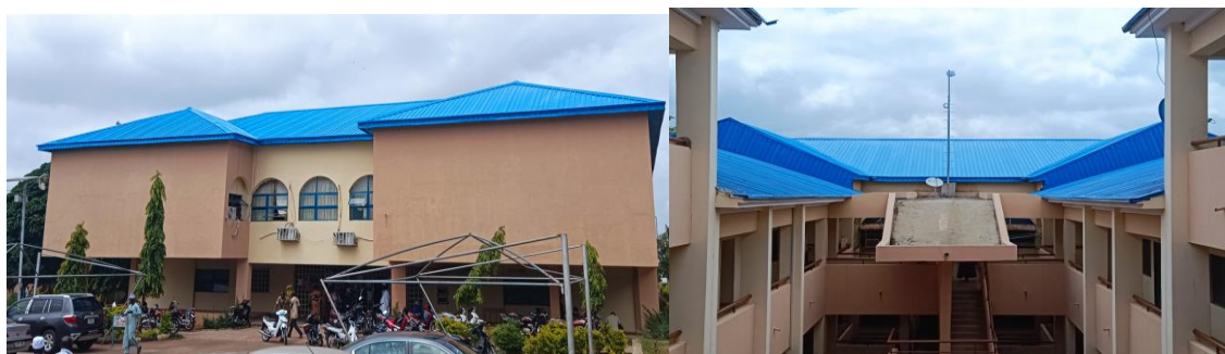
Picture 31: Rehabilitated Administrative Block at Federal Polytechnic, Bida
