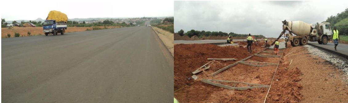
Picture 6: Ongoing Dualisation of Ibadan-Ilorin Road (Route A2), Section II: Oyo-Ogbomosho Road, C/No.1793A
