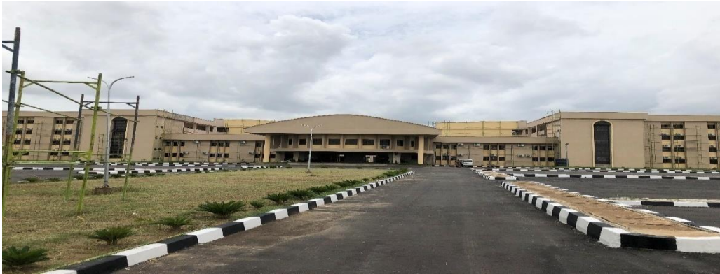
Picture 9: Ongoing Construction of Federal Secretariat, Gusau
