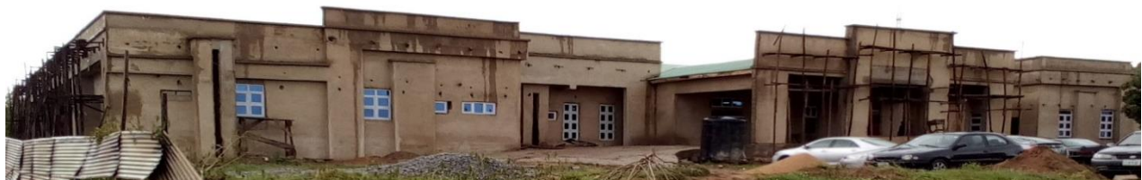
Picture 59: Ongoing Construction of Accident and Emergency Complex at Federal Medical Centre, Jalingo
