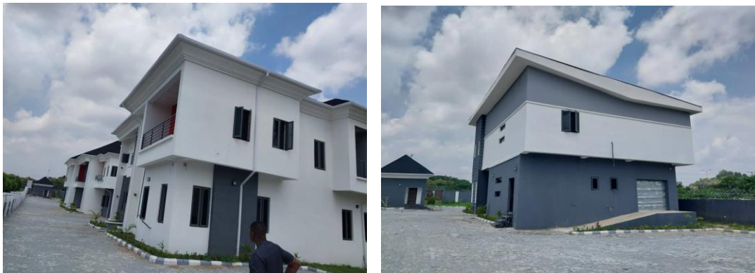
Picture 51: Completed Acquisition of Land and Construction of Barrack Accommodation for DSA at Karmo Abuja
