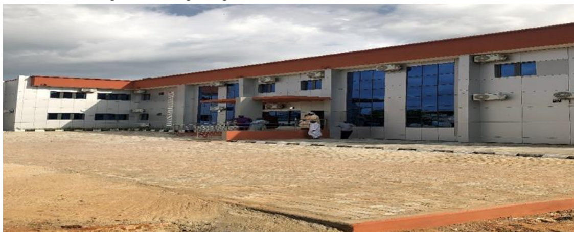
Picture 54: Completed Oncology Treatment Centre at ABUTH, Zaria.
