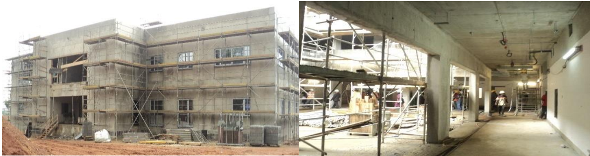
Picture 85: Ongoing construction of Presidential Wing State House Medical Centre, Abuja
