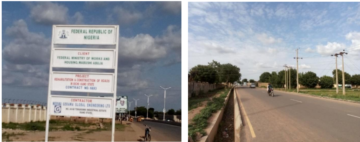
Picture 2: The Rehabilitated Portion of Bichi Road
