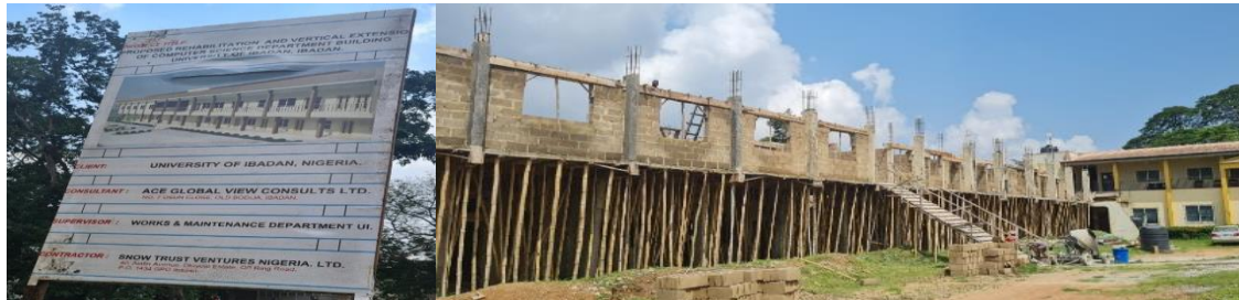
Pictures 34: Ongoing Rehabilitation and Extension of Computer Science Department Building at University of Ibadan
