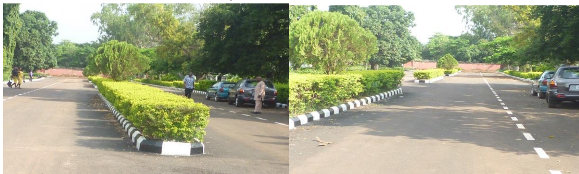
Picture 77: The Completed Rehabilitation of Internal Road Network at SEDI
