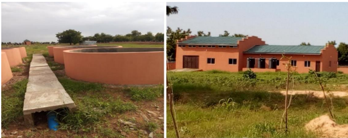
Picture 14: Completed Table Water Factory and Fish Pond at SRRBDA, Sokoto State
