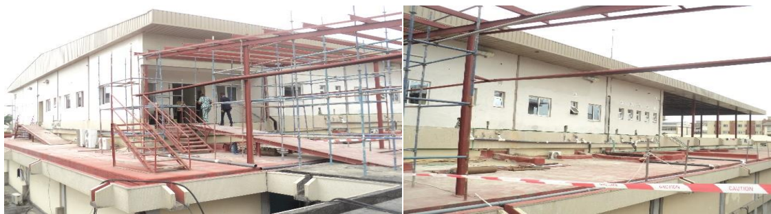
Picture 69: Ongoing Vertical Extension and Construction of ICU at LUTH
