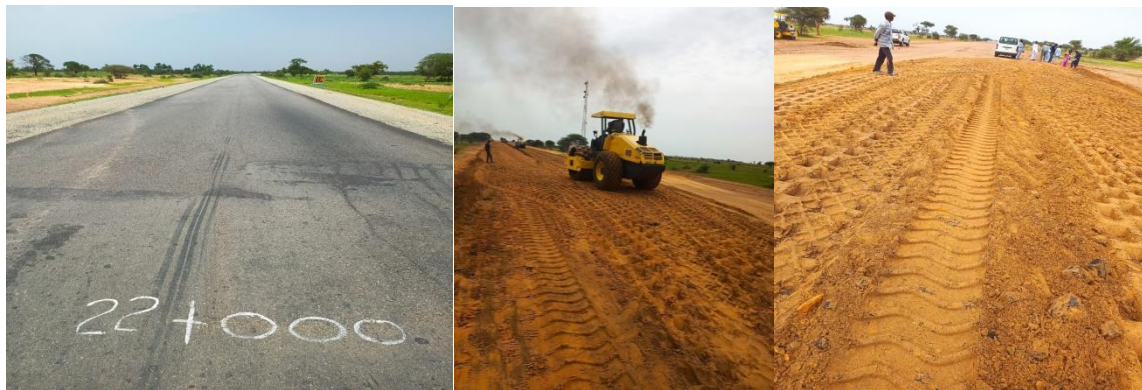
Picture 8: Completed Portion and On-going Works at the Rehabilitation of Nguru-Gashua-Bayamari Section II Phase II: (Gashua-Bayamari) Road in Yobe State
