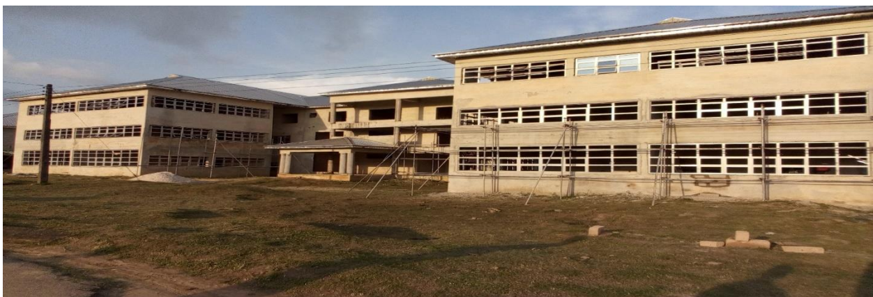
Picture 58: Ongoing Construction of Laboratory Building at University Teaching Hospital Uyo
