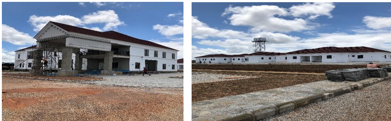
Picture 50: Ongoing Construction of Commandant's Residence at NDA, Kaduna
