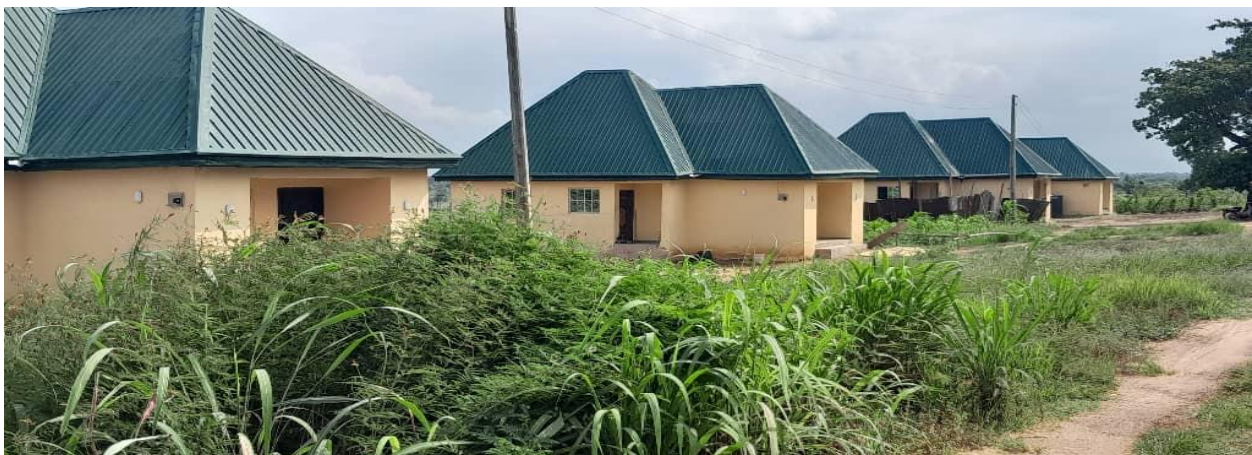
Picture 44: The Completed Farm Houses at Federal College of Agriculture Ishiagu
