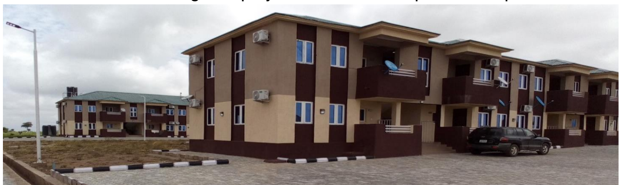
Picture 27: Completed Staff Accommodation at the Nigeria Army University, Biu
