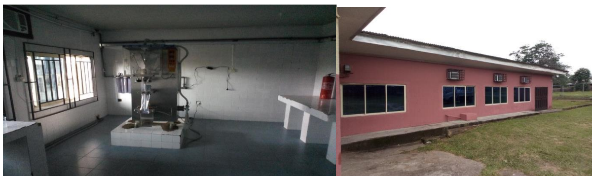
Picture 15: The Rehabilitated Water Factory and Supply/Installation of Water Dispensing Equipment and Accessories
