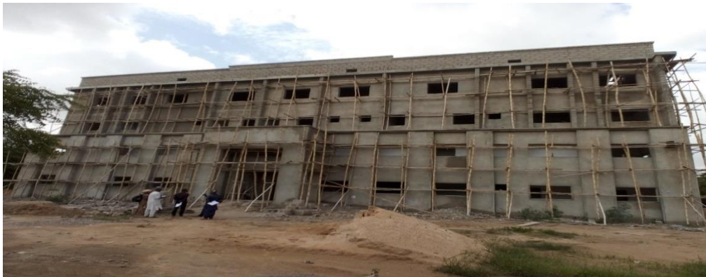
Picture 56: Ongoing Cardio Thoracic Centre Phase II at AKTH, Kano.
