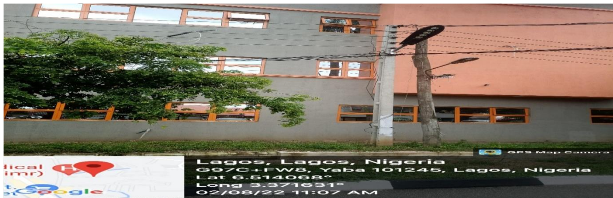
Picture 68: Ongoing Construction of Biorepository Facility Building at NIMR, Lagos State
