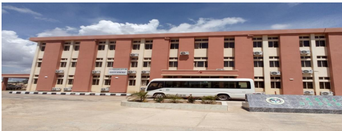
Picture 70: The Ongoing Construction of DG's Office at NITT, Zaria
