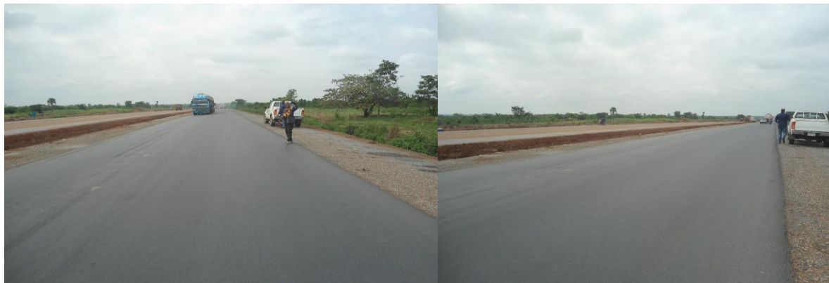
Picture 5: A portion of the Completed Asphalt Binder Course from KM 5.800 at Bode-Saadu Town Ilorin-Jebba Road
