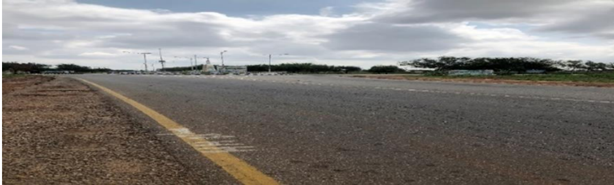
Picture 1: Completed Sokoto-Tambuwal - Jega – Kontagora Makera Road, Section I Sokoto/Kebbi State
