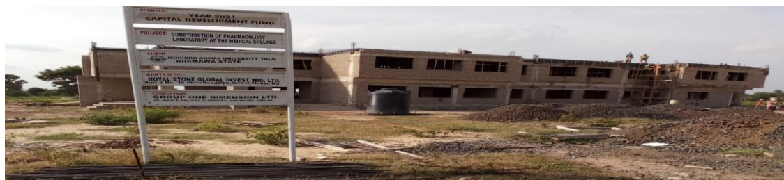
Picture 26: Ongoing Construction of Pharmacology Laboratory at the Moddibo Adama University, Yola
