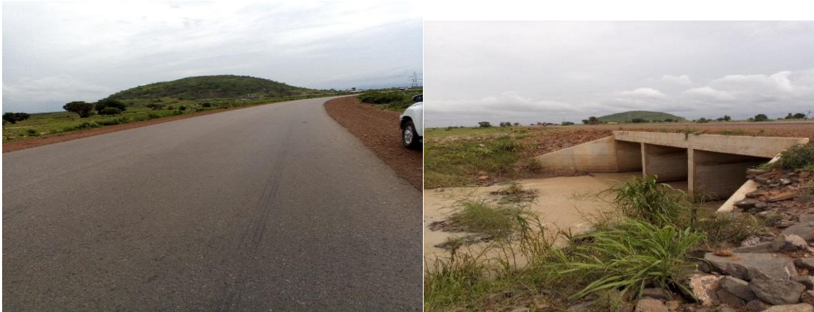
Picture 7: Ongoing Rehabilitation of Cham-Numan Section of Gombe - Yola Road in Adamawa State
