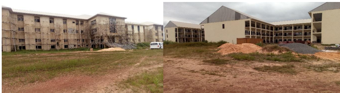
Picture 65: Ongoing Construction of a 2-Storey building at University of Nigeria Teaching Hospital, Enugu
