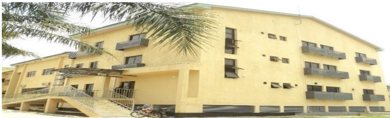
Picture 84: Completed Dental Wing Extension at State House Medical Centre
