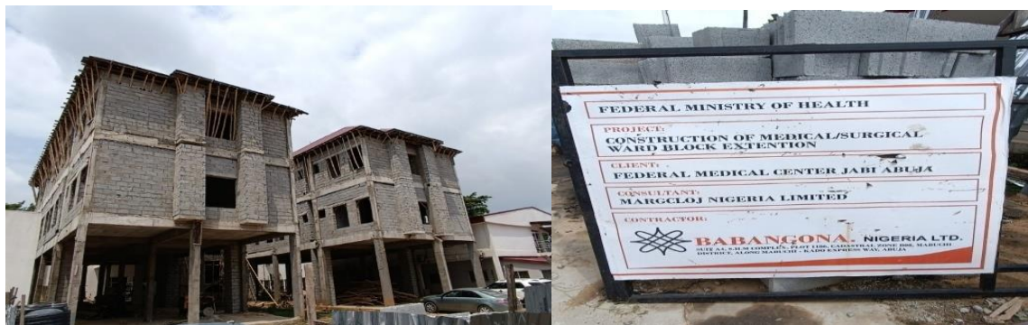
Picture 61: On-going Construction of Medical/Surgical Ward Block Extension at Federal Medical Centre, Jabi, Abuja
