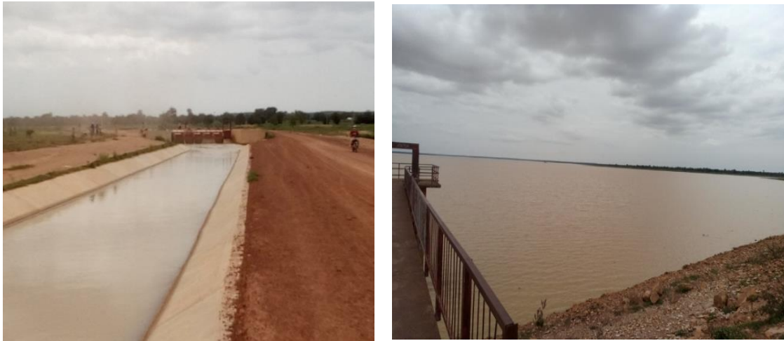
Picture 13: The Rehabilitated Gari Dam and the Distributary Canal at Gari Local Government Area of Kano State
