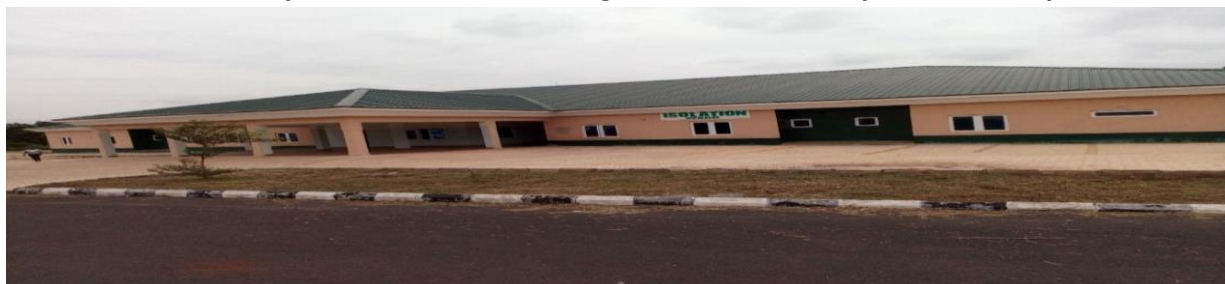
Picture: 64: Completed Isolation Centre at National Orthopaedic Hospital Enugu
