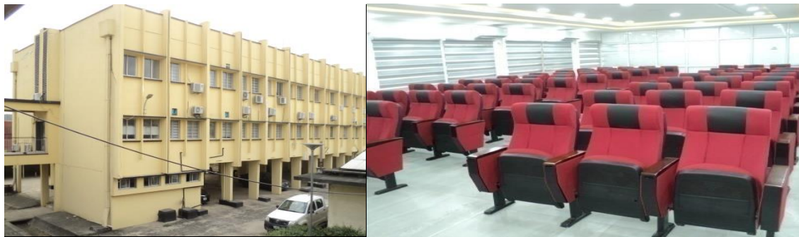
Picture 72: Completed Renovation of Directors' Block Building at NRC, Ebute-Metta
