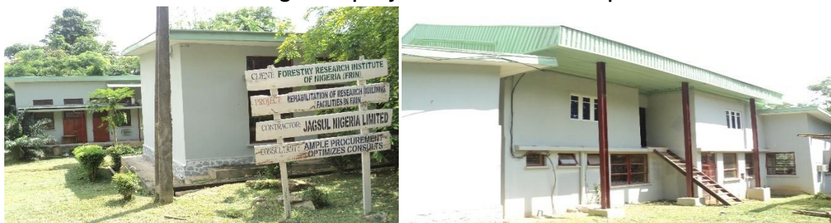
Picture 86: The Rehabilitated Research Building/Facilities at Forestry Research Institute of Nigeria
