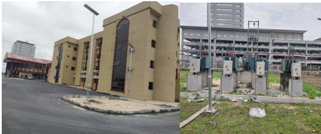
Picture 11: Ongoing Construction of Federal Secretariat Yenegoa, Bayelsa State
