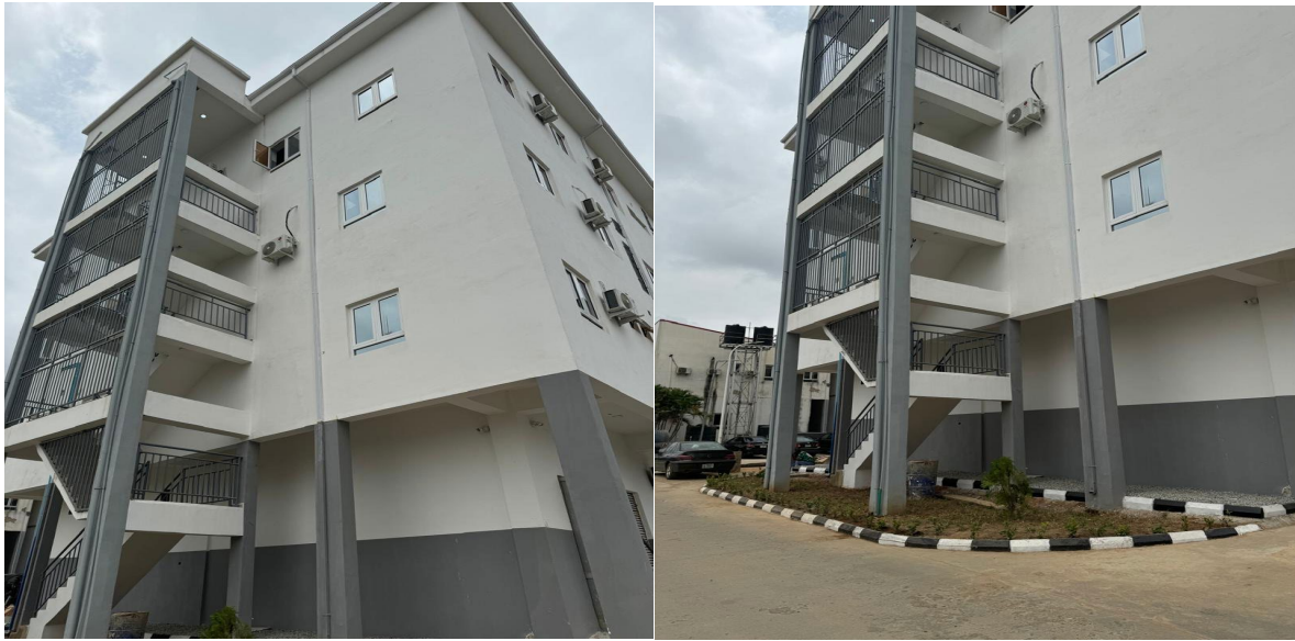
Picture 1: Completed 3-Storey Block of Clinical Services at FMC, Jabi.
