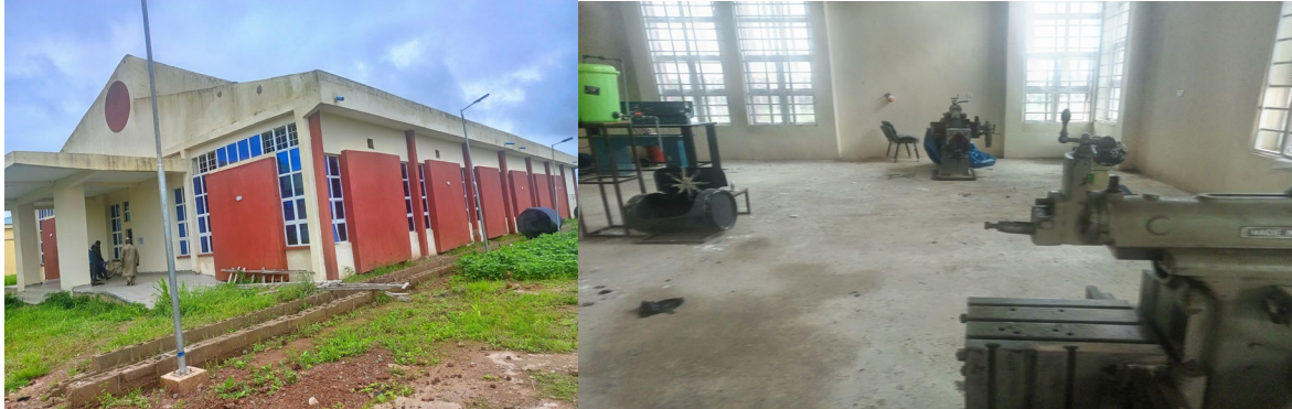
Picture 44: Completed Engineering Workshop in the Department of Civil Engineering at Nigeria Army University Biu
