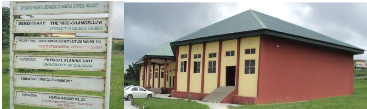
Picture 39: Completed 500-Seat Lecture Theatre for Faculty of Engineering at the University of Calabar.
