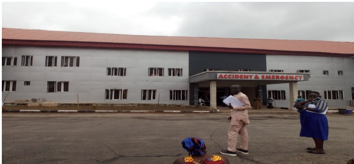
Picture 16: Completion of accident and Emergency complex at FMC Owo.
