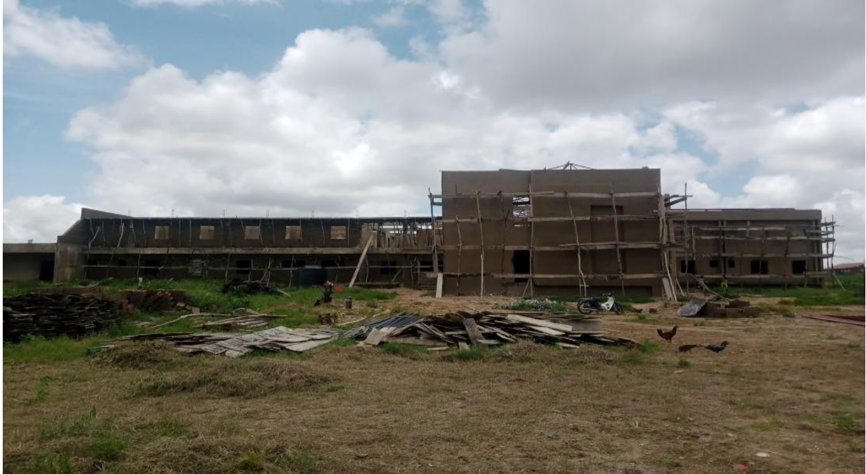
Picture 5: Ongoing Construction of Cardiology and Cardiothoracic Complex at ABUTH, Zaria.
