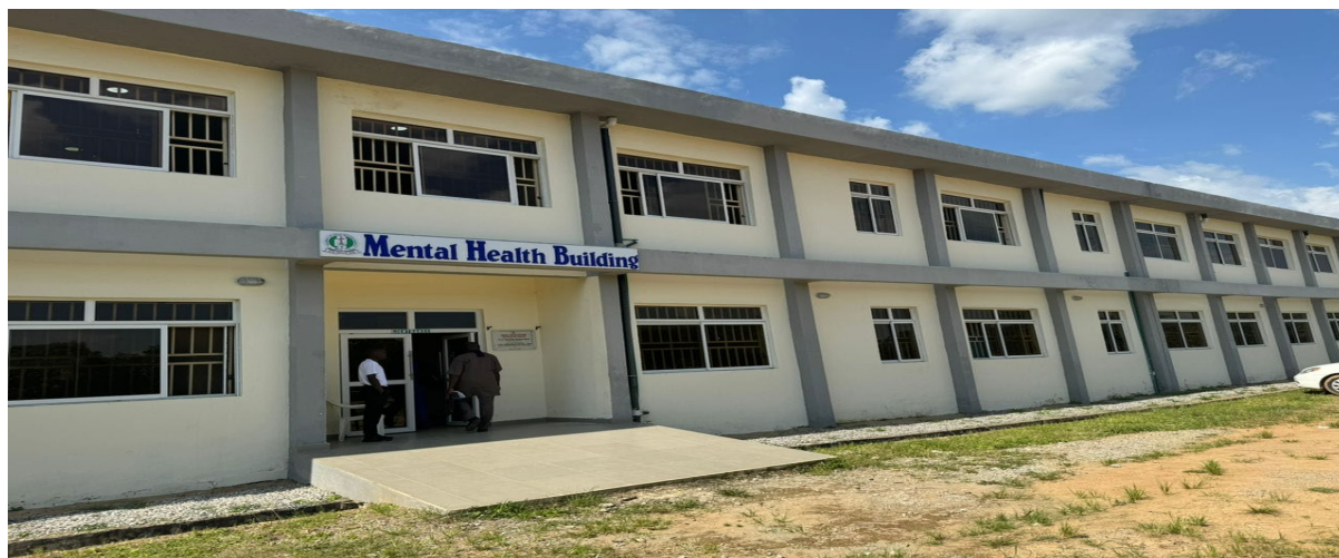
Picture 2: completed Mental Health Block at UATH, Gwagwalada
