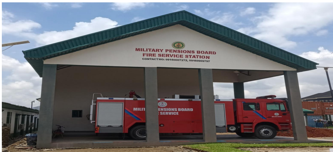
Pictures 67: Completed Fire Station at Military Pensions Board, Dutse, Abuja.
