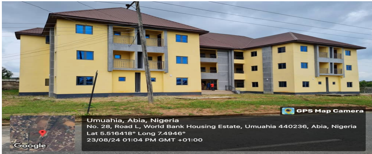
Picture 27: Completed Interns Quarters at FMC Umuahia, Abia State.
