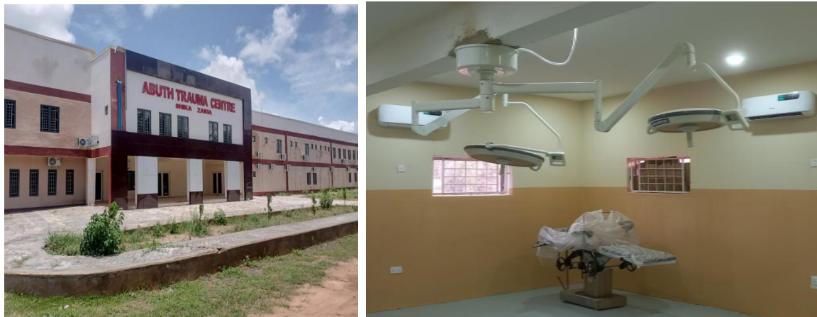
Picture 4: Completed Trauma Centre at ABUTH, Zaria.
