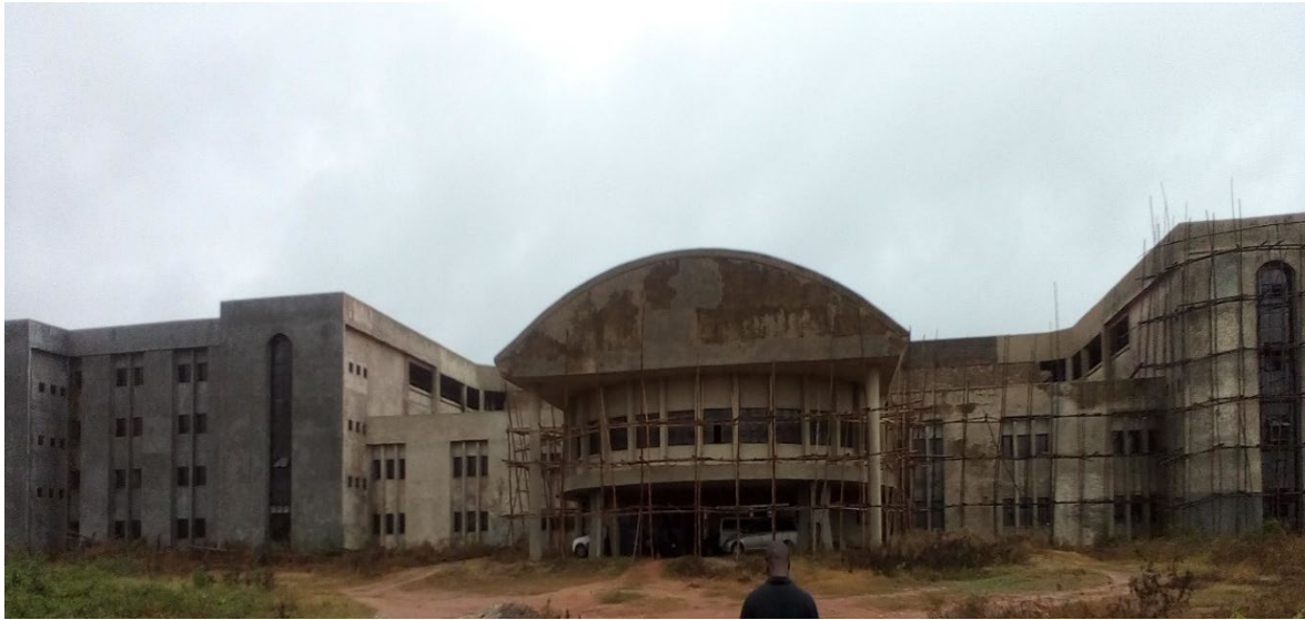
Picture 60: Construction of Federal Secretariat, Osun State.
