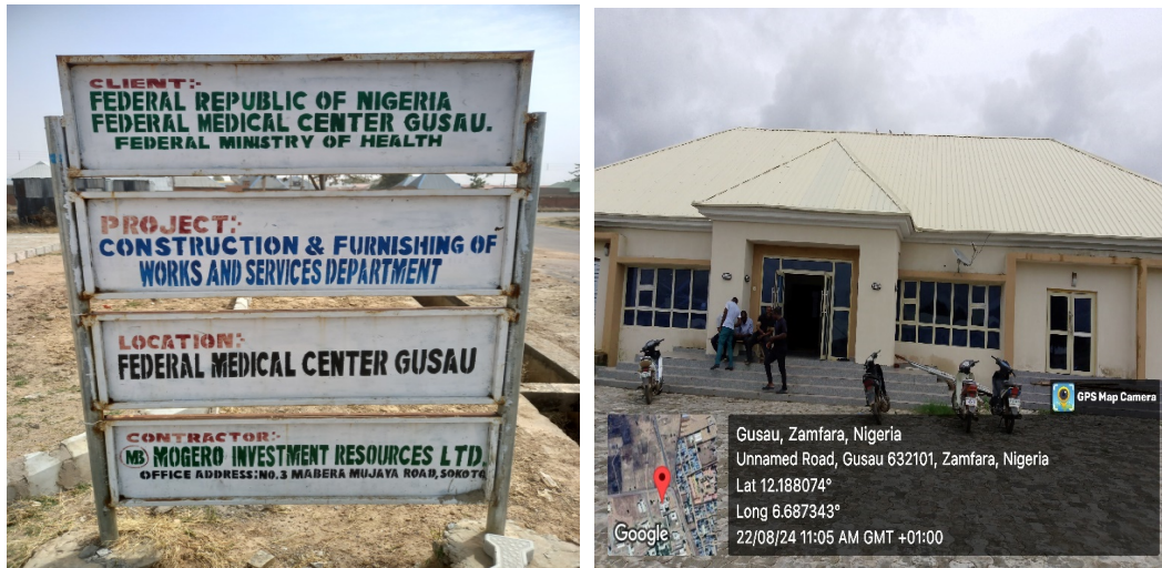
Picture 12: Completed Works and Services department building at FMC, Gusau
