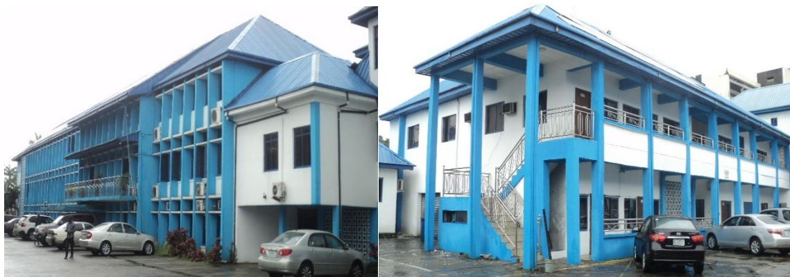
Picture 53: Rehabilitated Headquarters of Niger Delta River Basin Development Authority, Port Harcourt.
