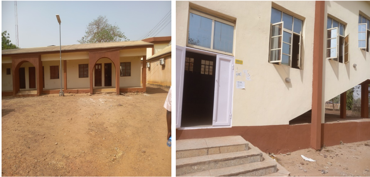
Picture 72: Rehabilitated classroom at Federal Cooperative College, Kaduna
