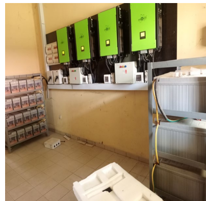
Picture 80: Installed Solar Power Back-Up Infrastructure for Sensitive High-Tech Equipment and Life Science.
