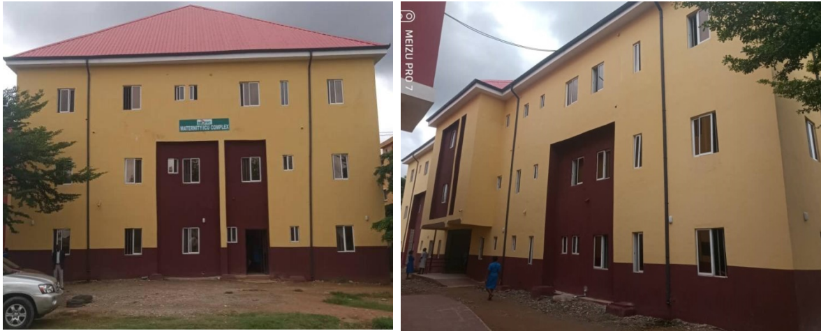
Pictures 20: Completed ICU Complex at National Obstetric Fistula Centre Abakaliki.
