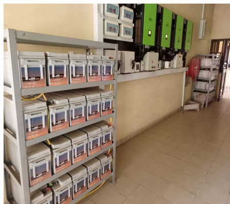
Picture 80: Installed Solar Power Back-Up Infrastructure for Sensitive High-Tech Equipment and Life Science.
