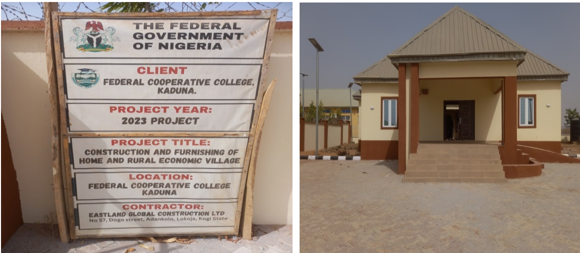
Picture 73: Completed home and rural economic village at Federal Cooperative College, Kaduna.
