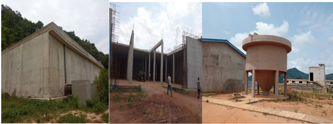
Picture 51: Ongoing water treatment reservoir in Kashimbilla and Takum town.
