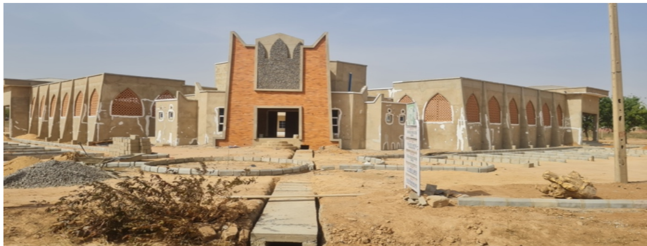
Picture 47: Ongoing Construction of Convocation Square at FCE, Katsina.
