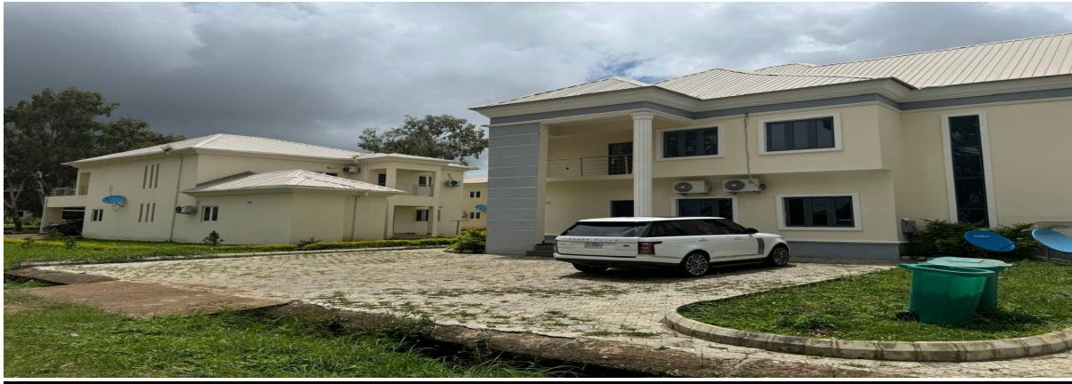
Picture 85: Renovated Research Fellows Quarters at NIPSS
