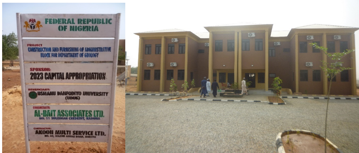
Picture 46: Completed construction and furnishing of Admin block for Geology Dept. at Usman Danfodio University, Sokoto.
