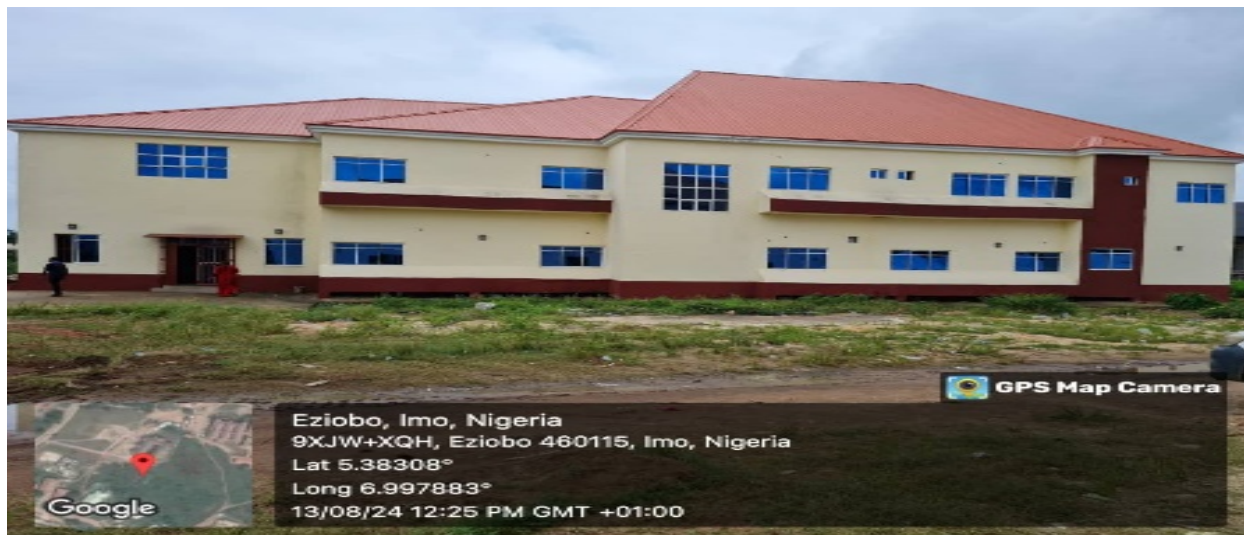
Picture 48: Completed Centre for Energy and Power Systems Research at Federal University of Technology Owerri.
