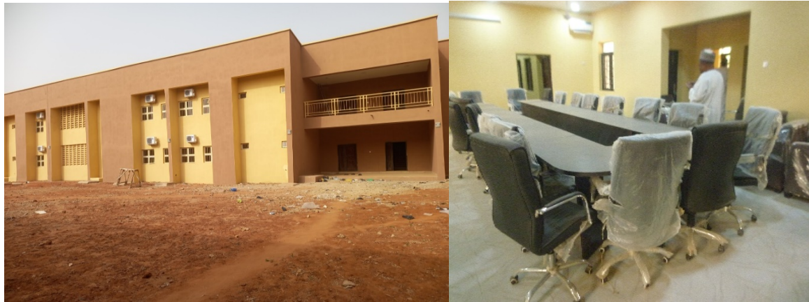
Picture 45: Constructed faculty of Veterinary Medicine at Usman Dan Fodio University, Sokoto.
