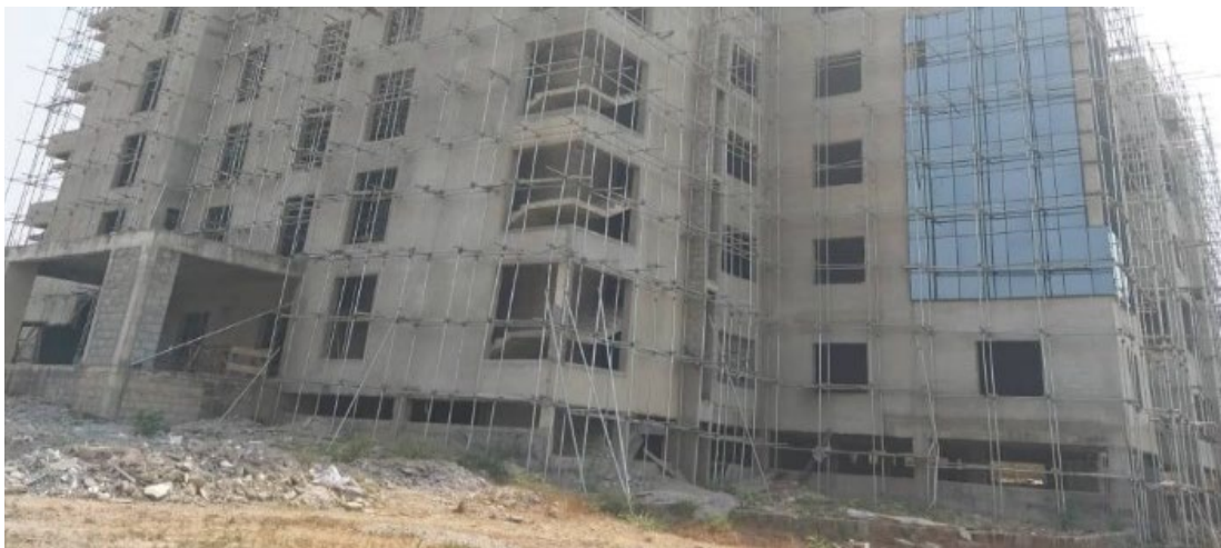
Picture 68: Ongoing construction office building at DRDB, Abuja.
