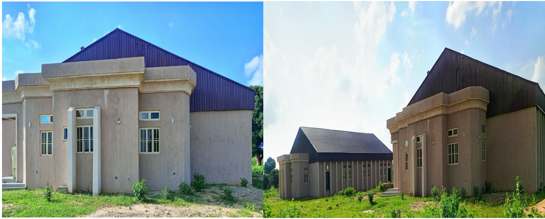
Picture 43: Constructed 200-seater CBT Centre at FCE, Jama'are.
