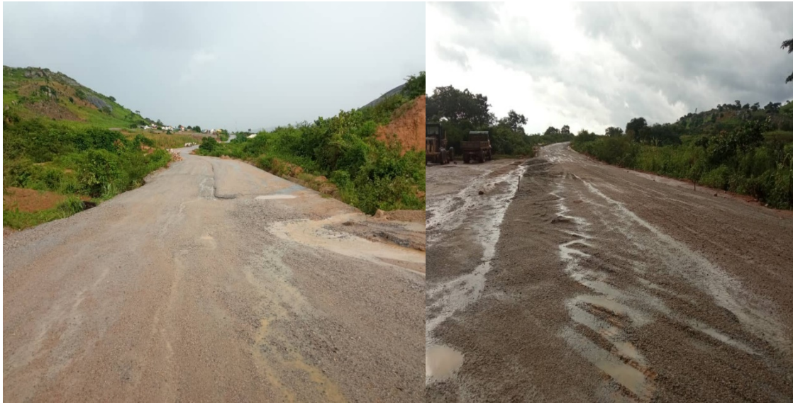
Picture 86: Ongoing Completion of 14.15km of Mpape-Guluwyi/Shere
