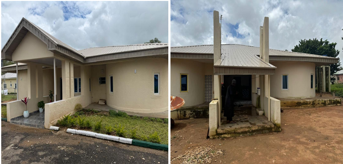
Picture 84: Renovated Participants Quarters at NIPSS, Kuru.
