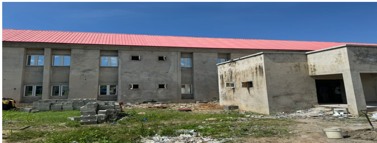
Picture 3: Ongoing Construction of Call Duty Block at UATH.
