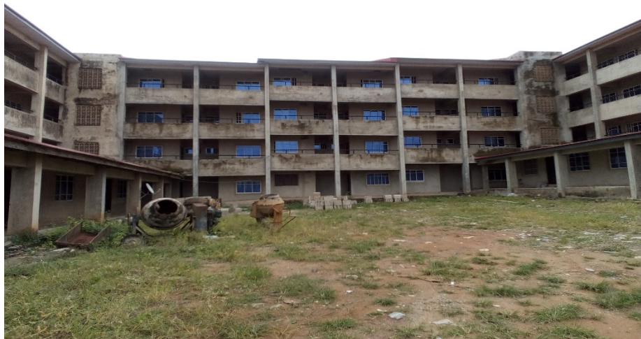
Picture 14: Ongoing construction of House Officers' building at UCH, Ibadan.
