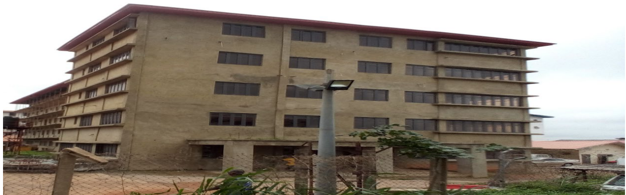
Picture 15: Construction of Accident and Emergency Clinic in UCH, Ibadan.
