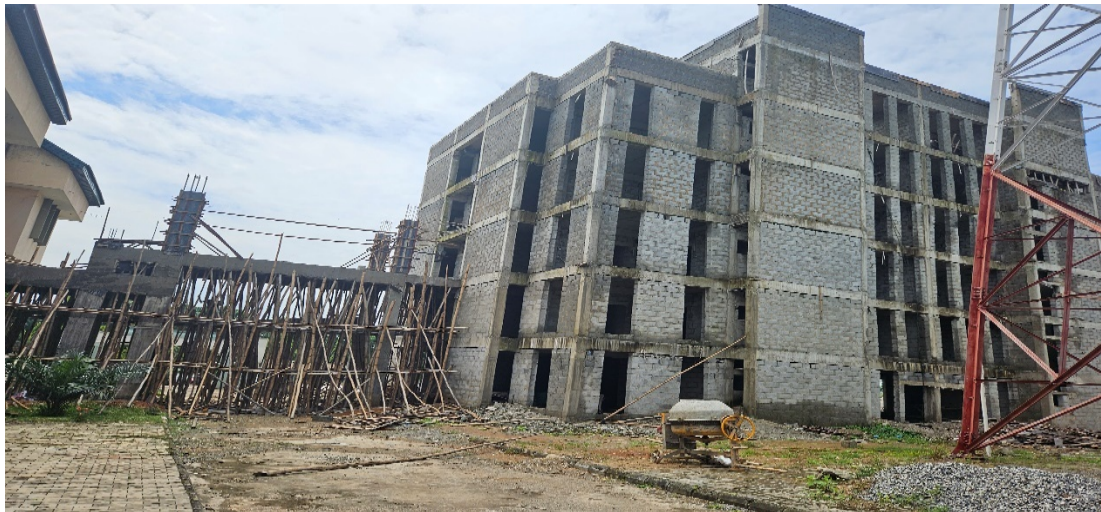
Picture 78: Ongoing Construction of ARCN Administrative Building.
