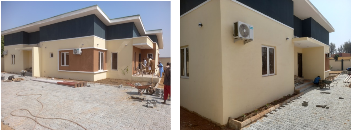
Picture 63: Completed Bursar and other quarters at NITT, Zaria.
