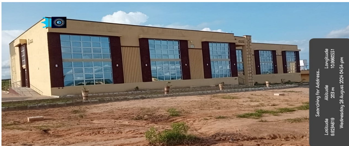
Picture 35: Completed Physiology Department at the Federal University Kashere Gombe
