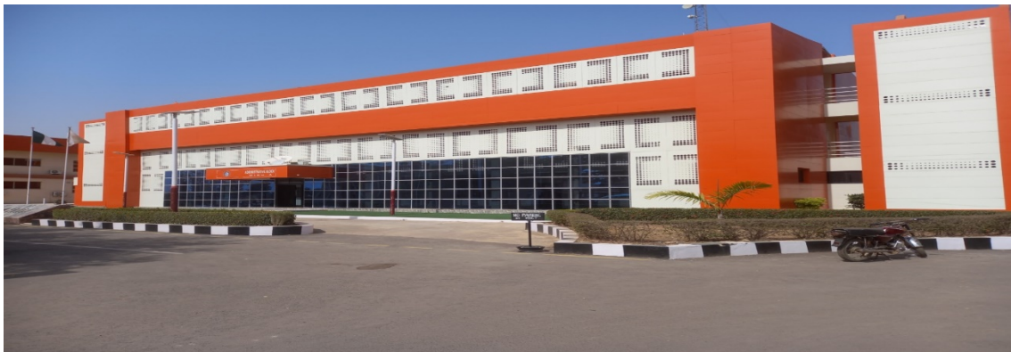
Picture 62: Completed remodelling of administrative building at NITT, Zaria.
